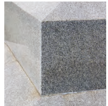
Close-up of granite
