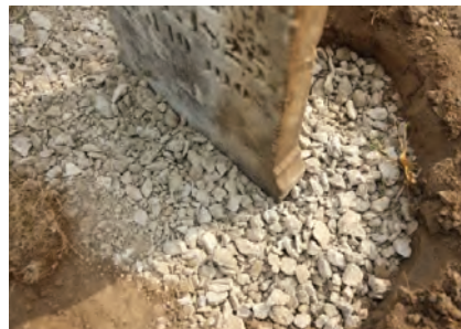
Level base of hole & add gravel
