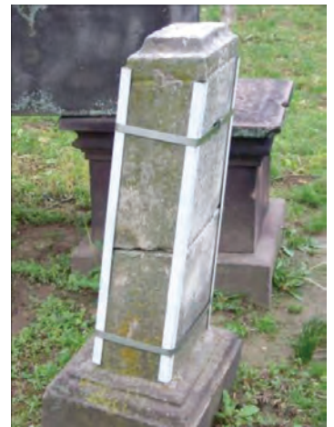
Improper repair
