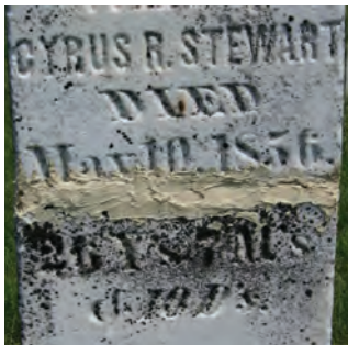
Improper repair
