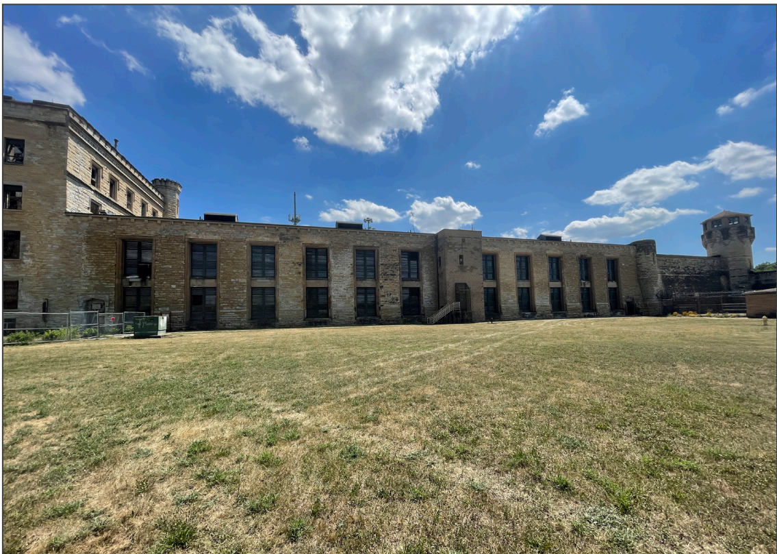
11. West Cell Block (#3), north elevation, view south.
