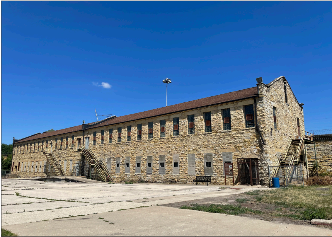
20. North Industrial Shop/Honor Dorm (#10), south elevation, view north.
