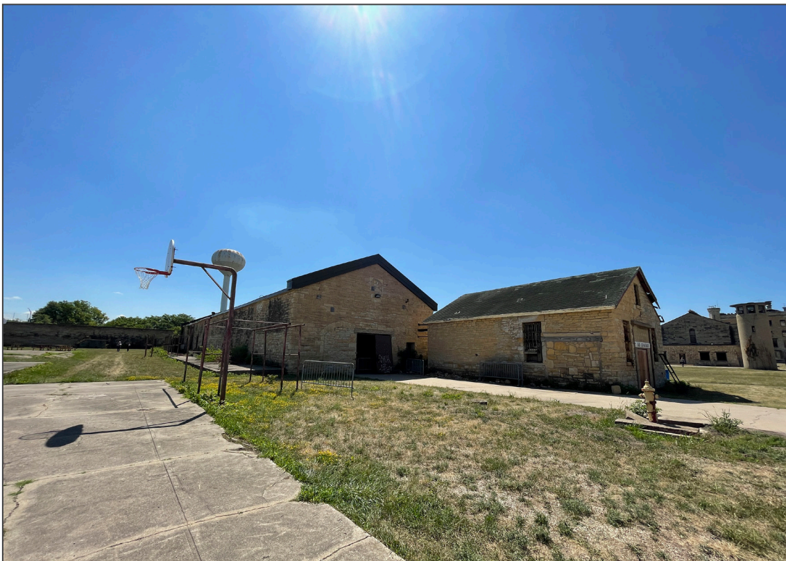
21. Mule Barn (#17) and Warehouse/Stable (#18), west and north elevations, view southeast.
