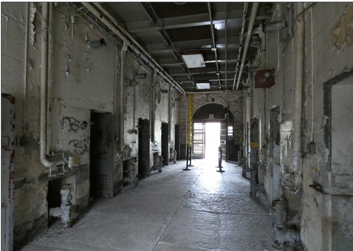
27. Separate System Prison (#15), first floor, view south to front entrance.
