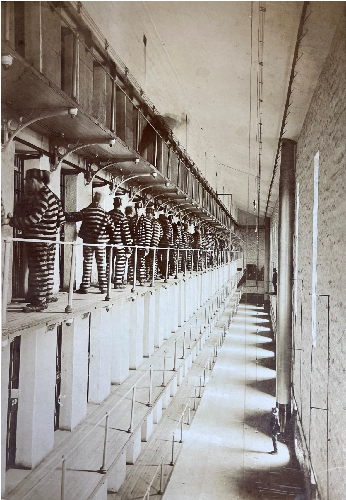
Figure 22: Joliet Penitentiary, East Cell Block, c. 1900, looking east (Joliet Area Historical Museum)
