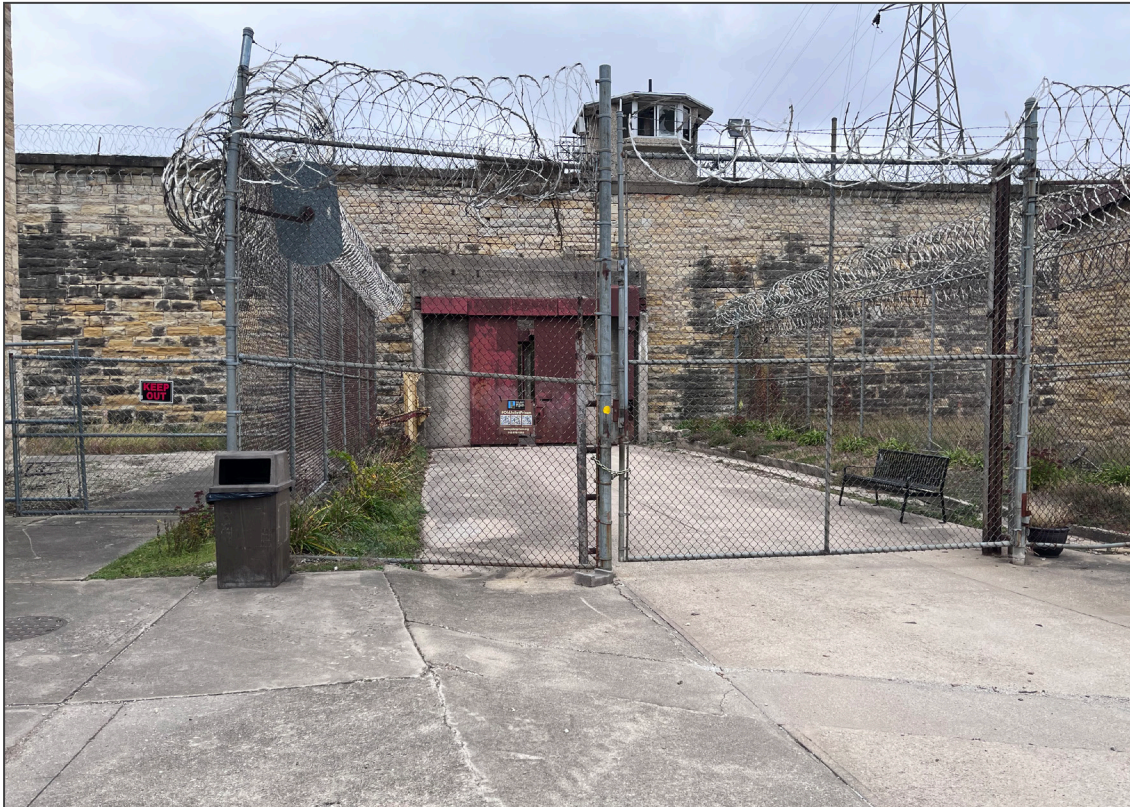
16. Gate at West Prison Wall (#30c), view west.
