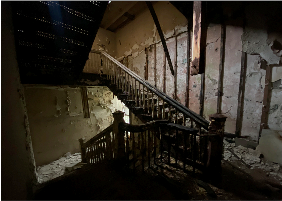
38. Women's Prison, Administration Building (#34), second floor, principal staircase.
