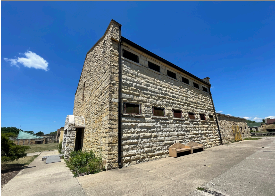
26. Separate System Prison/Solitary Building (#15), east and south elevations, view northeast.
