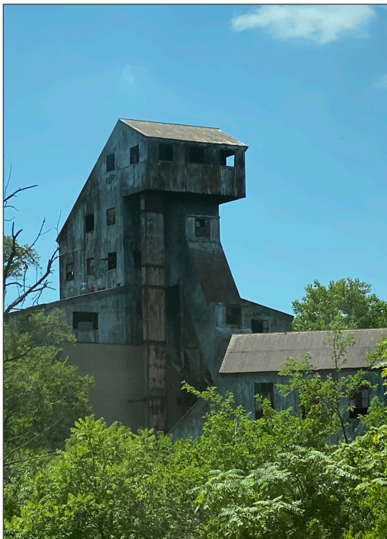
41. Quarry Crusher Plant (#47), view northwest.
