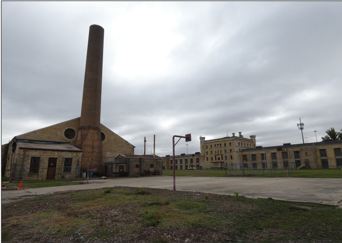
34. Prison Yard, view southeast, with Powerhouse (#13) at left and north elevations of Administration Building (#2a) and cellblocks (#3 and #29) center-right.
