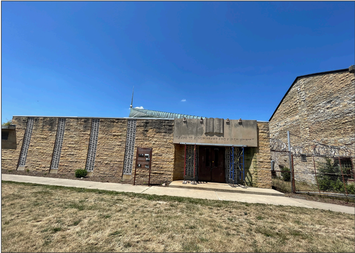
14. Chapel (#6), front façade, view west.
