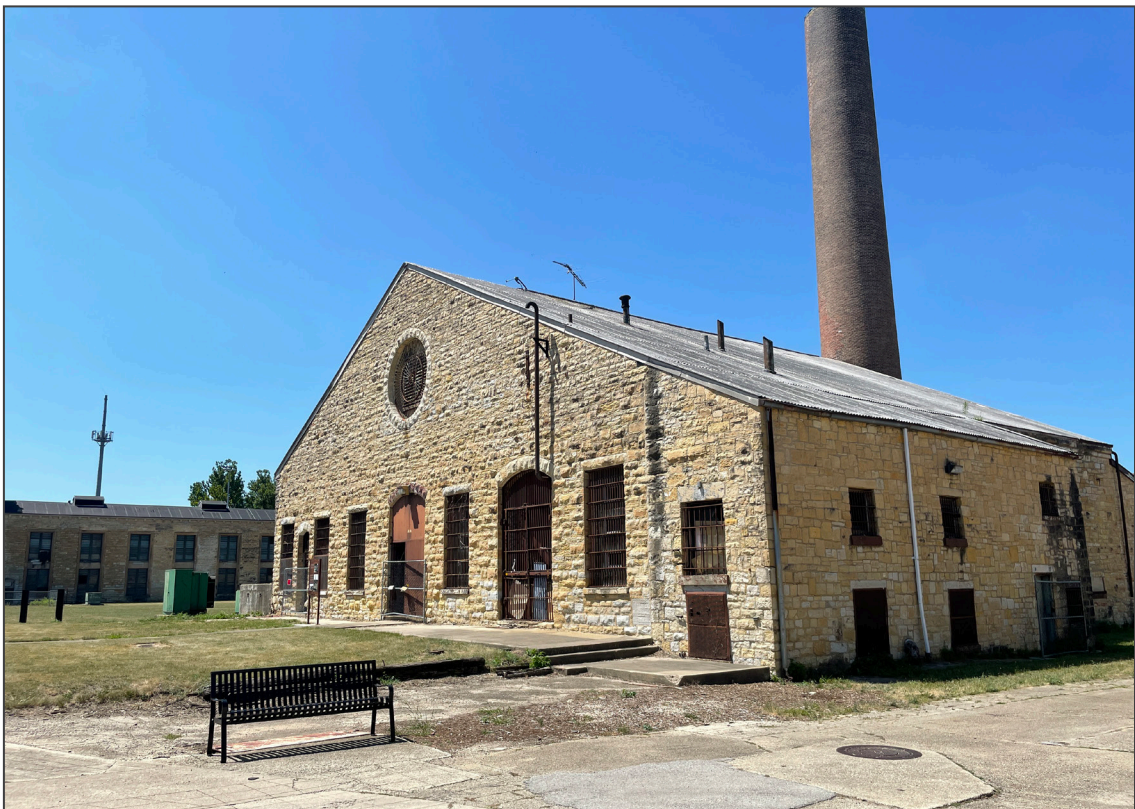
15. Powerhouse (#13), south and east elevations, view northwest.
