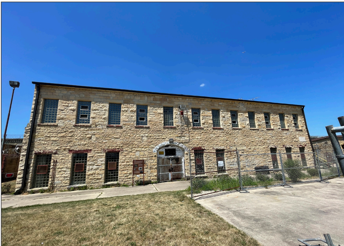
17. Center-West Industrial Shop (#7), east elevation, view west.
