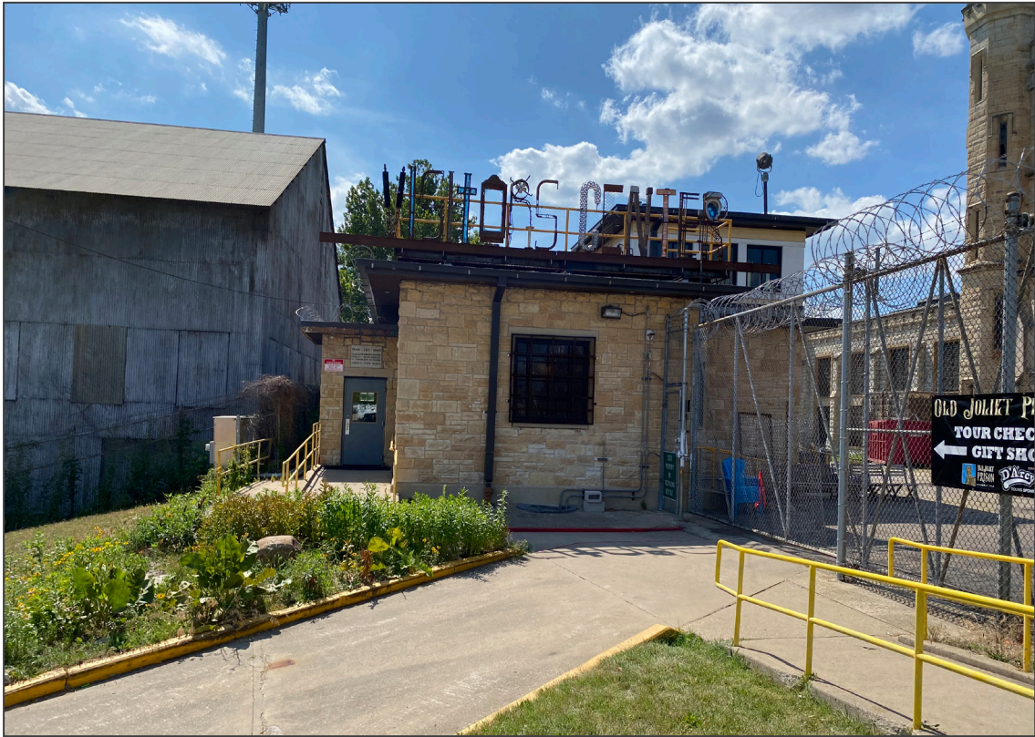
1. Gate House (#1), view west.
