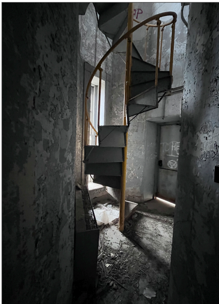
9. Administration Building (#2a), southwest turret interior, view southwest.
