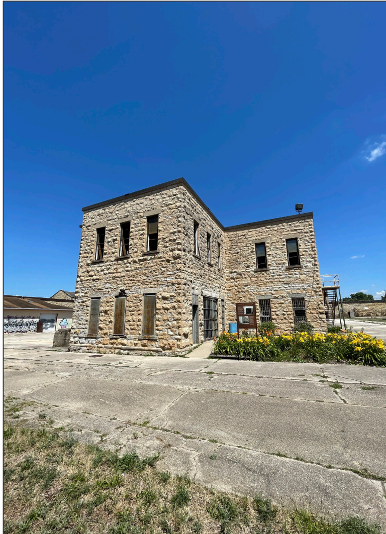
25. Fire House (#11), south and east elevations, view northwest.
