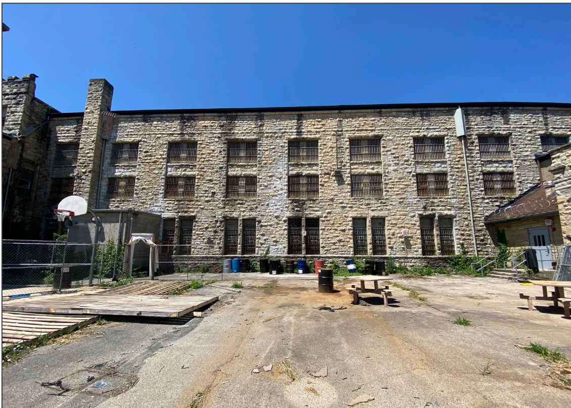
37. Women's Prison, Cellblock (#35), east elevation, view west.
