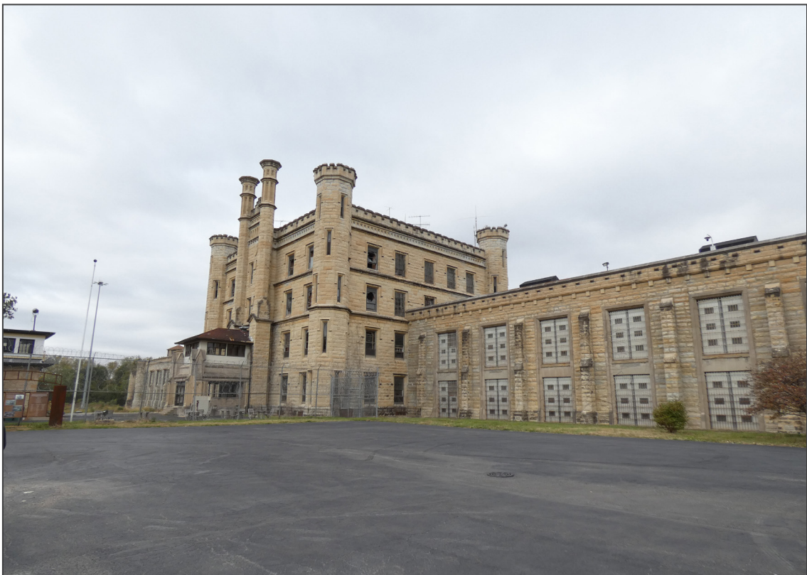
2. Administration Building (#2) and East Cellblock Wing (#29, partial), view northwest.
