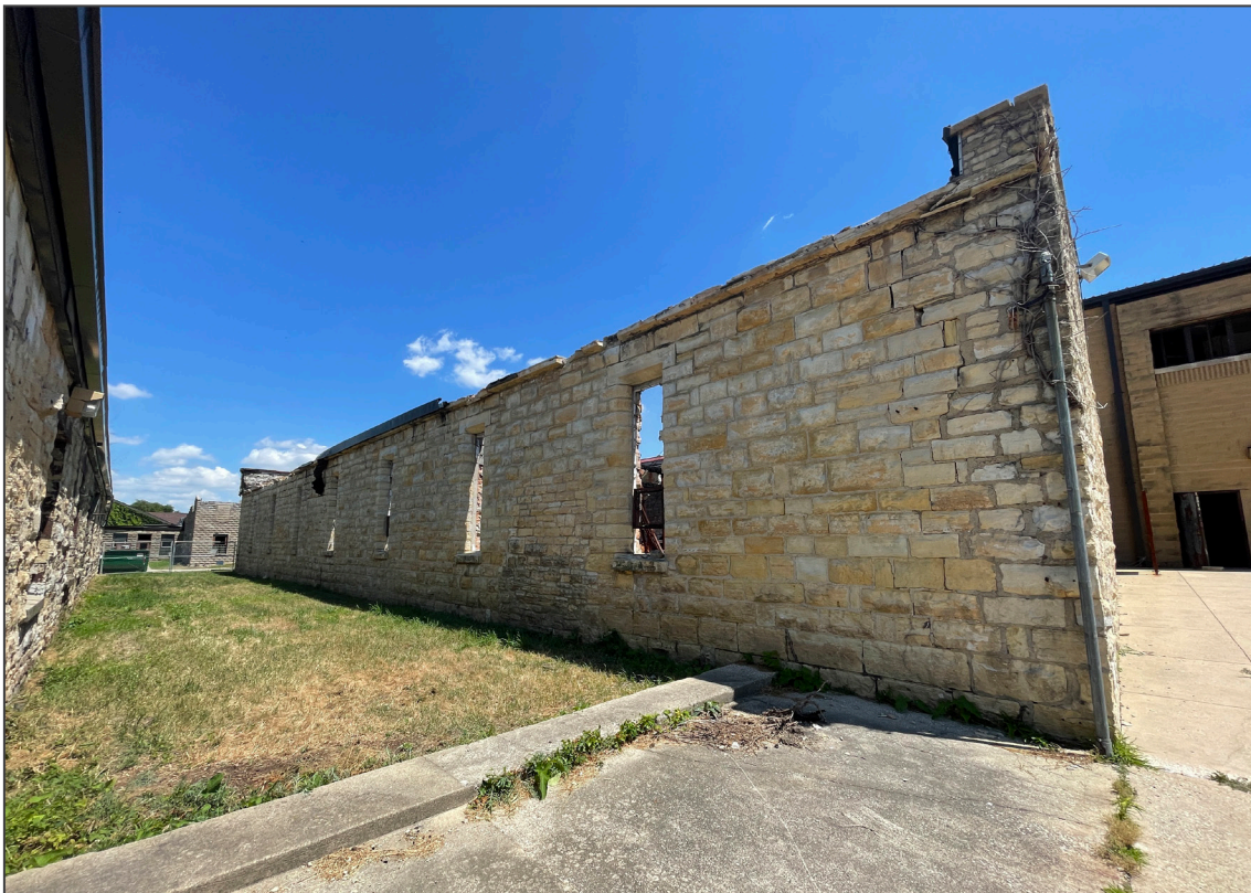
29. Women's Cellblock /Clothing Department/Bath House (#24), west elevation, view north-east.
