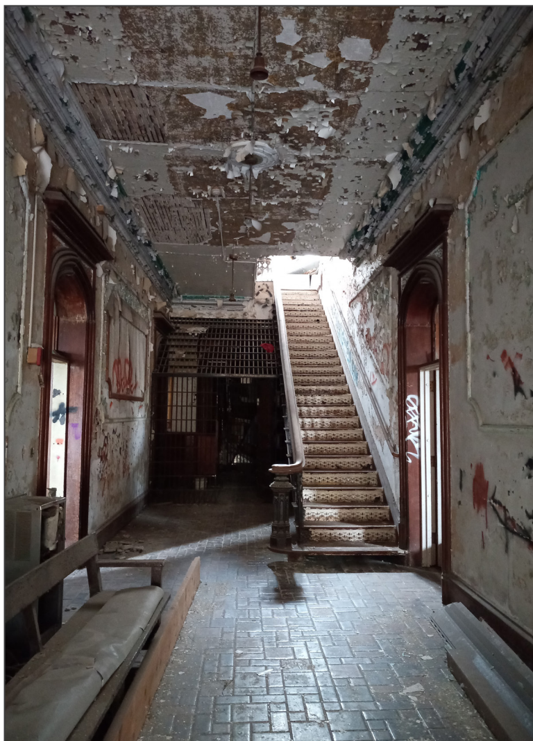
6. Administration Building (#2), first floor, hallway and staircase, view north.
