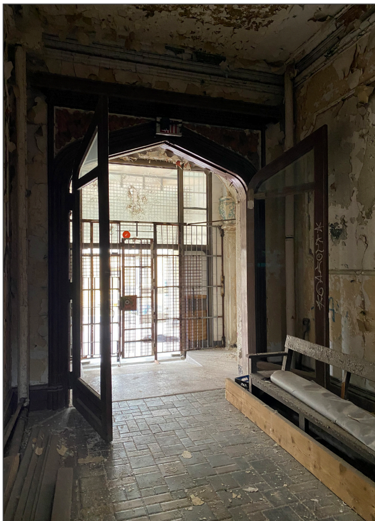
5. Administration Building (#2), first floor, view south from hallway to vestibule.
