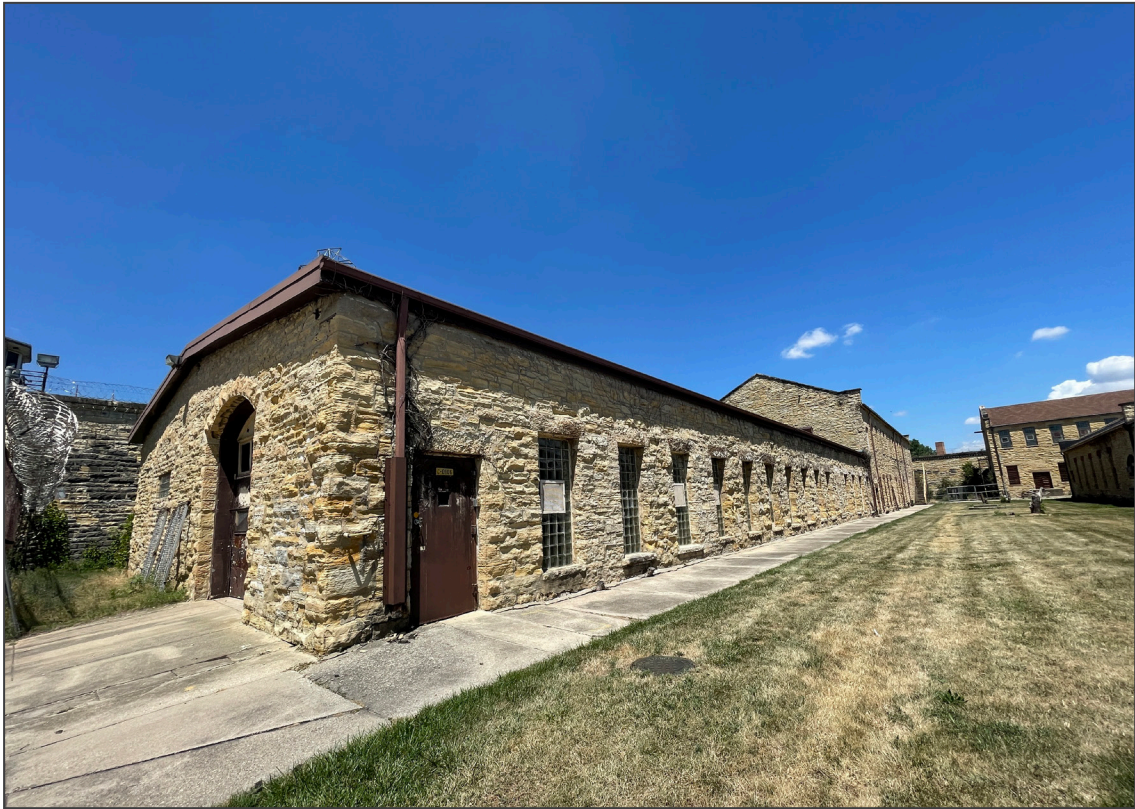
18. Northwest Industrial Shop (#8), south and east elevations, view northwest.
