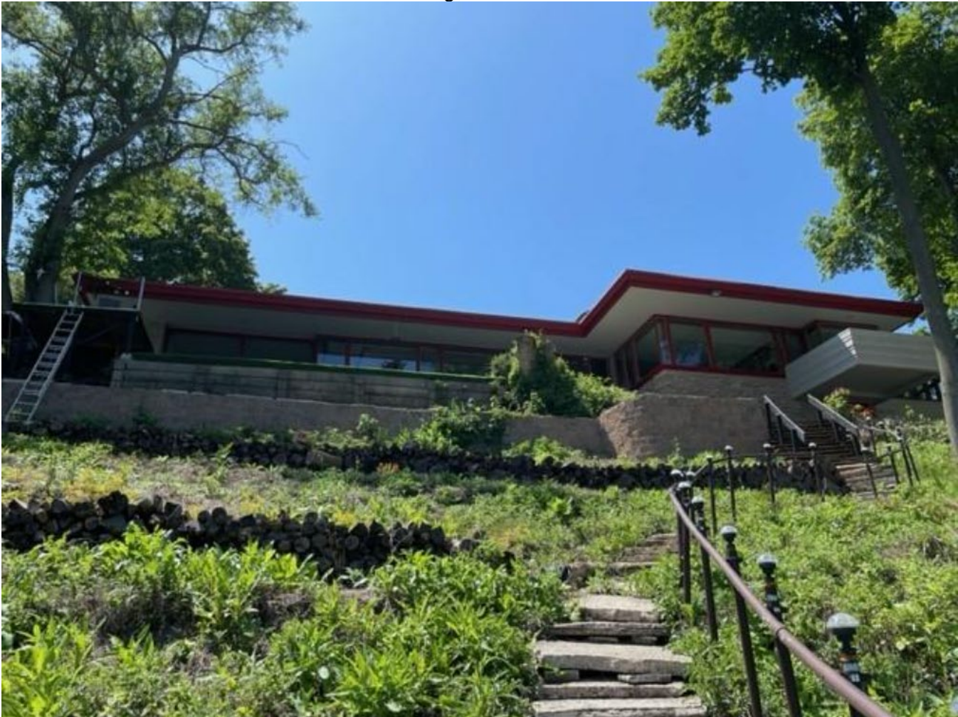
Photo 7 of 13: Back of the house, camera facing west.
