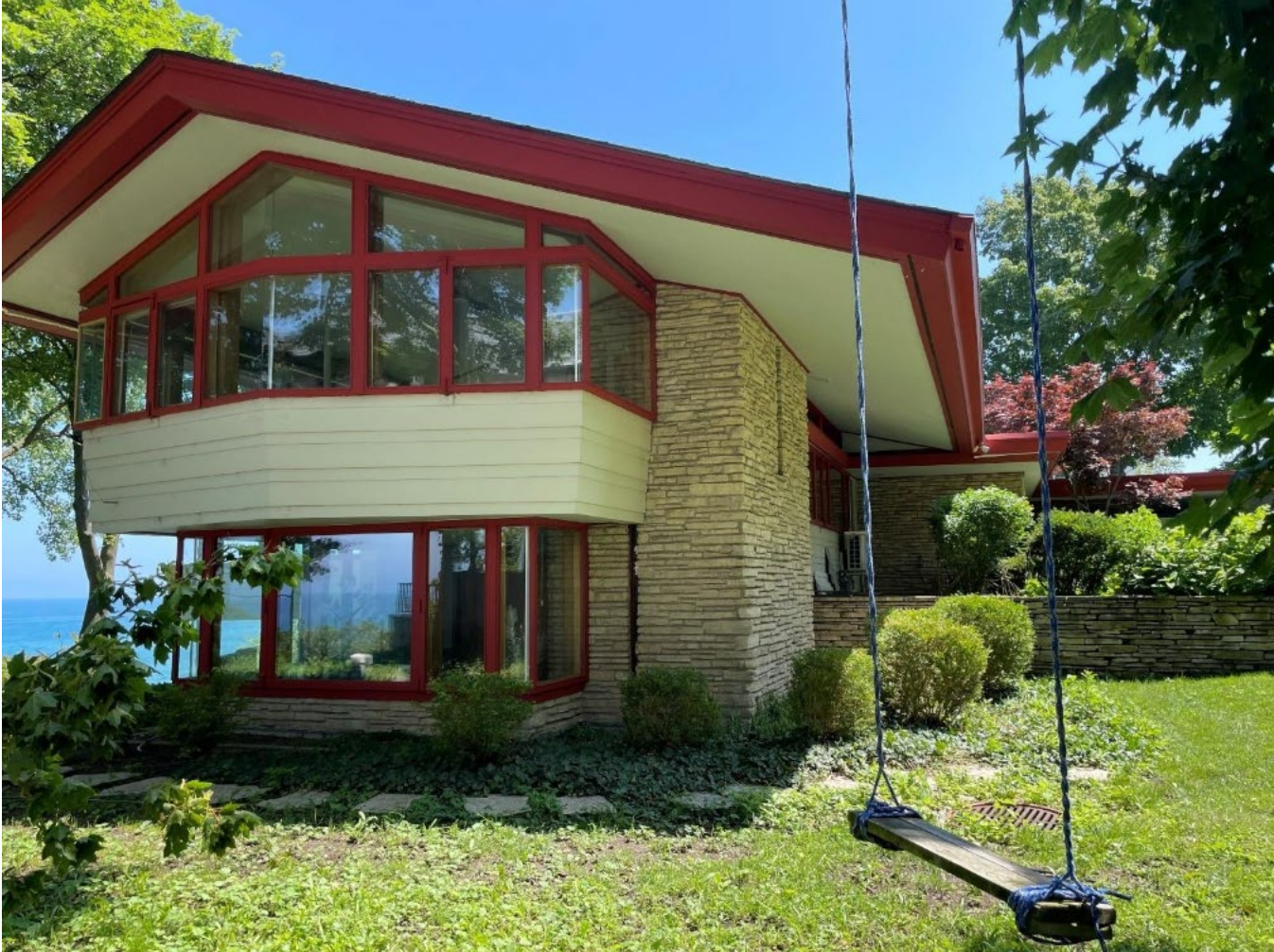
Photo 5 of 13: North side of the house, camera facing south and slightly east.
