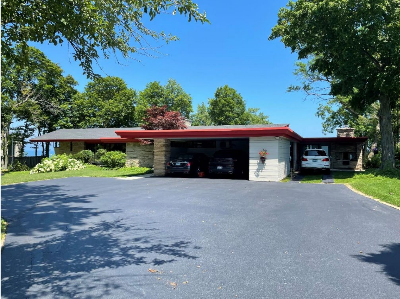
Photo 2 of 13: Approach and carport, camera facing east.
