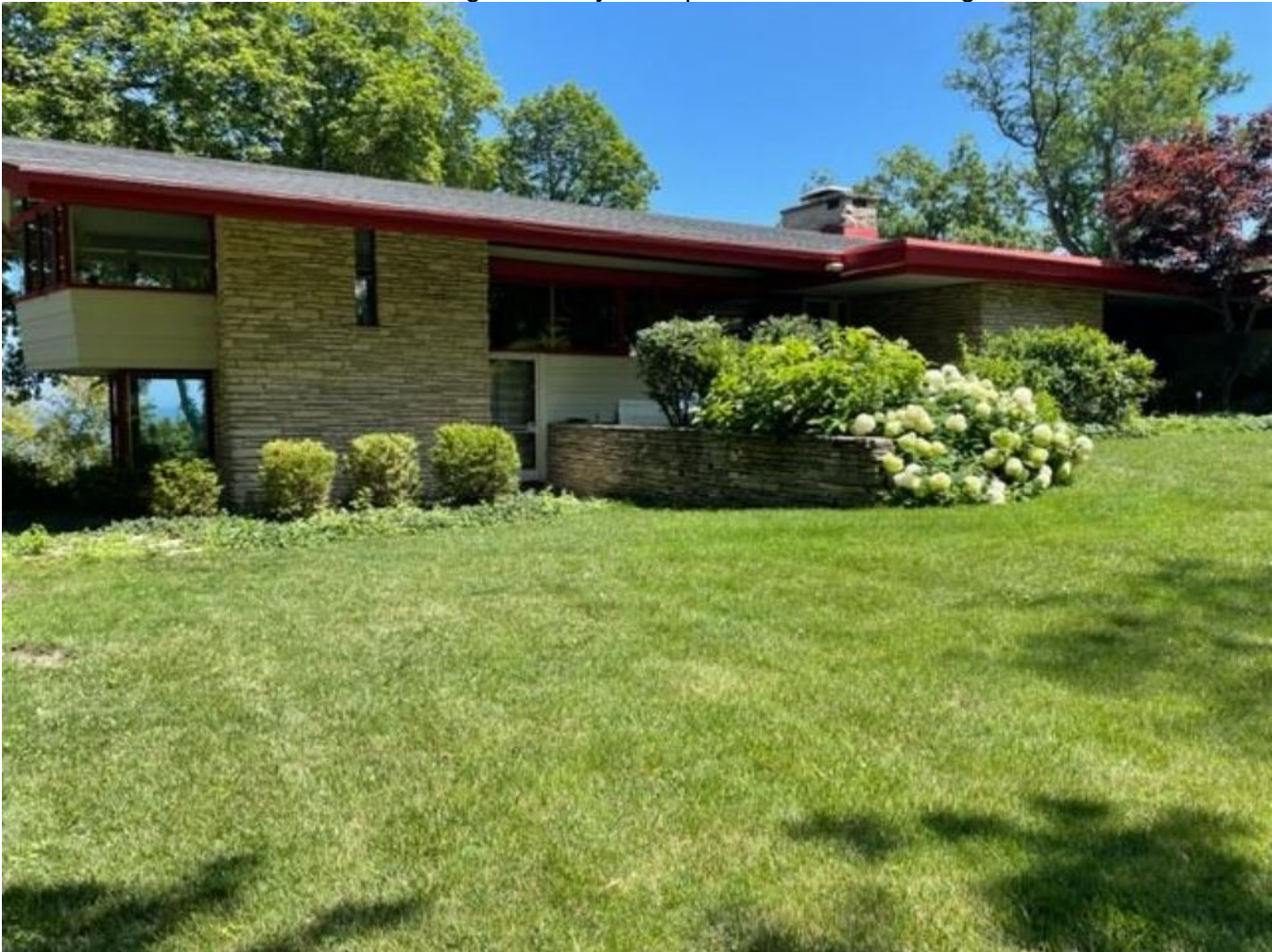
Photo 4 of 13: Front of house showing clerestory and split-level, camera facing east.
