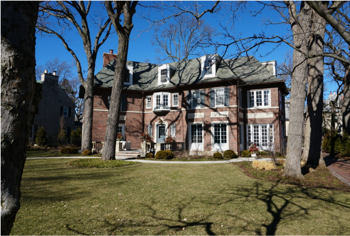
0001 of 35: Front façade looking northwest.
