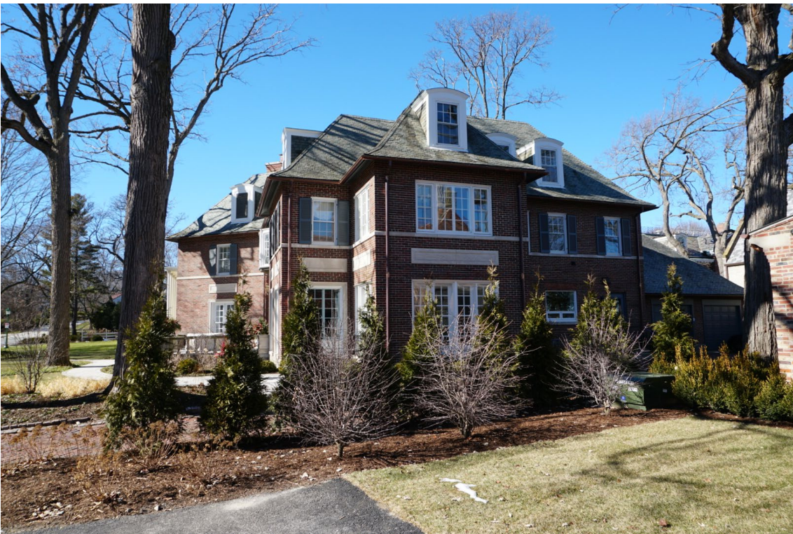
0002 of 35: East façade looking west.
