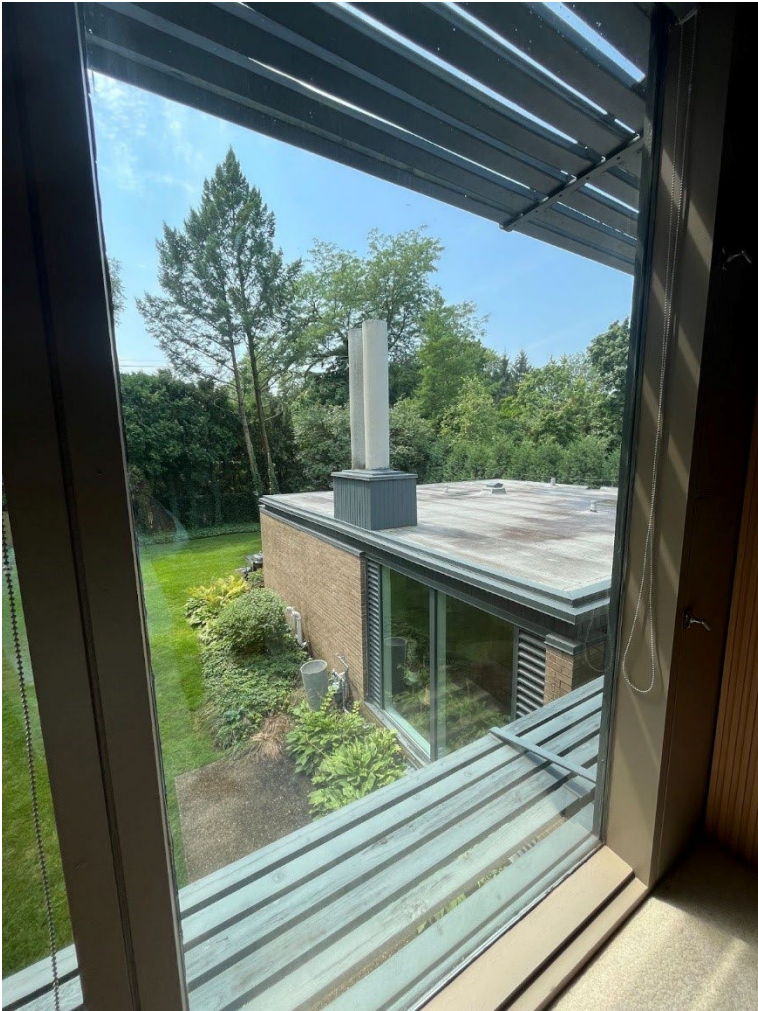
View of Chimney Stack, camera facing southwest
