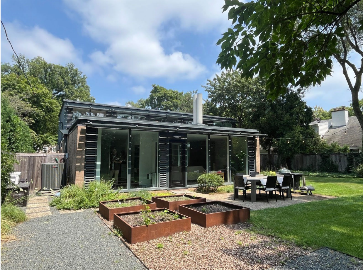
South (Rear) Wing South Elevation, camera facing northeast
