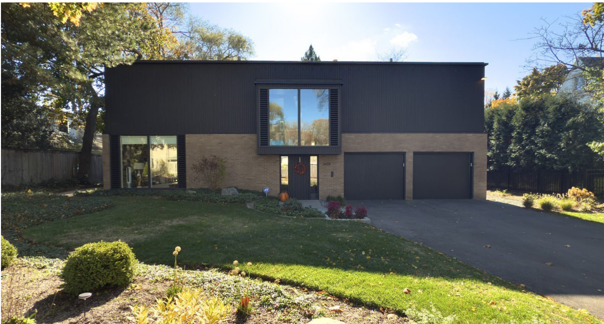
North Elevation, camera facing south
