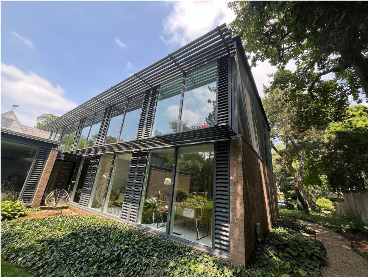
North (Front) Wing South and East Elevation, camera facing northwest
