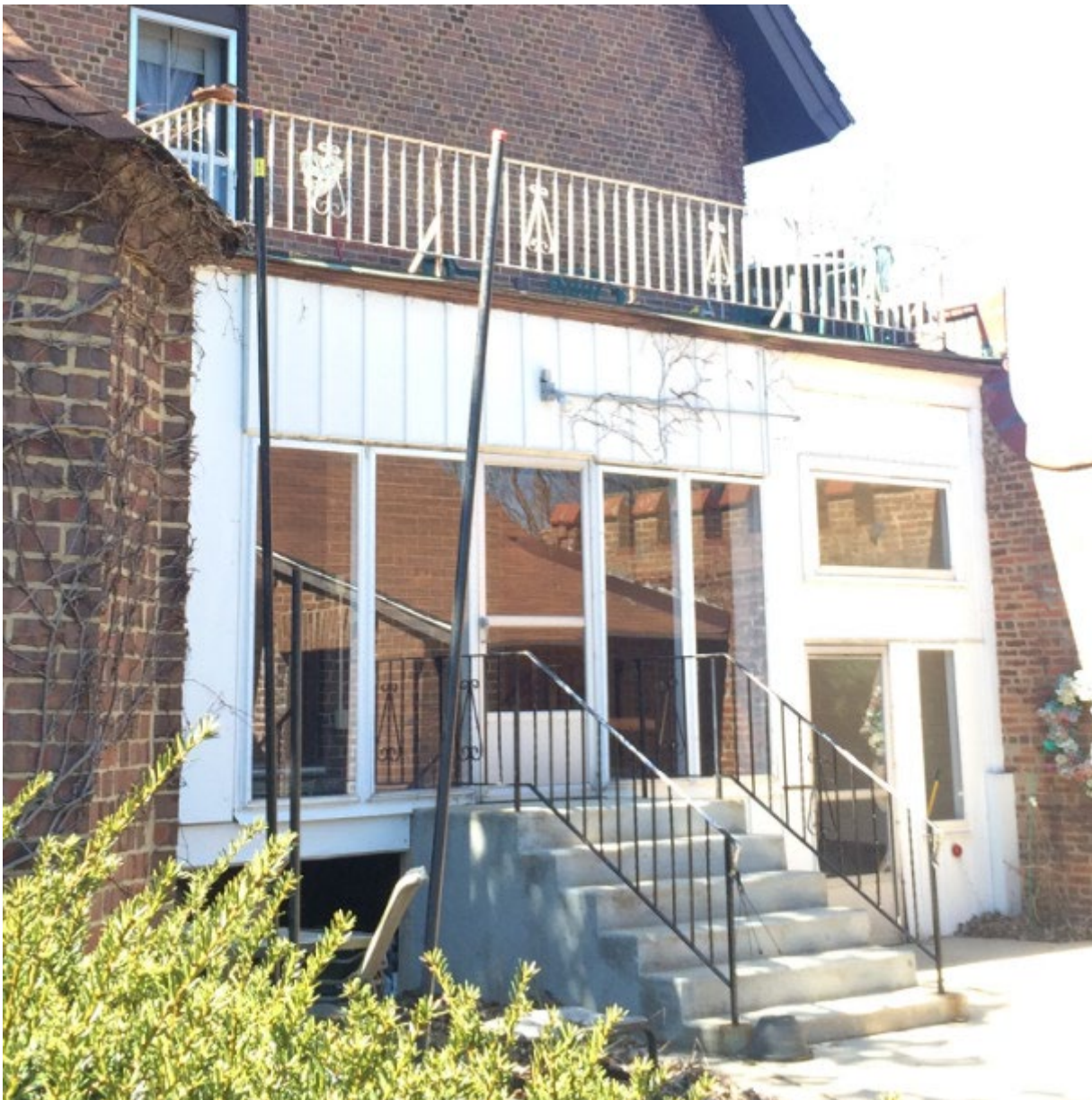
Figure 10: East porch (not original) removed during relocation.
