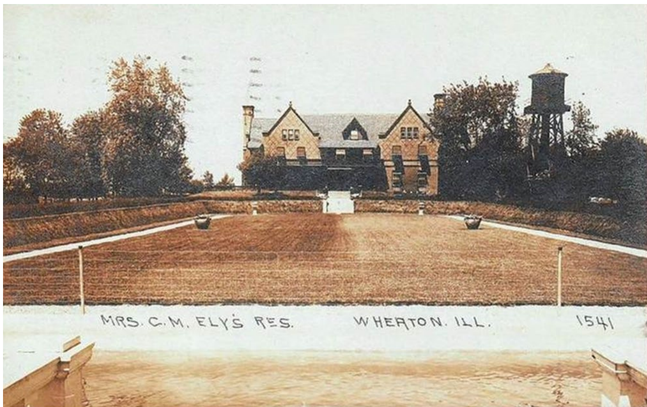
Figure 4: Historic photograph showing the south elevation.
