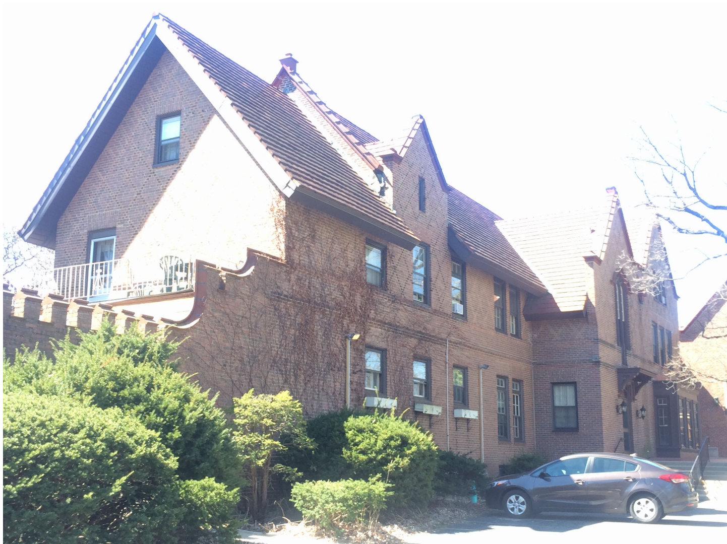
Figure 8: House prior to move. East wall jutting out at northeast corner (not original) was removed.
