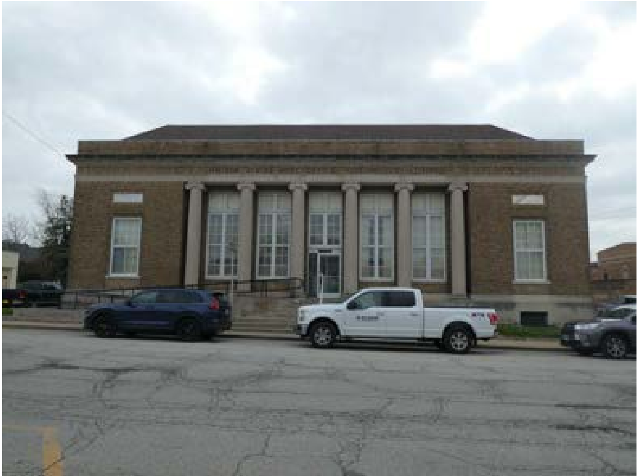
Photo 35: Building 81 facing east
