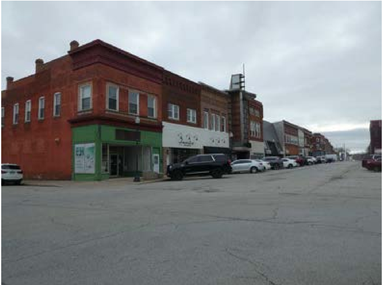
Photo 3: Buildings 8-15 facing northeast
