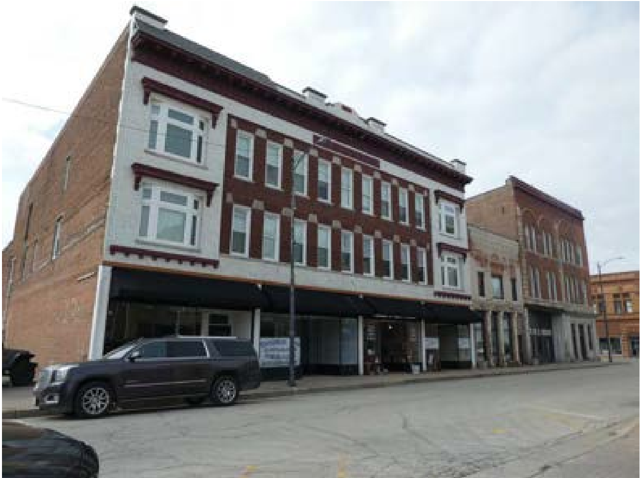
Photo 29: Buildings 70-72 facing southwest
