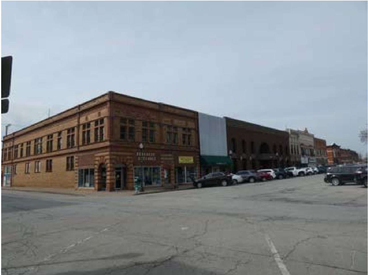
Photo 27: Buildings 65-69 facing southwest
