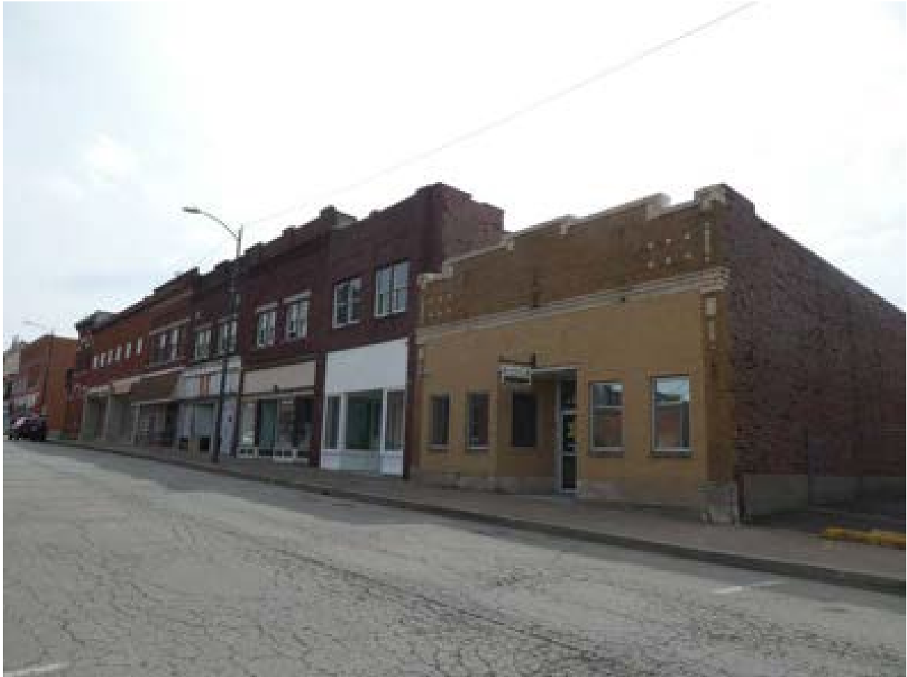
Photo 25: Buildings 58-64 facing southeast
