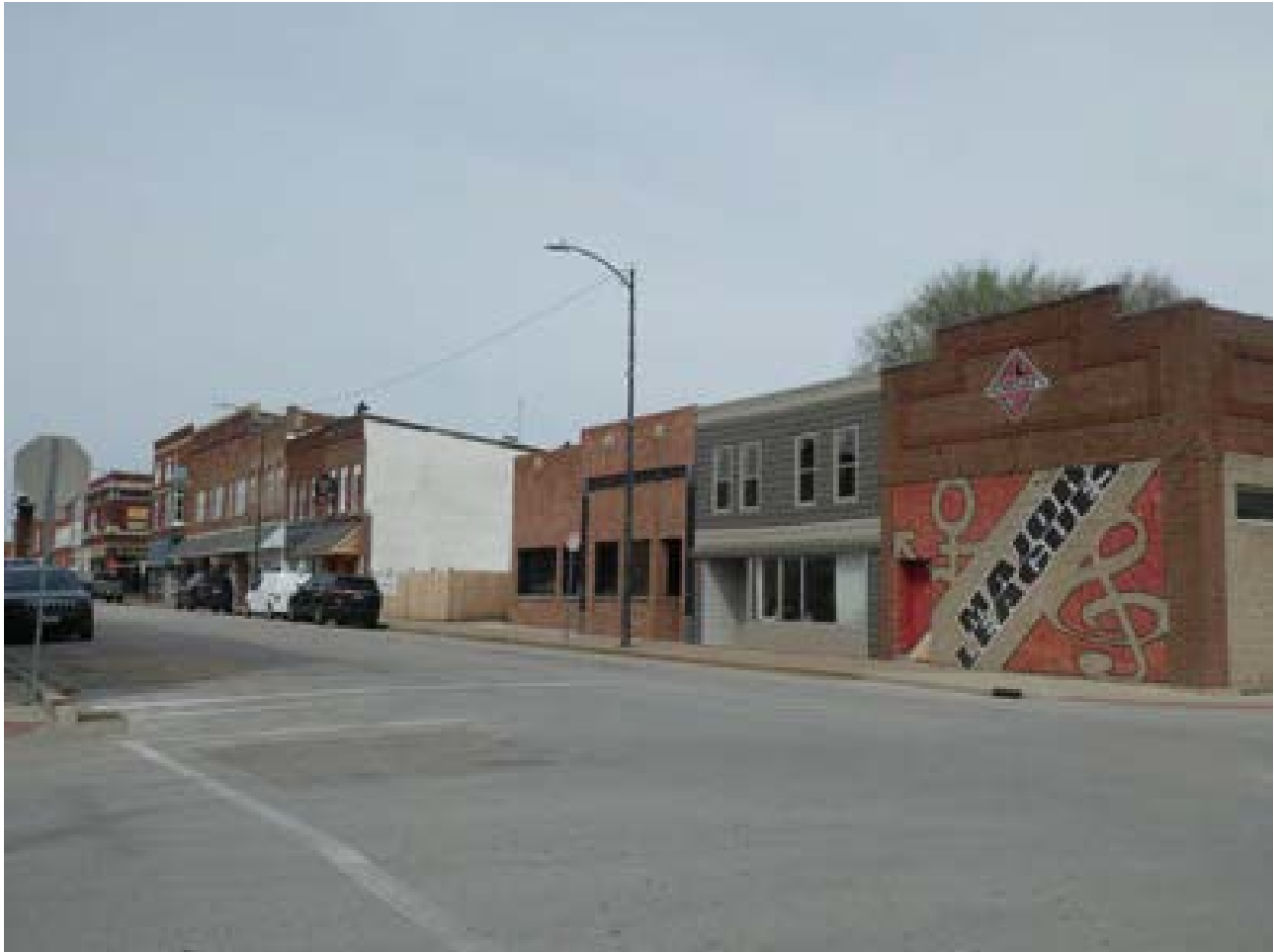
Photo 7: Buildings 17-24 facing northwest
