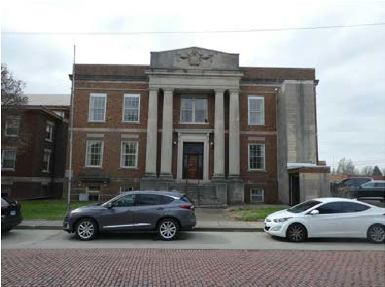
Photo 36: Building 82 facing south
