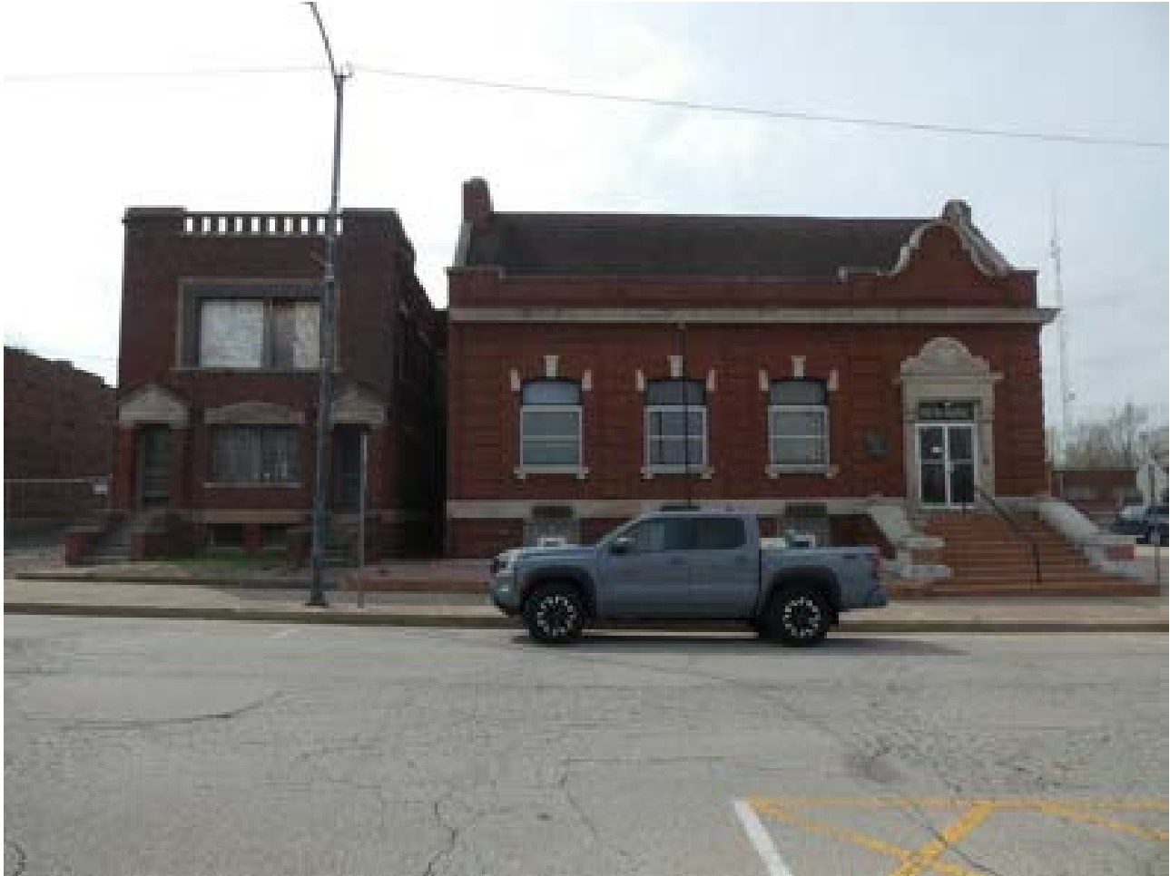
Photo 24: Buildings 56 and 57 facing south
