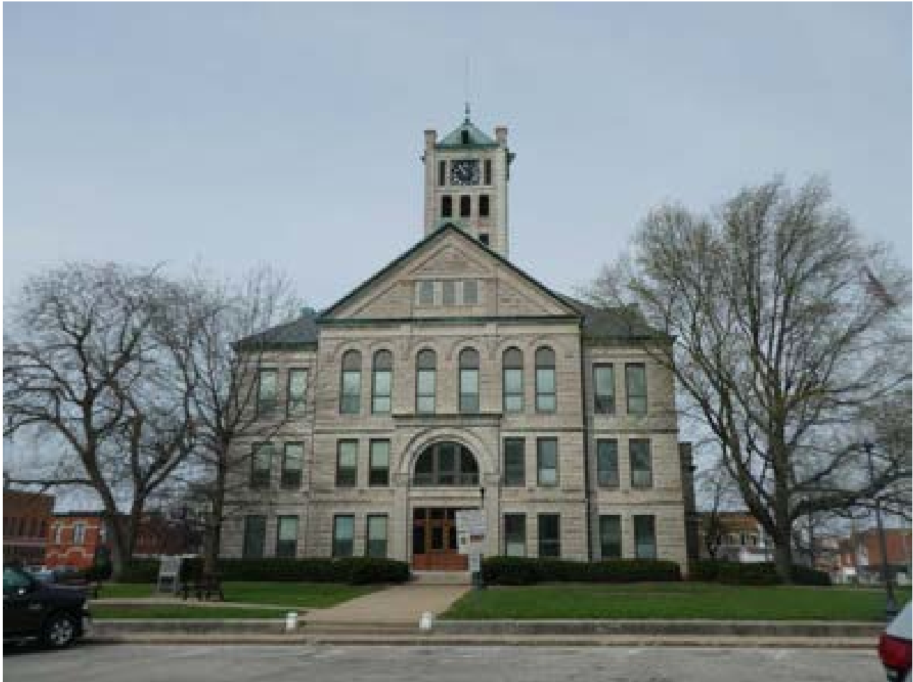
Photo 20: Building 45 facing west
