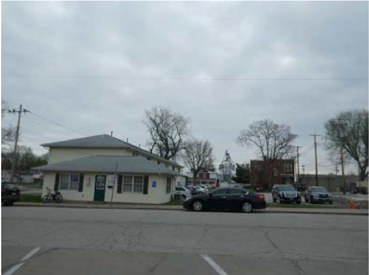
Photo 10: Building 28 facing east (Demolished and Replaced)
