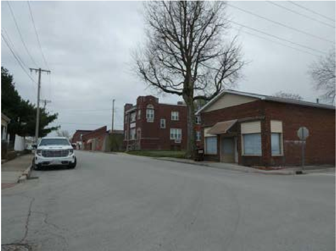
Photo 8: Buildings 24-27 facing southwest (Building 26 - Mid-Block - Demolished)
