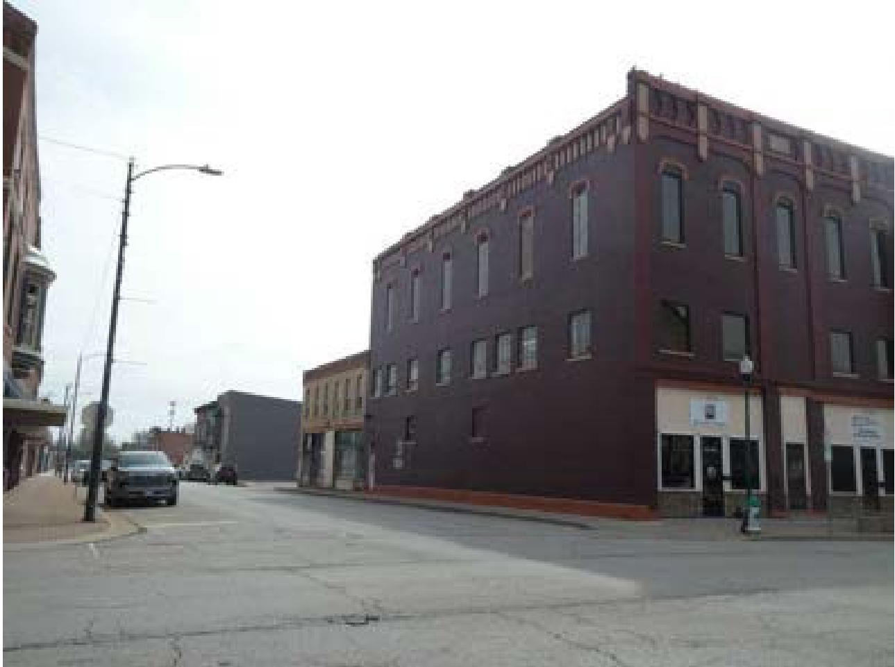
Photo 13: Buildings 31-33 facing southeast
