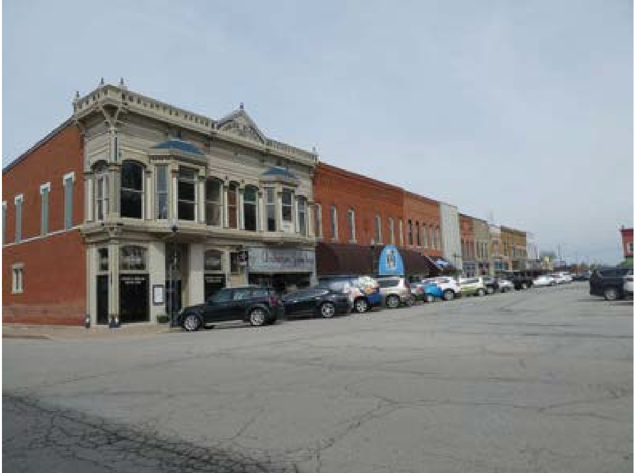
Photo 22: Buildings 46-54 facing northwest
