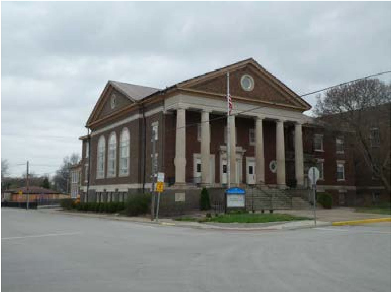
Photo 37: Building 83 facing southwest
