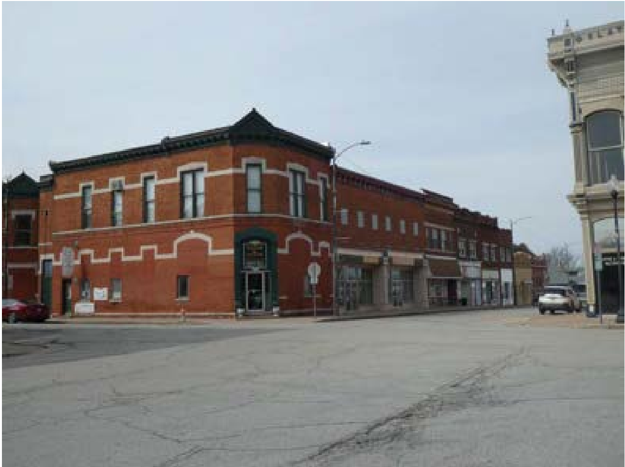
Photo 26: Buildings 56-64 facing southwest
