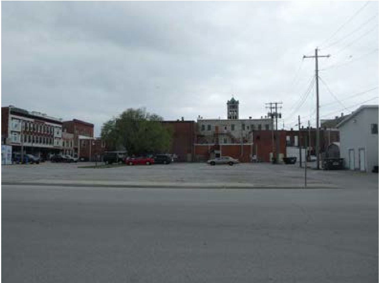
Photo 16: Building 35 facing west (Demolished)
