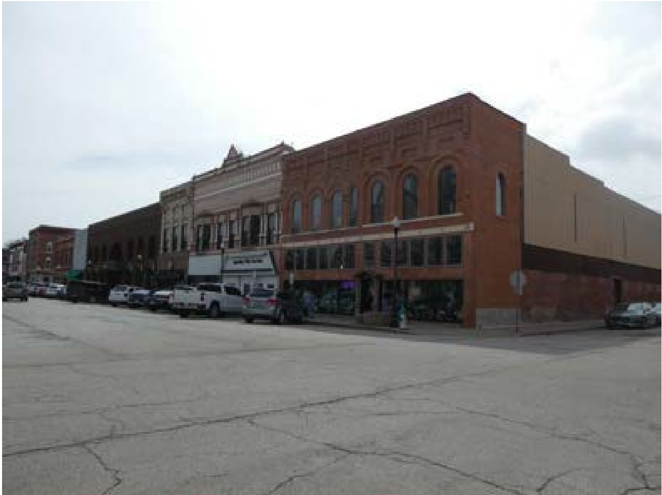
Photo 28: Buildings 65-69 facing southeast
