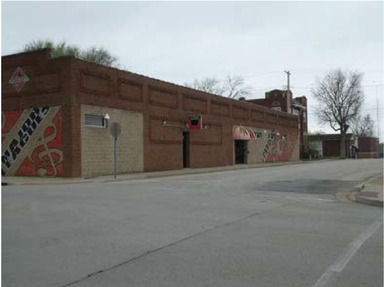
Photo 9: Buildings 24-27 facing northwest
