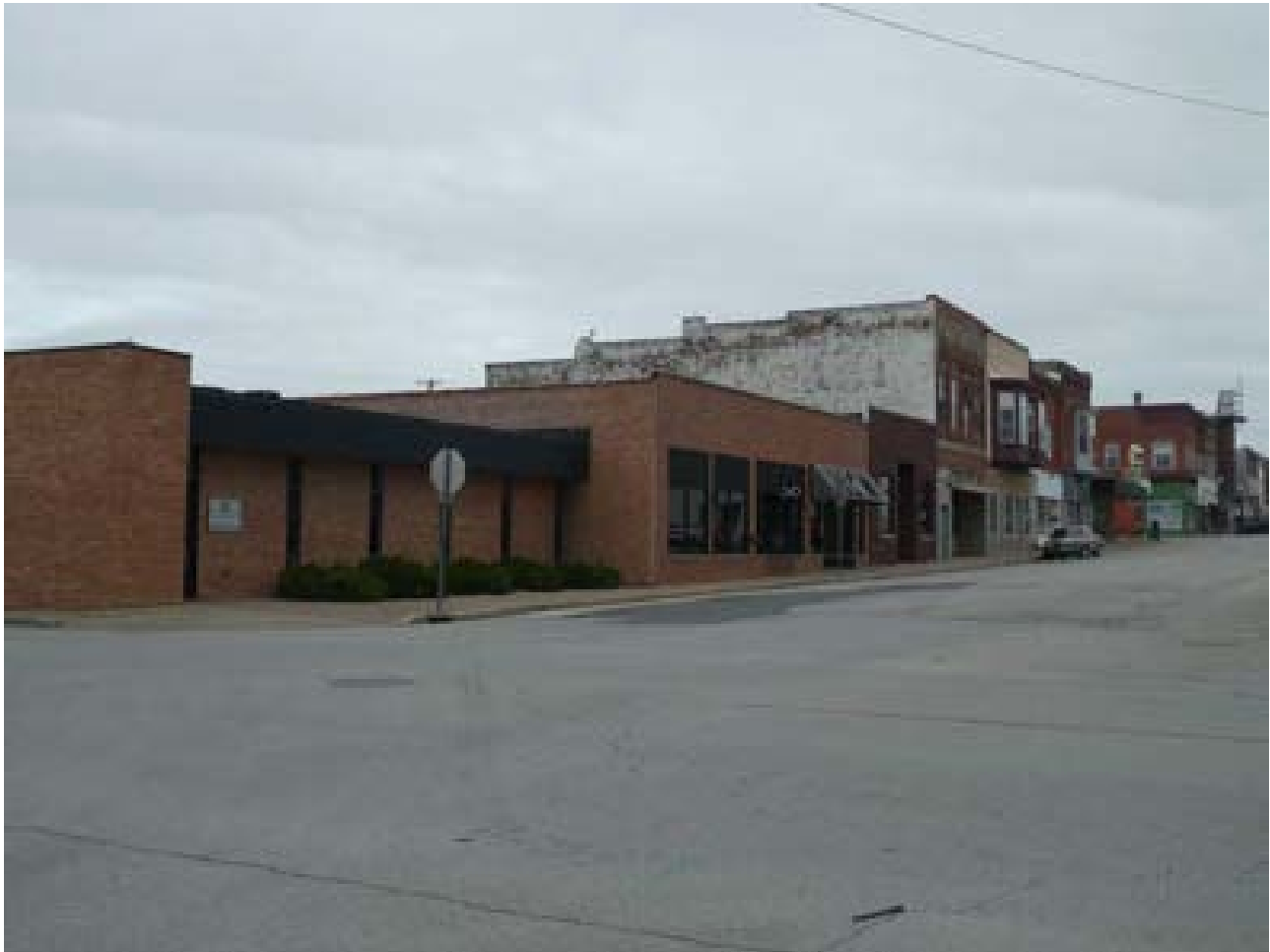
Photo 1: Buildings 1-7 facing northeast
