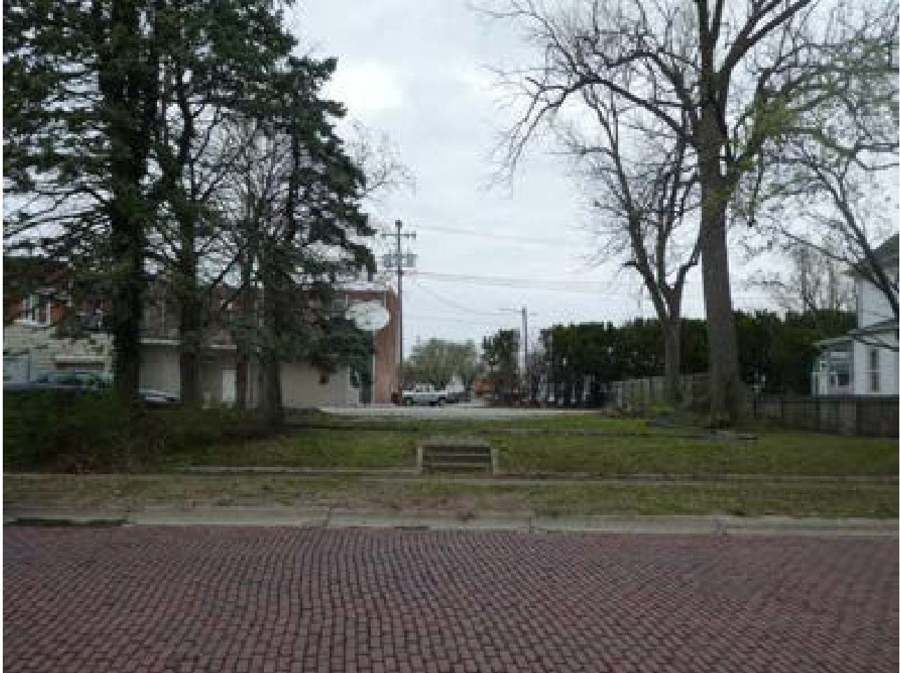
Photo 32: Building 75 facing north (Demolished)
