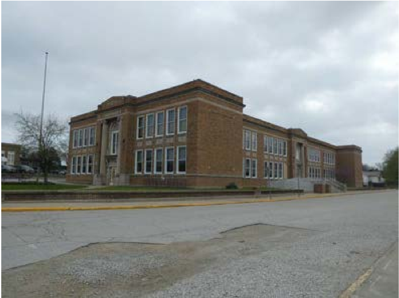
Photo 38: Building 84 facing northeast
