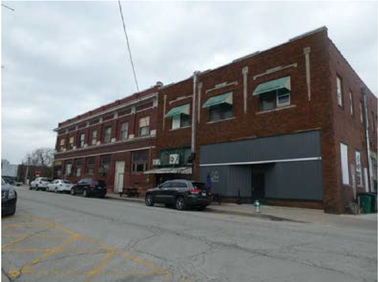
Photo 5: Building 16 facing southwest
