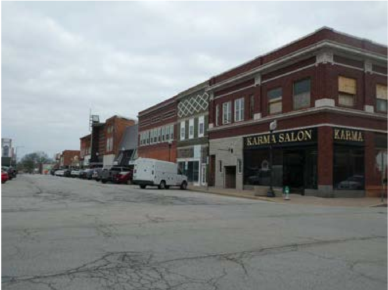
Photo 4: Buildings 8-15 facing northwest
