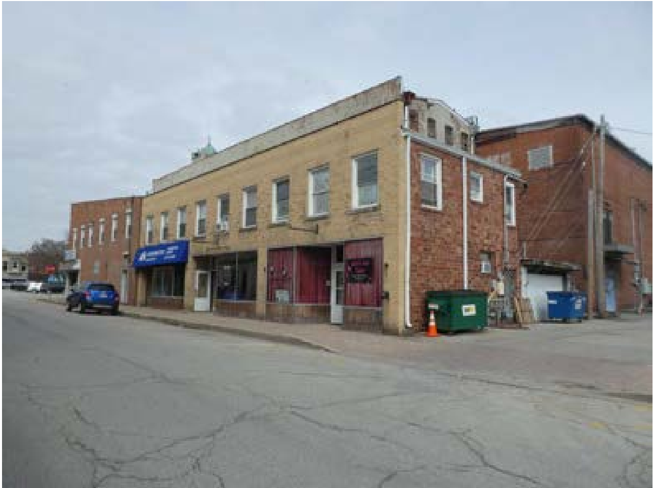
Photo 17: Building 36 facing northwest
