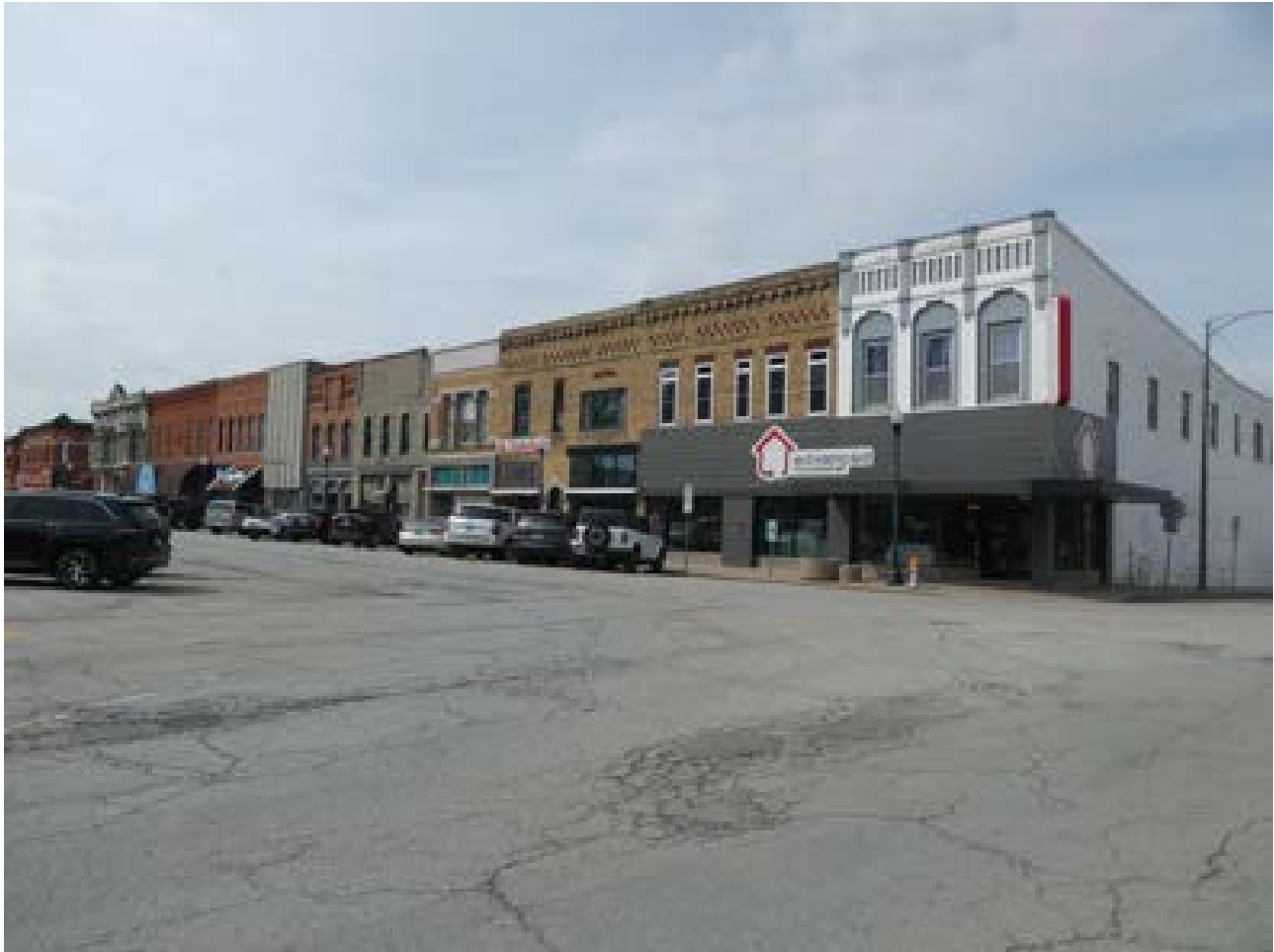
Photo 21: Buildings 46-54 facing southwest
