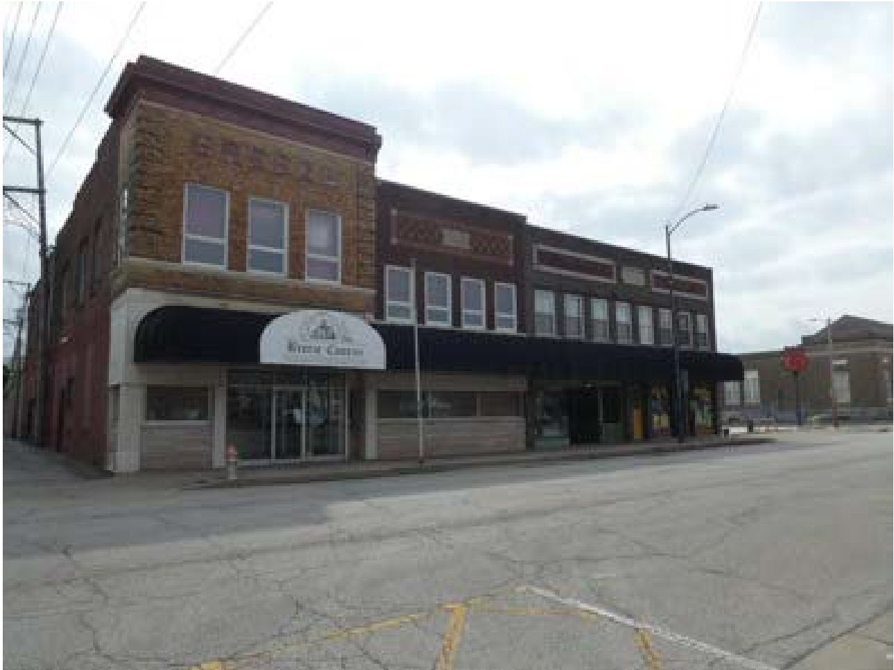
Photo 33: Buildings 76-79 facing southeast
