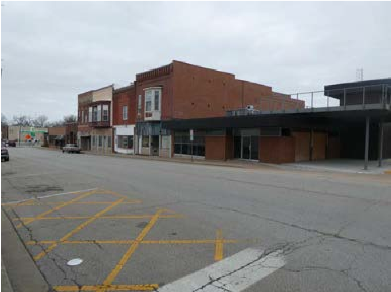
Photo 2: Buildings 1-7 facing northwest
