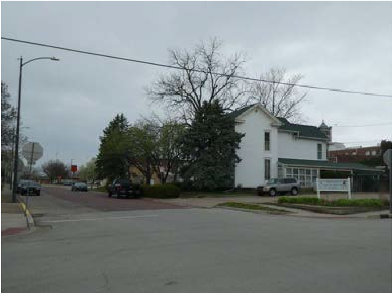
Photo 31: Building 74 facing northwest
