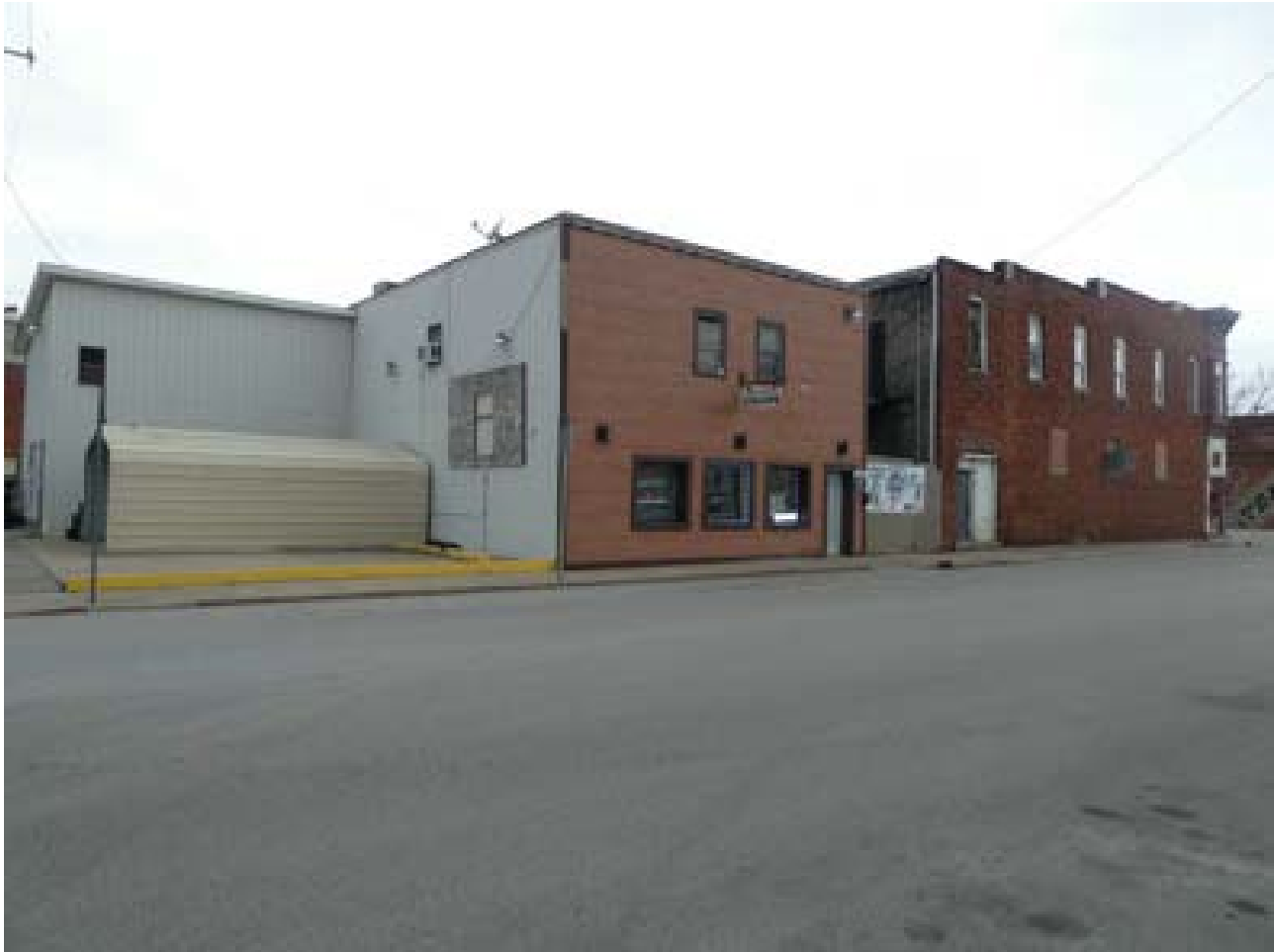
Photo 15: Building 34 facing northwest
