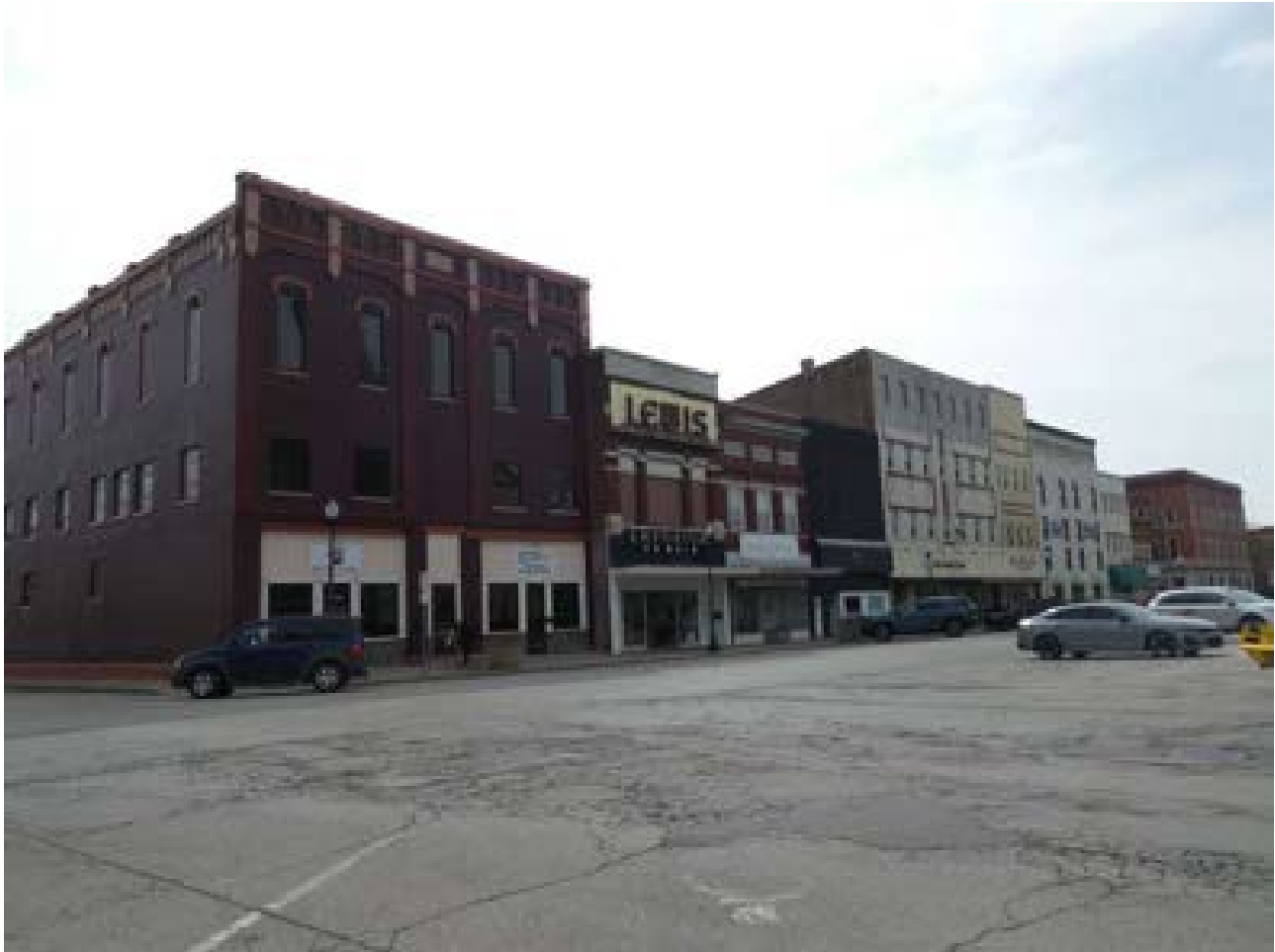
Photo 19: Buildings 37-44 facing southeast
