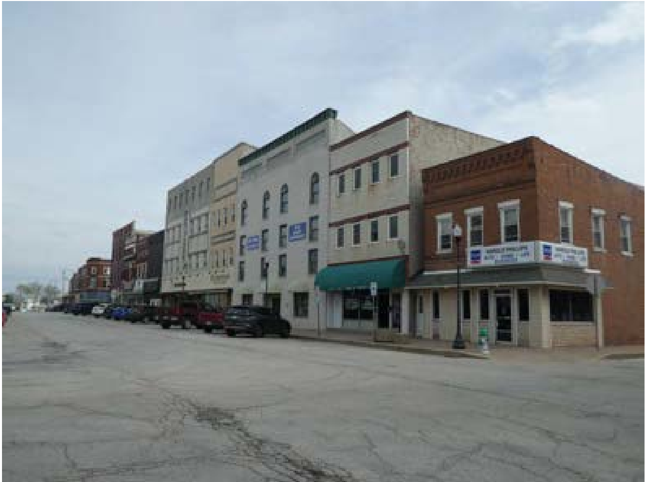
Photo 18: Buildings 37-44 facing northeast
