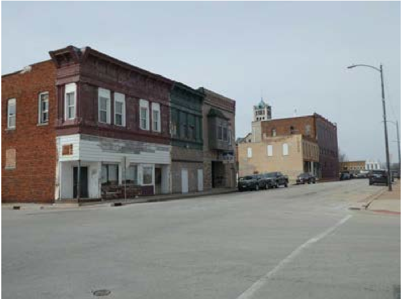
Photo 14: Buildings 31-33 facing southwest
