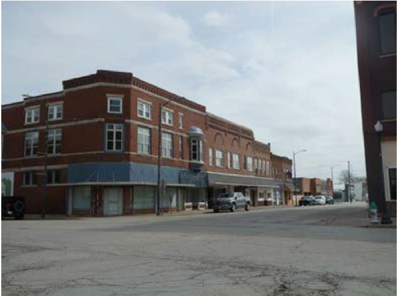
Photo 6: Buildings 17-24 facing northeast
