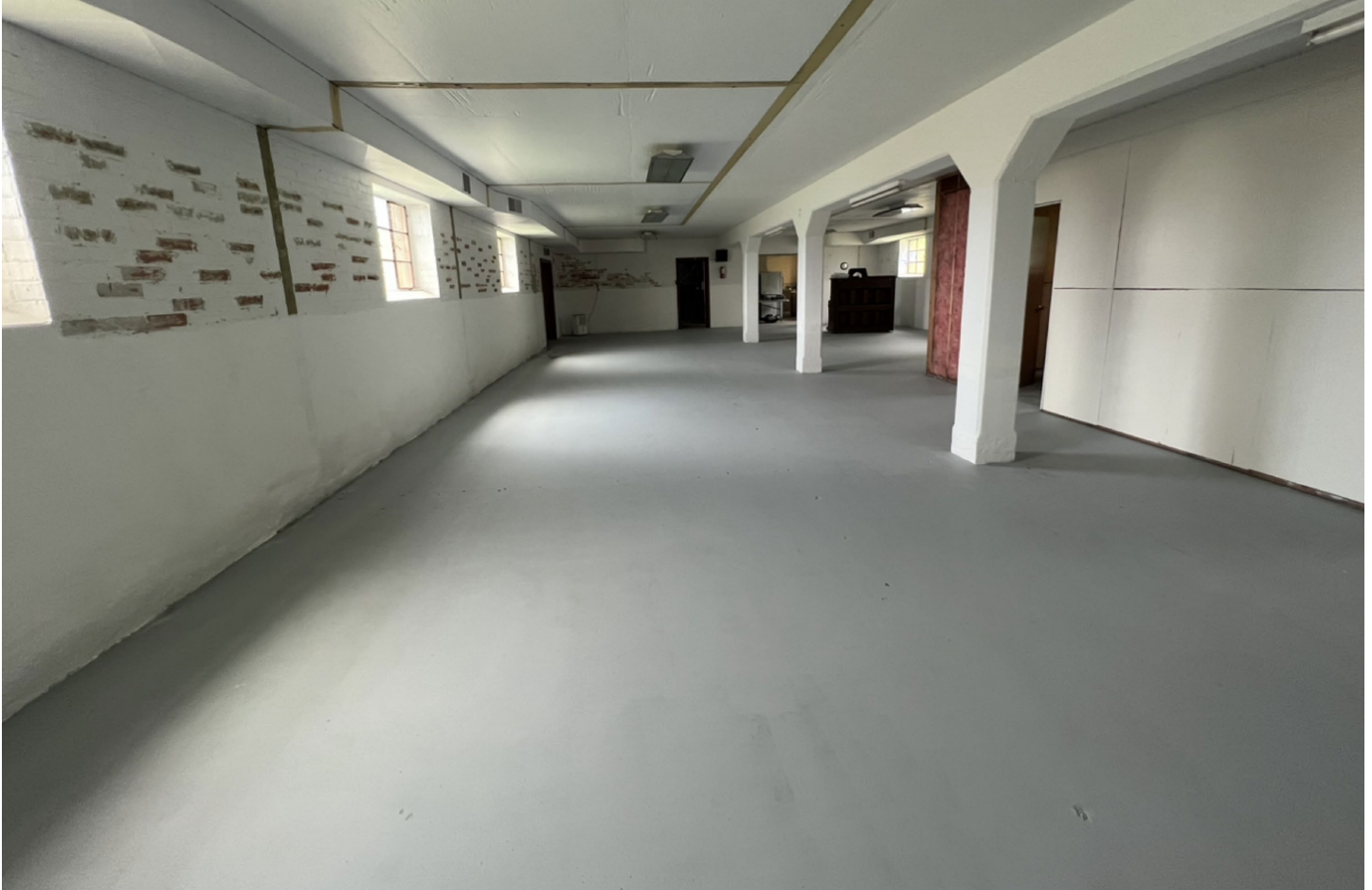
Photo 12: Basement, Looking North
