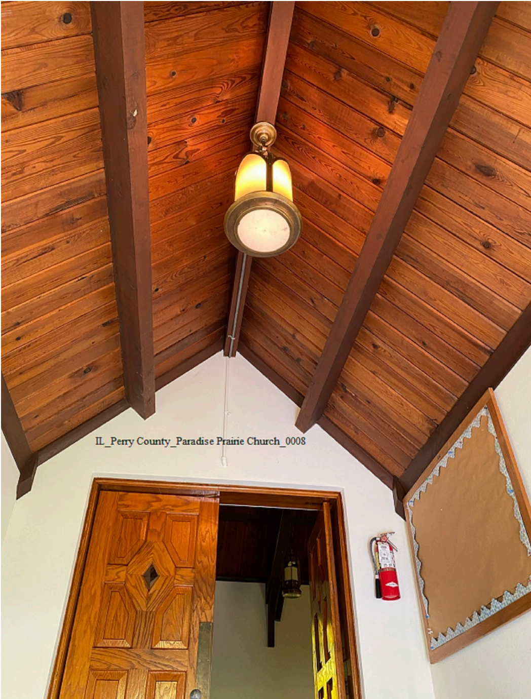
Photo 6: Interior of west entrance, looking east
