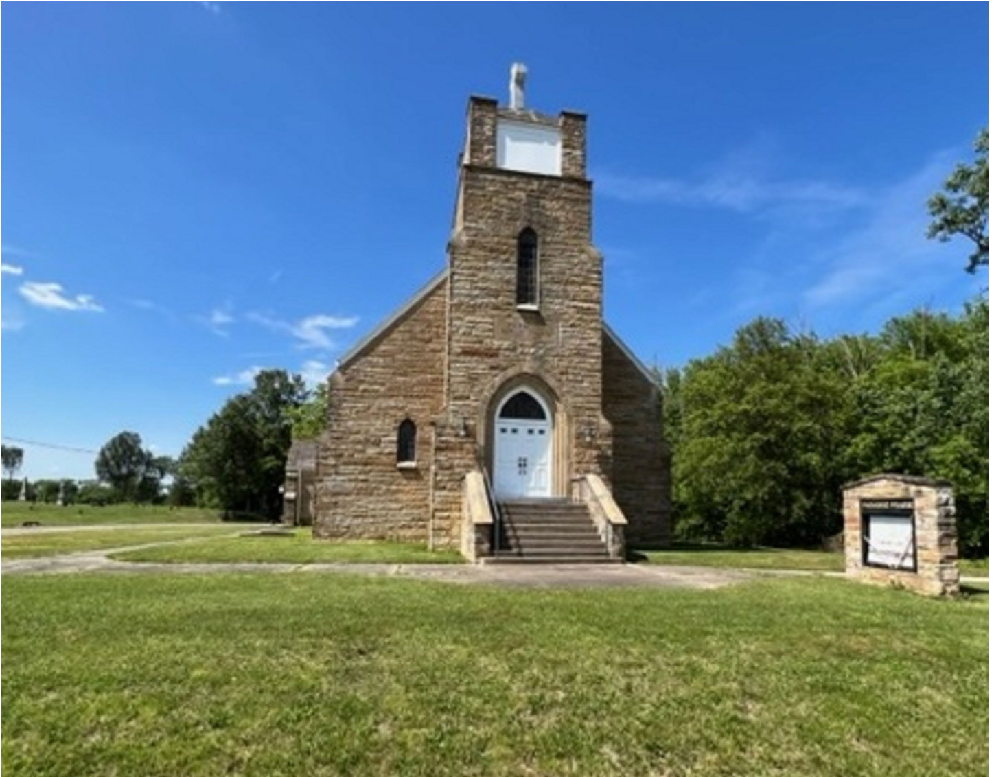
Photo 1: South Elevation of Church, looking north
