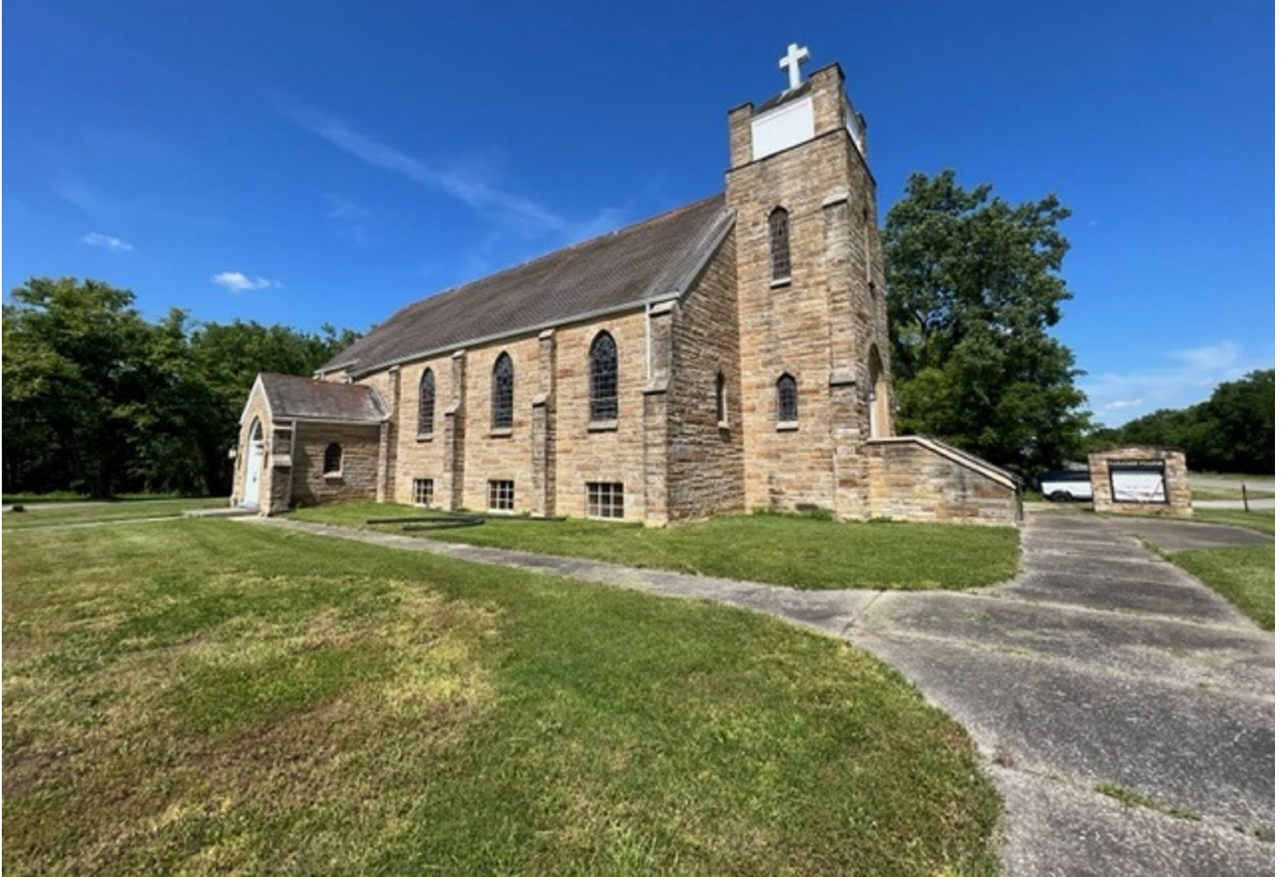
Photo 3: South and West Elevation, looking north
