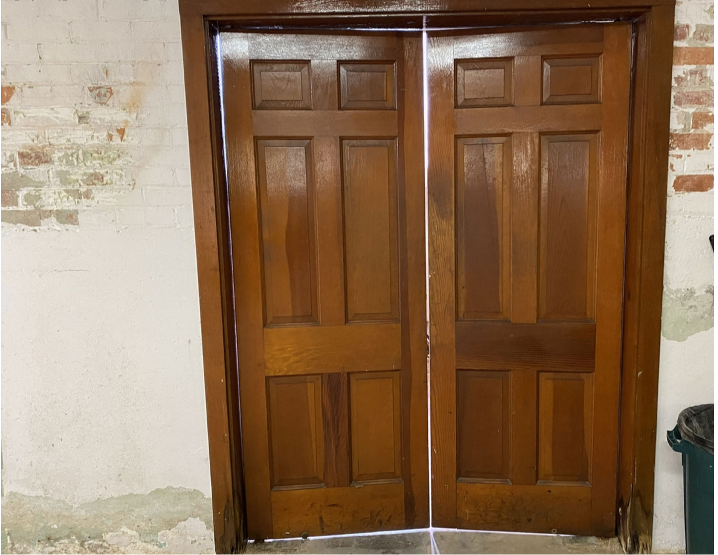
Photo 11: Basement, Original Doors
