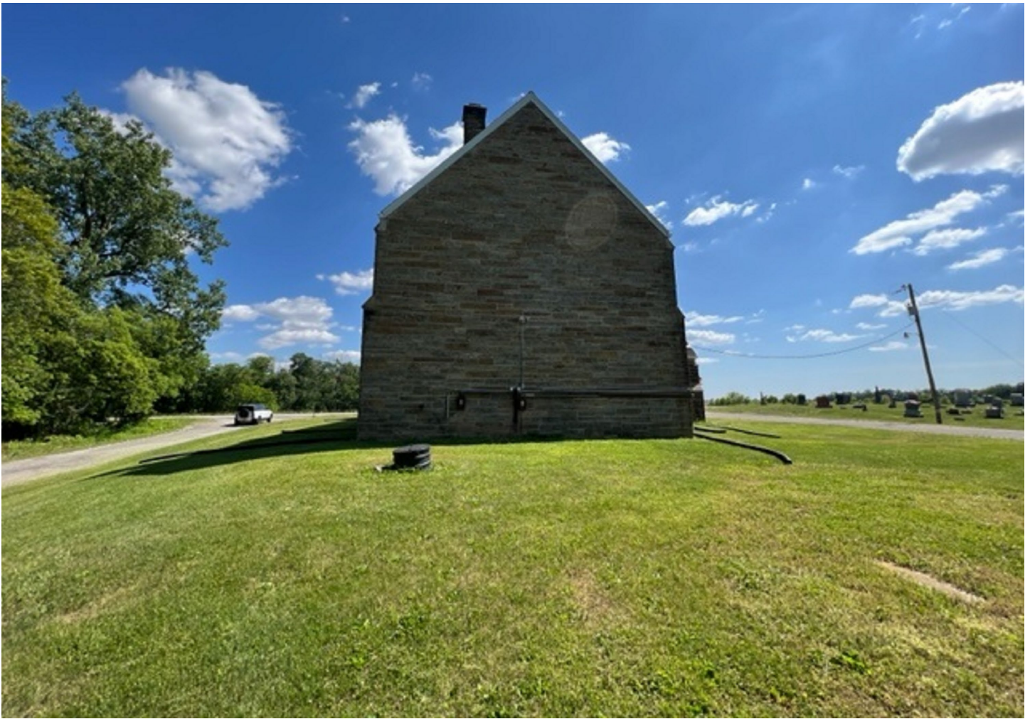
Photo 4: North Elevation looking south
