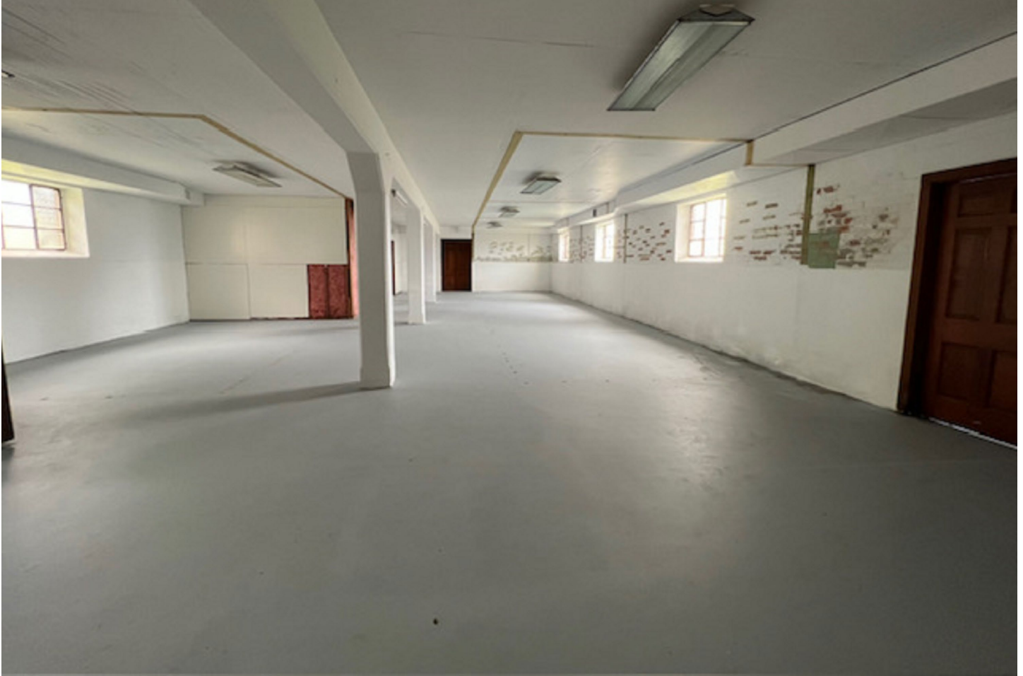
Photo 12: Basement, Looking South
