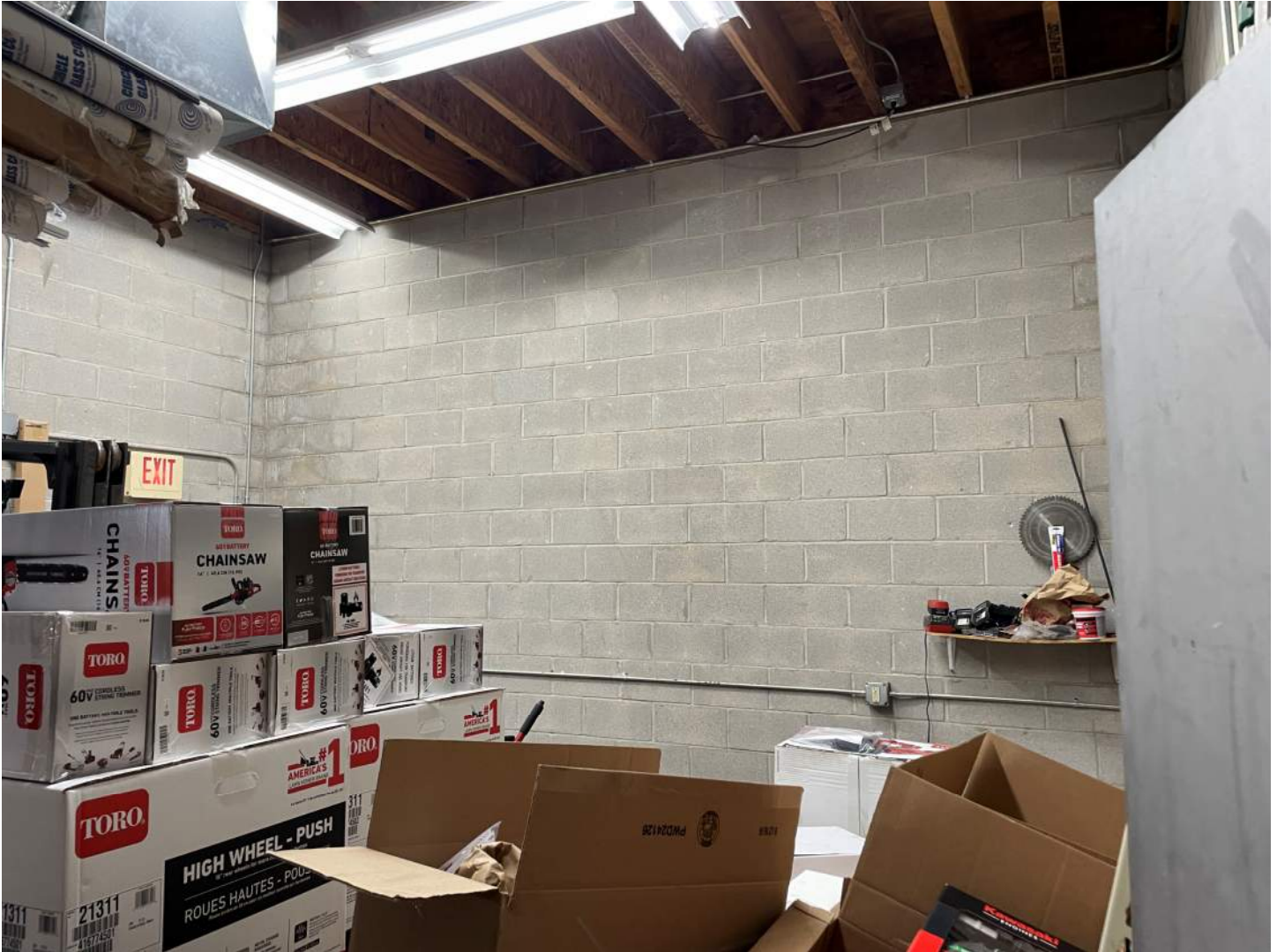
Photo 13 of 17: First floor addition; looking northwest
