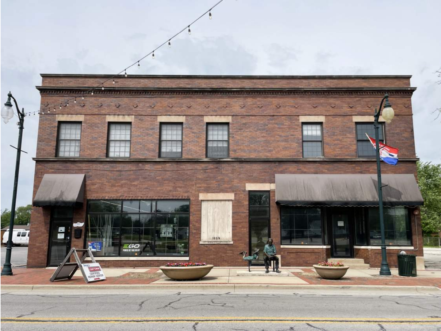
Photo 1 of 17: Primary (east) façade; looking west
