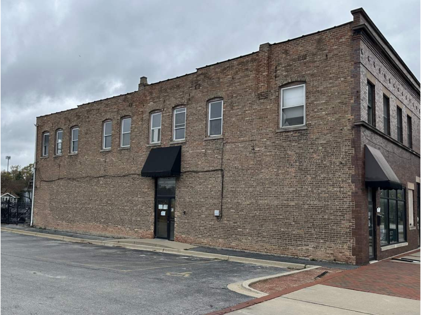
Photo 2 of 17: South elevation and side parking lot; looking northwest
