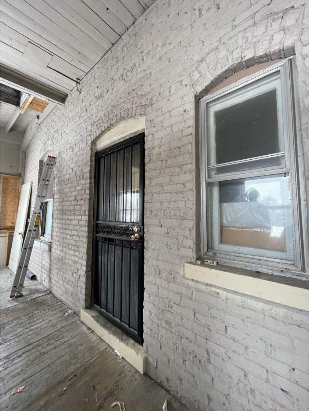
Photo 16 of 17: Second floor of stair enclosure; looking northeast – showing former exterior wall and openings
