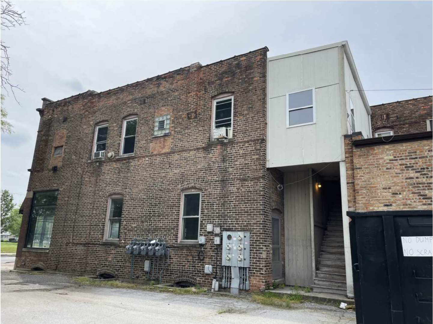
Photo 5 of 17: North elevation and stair enclosure; looking southeast
