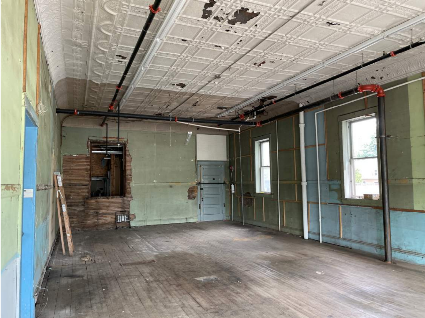
Photo 7 of 17: First floor north retail space; looking northwest
