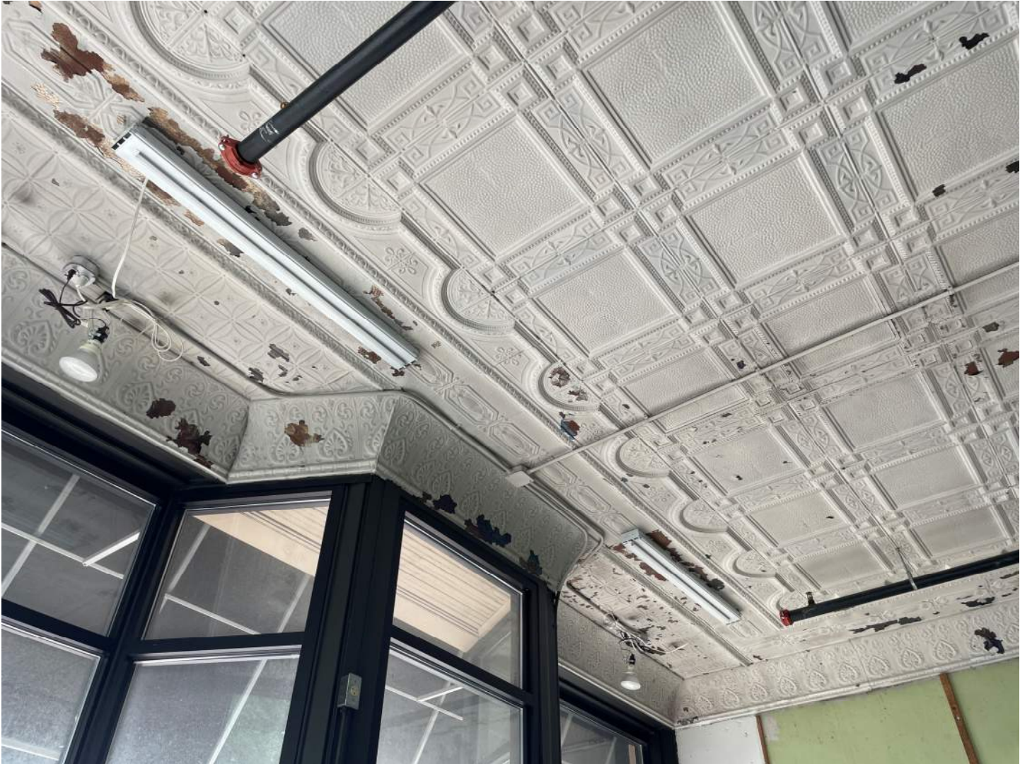
Photo 9 of 17: First floor north retail space – ceiling detail; looking southeast
