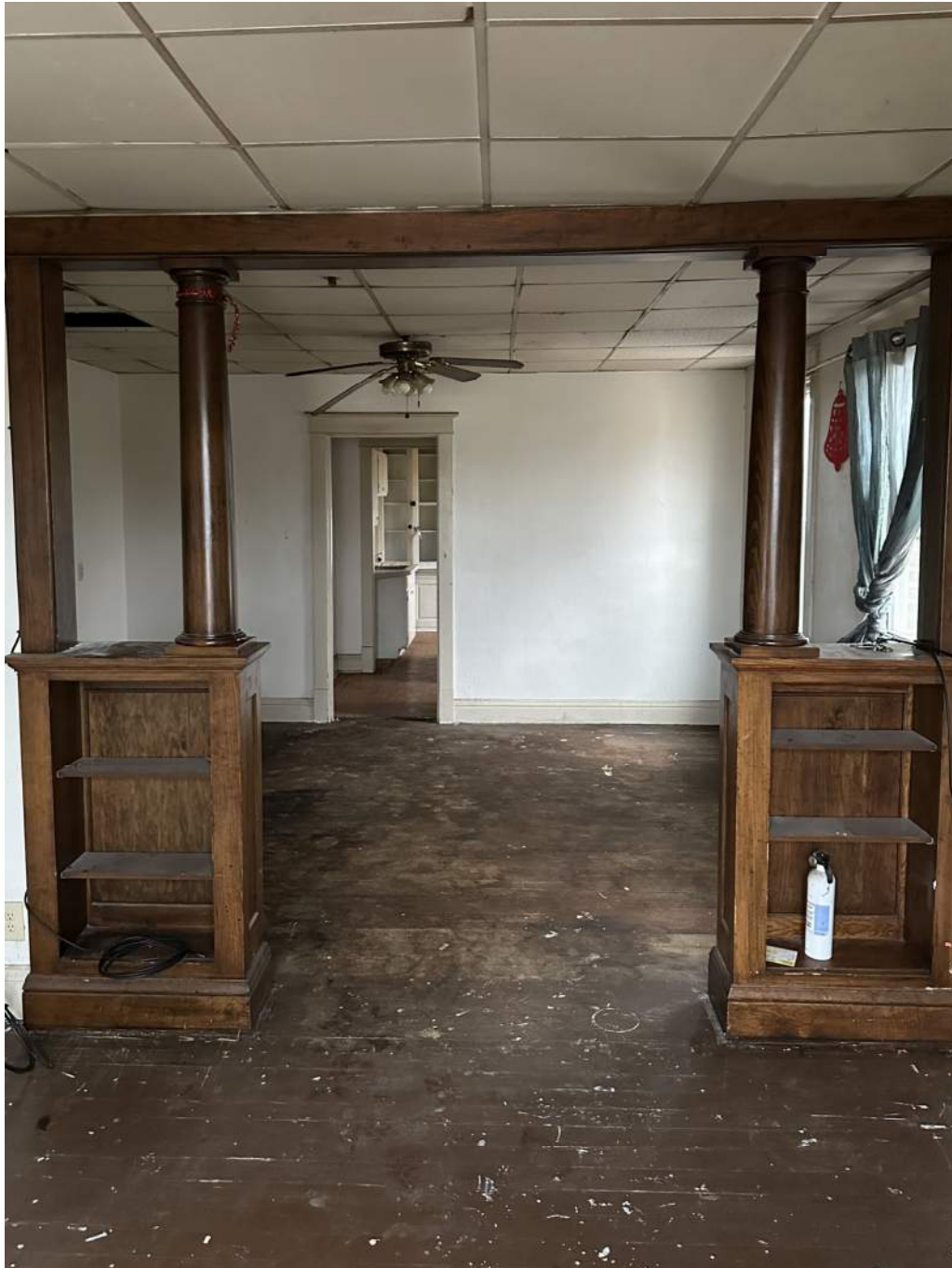
Photo 14 of 17: Second floor apartment; looking west – showing wooden colonnade room divider
