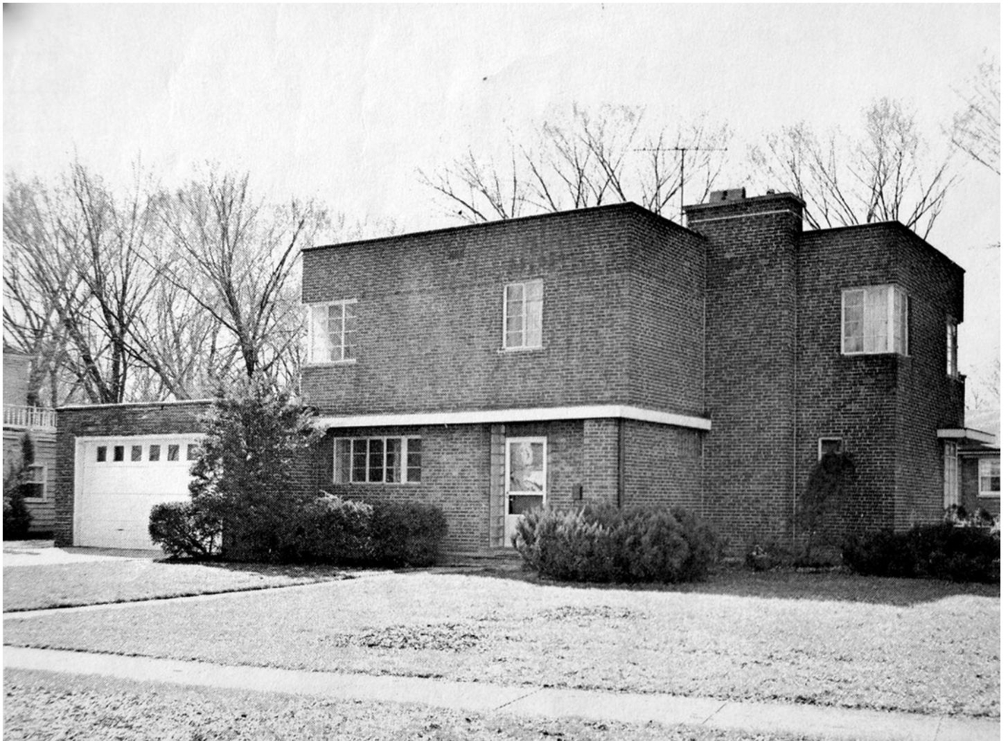
Fig. 9. Benda House Photograph (c. mid 1960s), North / West View
