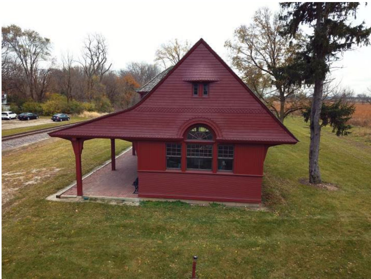
Photo 1: Exterior north elevation, camera facing South
