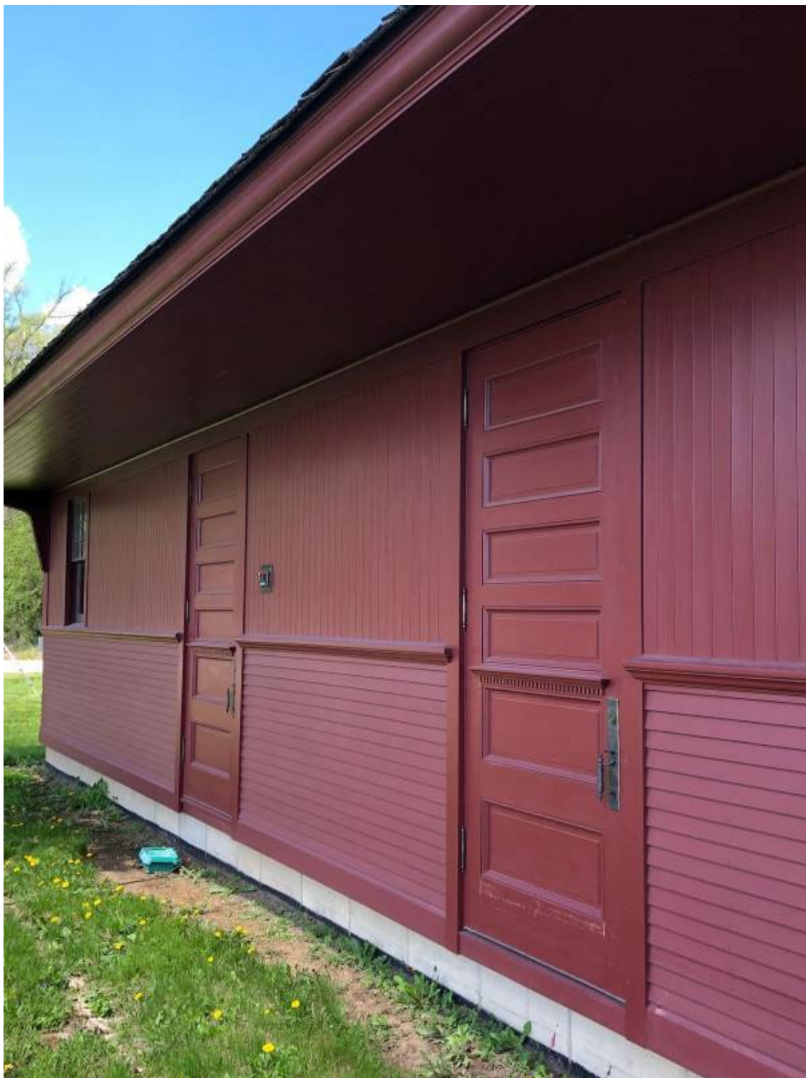
Photo 9: Close up of two doors from west elevation, camera facing east
