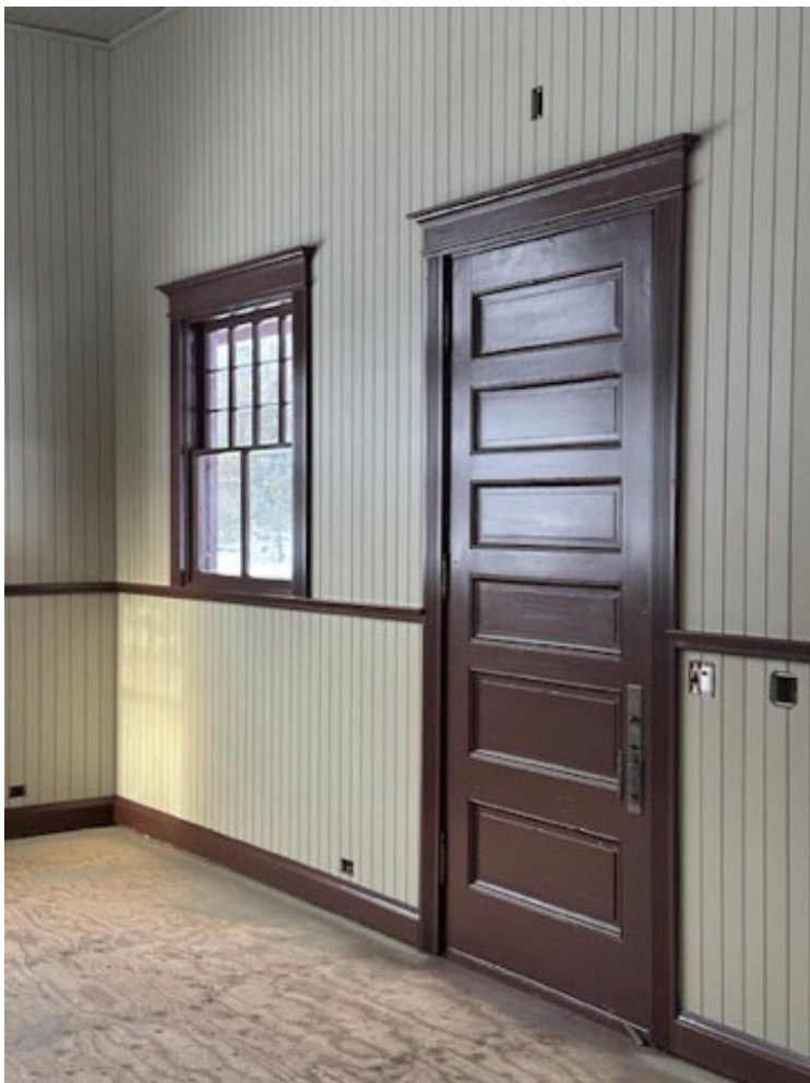
Photo 15: Interior, northeast corner.
