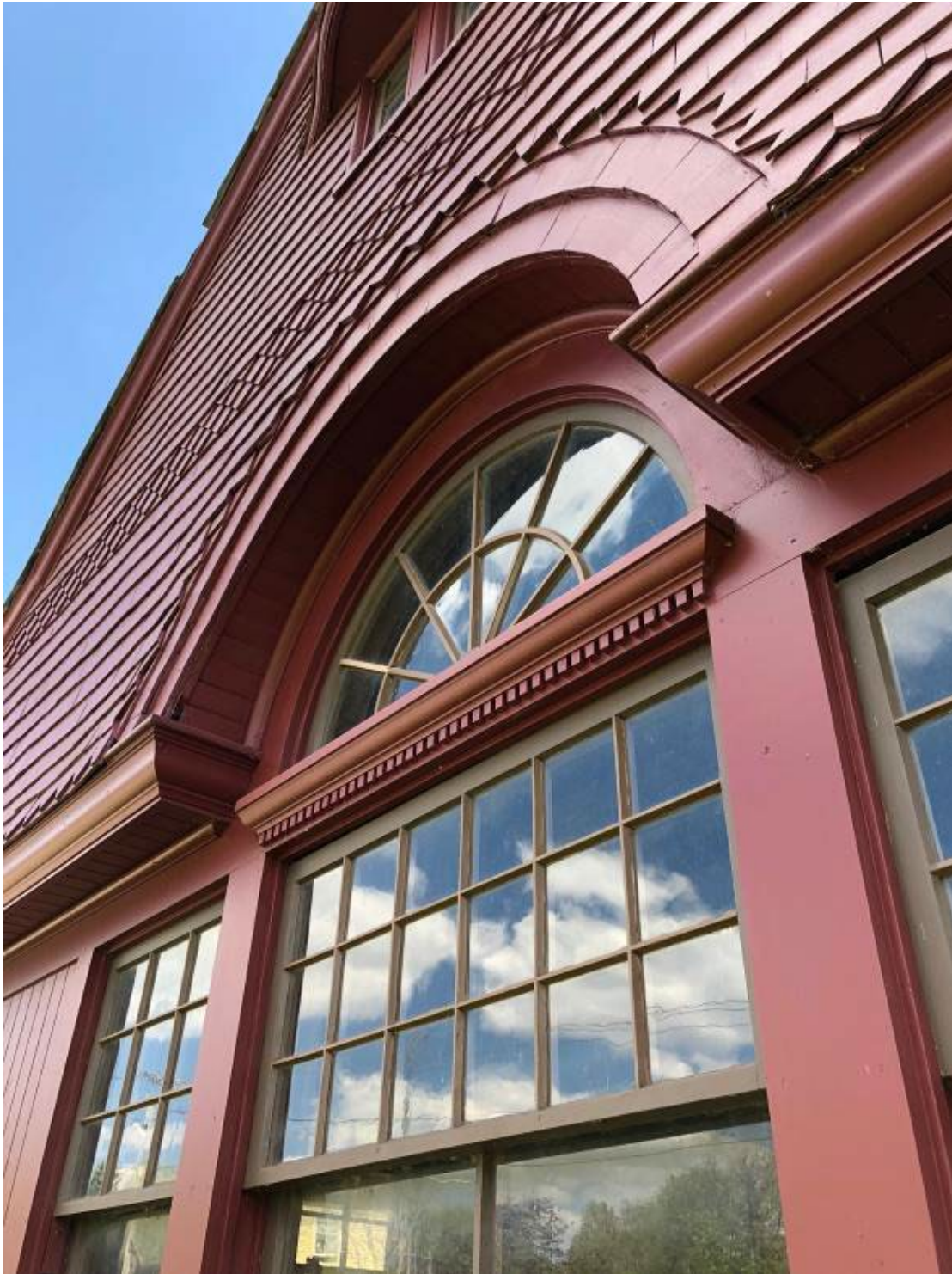
Photo 5: Close up North elevation camera facing South
