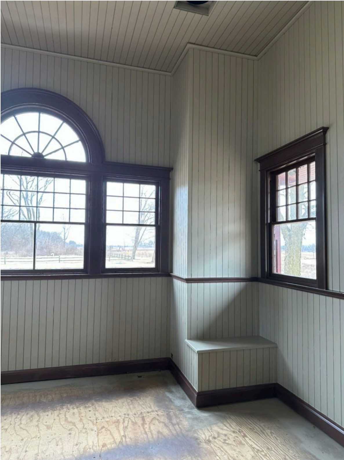
Photo 14: Interior, southwest corner.
