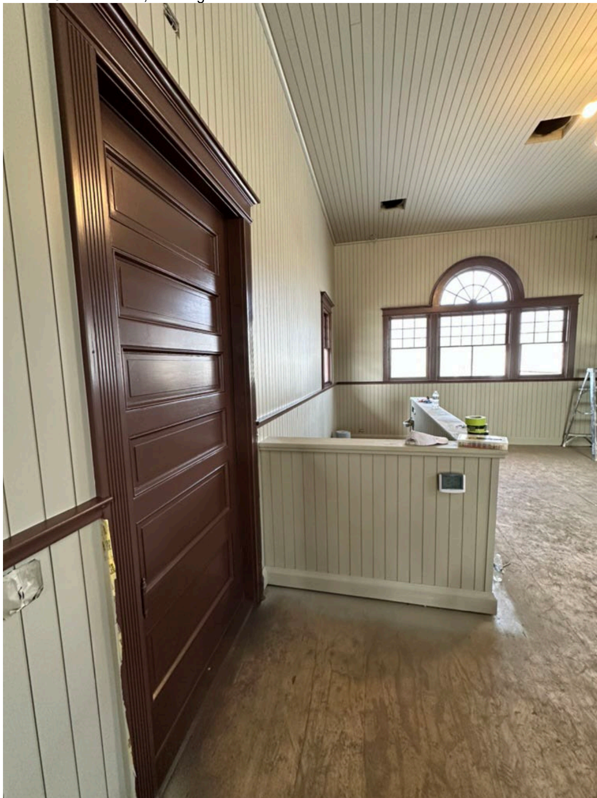
Photo 13: Interior, showing west and north walls.
