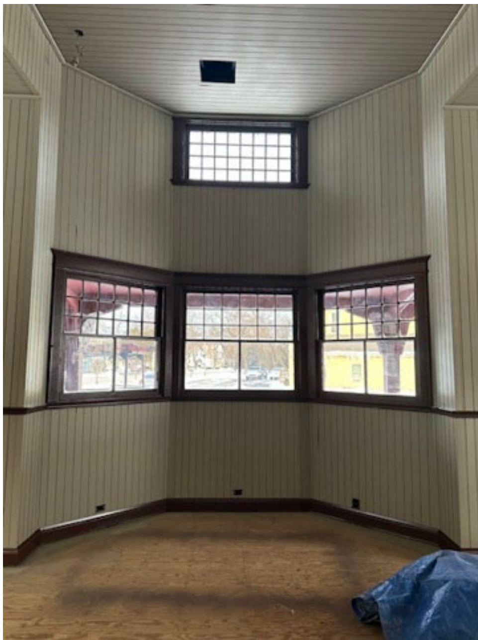
Photo 11: Interior, close up of bay on east wall.
