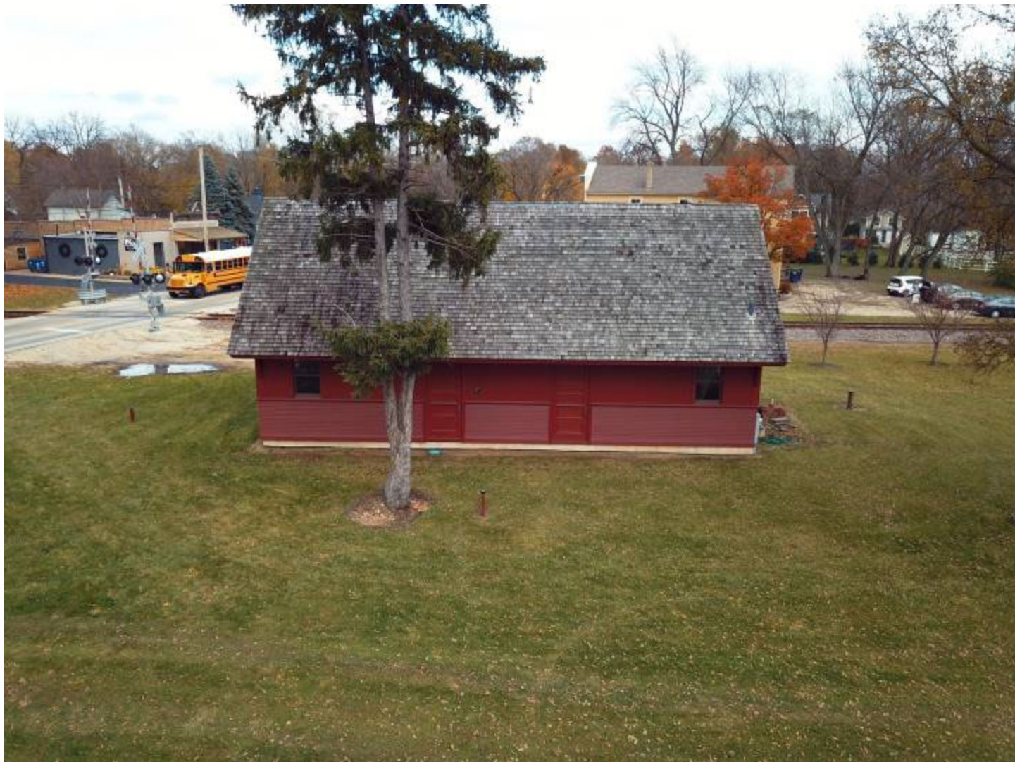
Photo 4: Exterior west elevation, camera facing East
