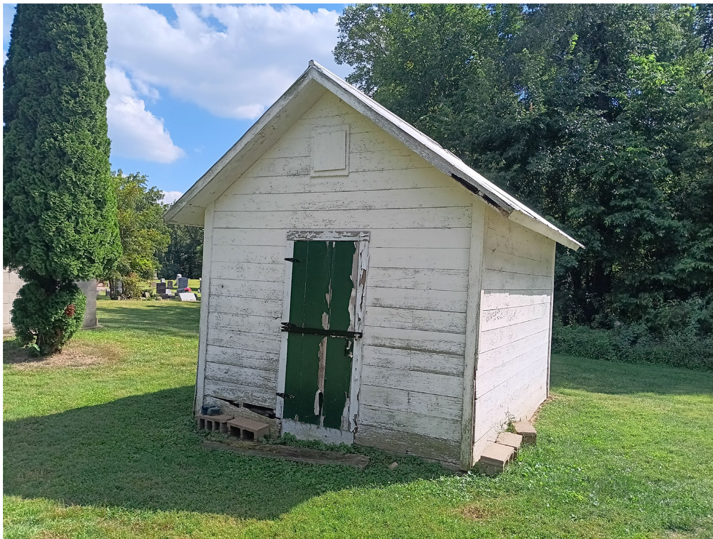
Photo 7 of 15: Storage Shed
