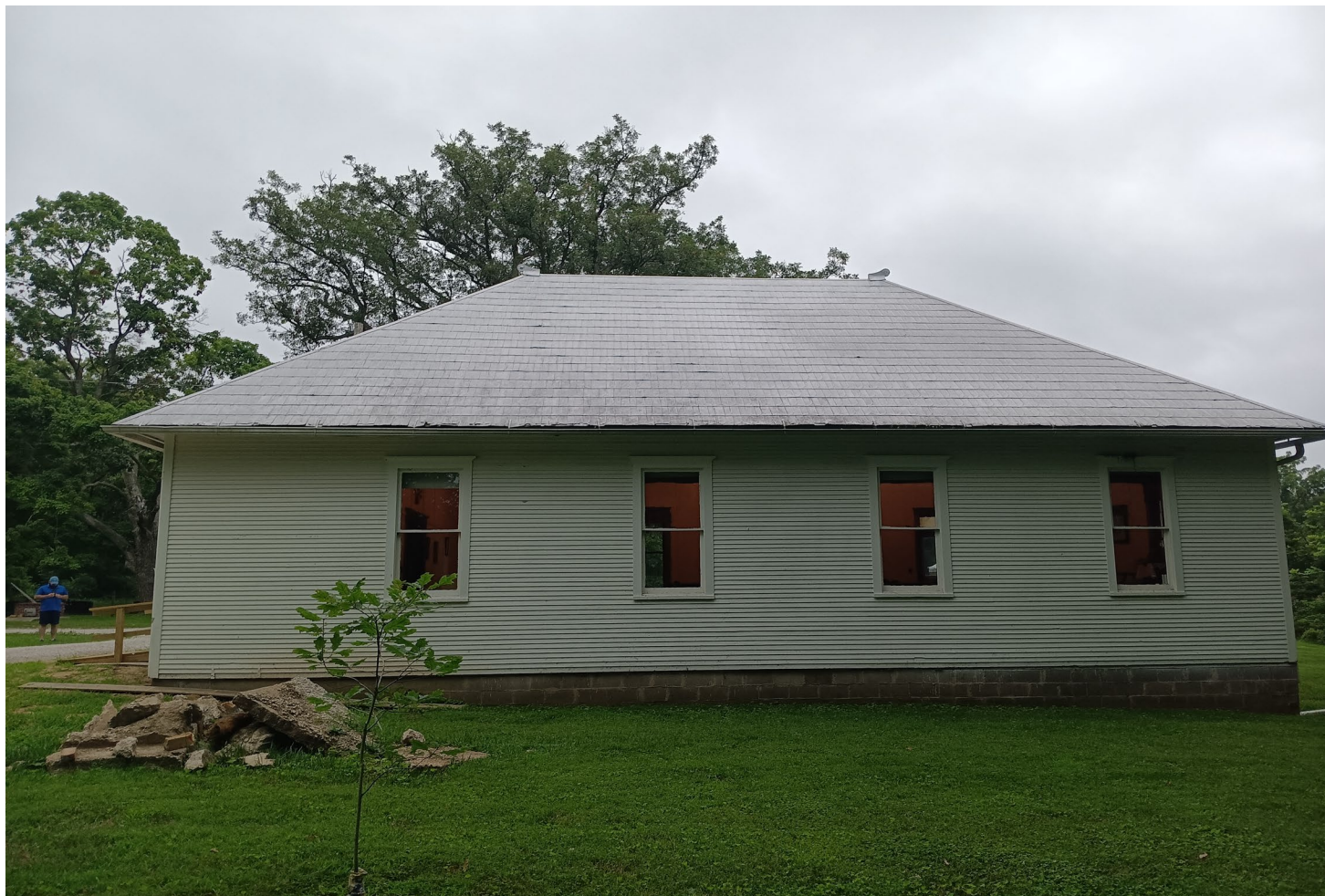
Photo 2 of 15: West side of building
