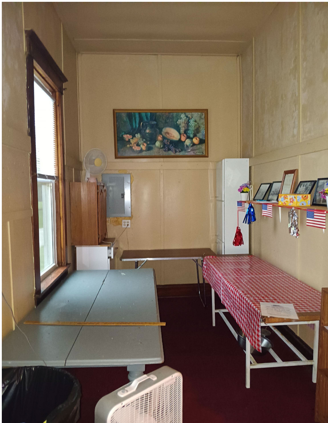
Photo 8 of 15: East wall, inside front door
