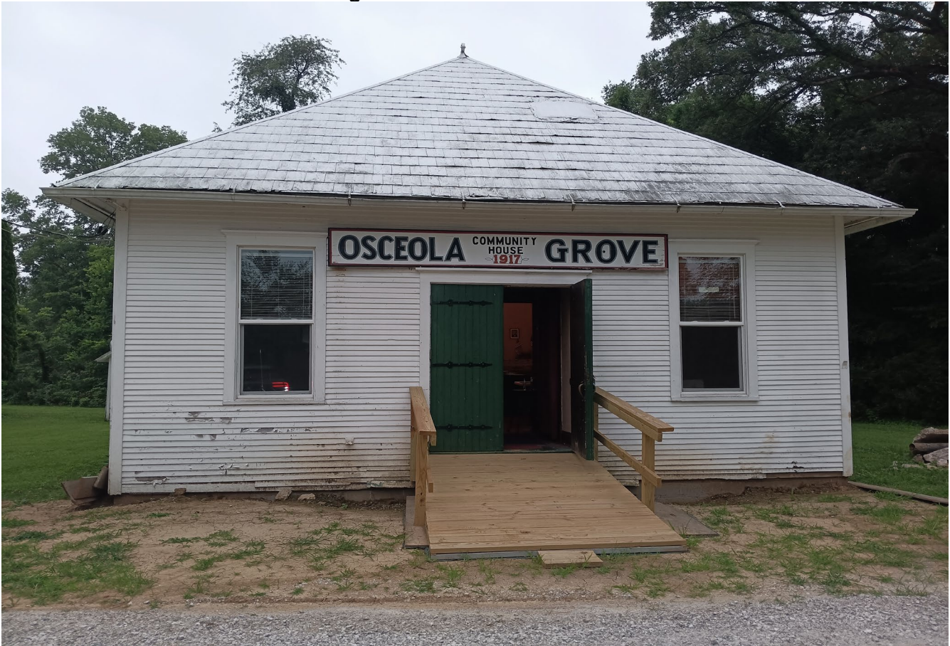
Photo 1 of 15: North side of building
