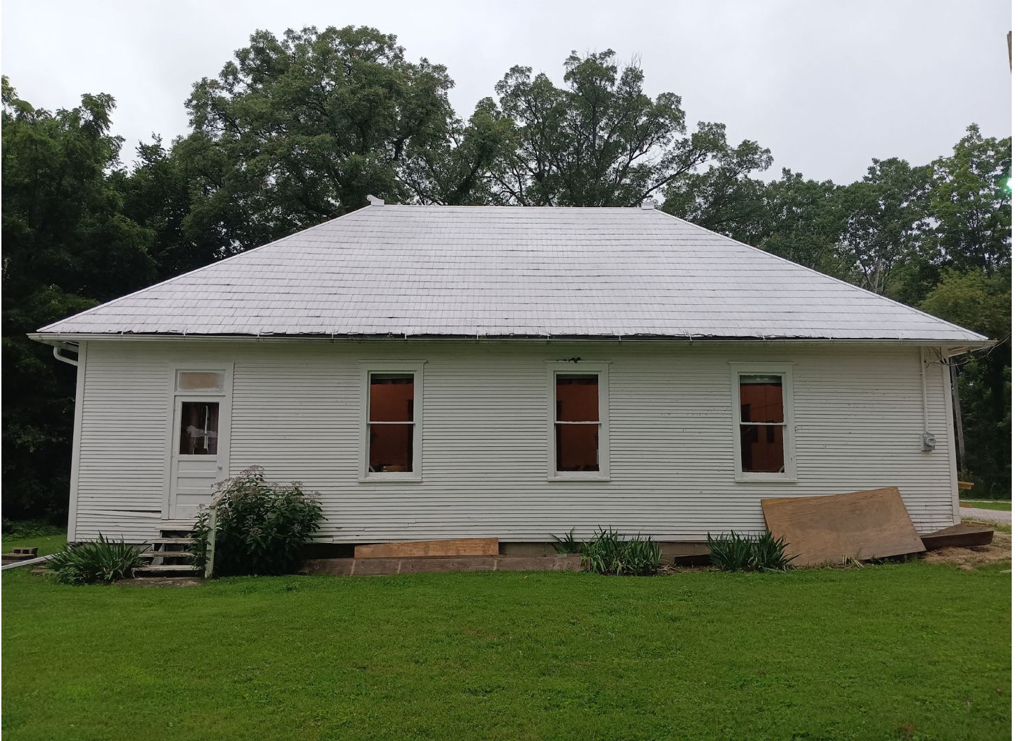
Photo 4 of 15: East side of building
