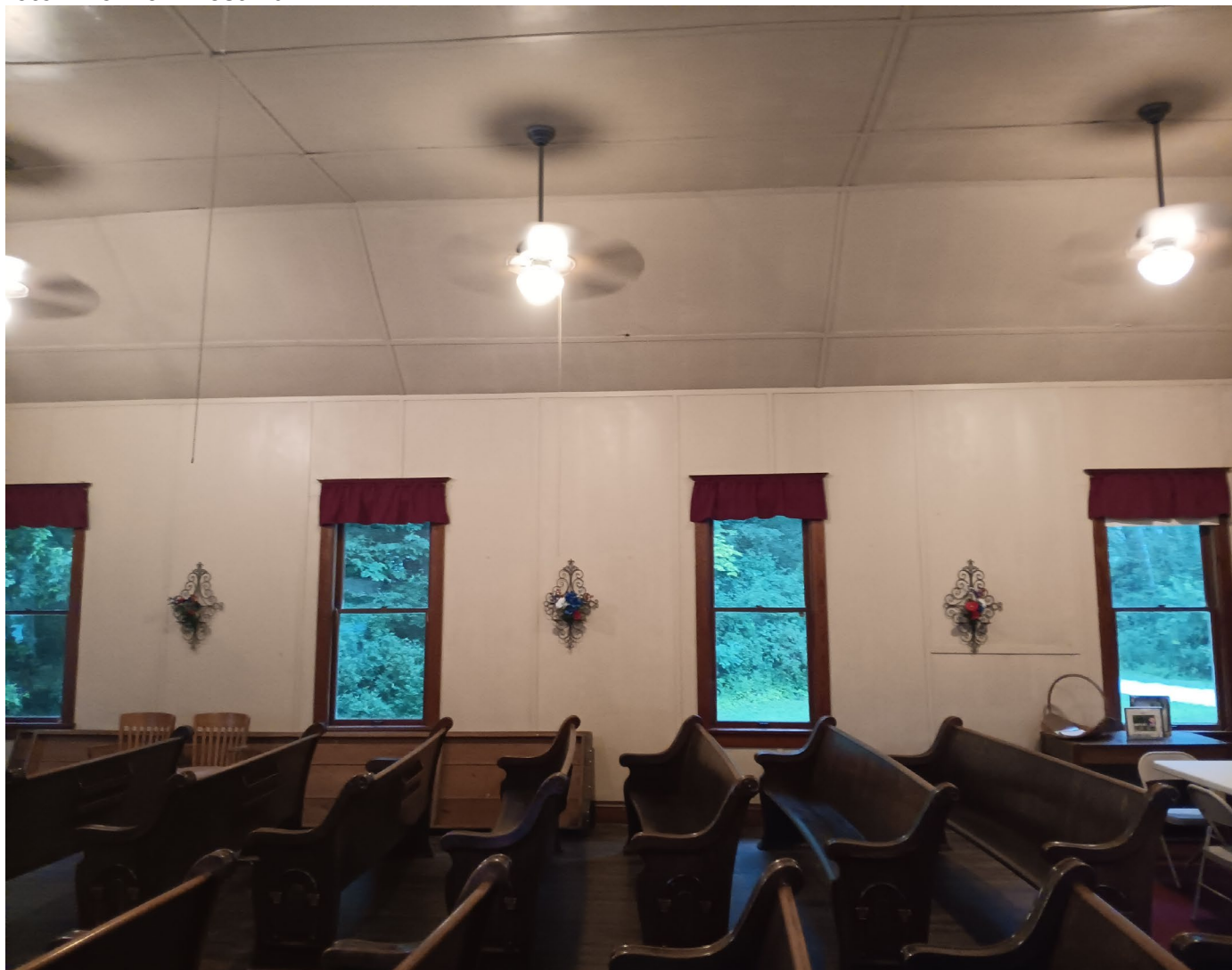
Photo 11 of 15: West wall
