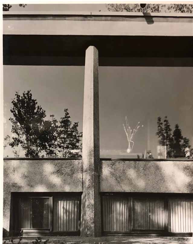
Figure 3: The Rockwell House, south elevation, detail, Olympia Fields, IL (1964). Brenner-Danforth-Rockwell, architects. Image: Hedrich-Blessing. Ryerson and Burnham Art and Architecture Archives, The Art Institute of Chicago.
