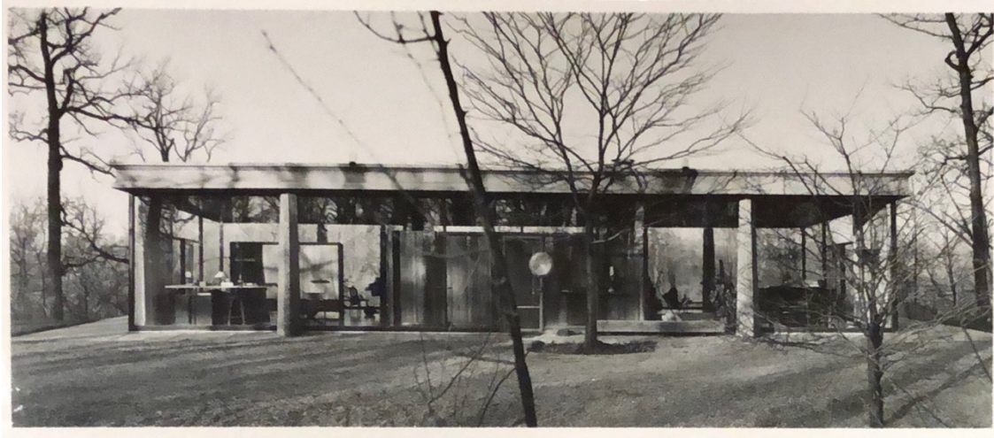
Figure 2: The Rockwell House, north elevation, Olympia Fields, IL (1964). Brenner-Danforth-Rockwell, architects. Image: Hedrich-Blessing. Ryerson and Burnham Art and Architecture Archives, The Art Institute of Chicago.
