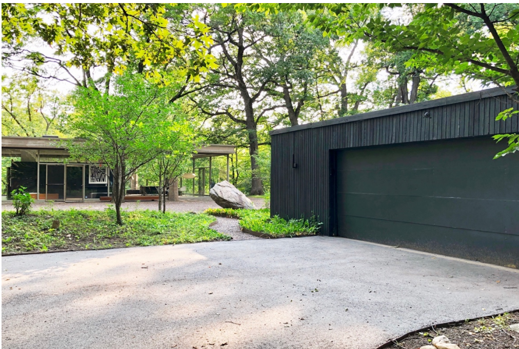
IL_Cook County_The Rockwell House_0014, Garage/Pool-House at center of lot, view toward forecourt and House, view south.
