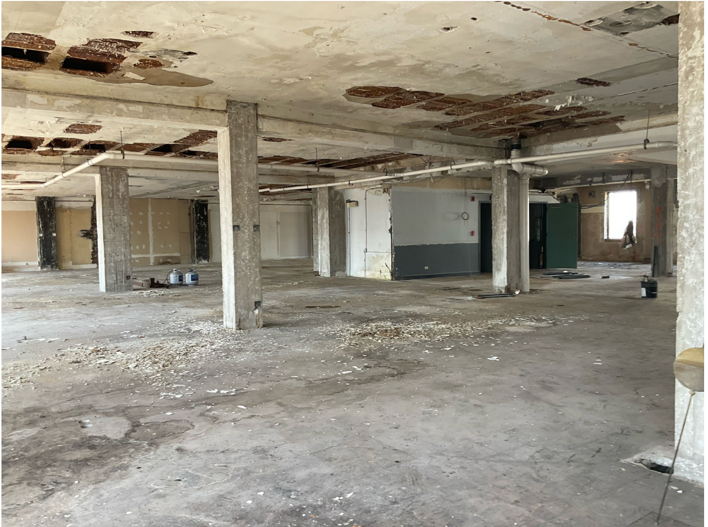
Photo 12 of 14: Oak Leaves Building, interior, 5th floor, looking northwest
