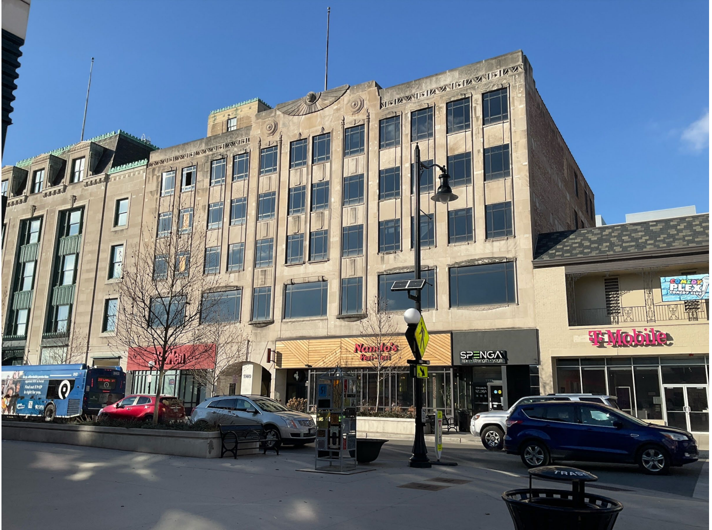
Photo 3 of 14: Oak Leaves Building, south elevation, facing northwest
