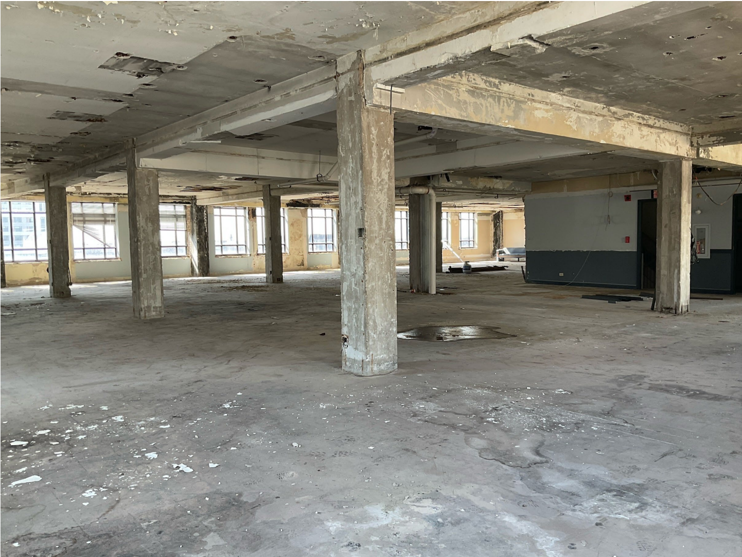
Photo 11 of 14: Oak Leaves Building, interior, 5 th floor, looking southwest
