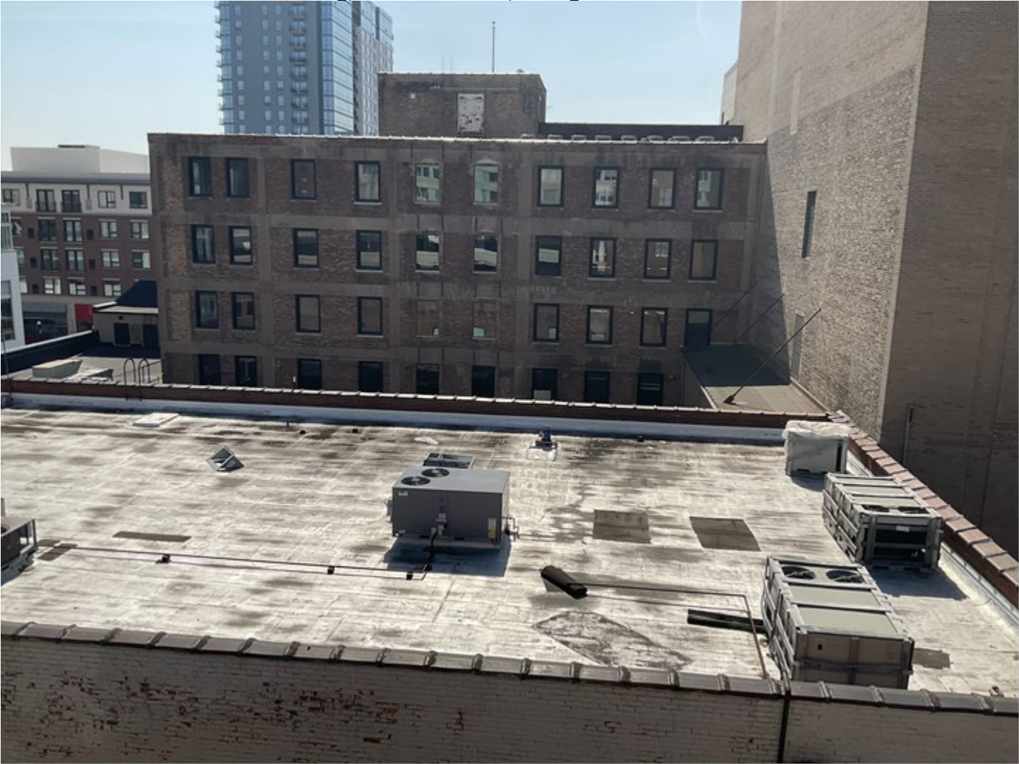
Photo 4 of 14: Oak Leaves Building, north elevation, facing south
