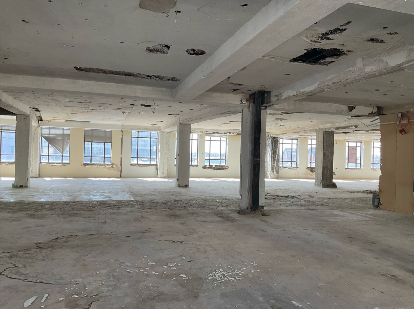
Photo 14 of 14: Oak Leaves Building, interior, 3rd floor, looking southwest
