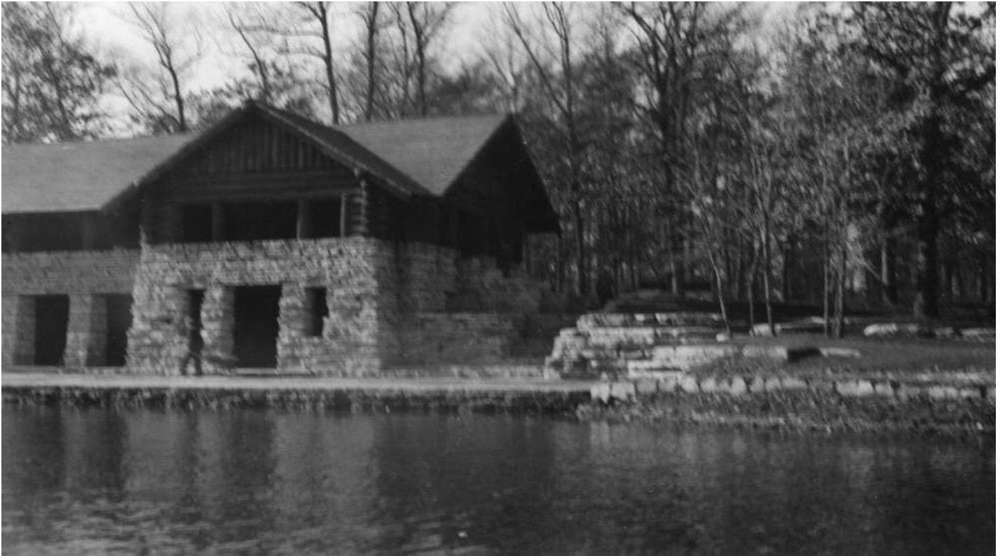
FIGURE 7: EXTERIOR VIEW OF THE BOATHOUSE IN NOVEMBER 1936, LOOKING SOUTHWEST. PHOTOGRAPH COURTESY OF THE FOREST PRESERVE DISTRICT OF DUPAGE COUNTY.
