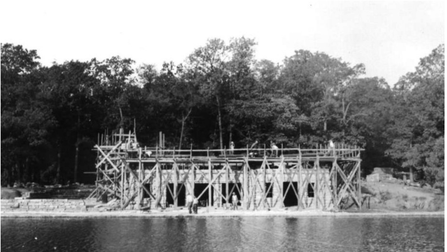
FIGURE 5: EXTERIOR VIEW OF THE BOATHOUSE UNDER CONSTRUCTION IN SEPTEMBER 1936, LOOKING WEST. COURTESY OF THE FOREST PRESERVE DISTRICT OF DUPAGE COUNTY.
