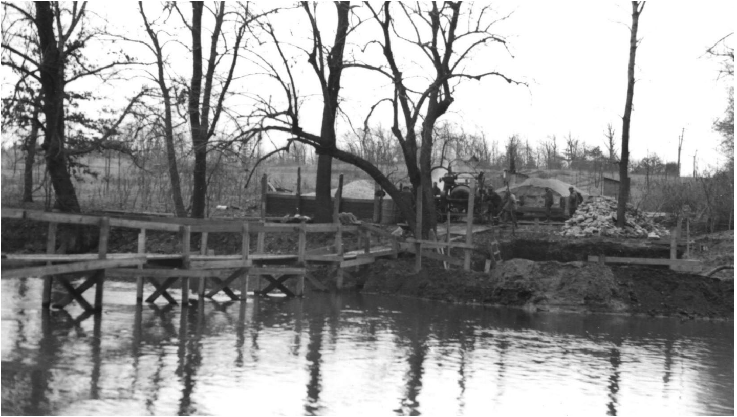
FIGURE 11: PHOTOGRAPH OF COMPANY V-1668 POURING CONCRETE FOOTINGS FOR THE FOOT AND HORSE BRIDGE, UNDATED. PHOTOGRAPH COURTESY OF THE FOREST PRESERVE DISTRICT OF DUPAGE COUNTY.
