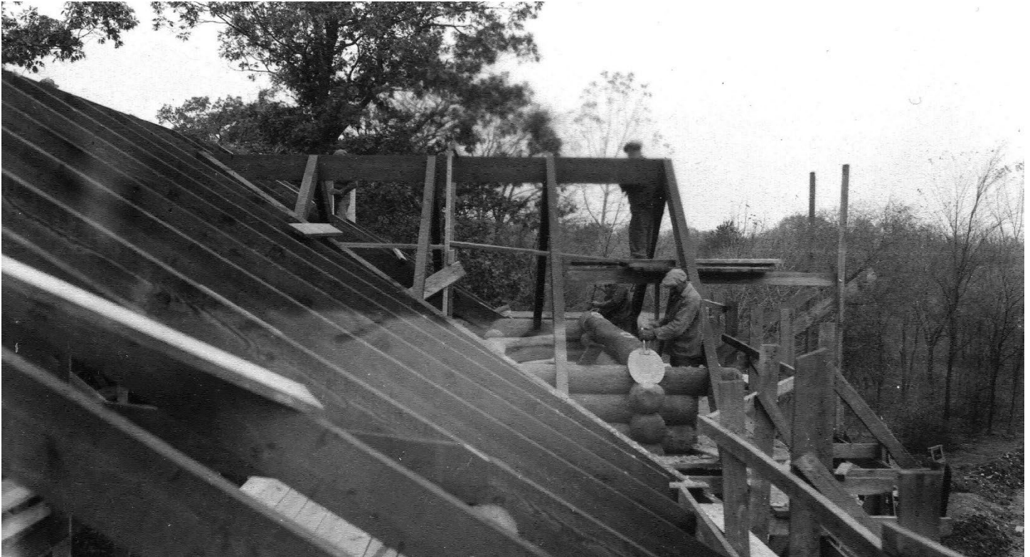
FIGURE 6: THE CONSTRUCTION OF THE BOATHOUSE ROOF, UNDATED. PHOTOGRAPH COURTESY OF THE FOREST PRESERVE DISTRICT OF DUPAGE COUNTY.
