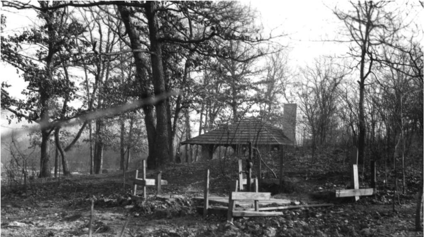
FIGURE 9: EXTERIOR VIEW OF A TYPICAL WELL WITH SHELTER COVER AND WATER PUMP UNDER CONSTRUCTION, NON-EXTANT, IN JANUARY 1937. THE KITCHEN AND PICNIC SHELTER IS IN THE BACKGROUND. COURTESY OF THE FOREST PRESERVE DISTRICT OF DUPAGE COUNTY.
