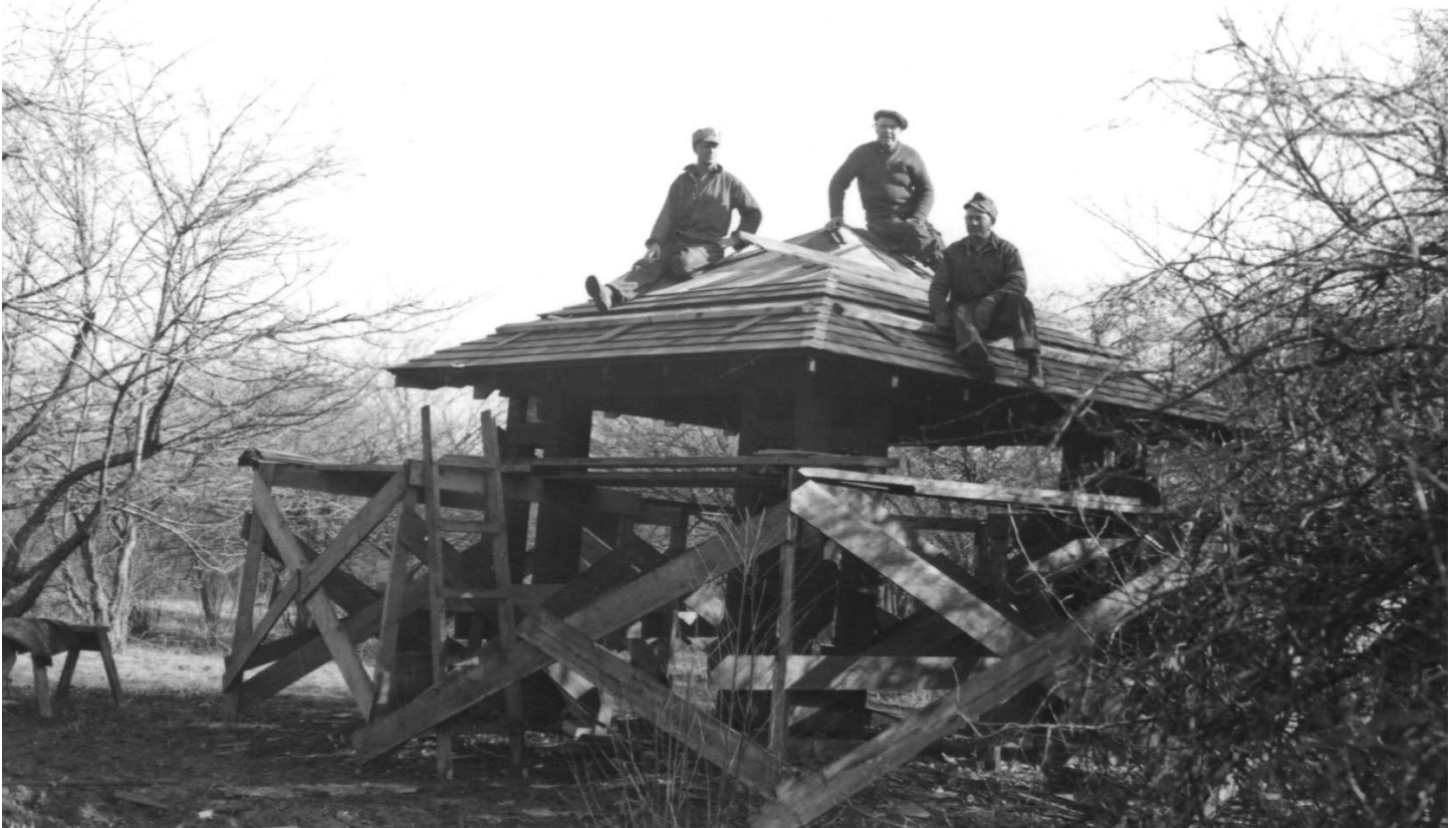
FIGURE 10: PHOTOGRAPH OF WELL 4 UNDER CONSTRUCTION, UNDATED. PHOTOGRAPH COURTESY OF THE FOREST PRESERVE DISTRICT OF DUPAGE COUNTY.
