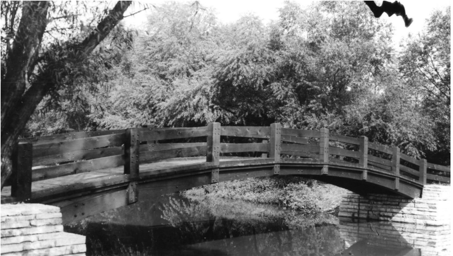
FIGURE 12: THE FOOT AND HORSE BRIDGE IN 1937. THE HISTORIC WOOD MEMBERS ARE NON-EXTANT. PHOTOGRAPH COURTESY OF THE FOREST PRESERVE DISTRICT OF DUPAGE COUNTY.
