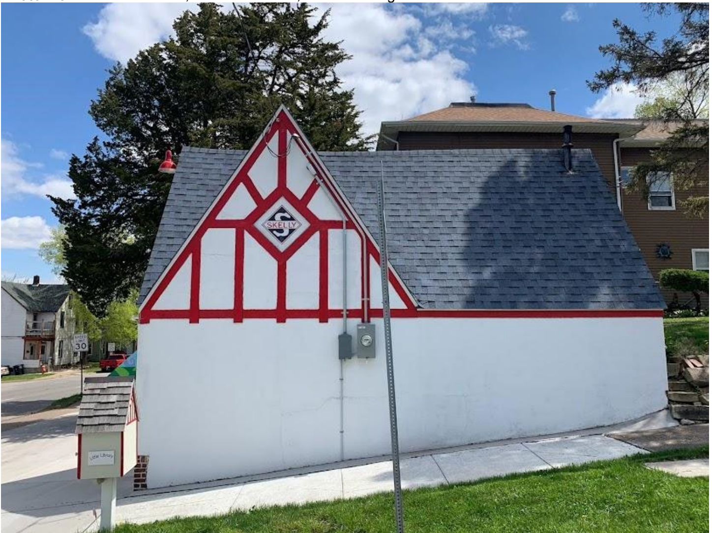
Photo 2 of 11: West Facade, view from 8th St, camera facing east.
