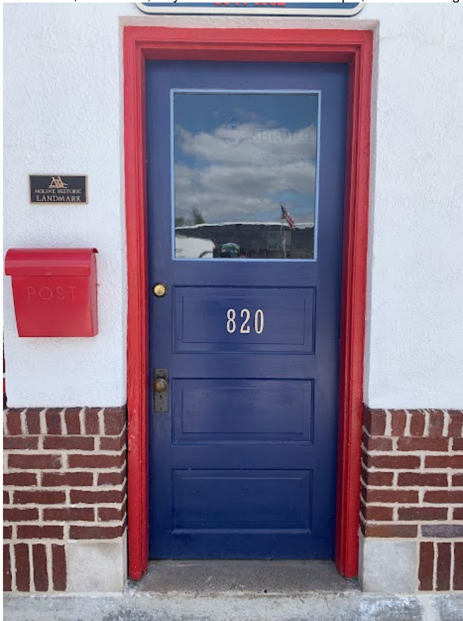
Photo 5 of 11: Front entrance, 1900 door, City of Moline Landmark Plaque, camera facing south.
