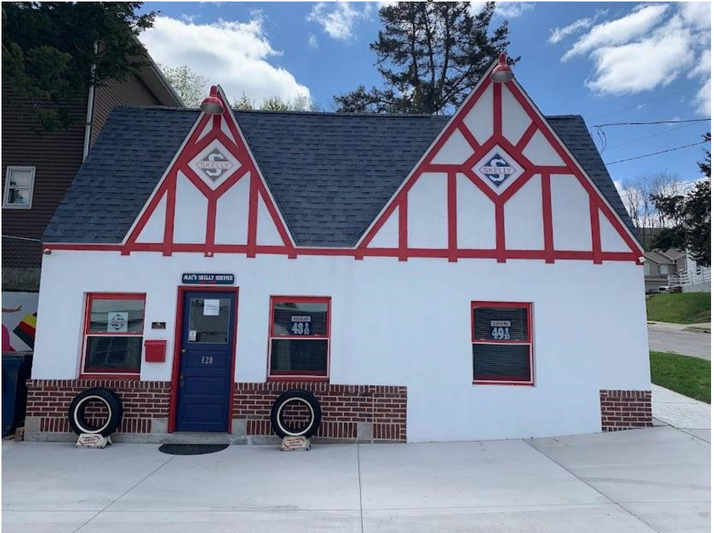
Photo 1 of 11: North Facade: view from 5th Avenue, camera facing south.
