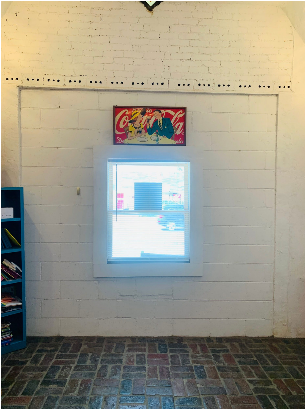
Photo 10 of 11: View from interior of enclosed service bay door opening, camera facing north.
