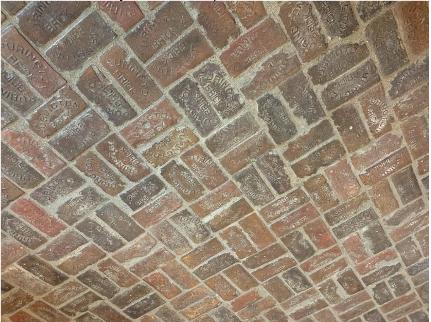
Photo 9 of 11: Restored Purington Bricks in service bay.
