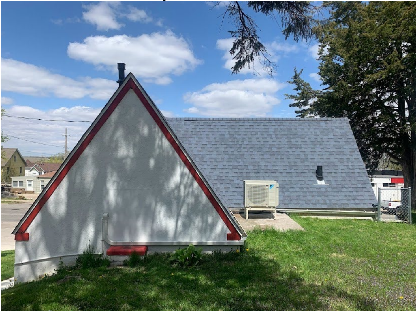
Photo 3 of 11: South facade, camera facing north.
