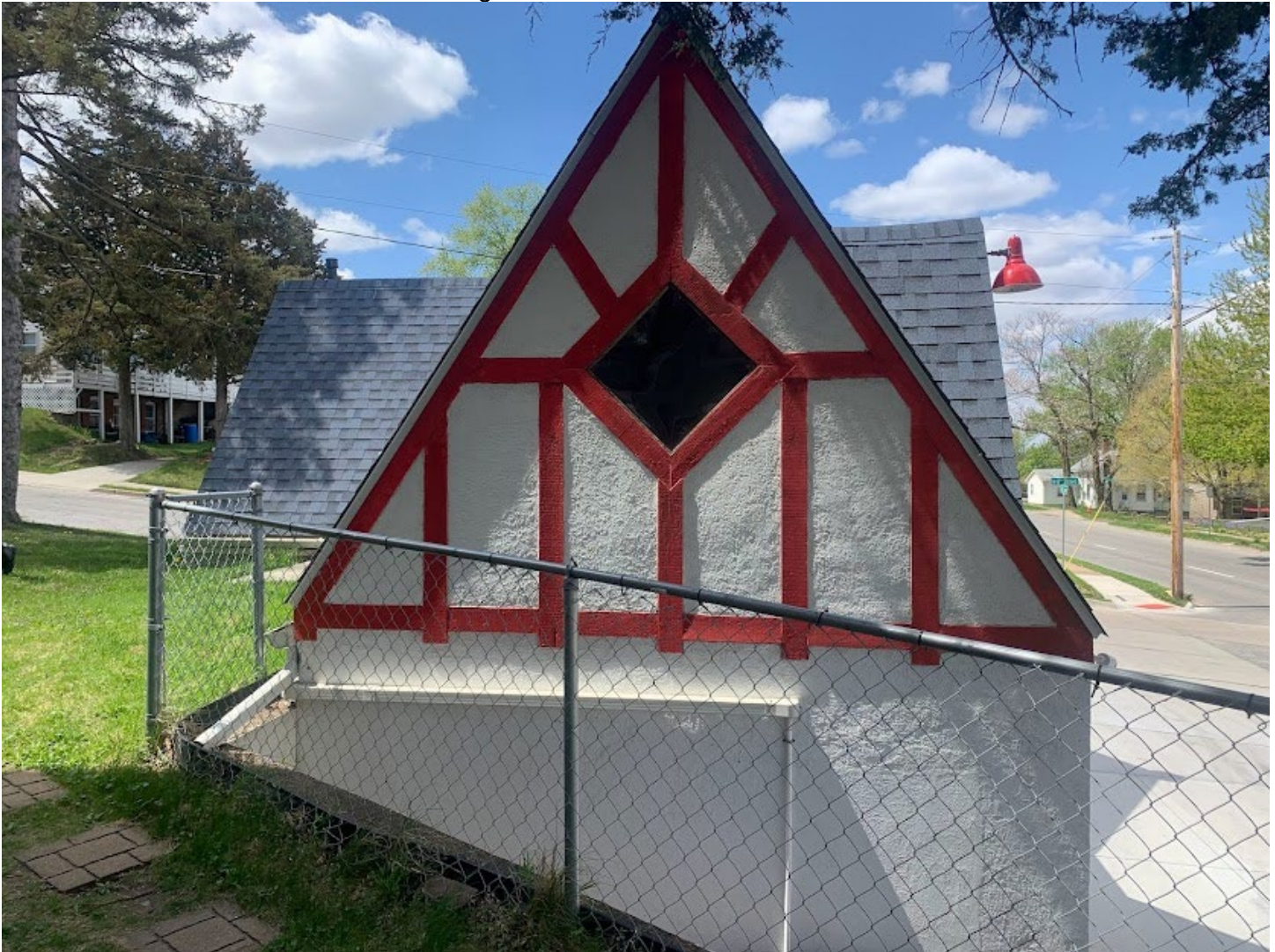
Photo 4 of 11: East facade, camera facing west.
