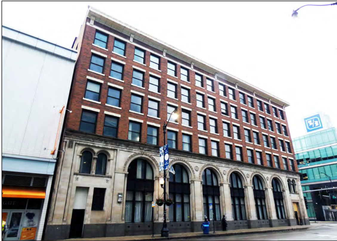
Photo 3 of 15: Halsted Street facade, looking northwest
