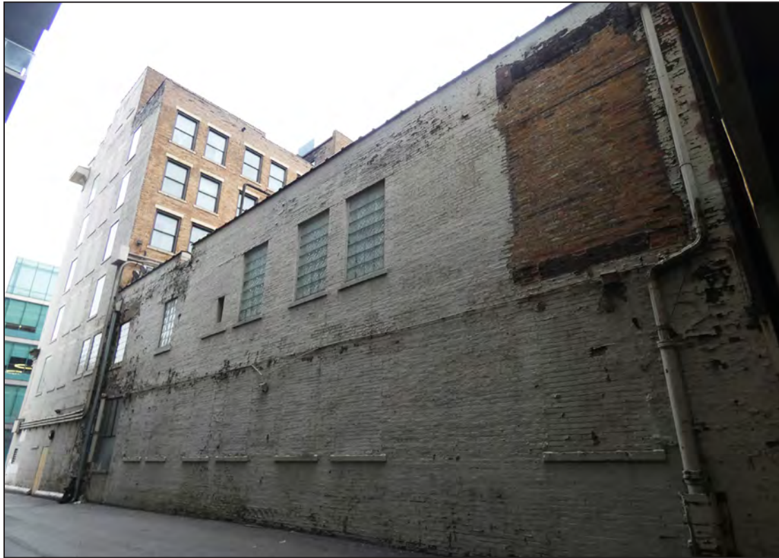
Photo 7 of 15: West alley façade, looking northeast
