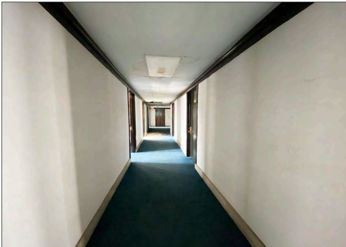
Photo 14 of 15: Typical upper floor corridor interior
