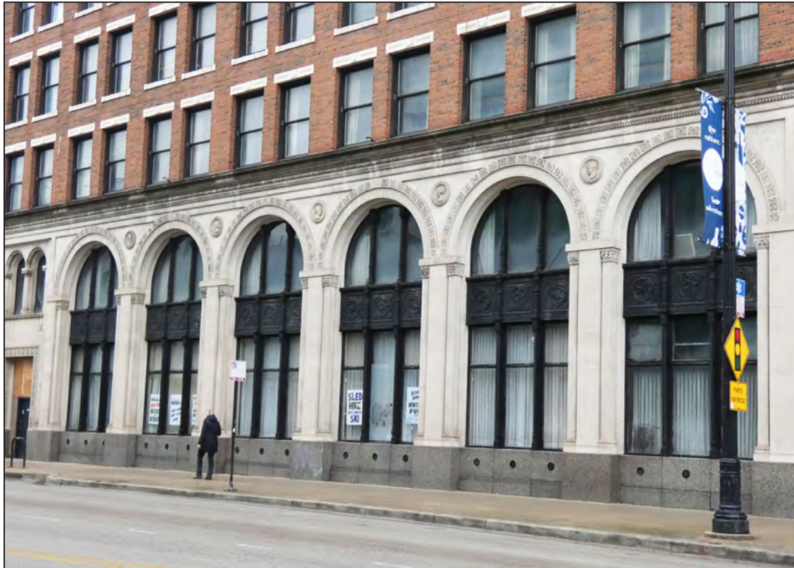
Photo 5 of 15: Halsted Street facade, looking southwest
