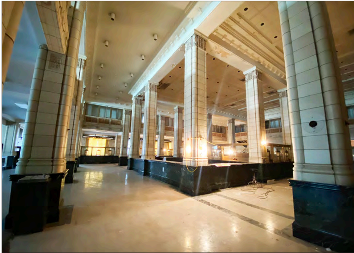
Photo 9 of 15: First floor interior, banking hall, looking southwest
