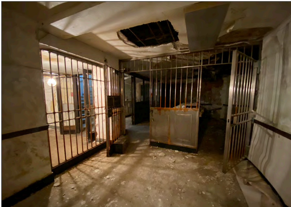
Photo 12 of 15: Basement vault lobby, looking north
