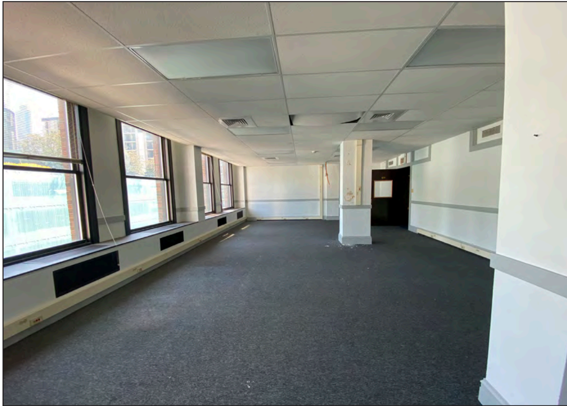
Photo 15 of 15: Typical upper floor office interior
