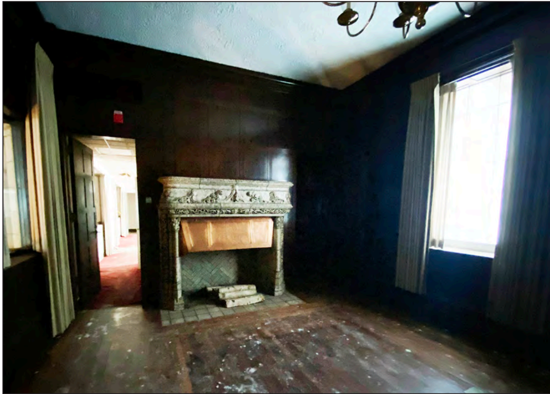
Photo 13 of 15: Second floor mezzanine interior, west executive office, looking south
