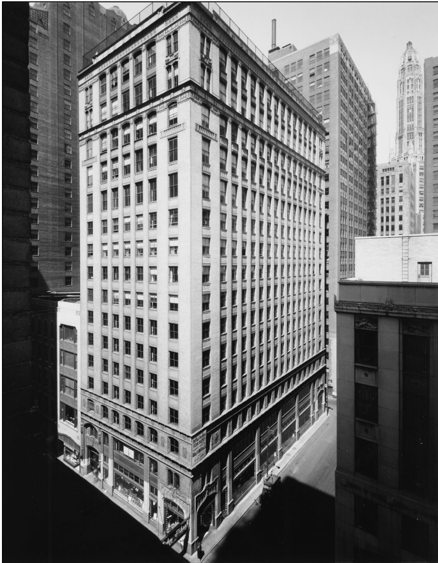
Figure 12. 1930 photograph of 64 East Lake Street, view northwest. Chicago History Museum, Hedrich-Blessing Collection.
