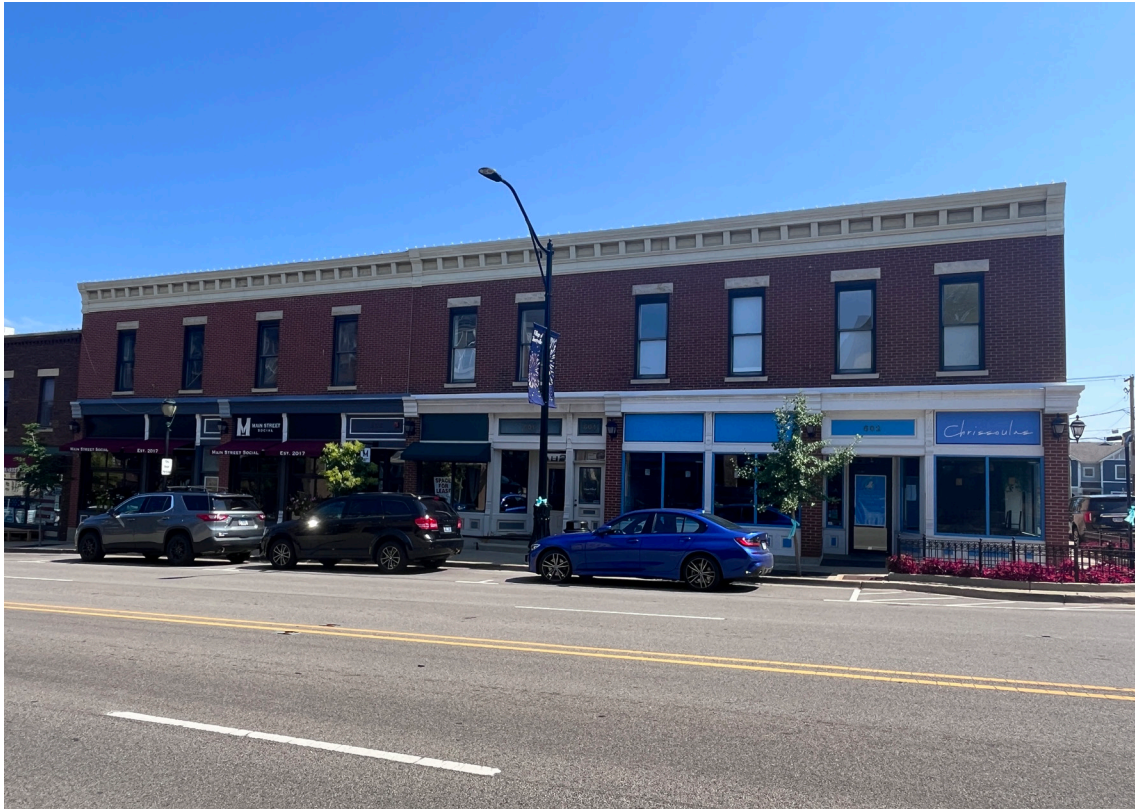
Photo 26: Bulkley Building, 602-610 N. Milwaukee Avenue, view east.
