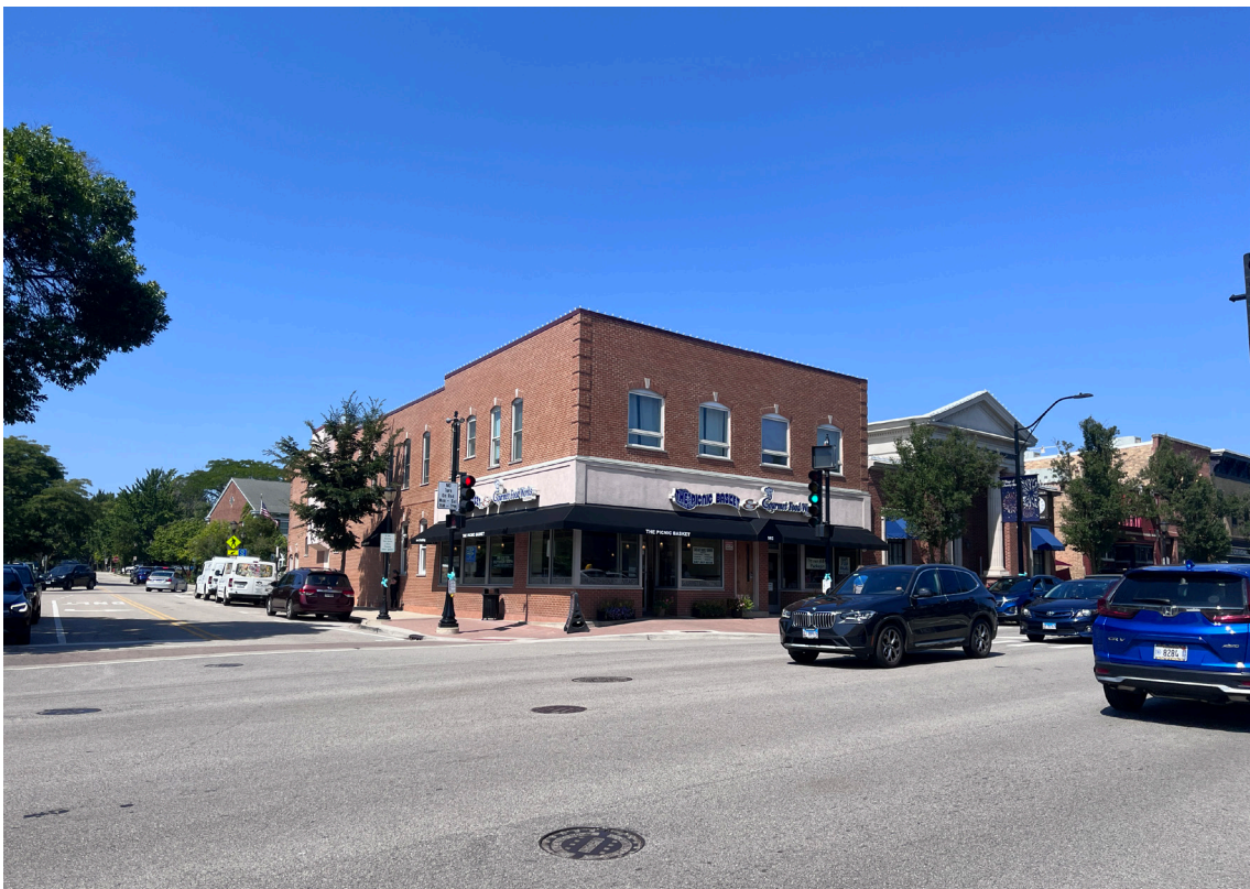
Photo 19: View west from the intersection of N. Milwaukee Avenue and Cook Avenue.
