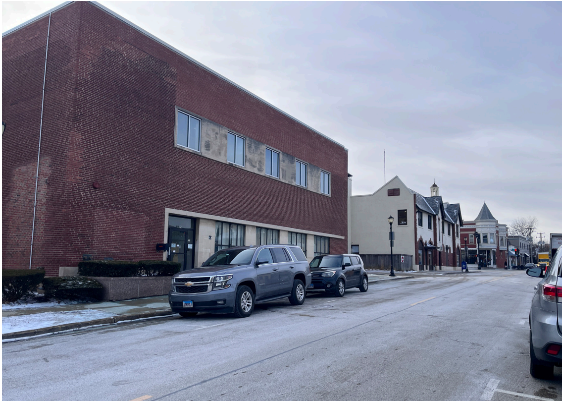
Photo 5. 100 Block of E. Church Street, south side, view southwest.
