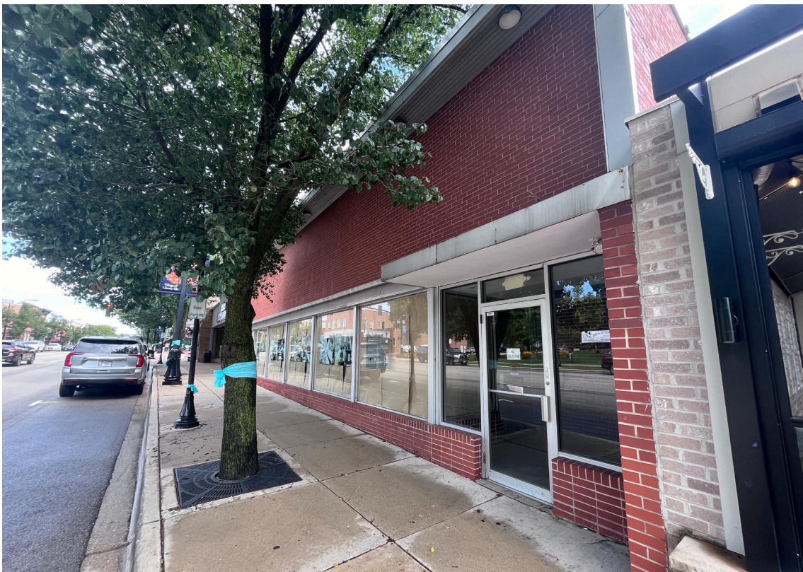
Photo 17: 416 N. Milwaukee Avenue, view northeast.
