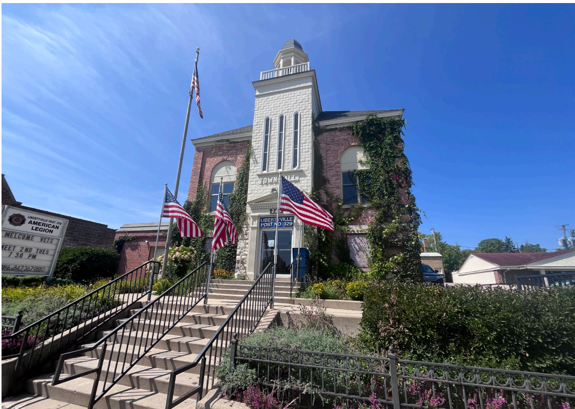
Photo 32: Libertyville Town Hall, 715 N. Milwaukee Avenue, view west.
