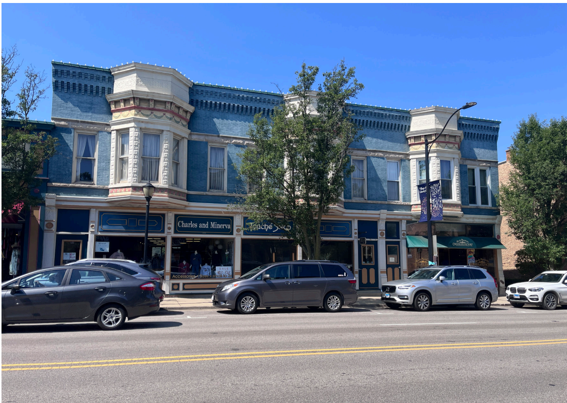
Photo 25: 535-541 N. Milwaukee Avenue, view west.
