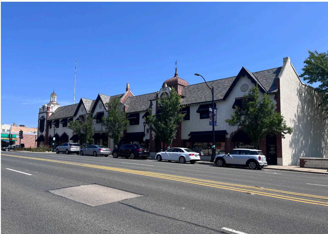
Photo 2: Public Services Building, 340-354 N. Milwaukee Avenue, view southeast.
