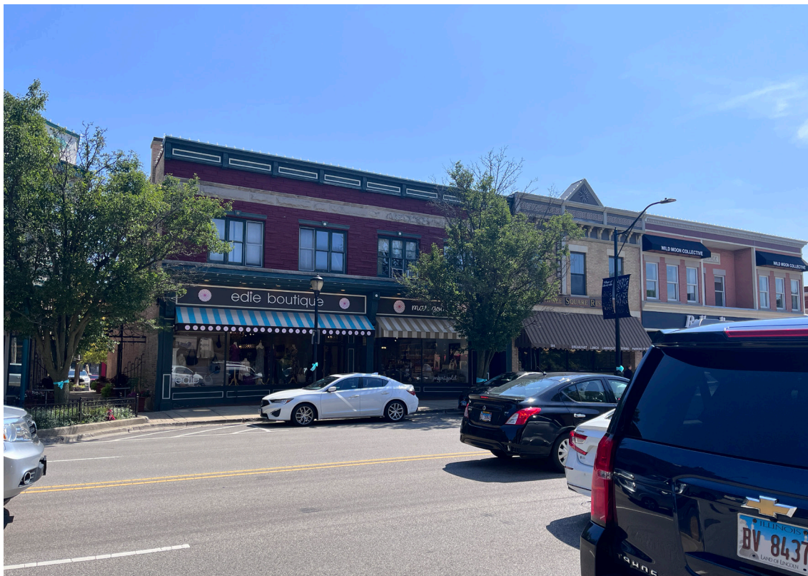
Photo 21: 500 Block N. Milwaukee Avenue, east side, view southeast.
