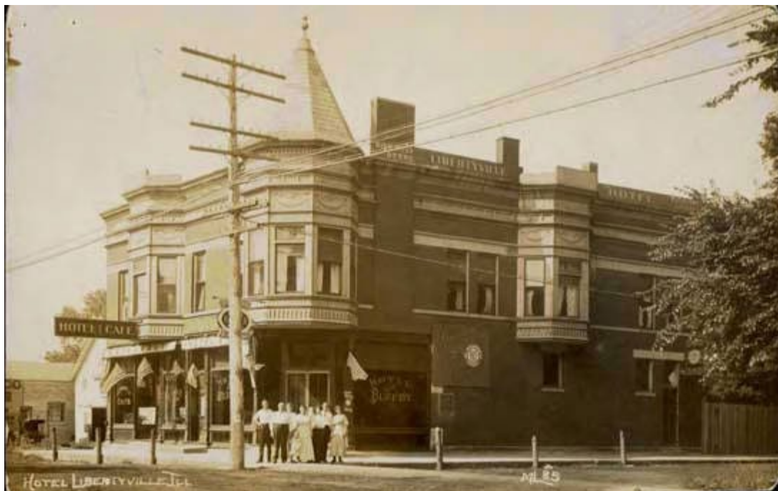
Figure 9. c. 1915 photograph of the Libertyville Hotel at the southwest corner of N. Milwaukee Avenue and W. Church Street.
