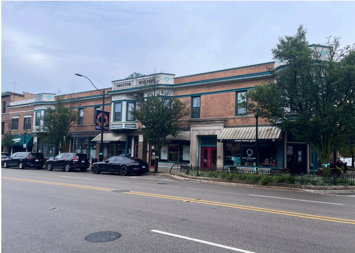
Photo 22: Proctor Building, 518-528 N. Milwaukee Avenue, view northeast.
