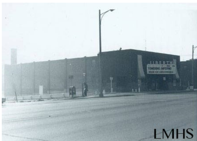
Figure 14. c. 1975 photograph of Liberty Theatre after 1960s remodeling
