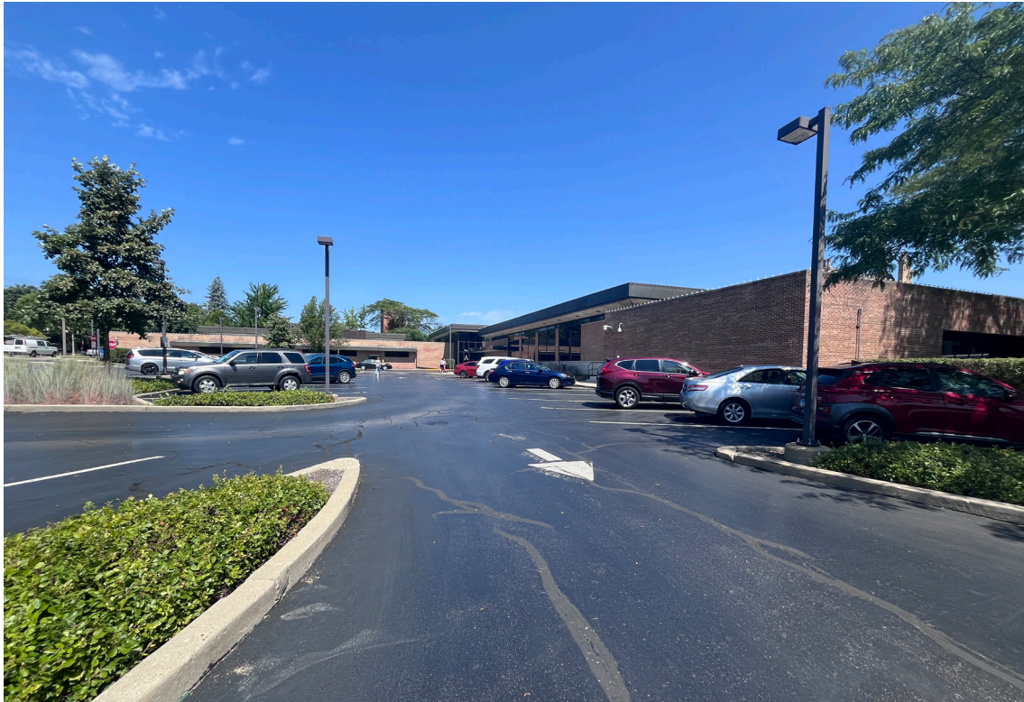
Photo 14: Cook Memorial Library, 413 N. Milwaukee Avenue, 1968 addition, south and west elevations, view north.
