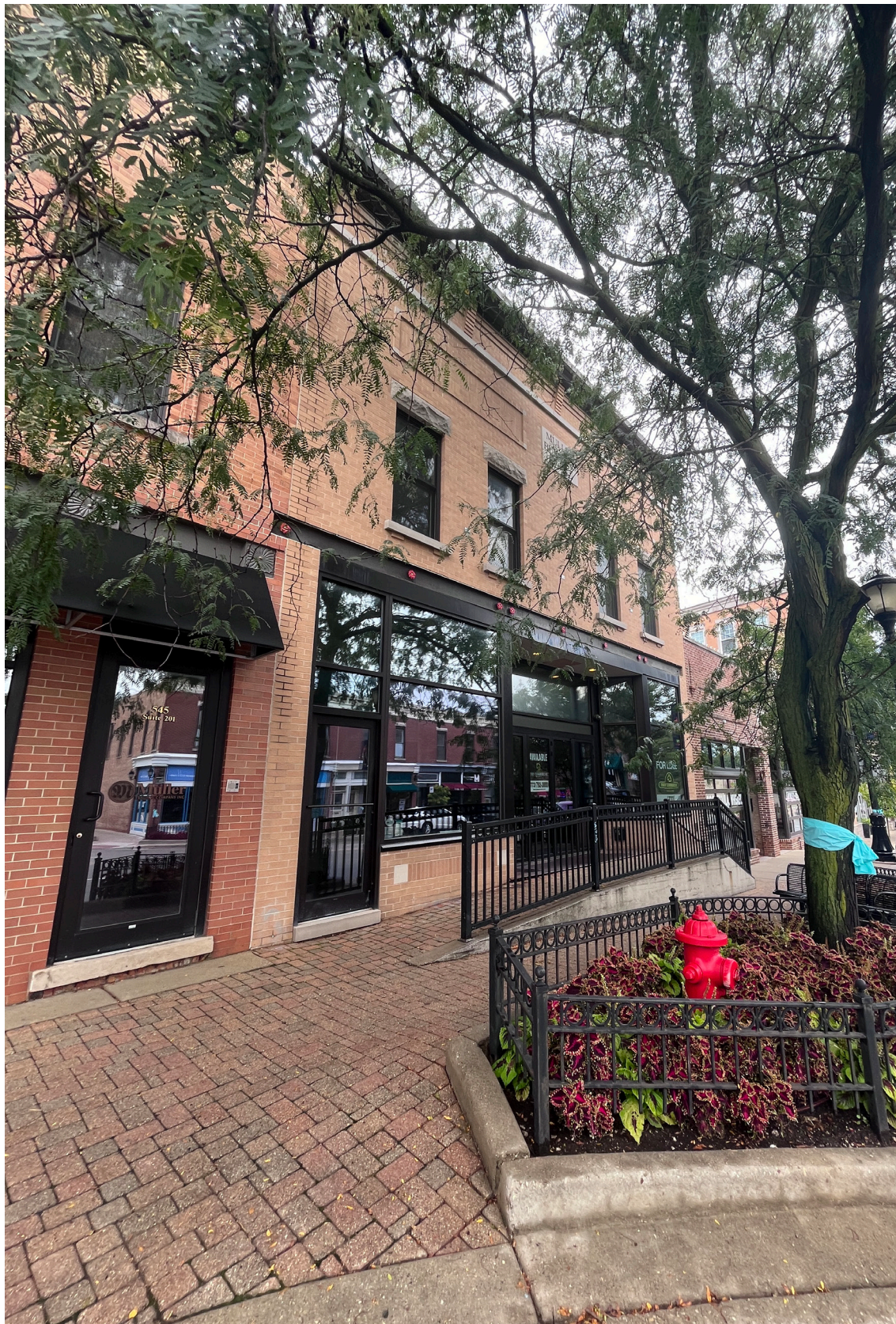
Photo 28: 600 Block of N. Milwaukee Avenue, view northwest.
