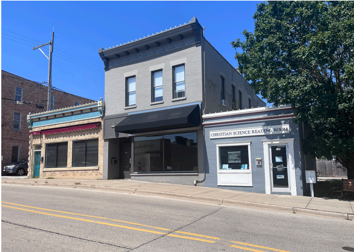
Photo 18: 100 Block of E. Cook Avenue, north side, view north.
