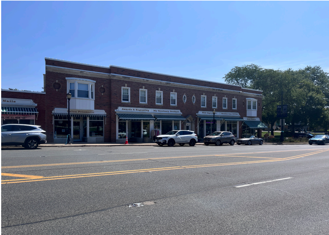
Photo 1: Bartholomay Building, 322-334 N. Milwaukee Avenue, view southeast.
