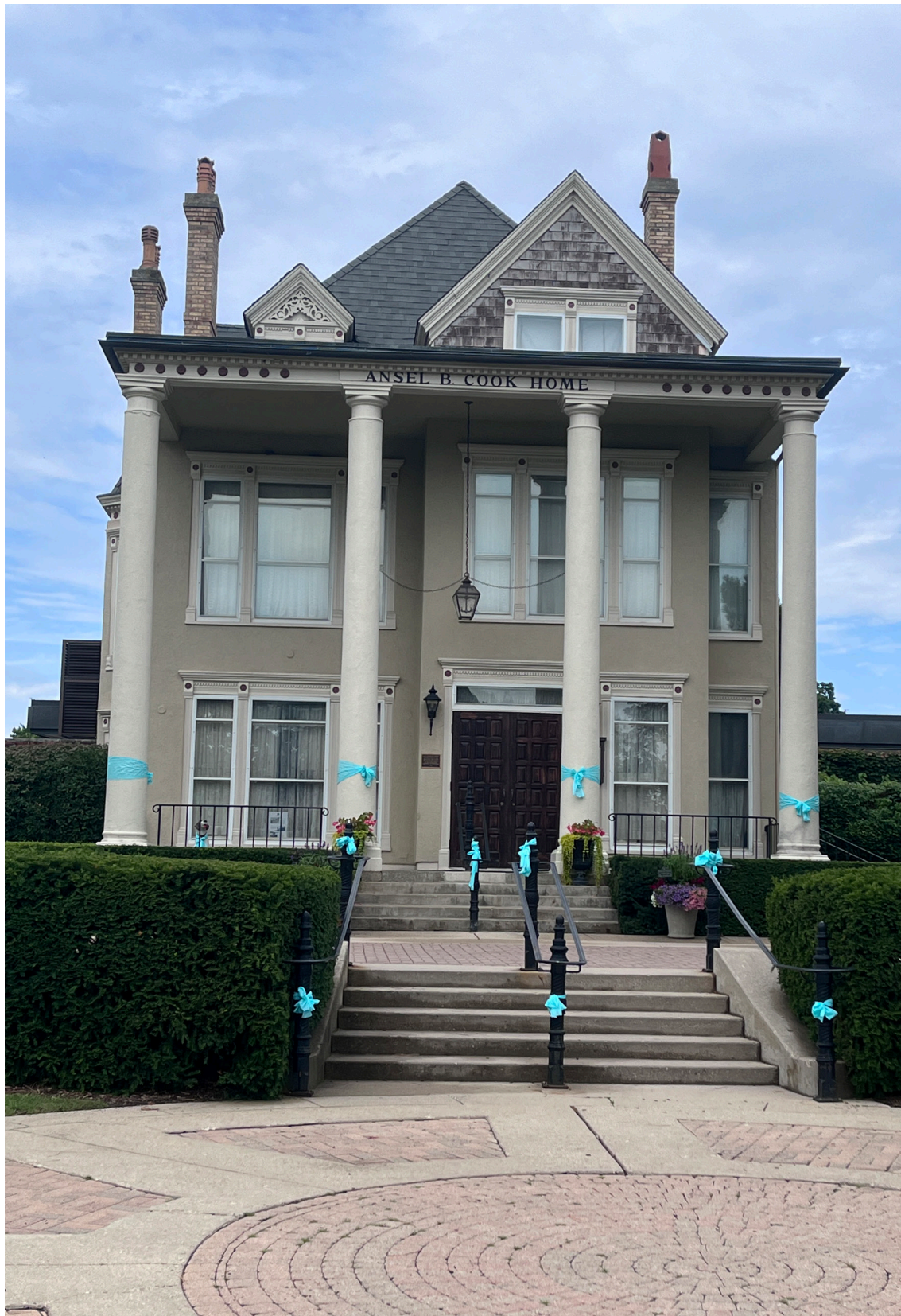
Photo 13: Ansel B. Cook House/Cook Memorial Library, 413 N. Milwaukee Avenue, view east.
