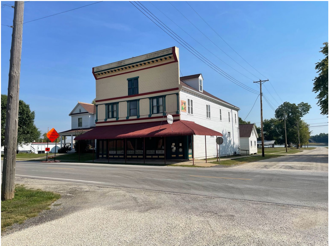
Figure 1. Historic Kamp Store. IL 100 (Broadway) is in the foreground. The shed, behind the Store, is included as part of this project and considered part of the Kamp Store.
