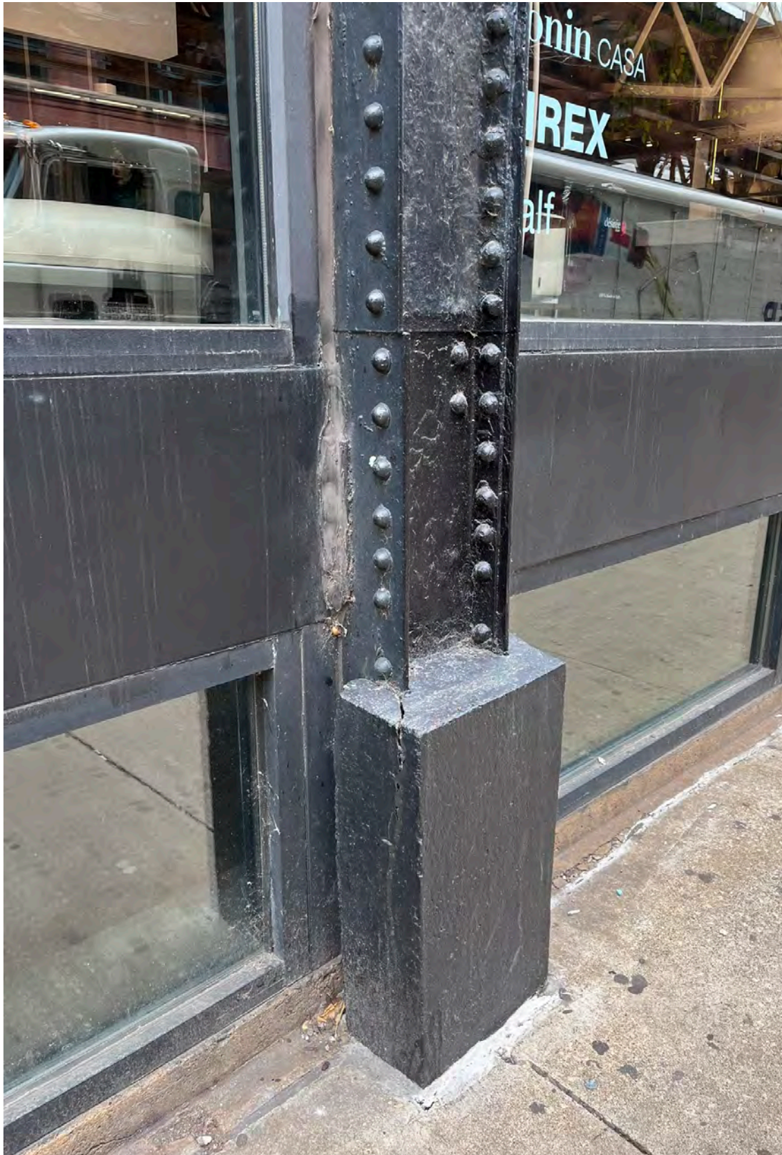
8. Detail of exposed steel girder at base of building, with window openings at basement level
