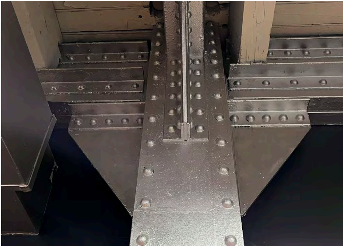
22. Detail of steel construction, typical upper floor
