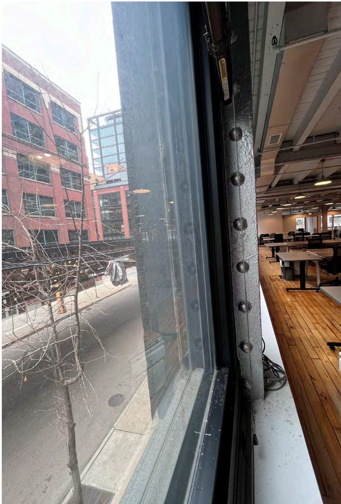
21. Detail of steel girder between window openings
