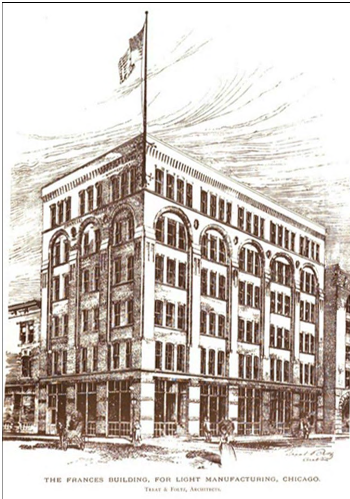
Figure 10: Frances Building, a hybrid steel and mill construction factory in Chicago designed by architects Treat & Foltz in 1889 ( Inland Architect and News Record , February 13, 1889)
