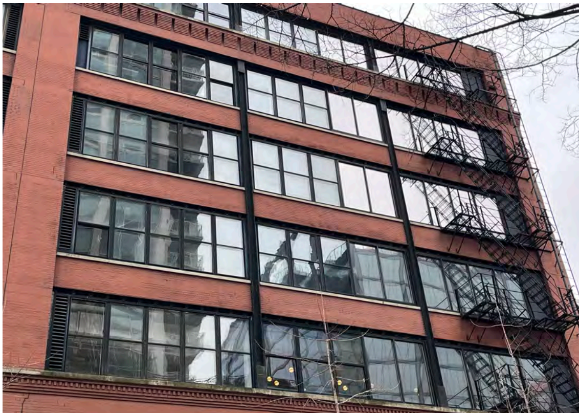
7. Upper floors, north elevation, showing exposed steel structure between large window openings
