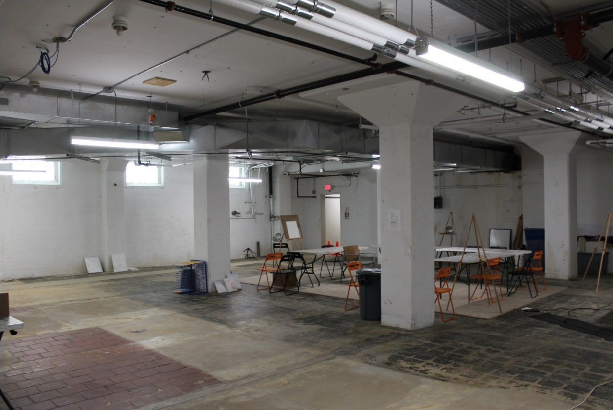
Photo 15 of 15: Interior, Basement, view looking southeast
