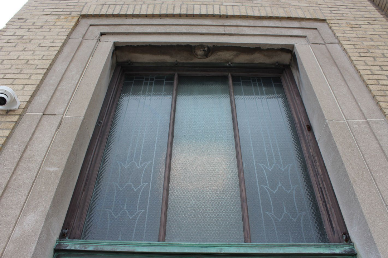
Photo 4 of 15: Exterior, east elevation, detail of historic transom at main entrance, view looking west
