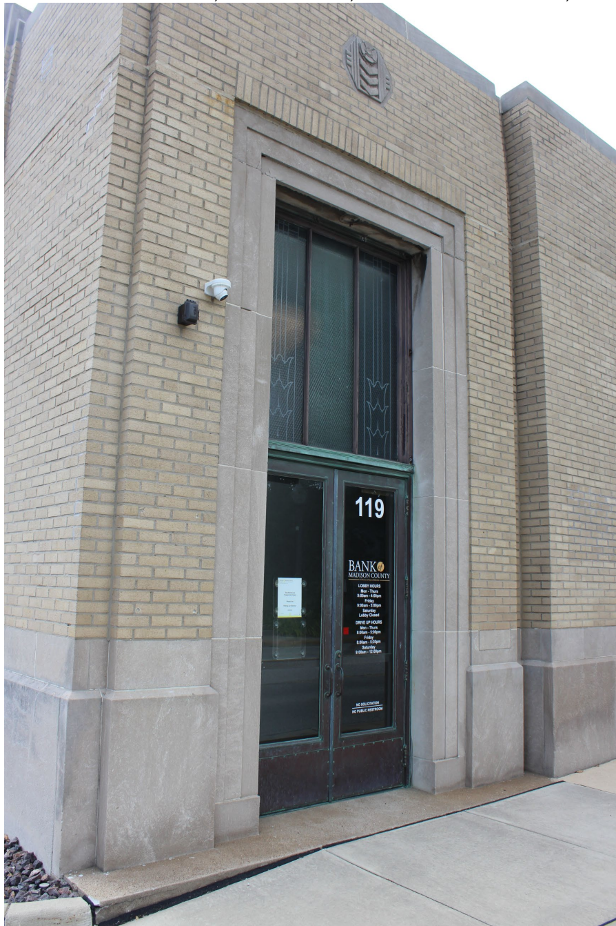
Photo 3 of 15: Exterior, east elevation, detail of main entrance, view looking west
