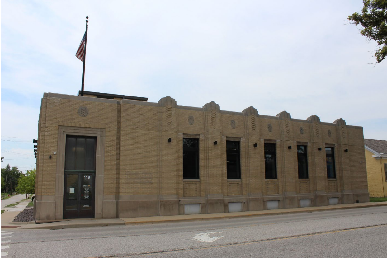
Photo 2 of 15: Exterior, east elevation, view looking west
