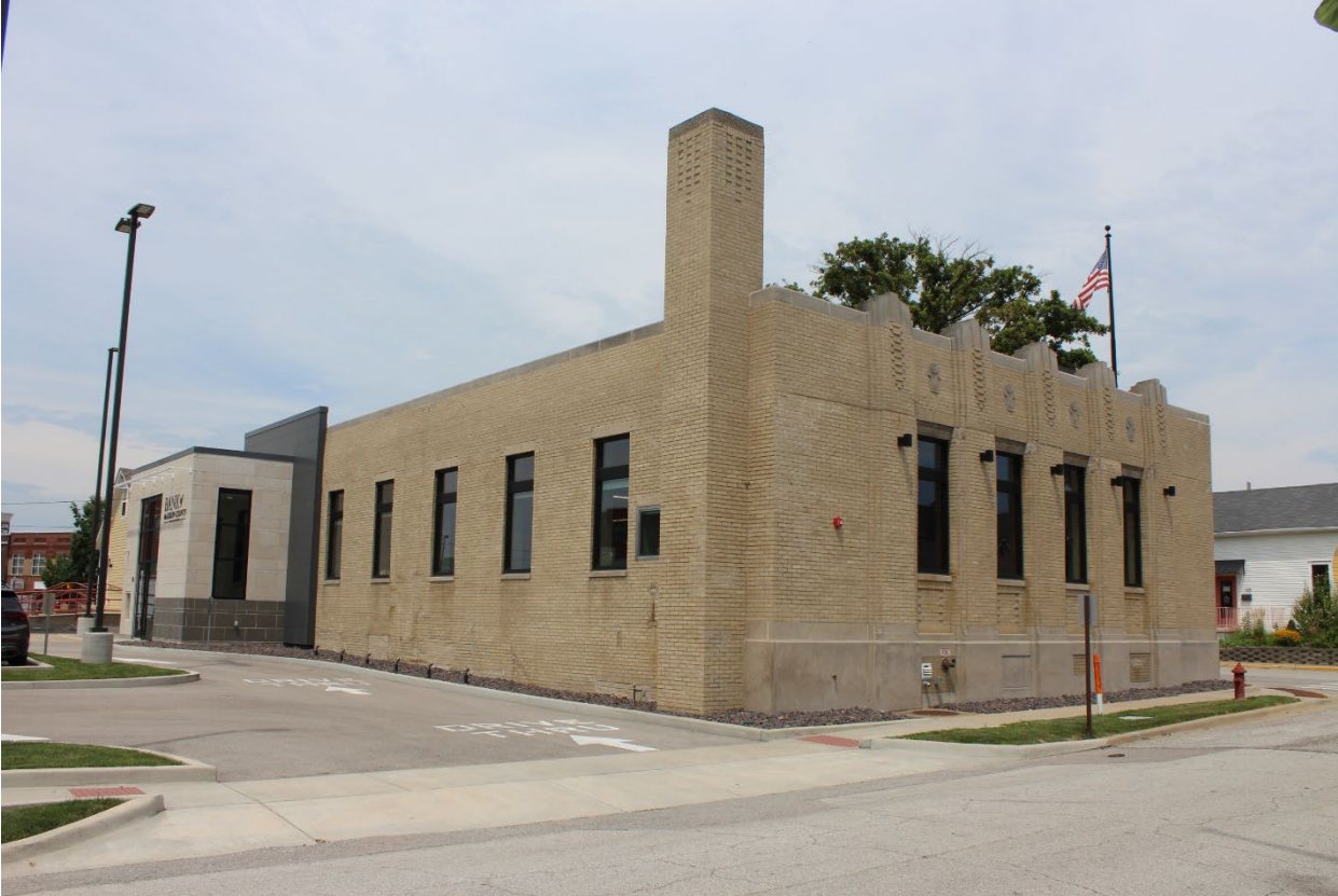
Photo 10 of 15: Exterior, west and south elevations, view looking northeast
