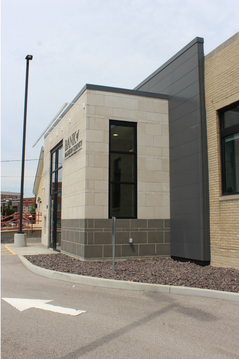
Photo 9 of 15: Exterior, west elevation, detail of addition, view looking northeast
