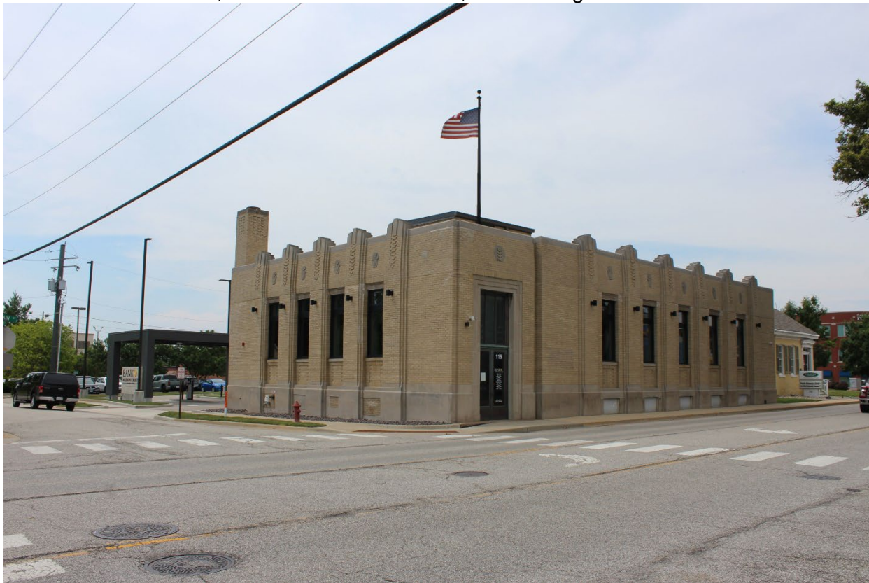
Photo 1 of 15: Exterior, south and east elevations, view looking northwest.
