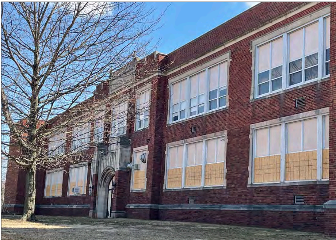
Photo 2. Grand Avenue (north) facade, looking southeast.
