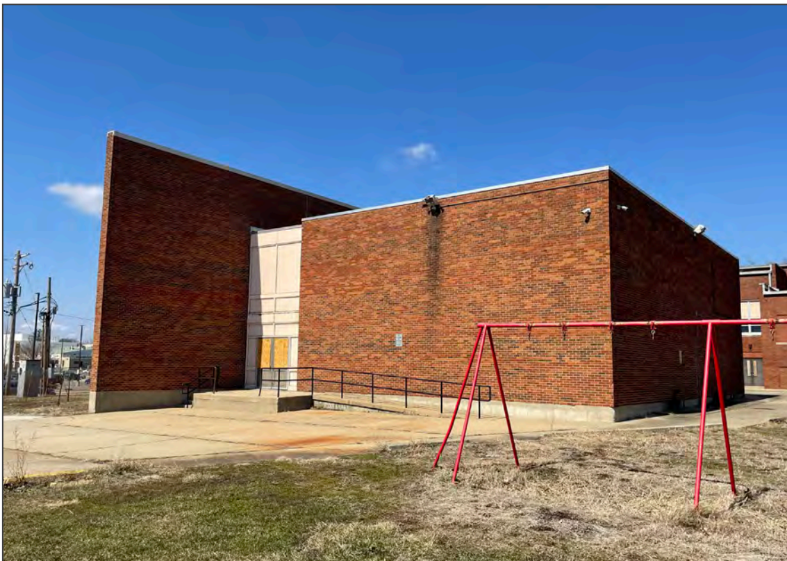
Photo 6. South facade, looking northwest.
