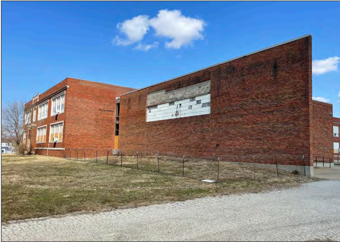
Photo 5. Oakland Avenue (west) facade, looking northeast.
