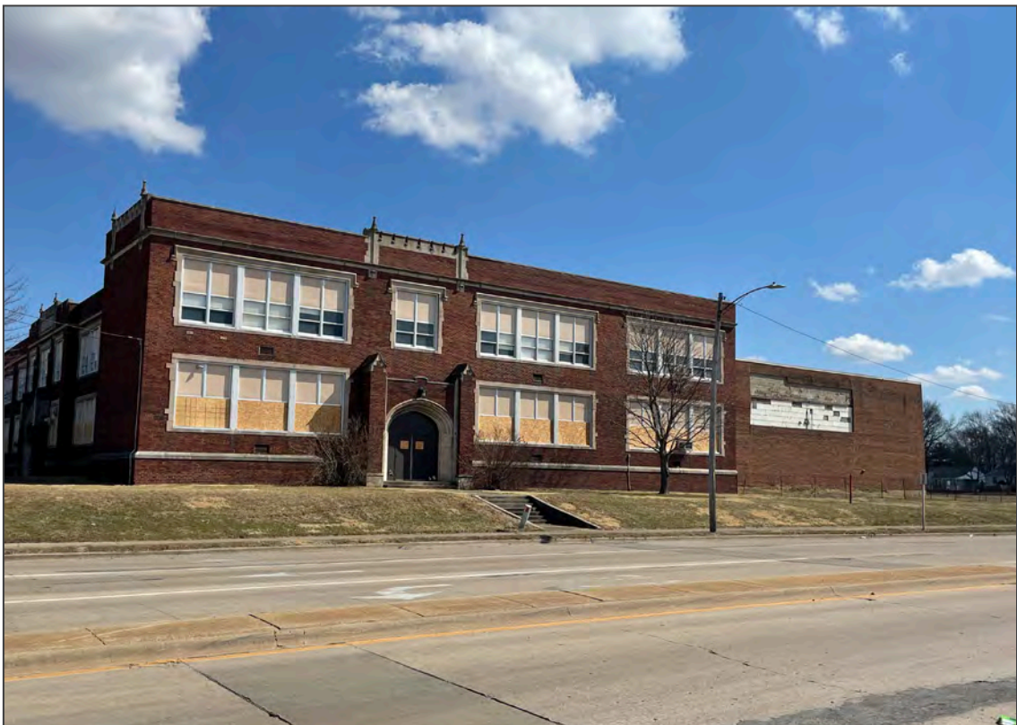
Photo 4. Oakland Avenue (west) facade, looking southeast.
