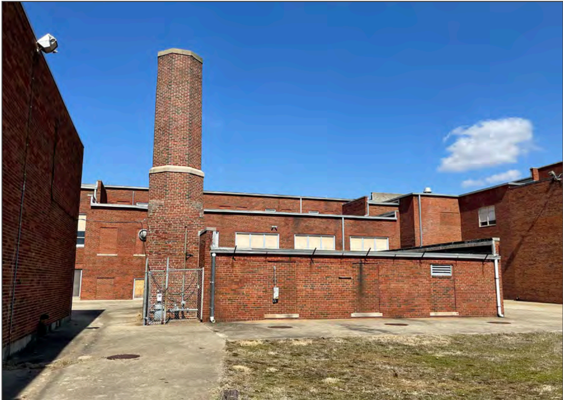
Photo 7. 1925 Powerhouse and south facade, looking north.
