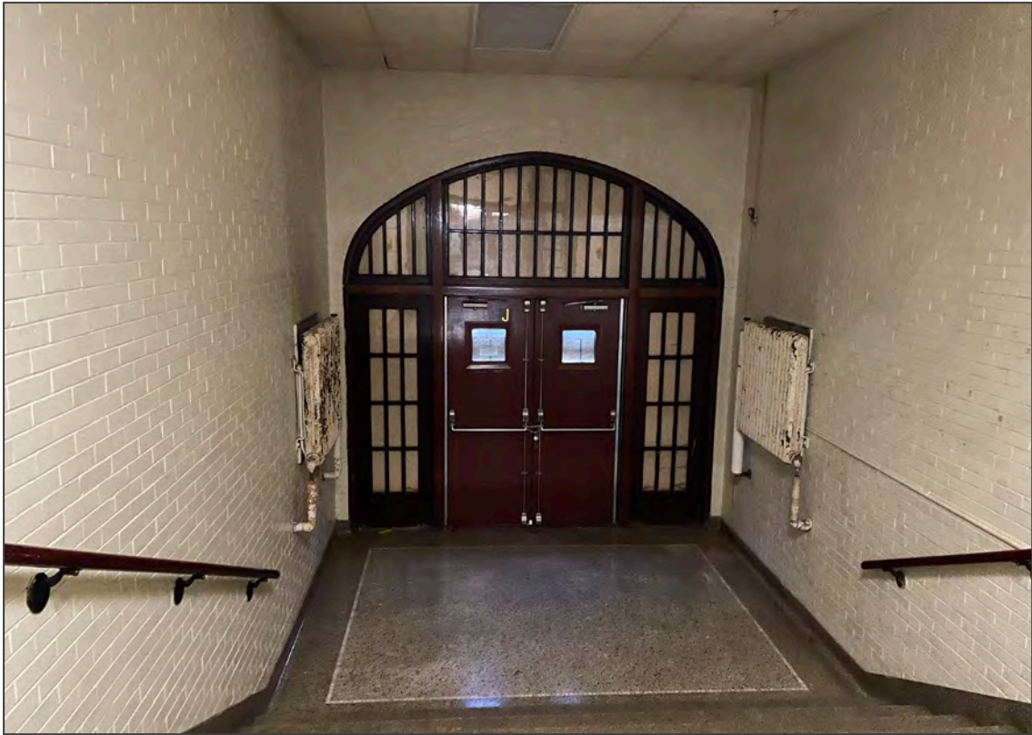
Photo 9. 1925 original block, 1st floor main entrance vestibule, looking north.
