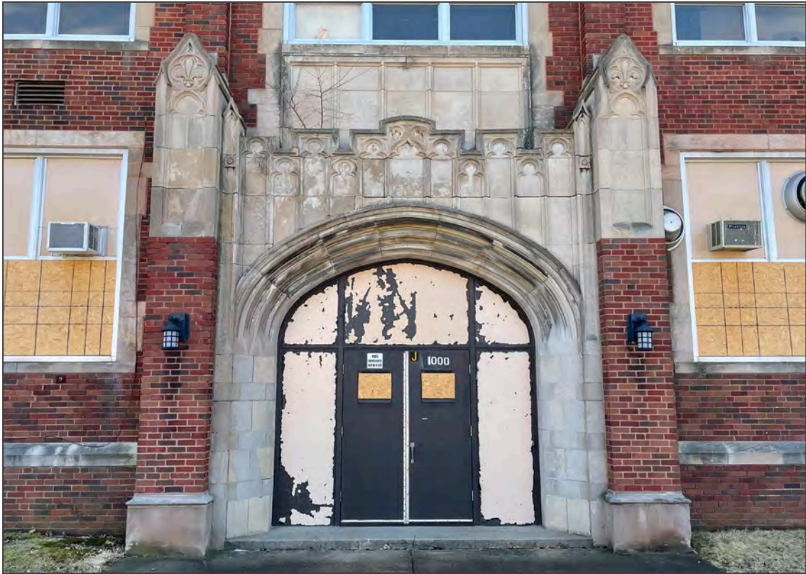
Photo 3. Grand Avenue (north) facade entrance detail, looking south.
