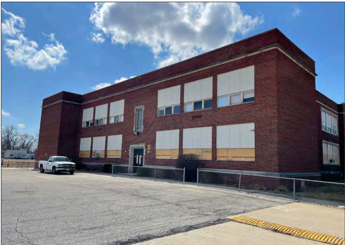
Photo 8. East facade, looking southwest.
