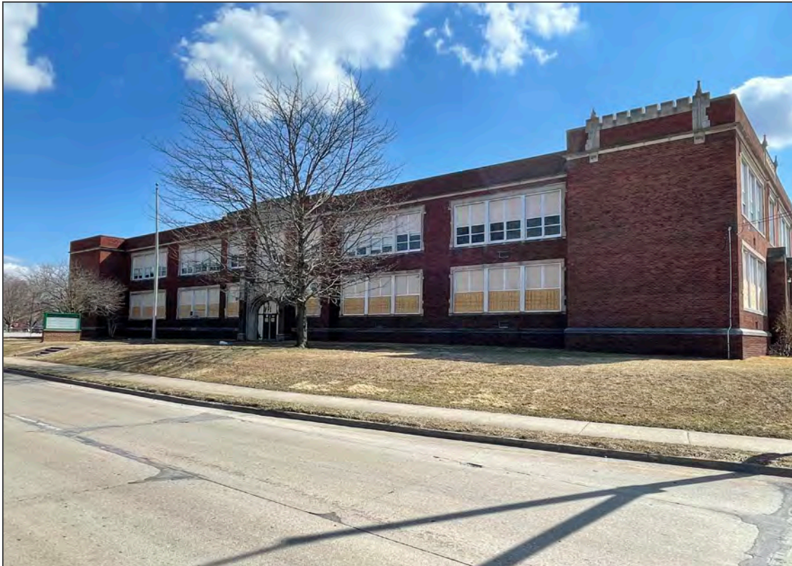
Photo 1. Grand Avenue (north) facade, looking southeast.
