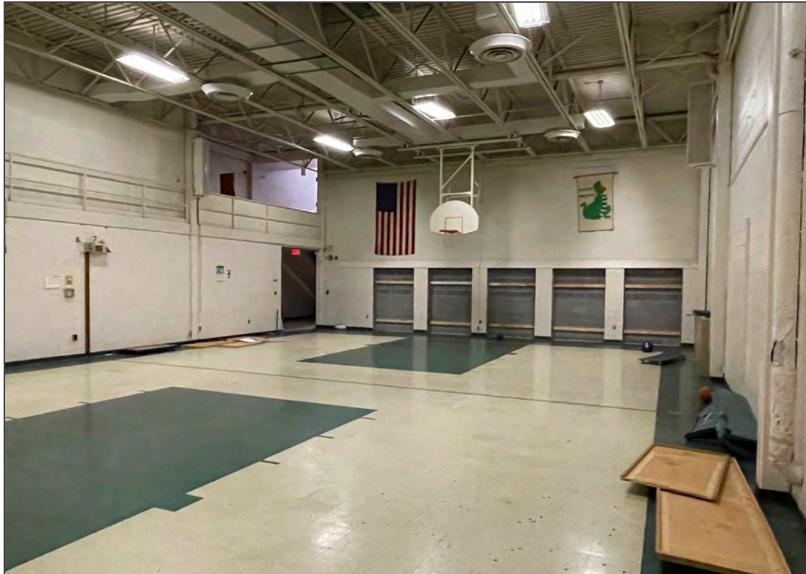
Photo 15. 1975 multi-purpose room addition, looking north.
