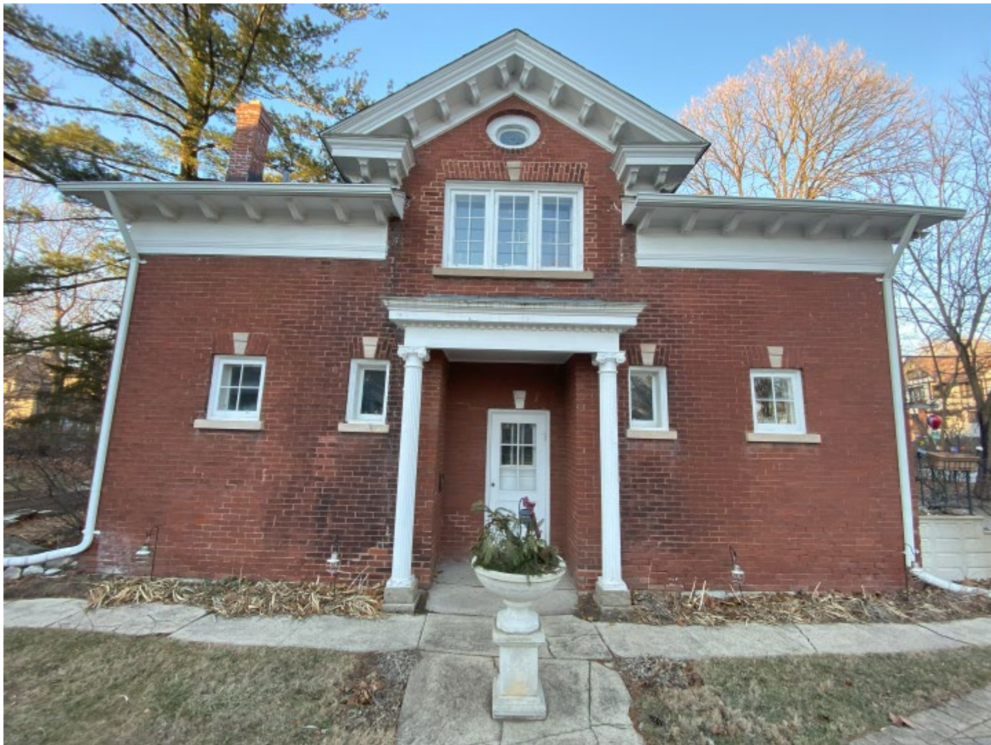
Photo 10 of 23: View of south face of carriage house
