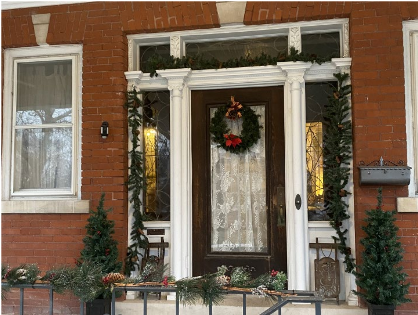
Photo 7 of 23: View of main entrance from porte-cochere
