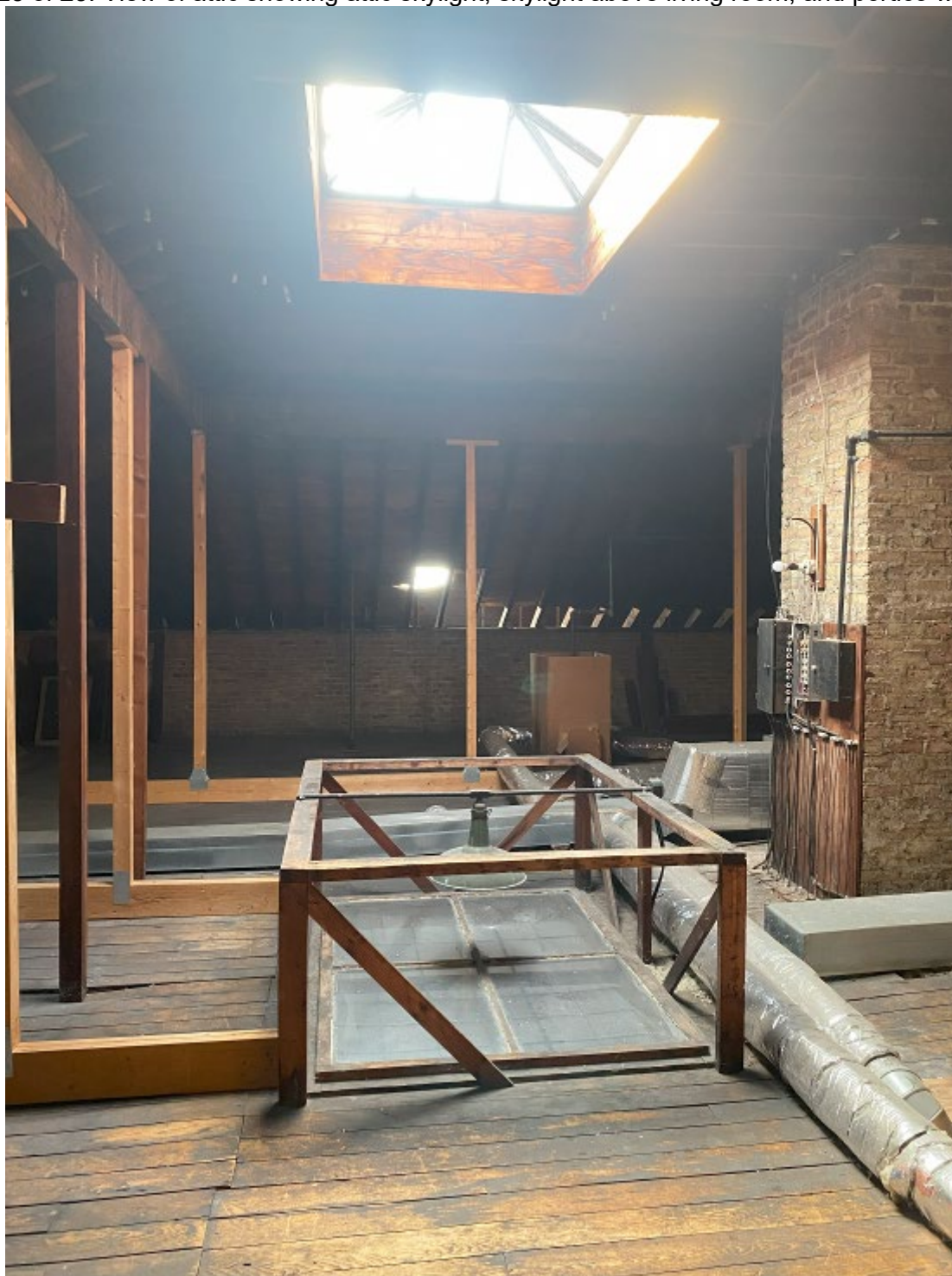
Photo 23 of 23: View of attic showing attic skylight, skylight above living room, and portico window in distance
