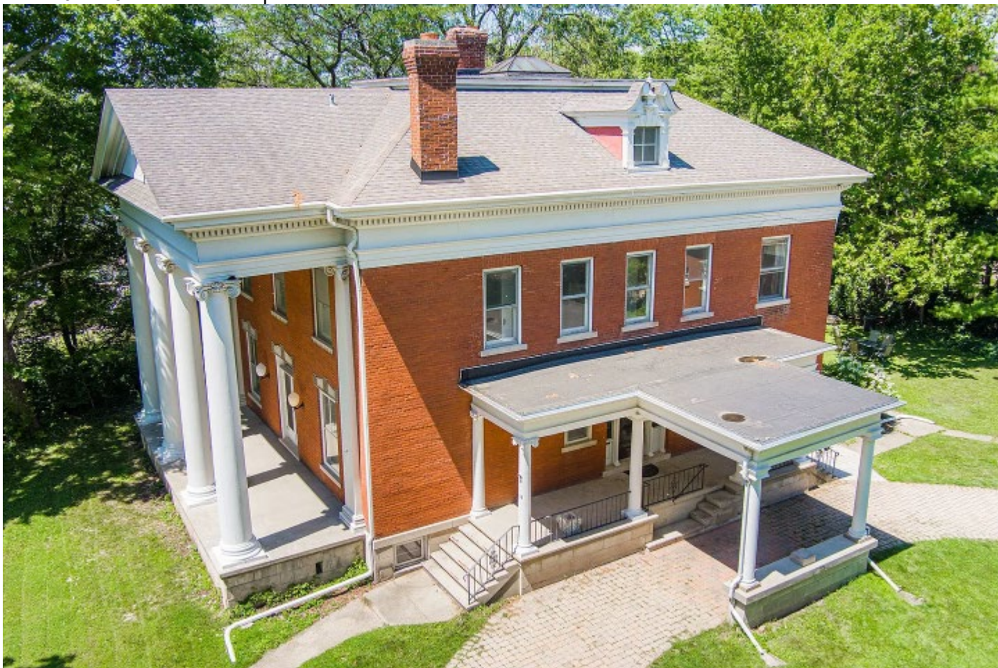
Photo 6 of 23: Aerial view of portico and east face of mansion
