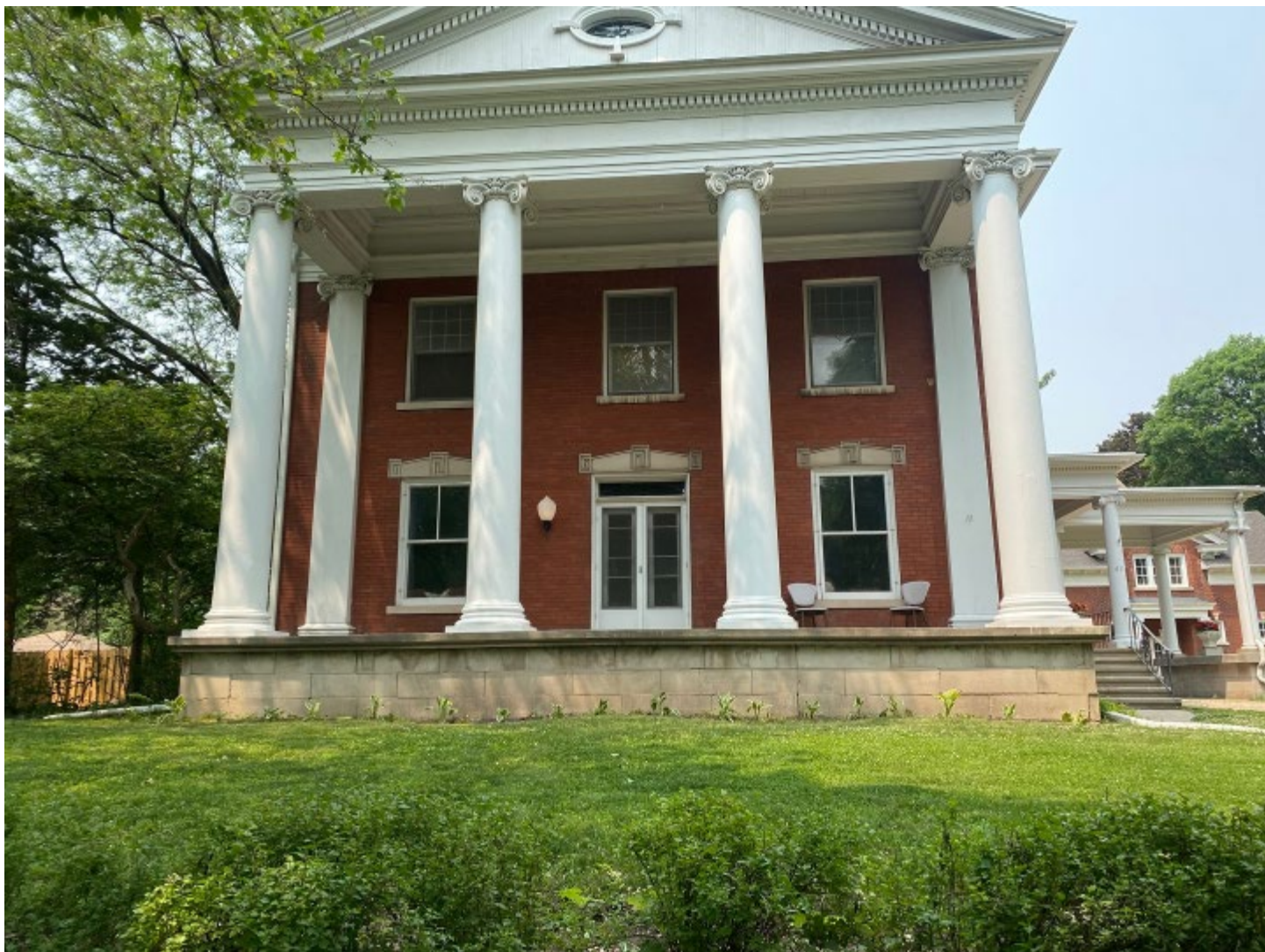
Photo 2 of 21: View of Portico taken from sidewalk along College Avenue
