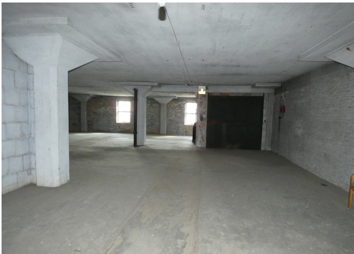
14. Typical upper floor interior, looking east to freight elevator
