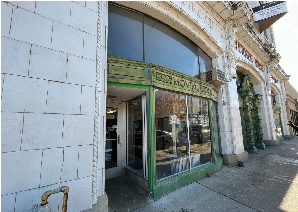
5. West elevation, north storefront, looking southeast
