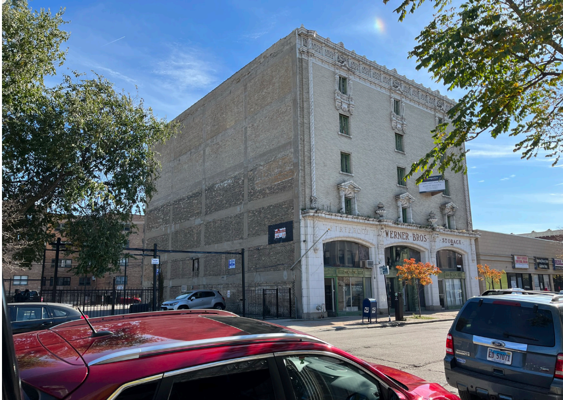
2. West and north elevations, looking southeast
