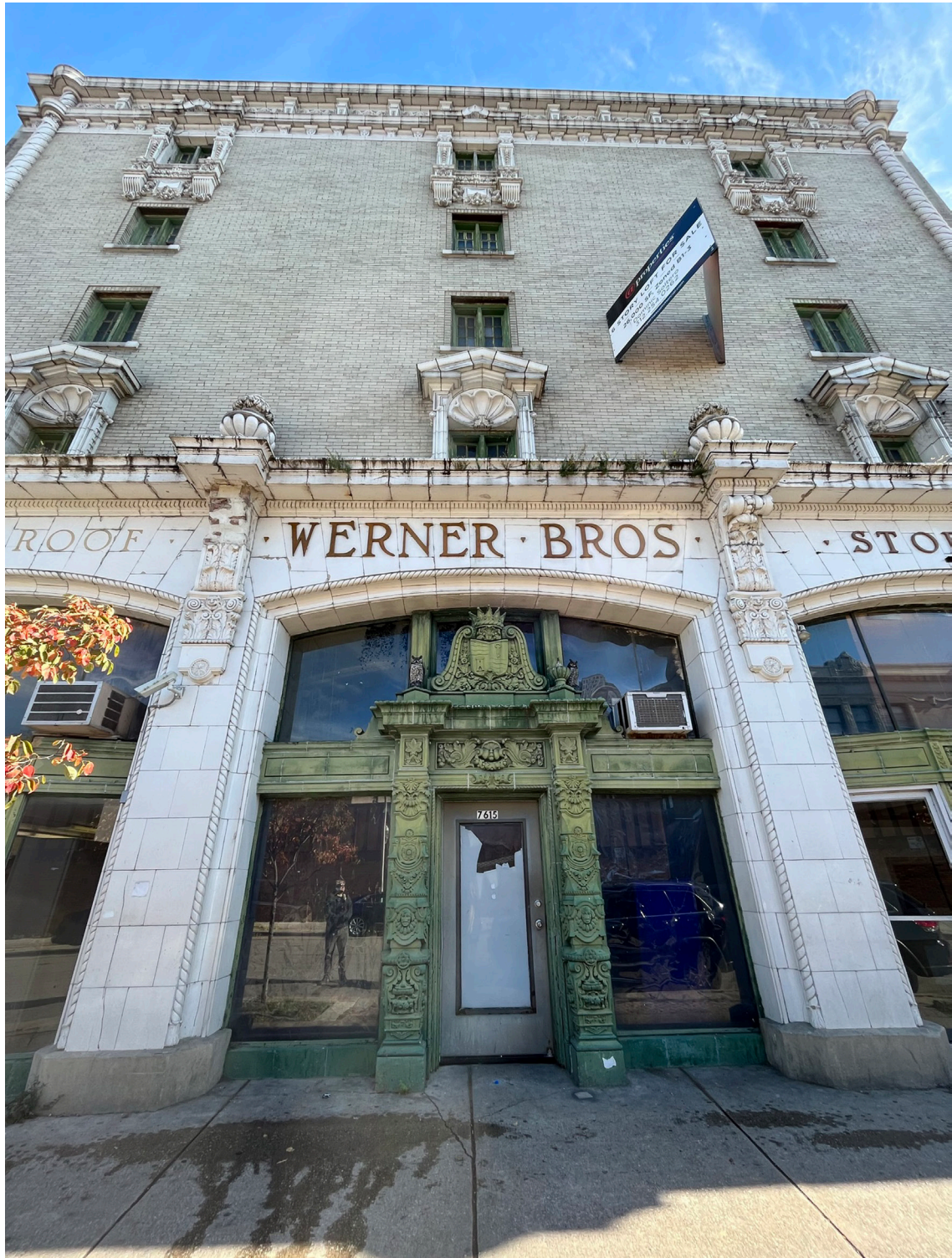
4. West elevation, entrance detail, looking east
