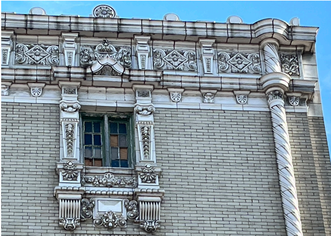
7. West elevation, parapet detail, looking east
