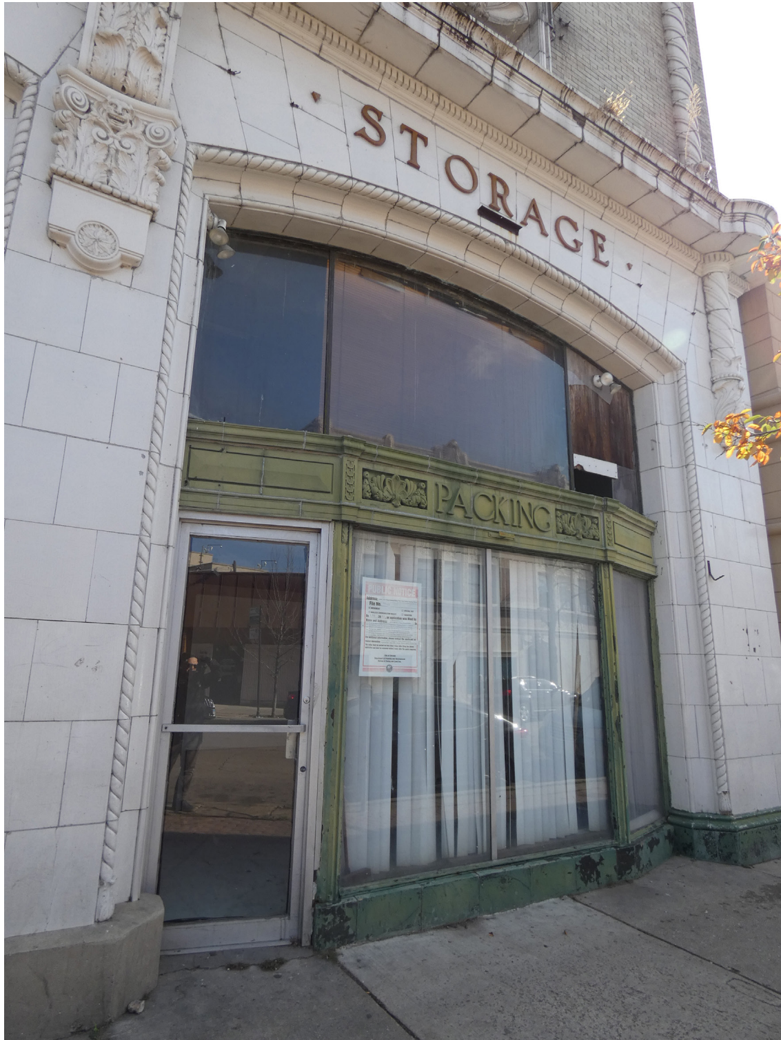
6. West elevation, south storefront, looking southeast
