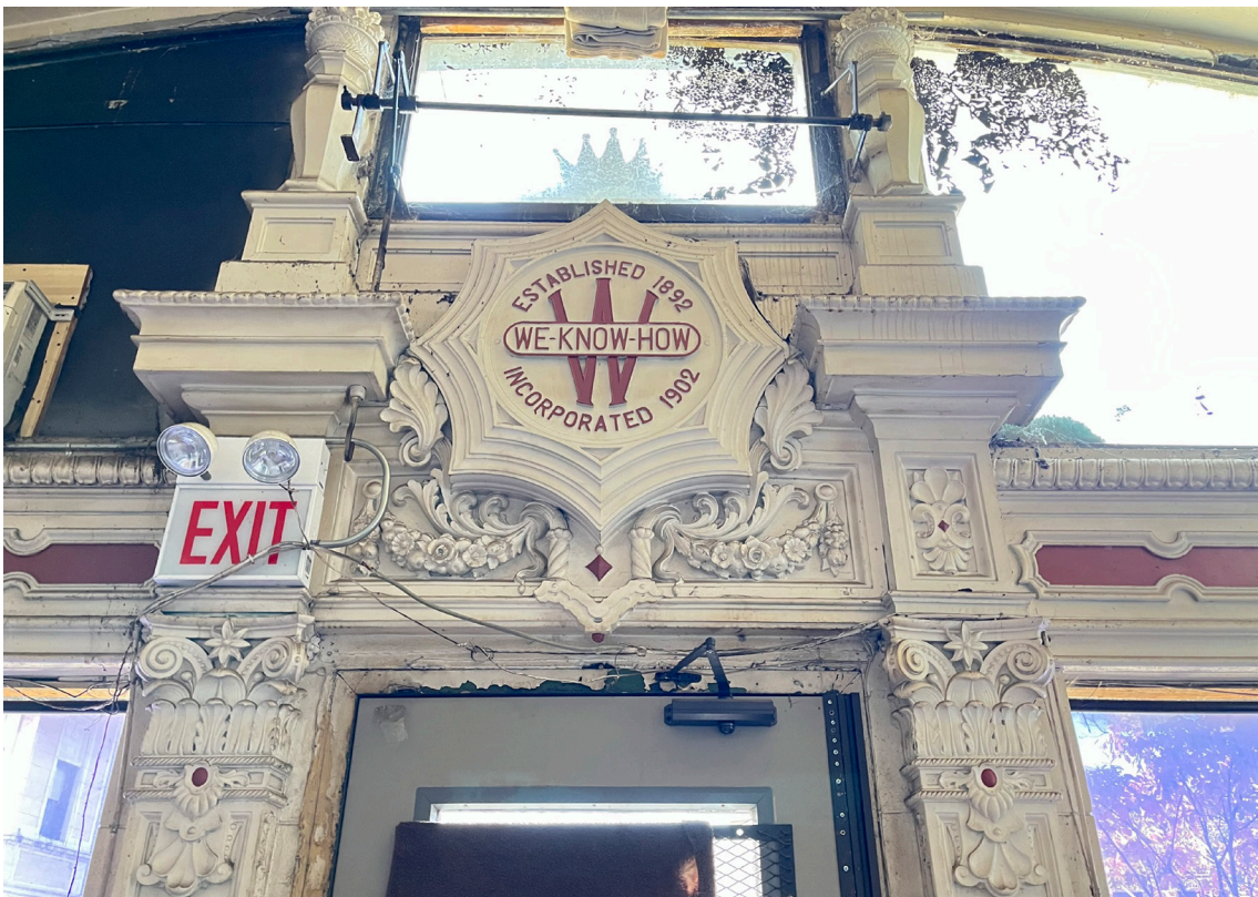
10. First floor lobby, entrance detail, looking west
