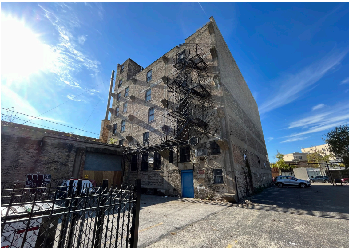
3. North and east elevations, looking southwest
