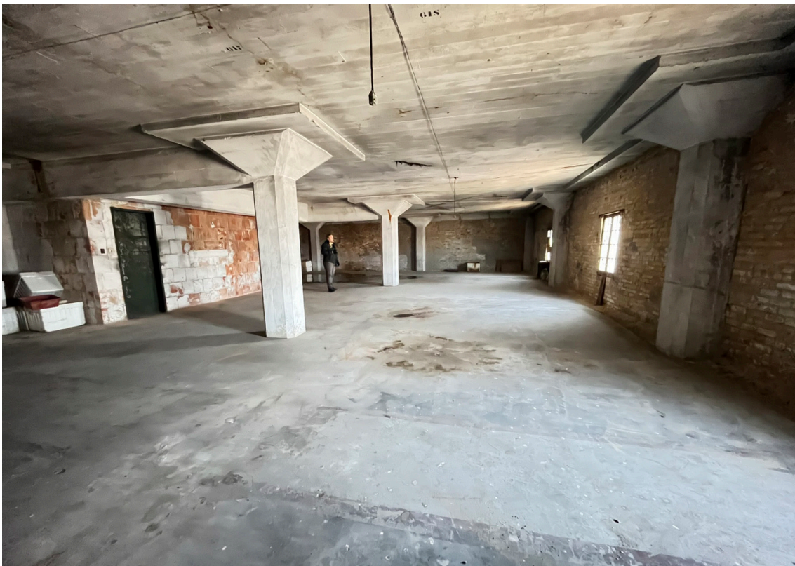
13. Typical upper floor interior, looking south with center stair/elevator at left
