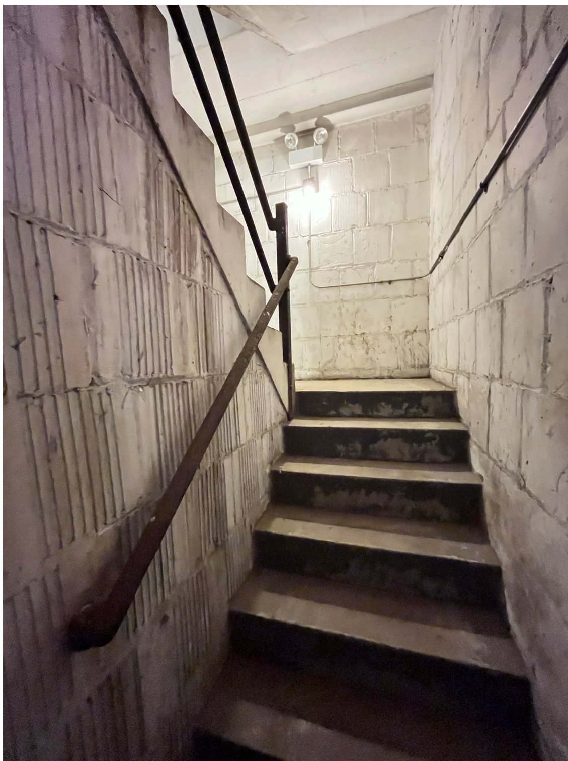
11. Interior stair, looking north
