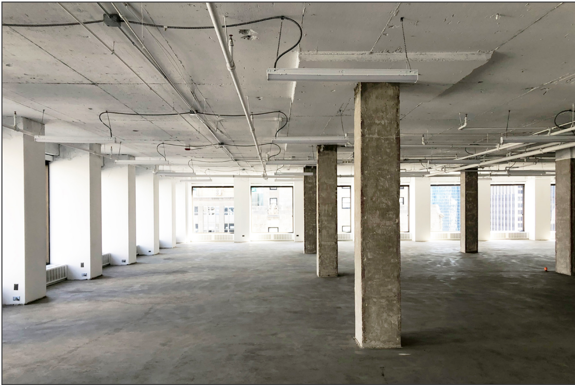
16. Typical unfinished office space showing exposed concrete structure – looking east
