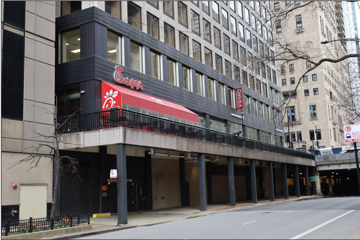
4. South elevation, showing original upper level sidewalk on Illinois Street completed with building in 1968 – looking northeast.
