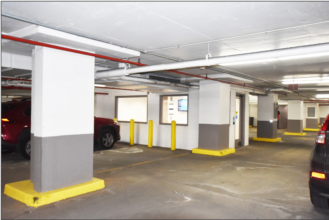
8. Lower Level 2, parking garage – looking southwest
