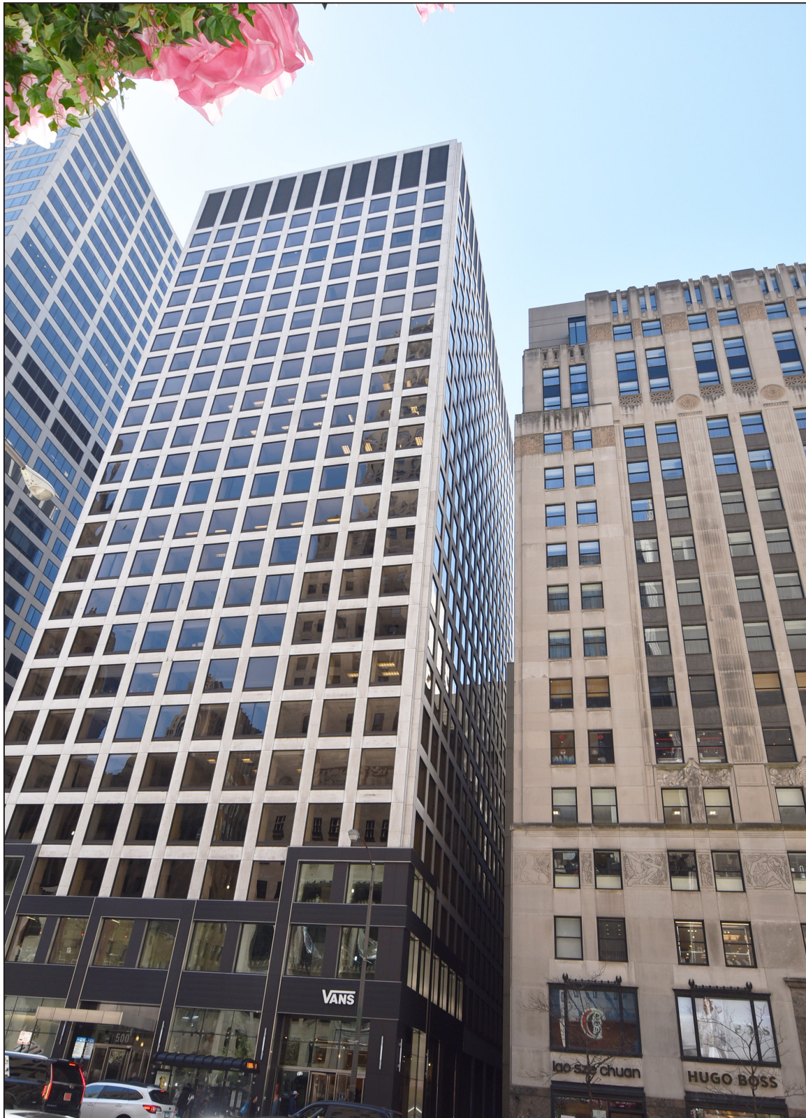
2. East and north elevations – looking southwest
