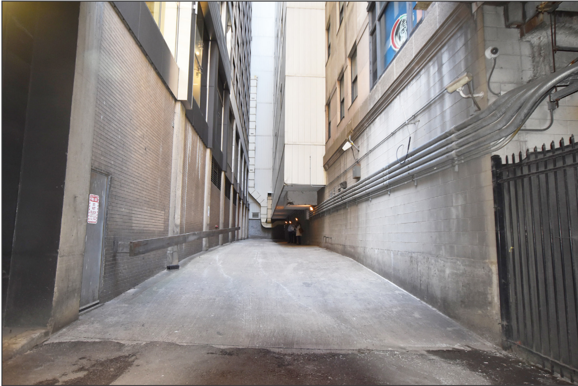
6. North elevation, on the lower public alley showing the Lower Level (LL1) of the north elevation (left) – looking west along alley from lower Michigan Avenue.
