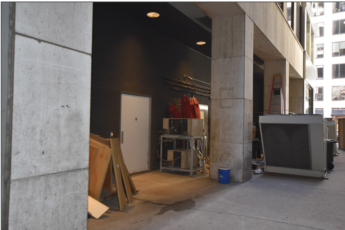
5. West elevation, on rear plaza and arcade – looking southeast.
