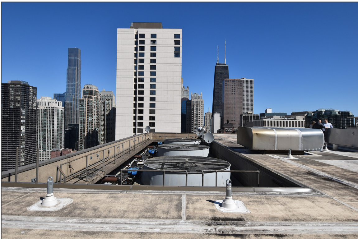
7. Roof – looking north from the southwest corner
