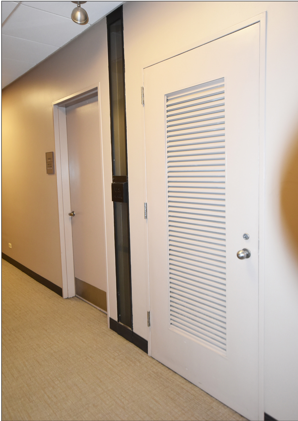
14. Typical corridor, showing detail of original mail chute – looking northwest.
