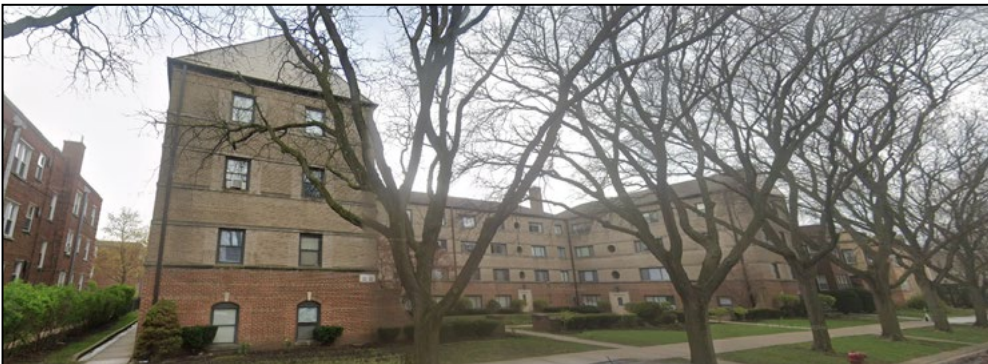
Figure 118. 2213-2231 W. Morse Avenue. Source: April 2025 Google Street View.
