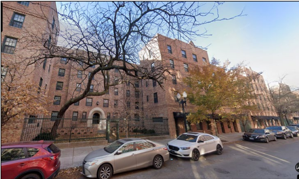
Figure 106. Marshall Field Garden Apartments. Source: November 2025 Google Street View.
