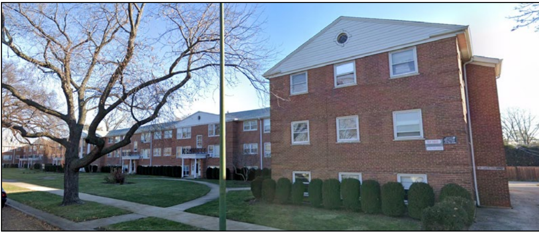
Figure 139. Williamsburg Apartments. Source: November 2018 Google Street View
