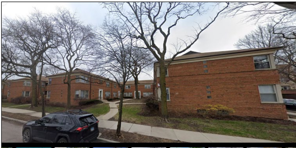
Figure 126. 2104-2112 W. Foster Avenue. Source: May 2025 Google Street View..
