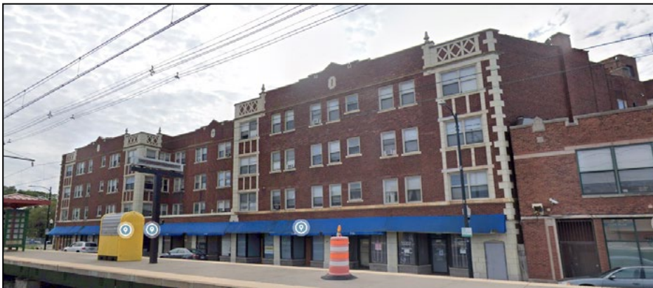
Figure 64. Yates Apartments, Exchange Avenue (east) facade. Source: October 2025 Google Street View.
