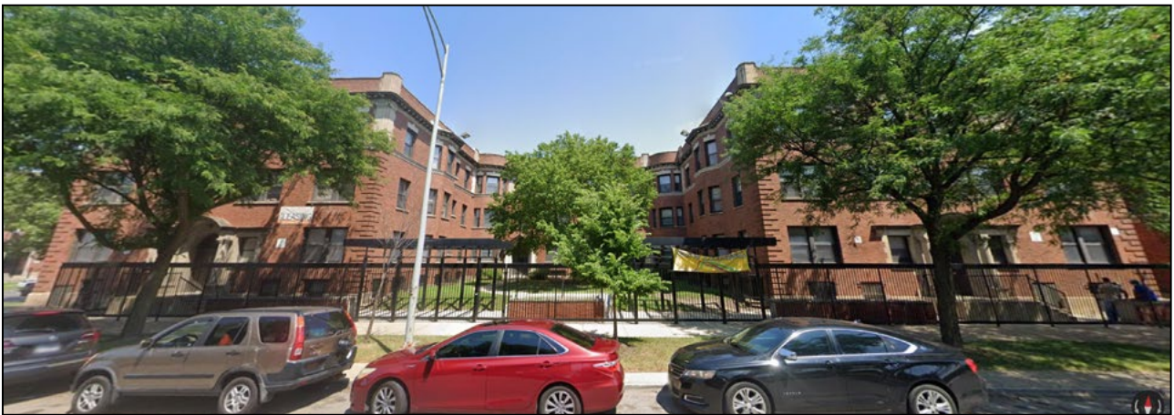
Figure 33. 200-216 E. Garfield Boulevard. Source: July 2025 Google Street View.
