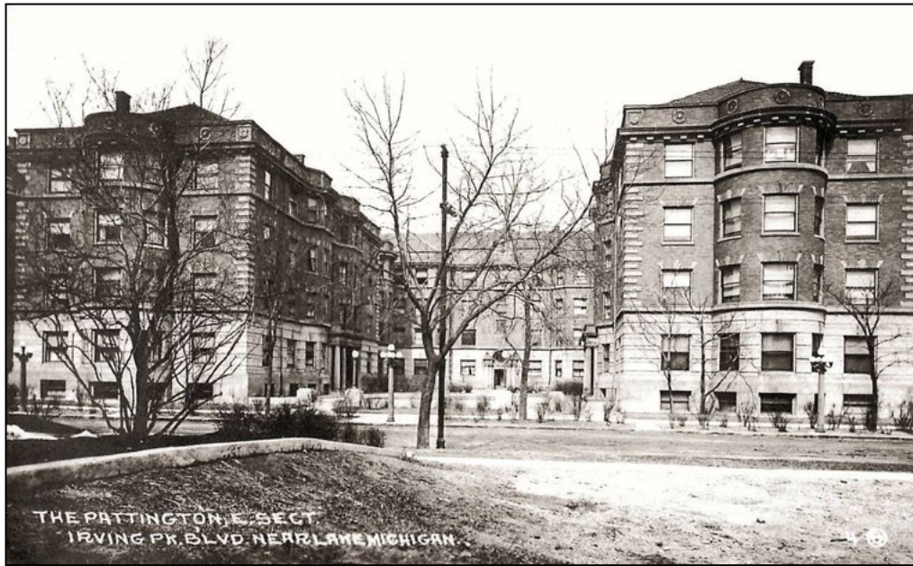
Figure 27. The Pattington, a well-known early example of a luxury courtyard apartment building. Source: Chuckman's Chicago website.
