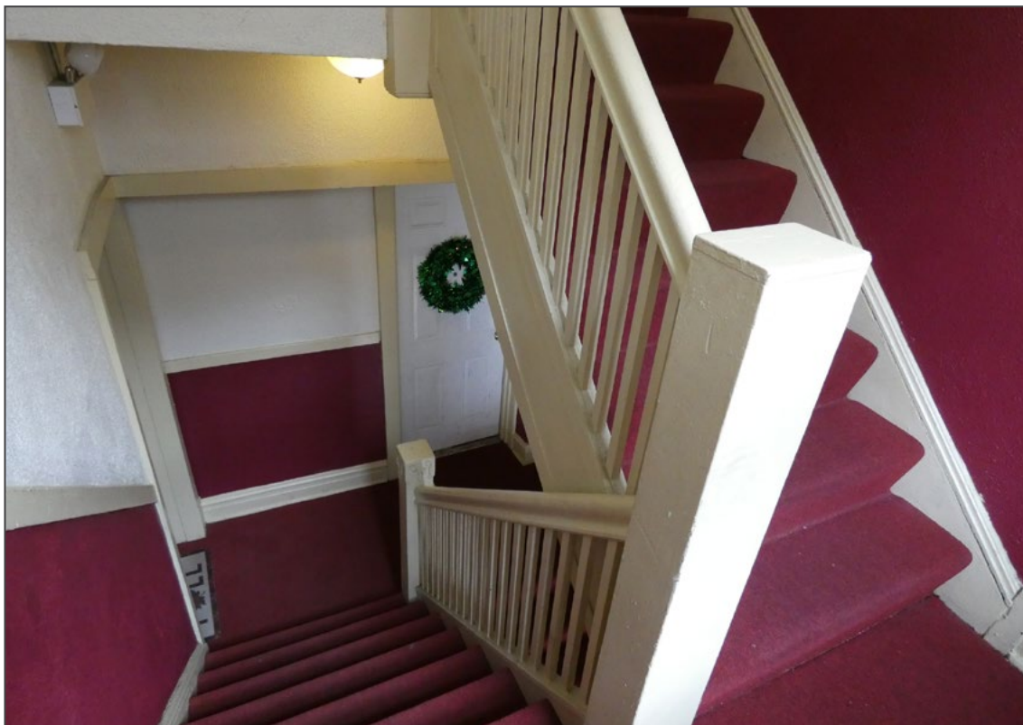
Photo 11. 5113 W. Washington Boulevard - upper floor stairwell, looking east at typical apartment entry landing.
