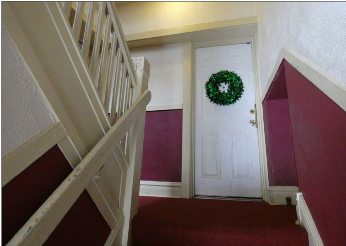
Photo 10. 5113 W. Washington Boulevard - upper floor stairwell, looking east at typical apartment entry landing.
