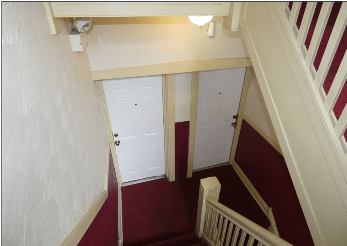
Photo 12. 5115 W. Washington Boulevard - upper floor stairwell, looking east at typical apartment entry landing.
