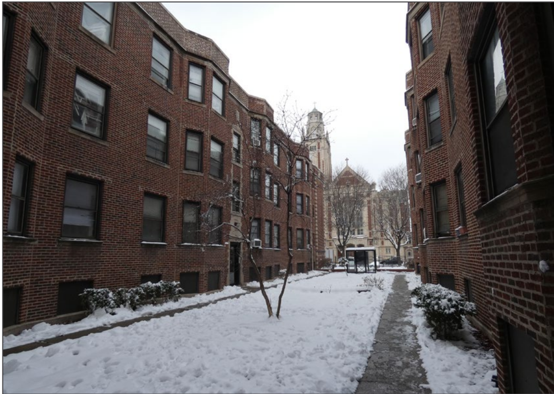
Photo 6. Courtyard, looking north.
