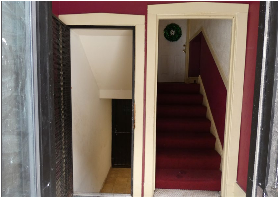
Photo 8. 5113 W. Washington Boulevard - 1st floor entrance vestibule, looking east.
