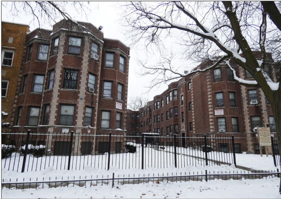
Photo 2. Washington Boulevard (north) facade, looking south.
