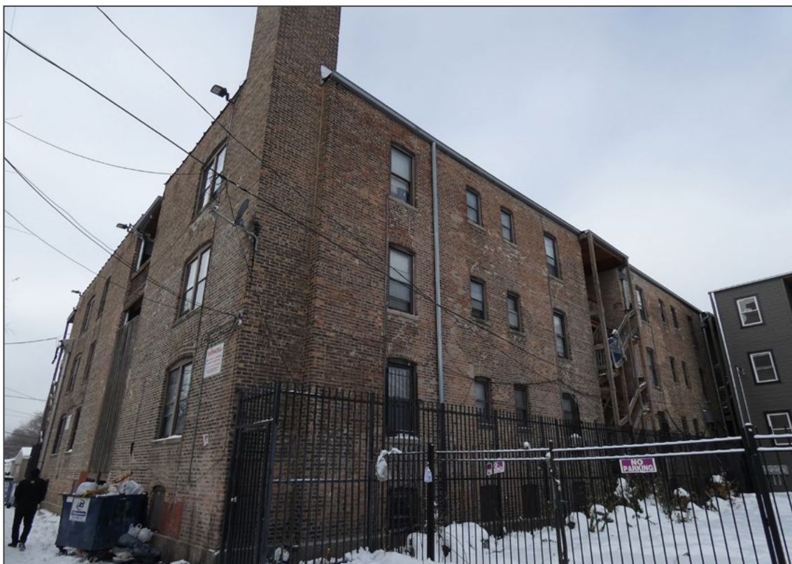
Photo 7. South (left) and east (right) facades, looking northwest.
