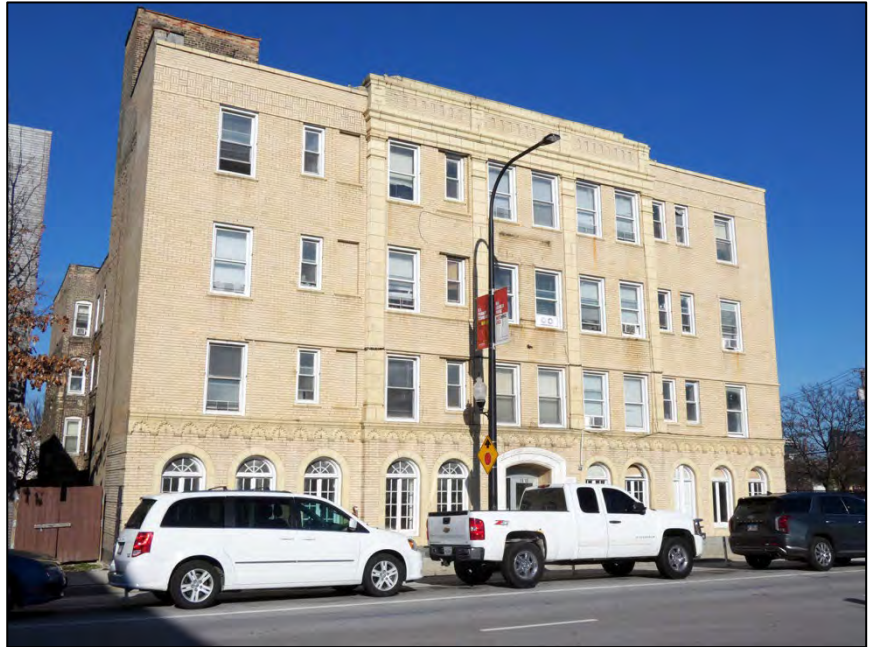
Figure 8. Royalton Hotel - 1810 W. Jackson Boulevard (completed 1926).
