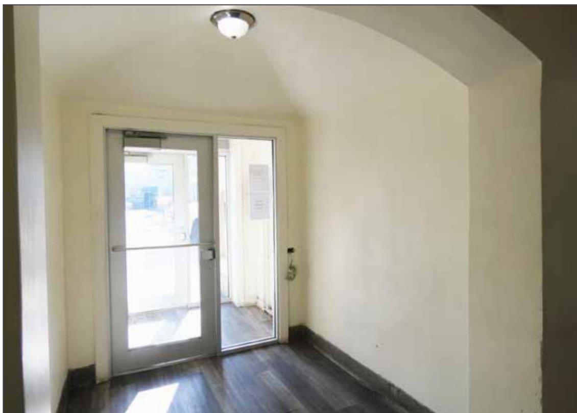
Photo 8 of 15. 1st floor, Jackson Boulevard entry vestibule, looking south.
