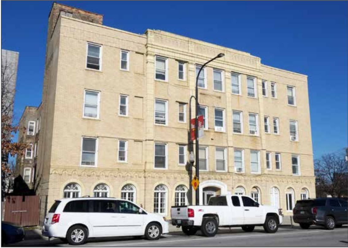
Photo 1 of 15. South (Jackson Boulevard) facade, looking northeast.
