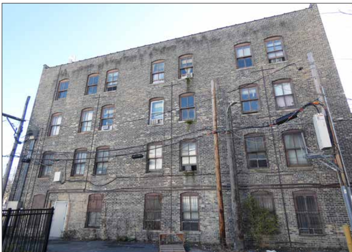
Photo 6 of 15. North facade, looking south.
