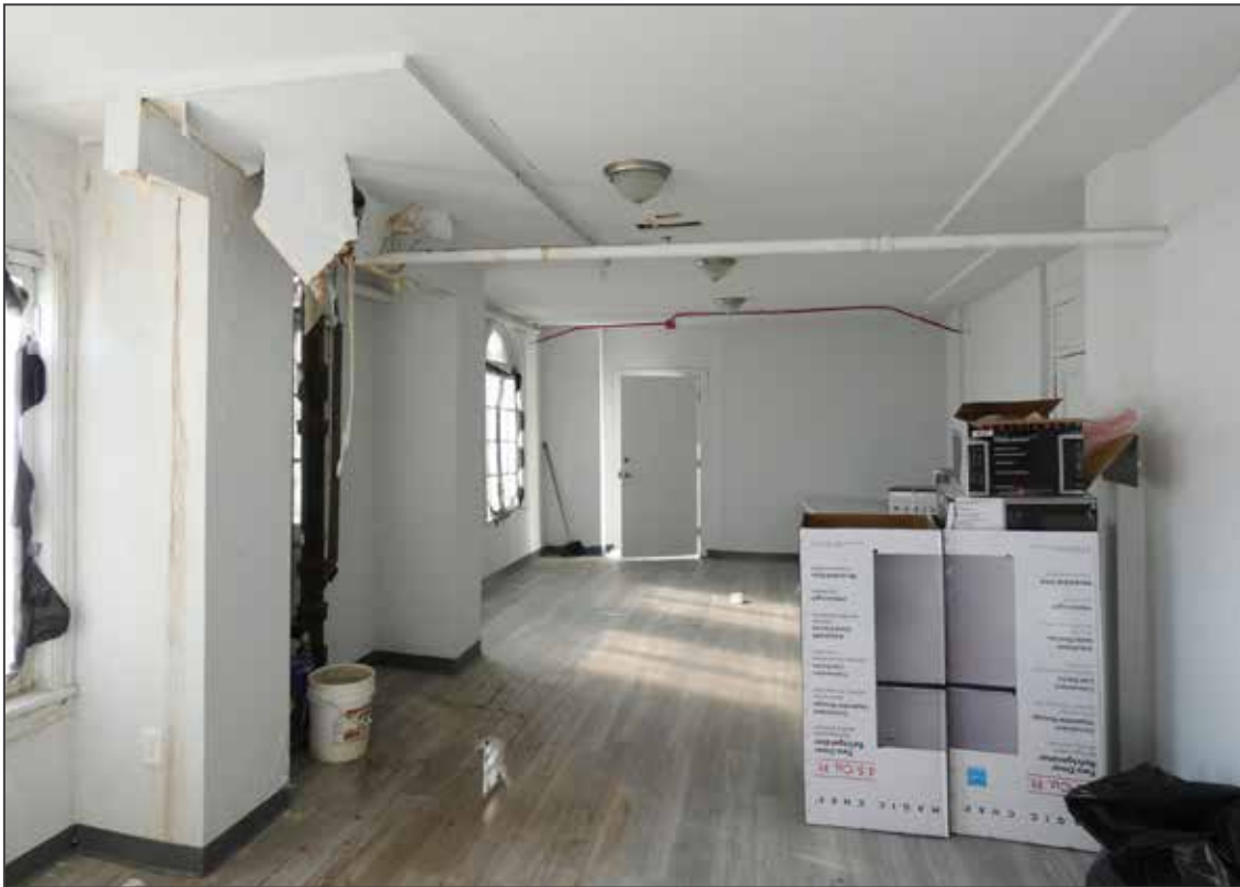
Photo 11 of 15. 1st floor, current office space, looking west.
