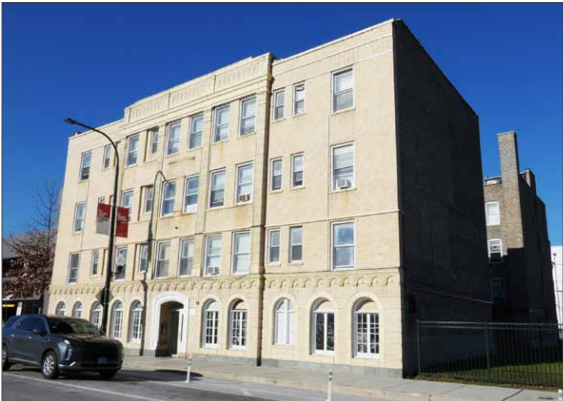
Photo 2 of 15. South (Jackson Boulevard) facade, looking northwest.
