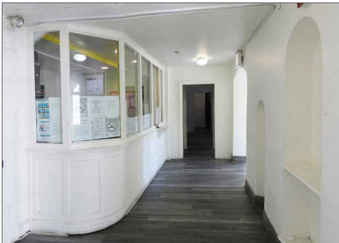
Photo 9 of 15. 1st floor, entry lobby, looking east.
