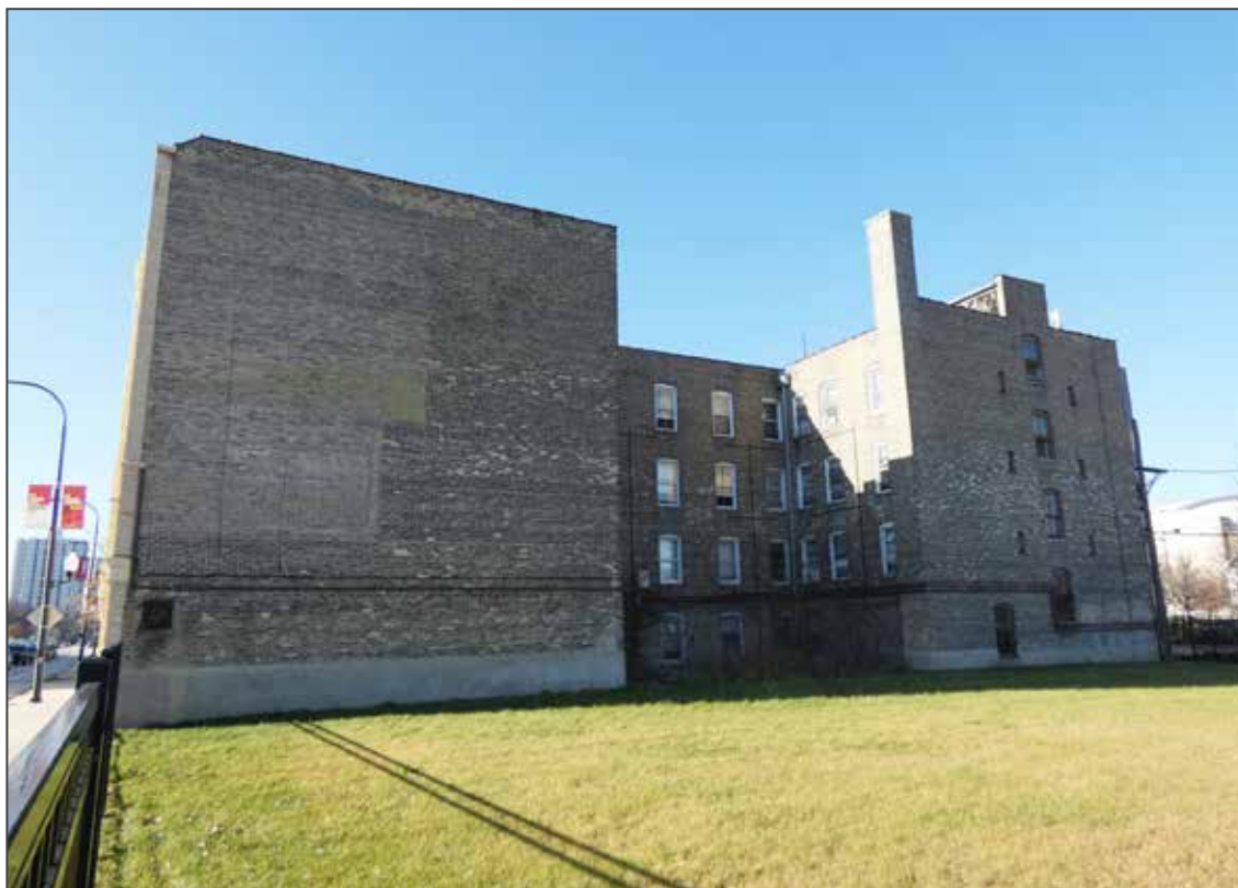
Photo 5 of 15. East facade, looking west.
