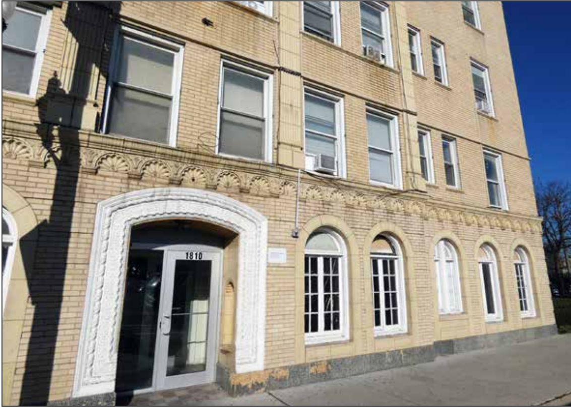
Photo 3 of 15. South (Jackson Boulevard) facade, looking northeast.
