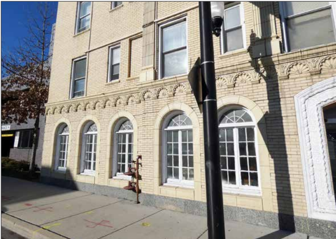
Photo 4 of 15. South (Jackson Boulevard) facade, looking northwest.
