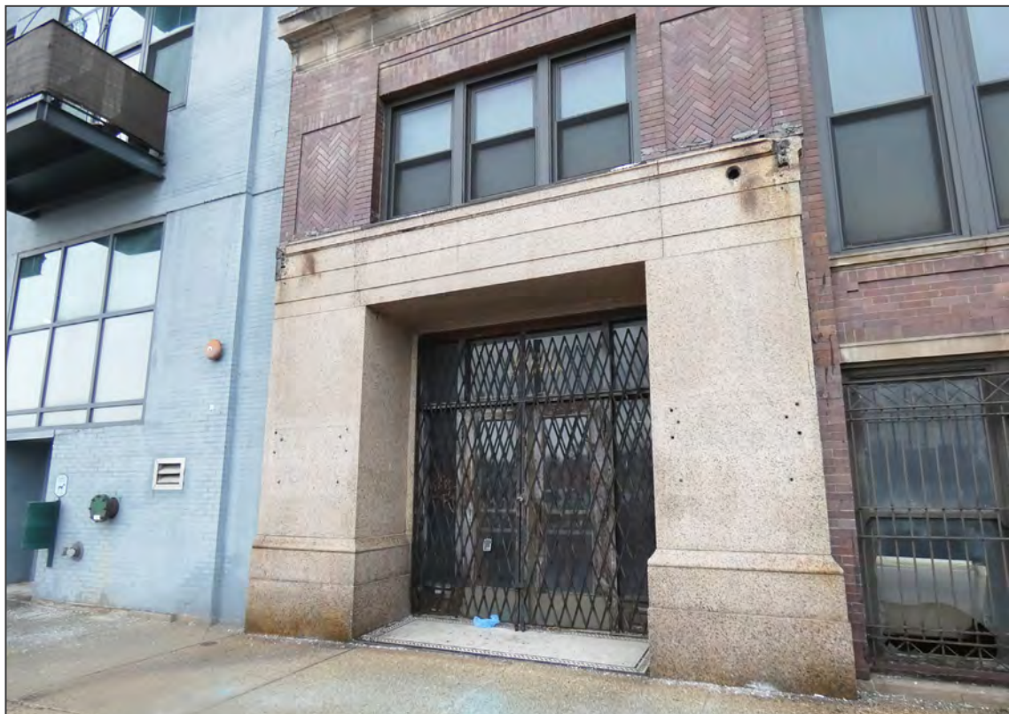
Photo 4. Van Buren Street (south) facade, looking north at main entrance.
