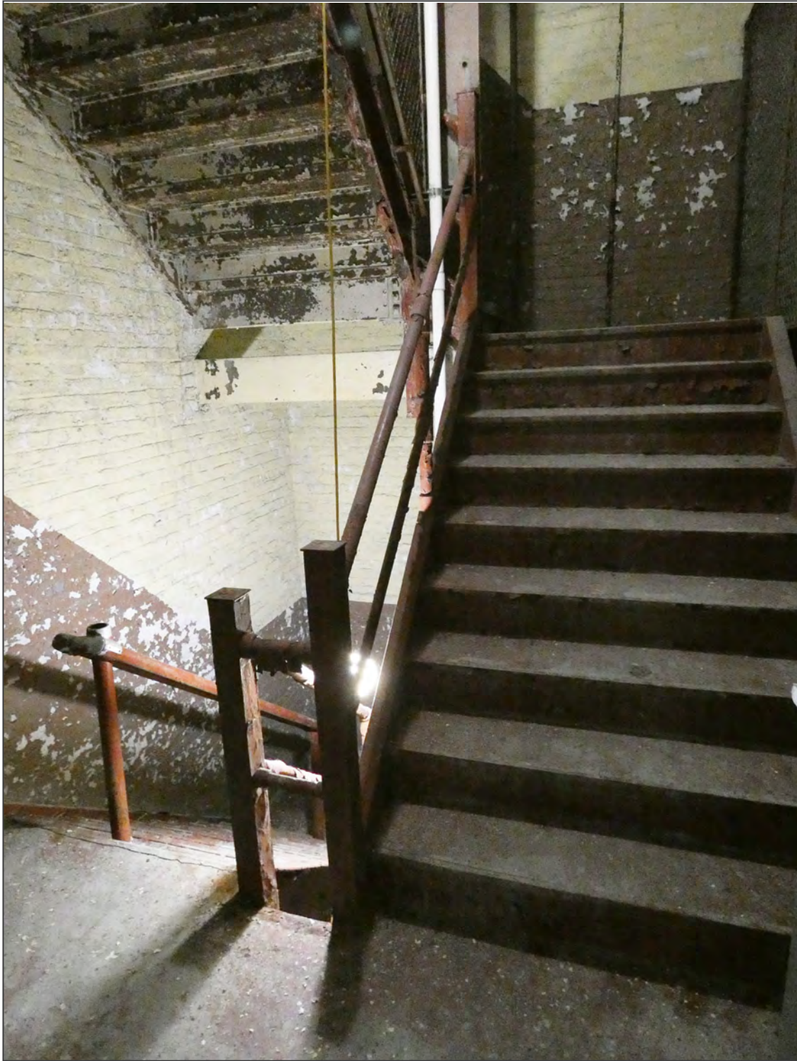
Photo 14. Center stairwell, typical view looking south.
