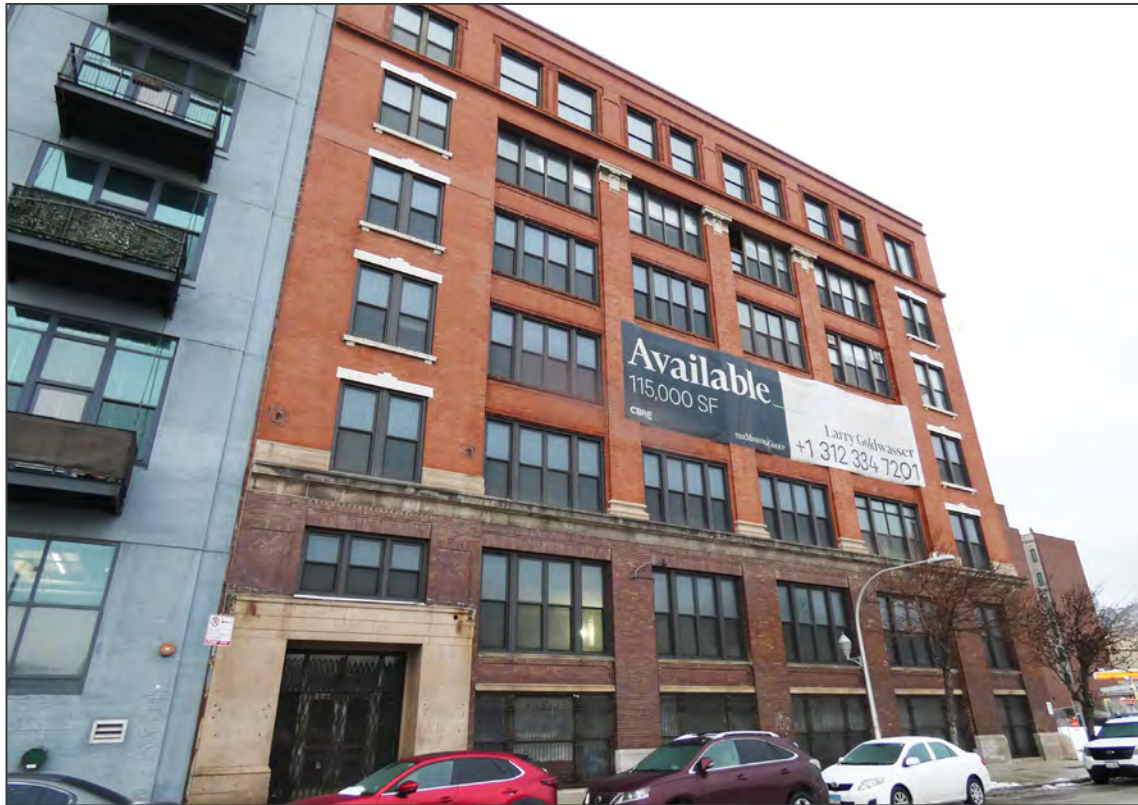
Photo 3. James C. Curtis & Co. Building, looking northwest.
