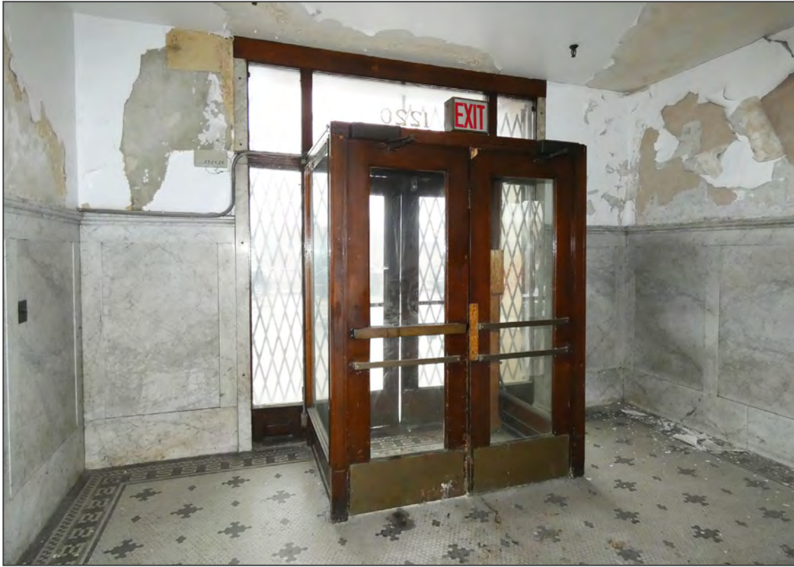
Photo 7. Ground floor entrance lobby, looking south at Van Buren Street entrance.
