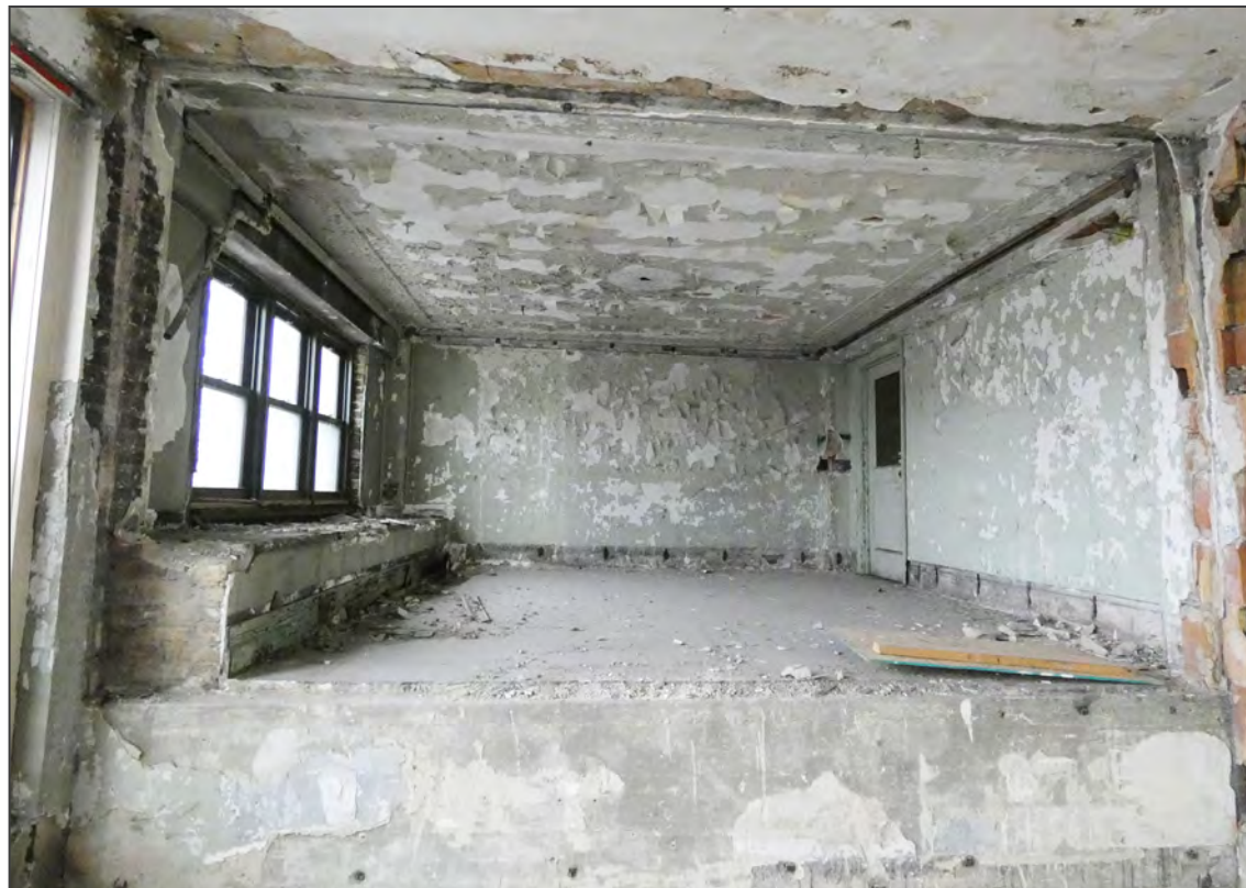
Photo 10. 2nd floor raised office, looking west.
