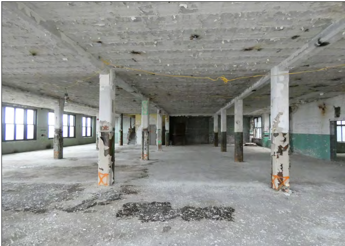
Photo 12. Typical upper floor south section, looking west.
