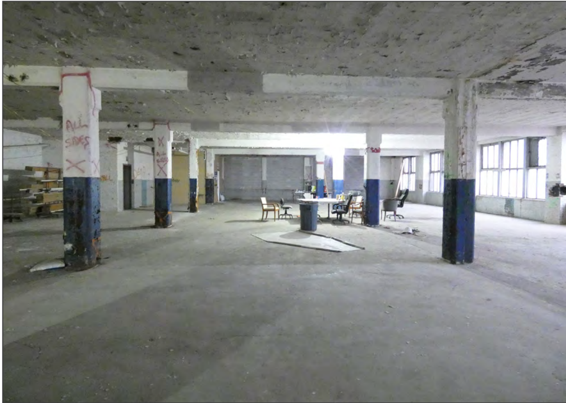
Photo 11. 2nd floor north section, looking north.
