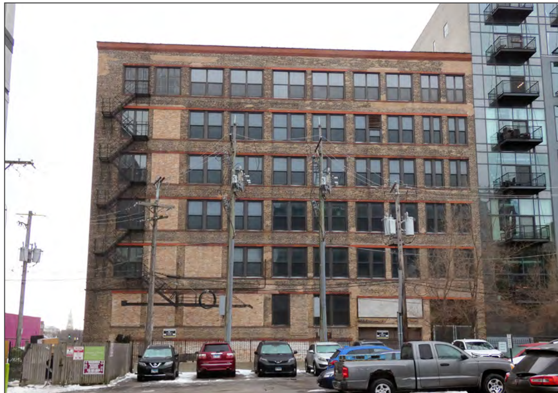
Photo 6. North alley facade, looking south.
