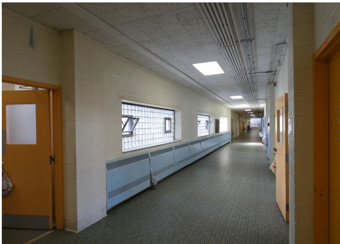
33. 1956 classroom addition, typical upper floor corridor
