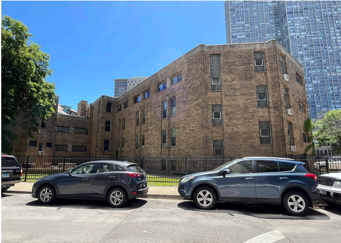
8. 1955 convent addition, looking southeast to dormitory wing
