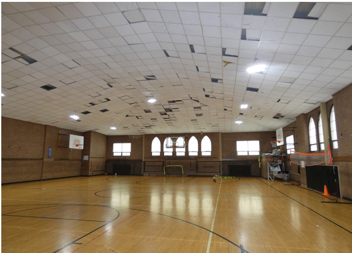
22. 1922 high school, gymnasium, looking east
