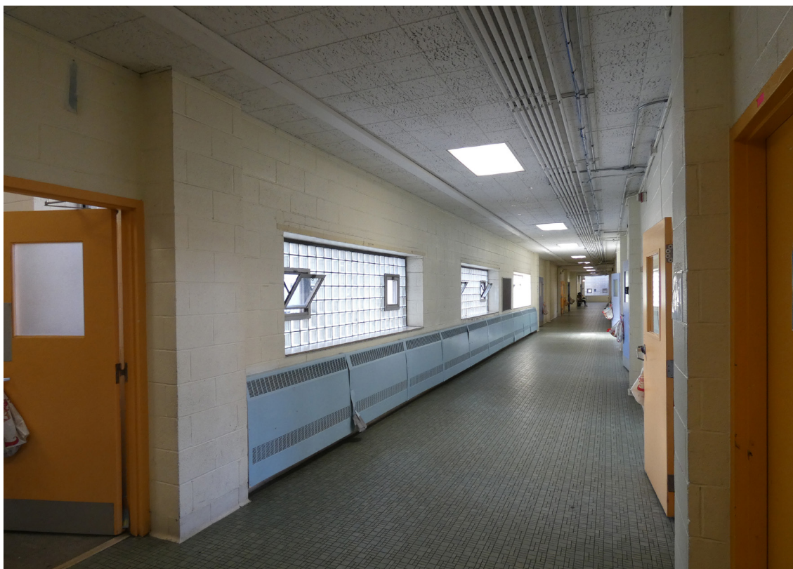
31. 1956 classroom addition, first floor corridor
