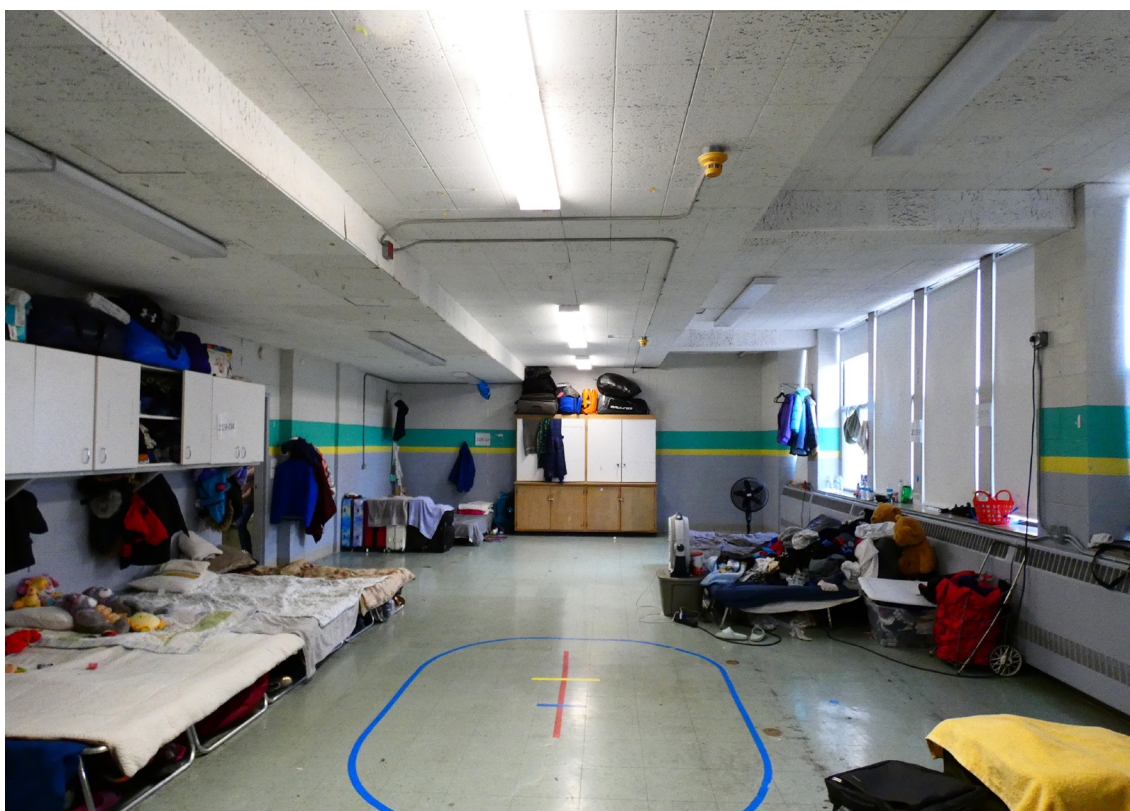
34. 1956 classroom addition, typical classroom
