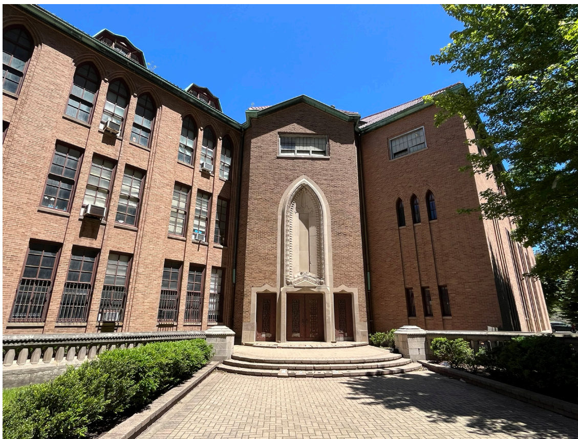
3. 1922 high school, looking northeast to main entrance
