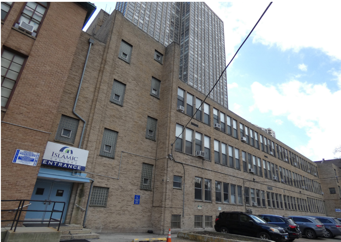
16. North elevation of 1956 classroom addition, looking southwest
