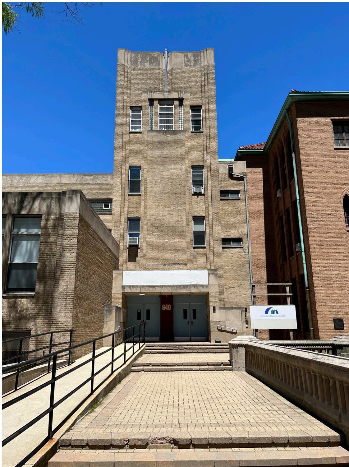
10. 1956 classroom addition, south entrance tower, looking north
