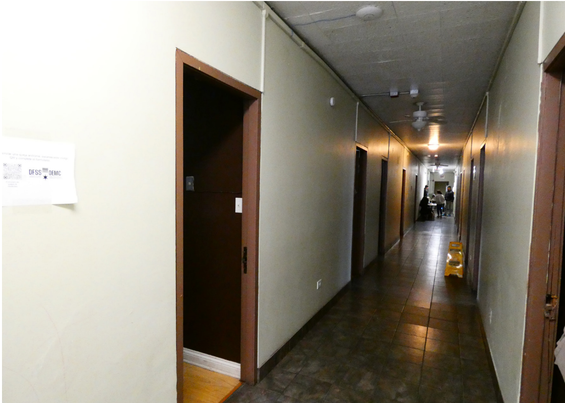
25. 1955 convent addition, typical corridor
