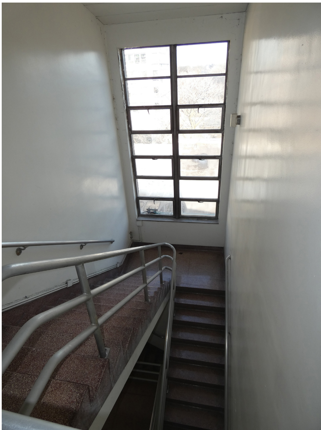
24. 1955 convent addition, stair connector, looking north
