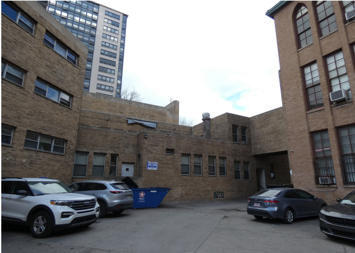
15. South elevation of 1955 convent addition, looking northeast
