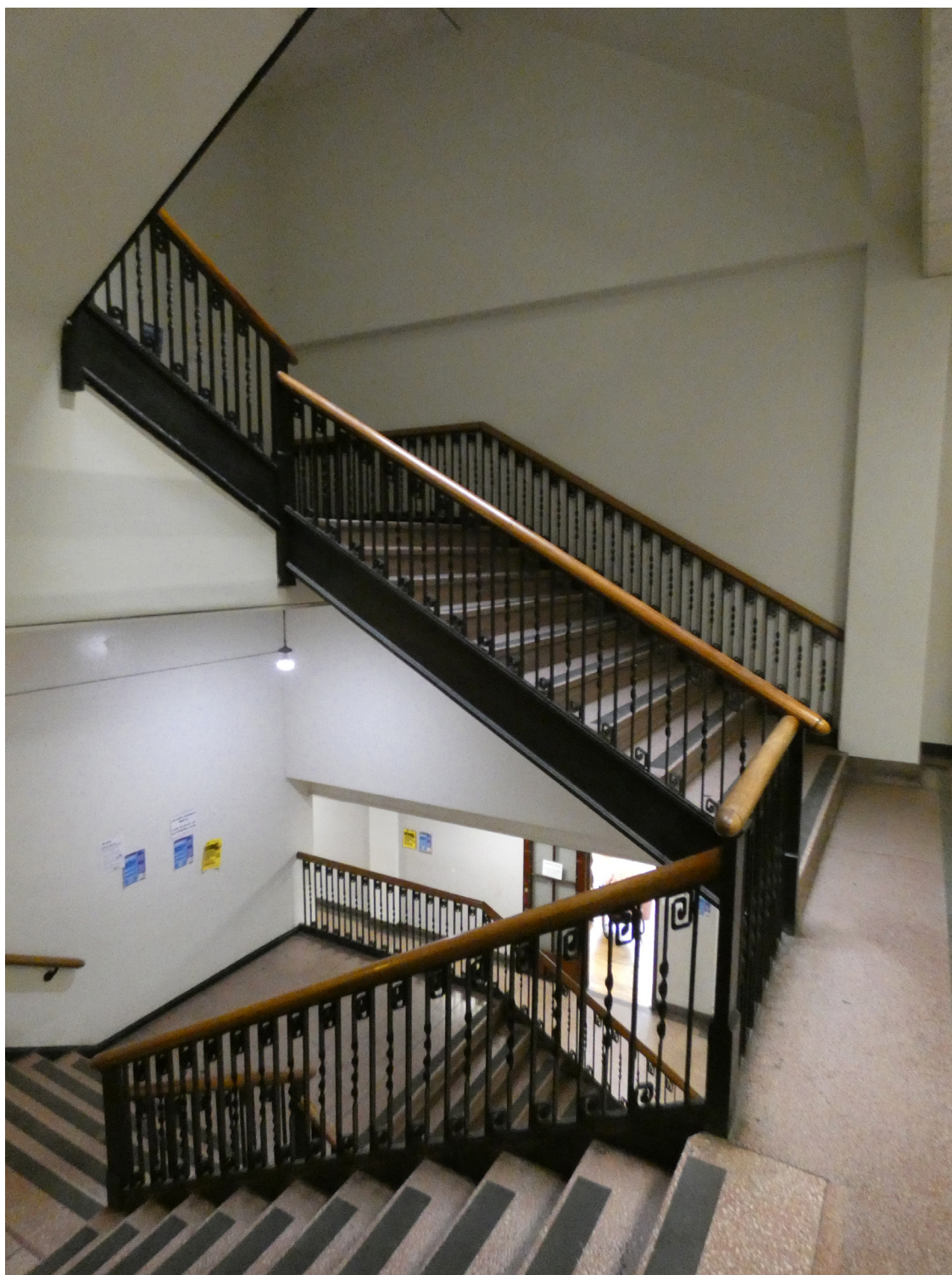
21. 1922 high school, main stair, looking east from second floor
