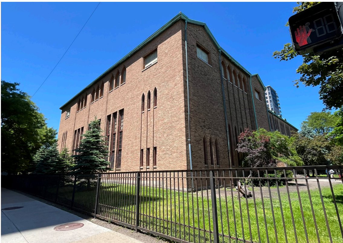
2. 1922 high school, south and east elevations of corner block, looking northwest
