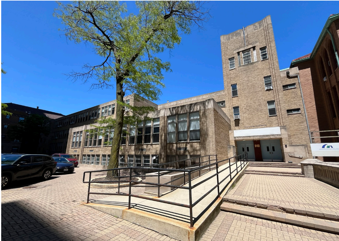
11. 1956 classroom addition, south elevation, looking northwest
