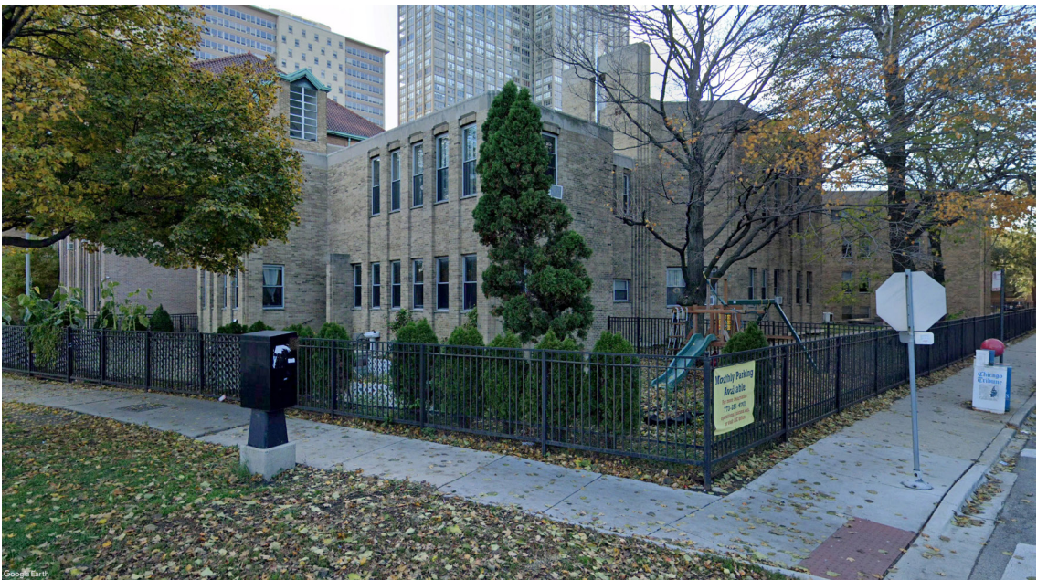
7. 1955 convent addition, east and north elevations, looking southwest
