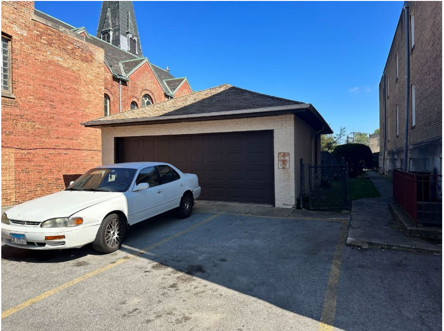
Photo 14 of 23: View of the hyphen connecting the church and rectory of Our Lady of the Holy Rosary Church looking north.
