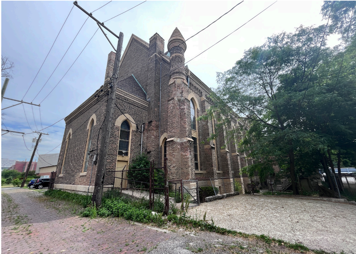
Photo 6: West and south elevations of church, looking northeast
