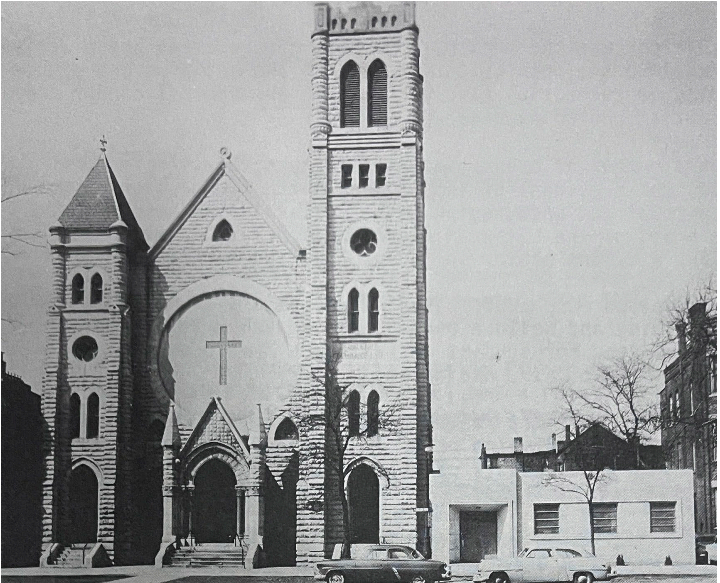
Figure 12: Exterior photograph showing 1952 addition and infill at rose window (First Immanuel archives)
