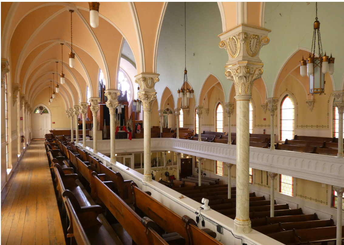
Photo 13: Church balcony, looking southeast
