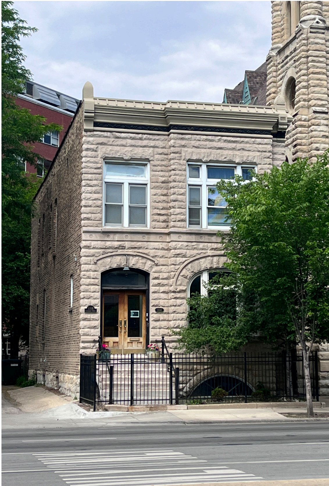
Photo 3: East and south elevations of parsonage, looking northwest
