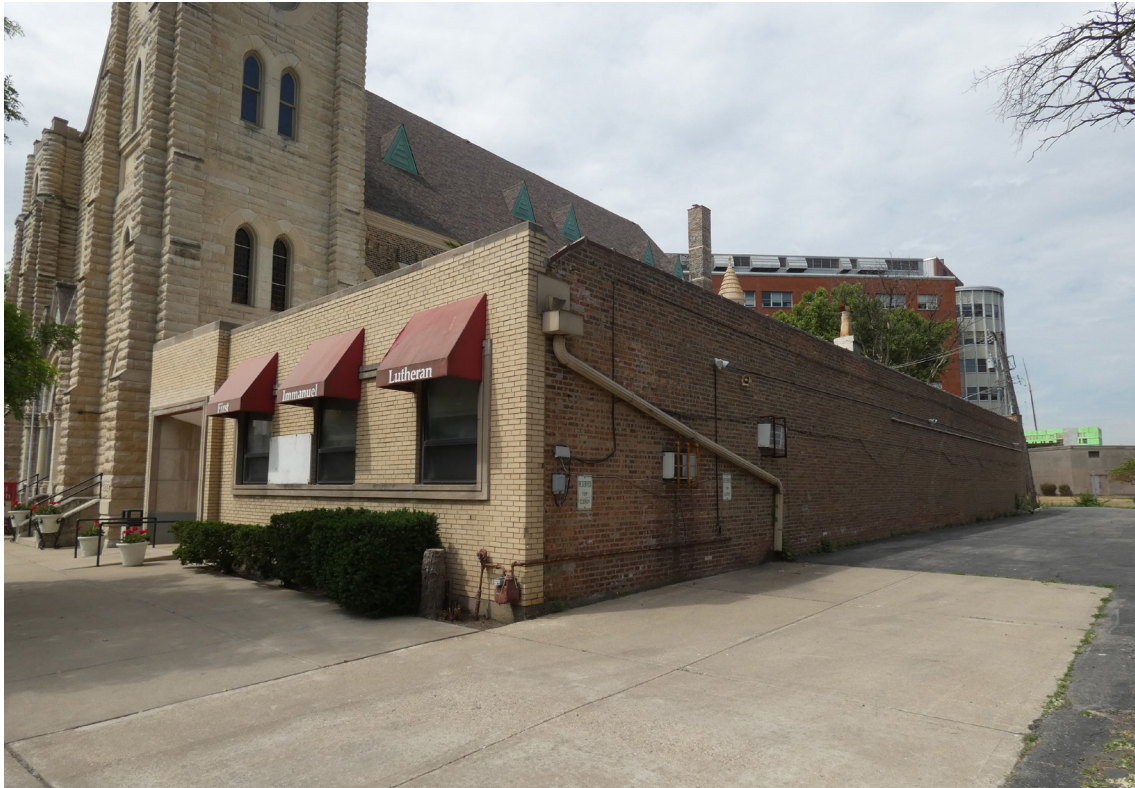
Photo 4: East and north elevation of 1952 addition, with north elevation of church in background, looking southwest
