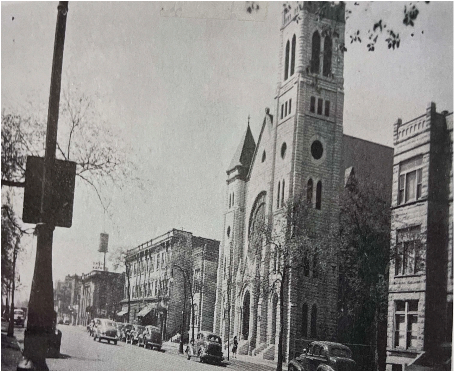
Figure 9: Streetview c. 1920 showing First Immanuel after removal of main steeple (First Immanuel archives)
