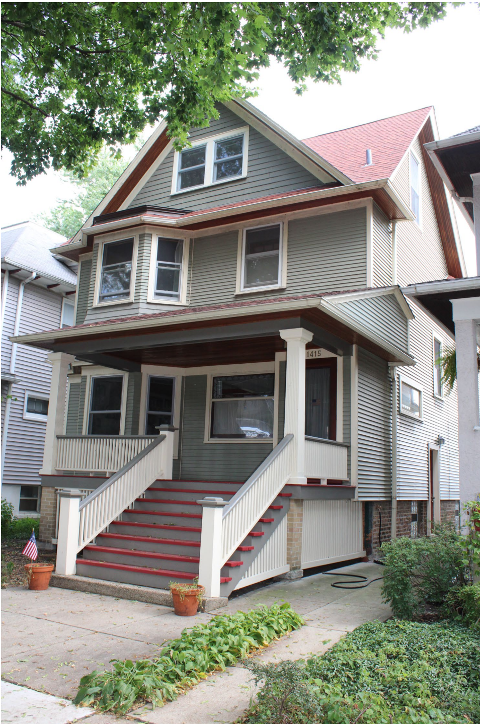
IMAGE 2: 1415 W. Glenlake: An example of a Queen Anne style house with full-width porch and cross-gable roof.
