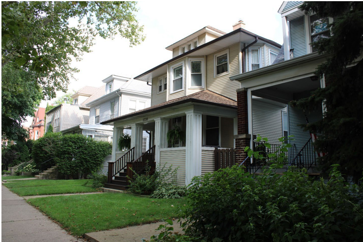
Photo #17: 1200 block W. Norwood Street, north side, view west.
