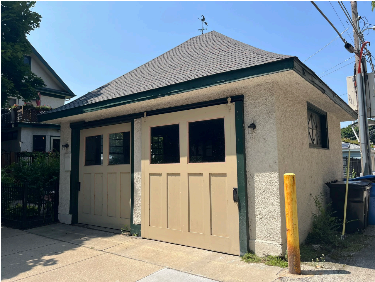
IMAGE 15: 1400 Hood: Example of a contributing garage with stucco cladding, hip roof with overhanging eaves, and sliding wood doors.
