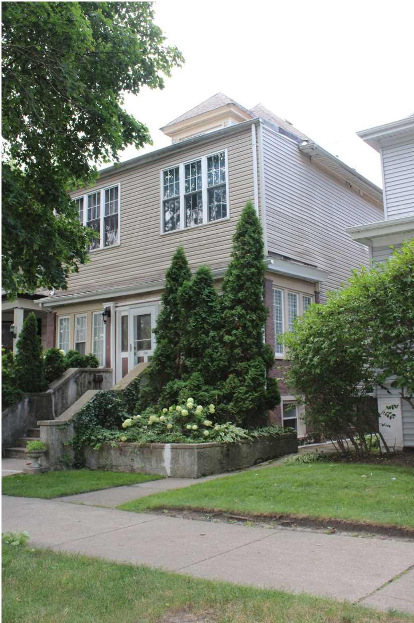
IMAGE 19: 1245 W. Norwood Avenue: Example of a non-contributing building that has lost its architectural integrity due to extensive alterations.
