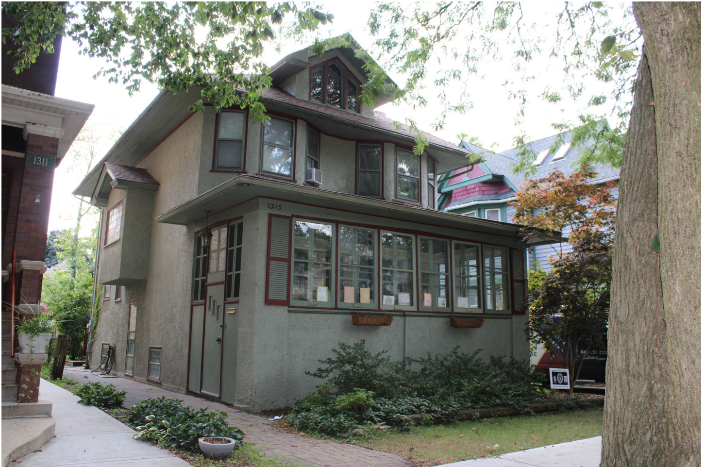
IMAGE 7: 1315 W. Hood Avenue: An example of a hip-roof, Prairie style house with full-width, enclosed porch and side entry.
