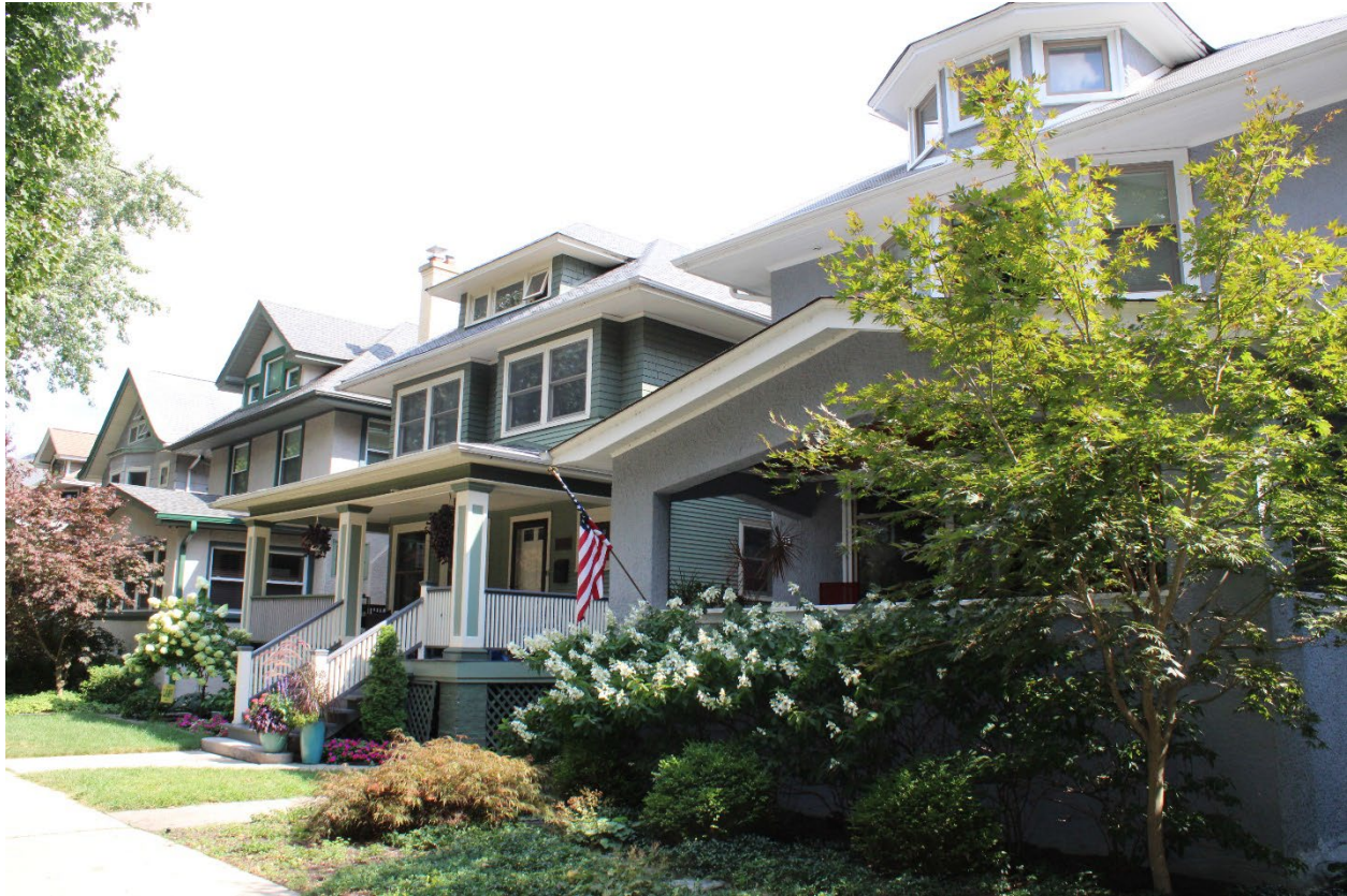
Photo #10: 1300 block W. Glenlake Avenue, south side, view east.
