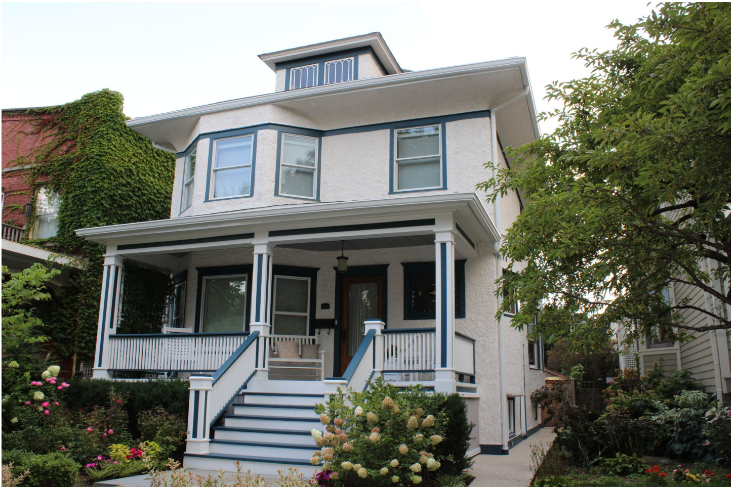
IMAGE 5: 1303 W. Norwood Street: An example of a hip-roof, Prairie style house with front entry and full-width porch.
