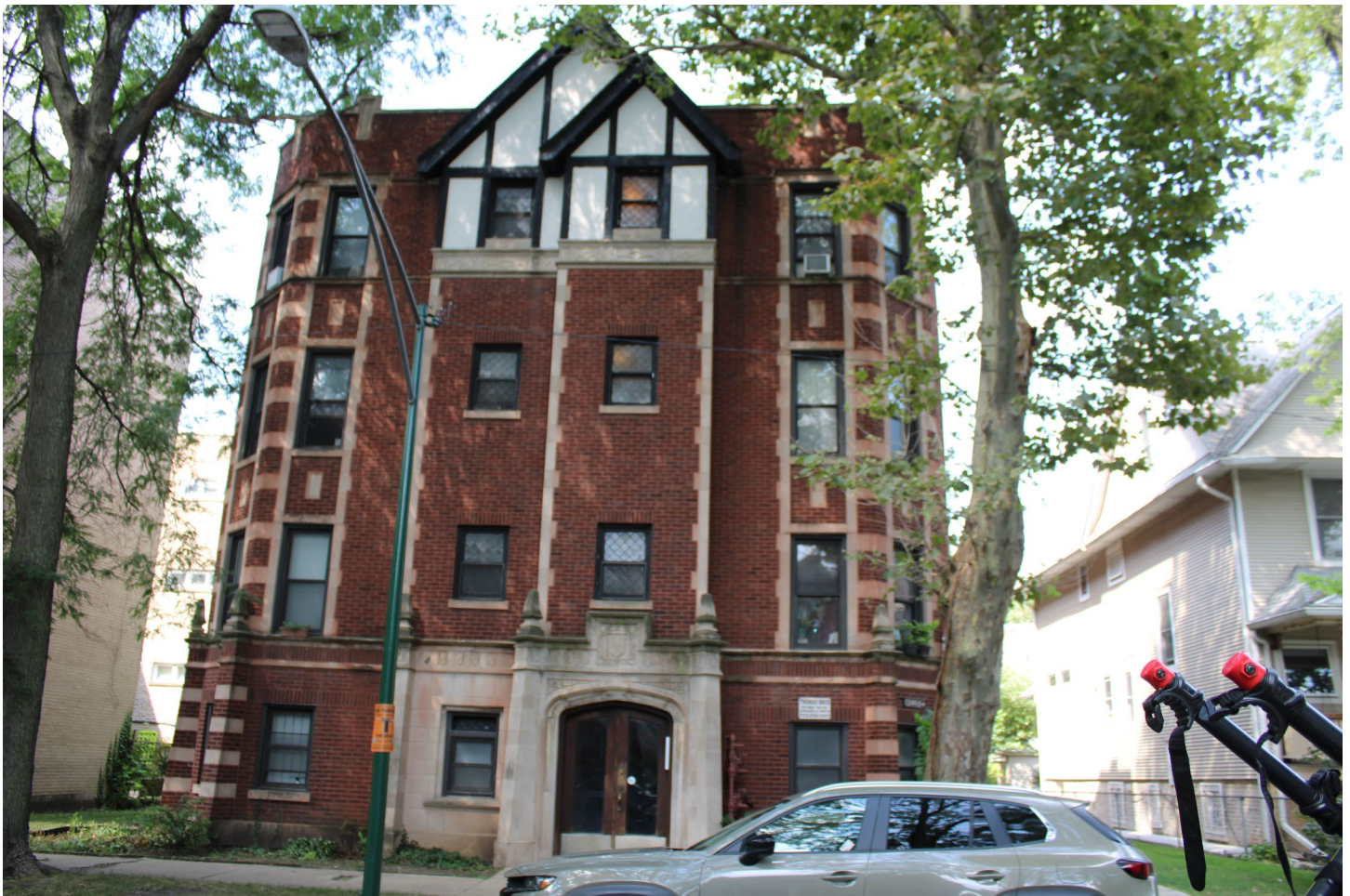
IMAGE 14: 1344-46 W. Hood Avenue: Rare example of a Tudor Revival style apartment building in the District.
