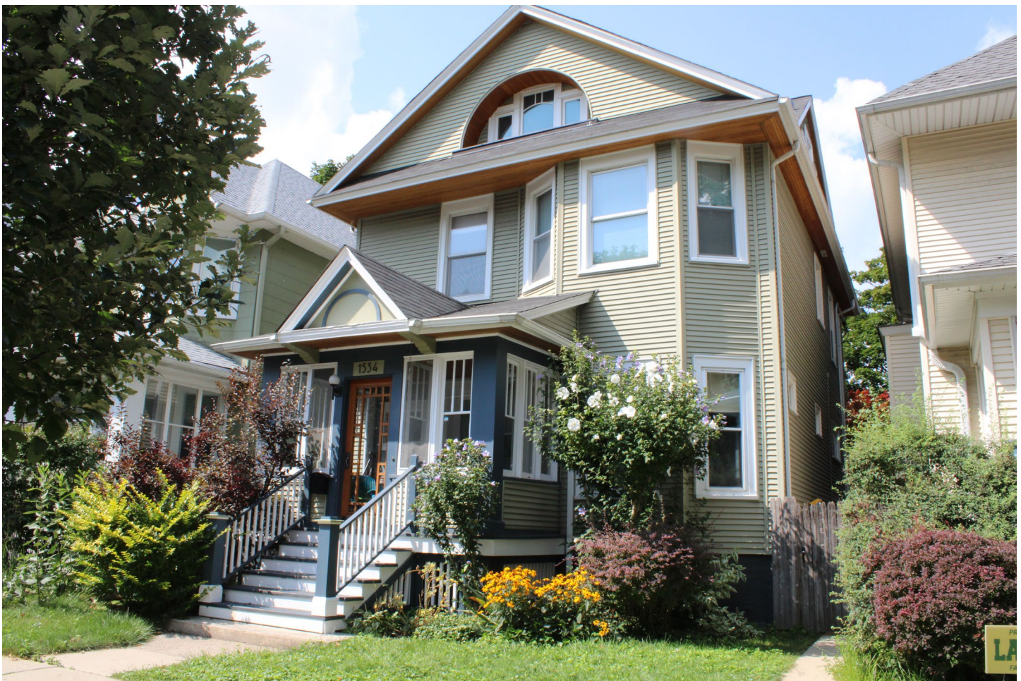
IMAGE 1: 1534 W. Glenlake: An example of a Queen Anne style house with a partial-width, enclosed porch and front-gable roof.
