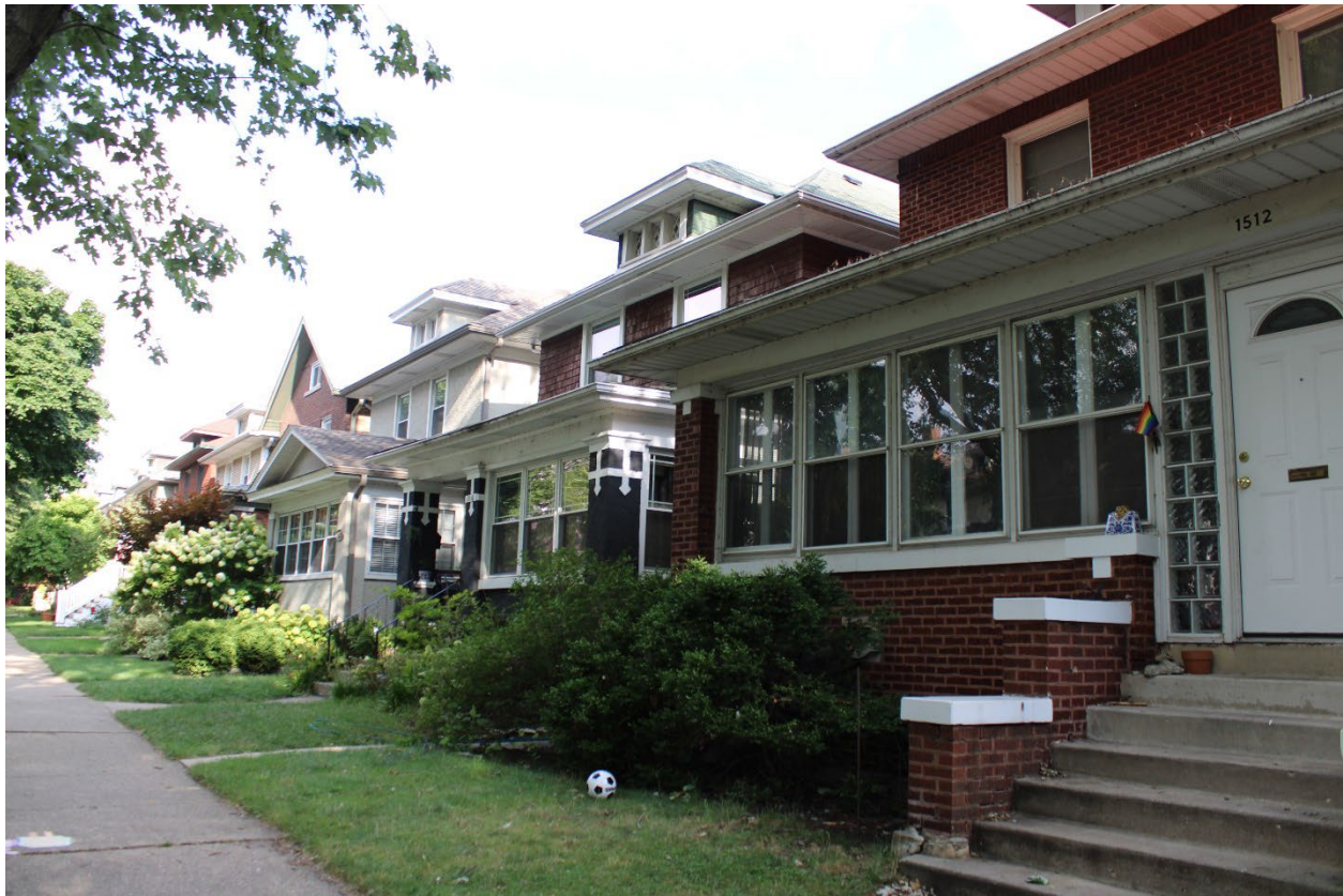
Photo #23: 1500 block W. Norwood Street, north side, view west.
