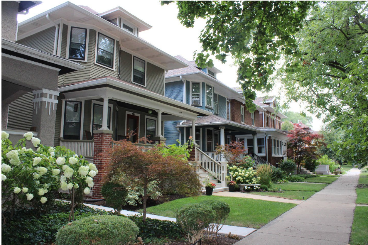
Photo #13: 1400 block W. Glenlake Avenue, south side, view west.
