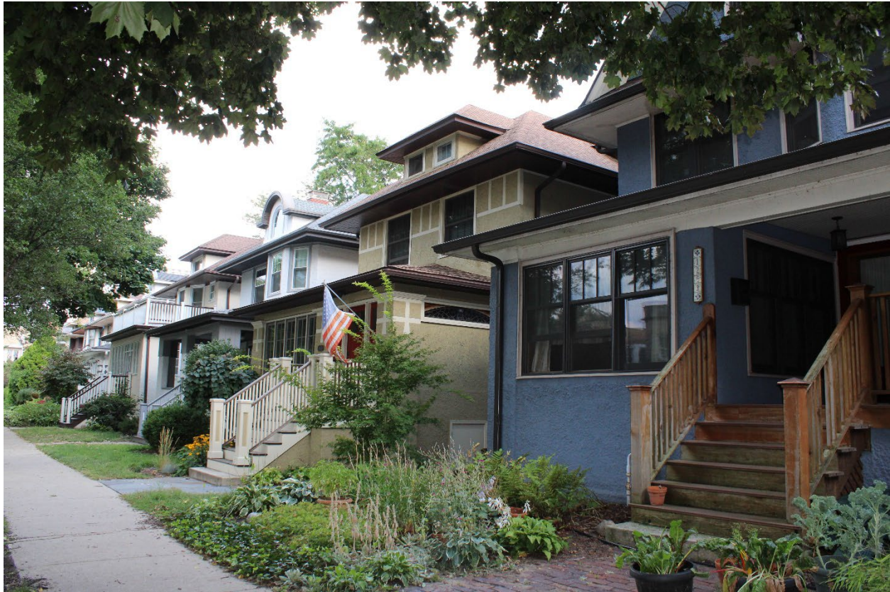
Photo #9: 1200 block W. Glenlake Avenue, south side, view east.
