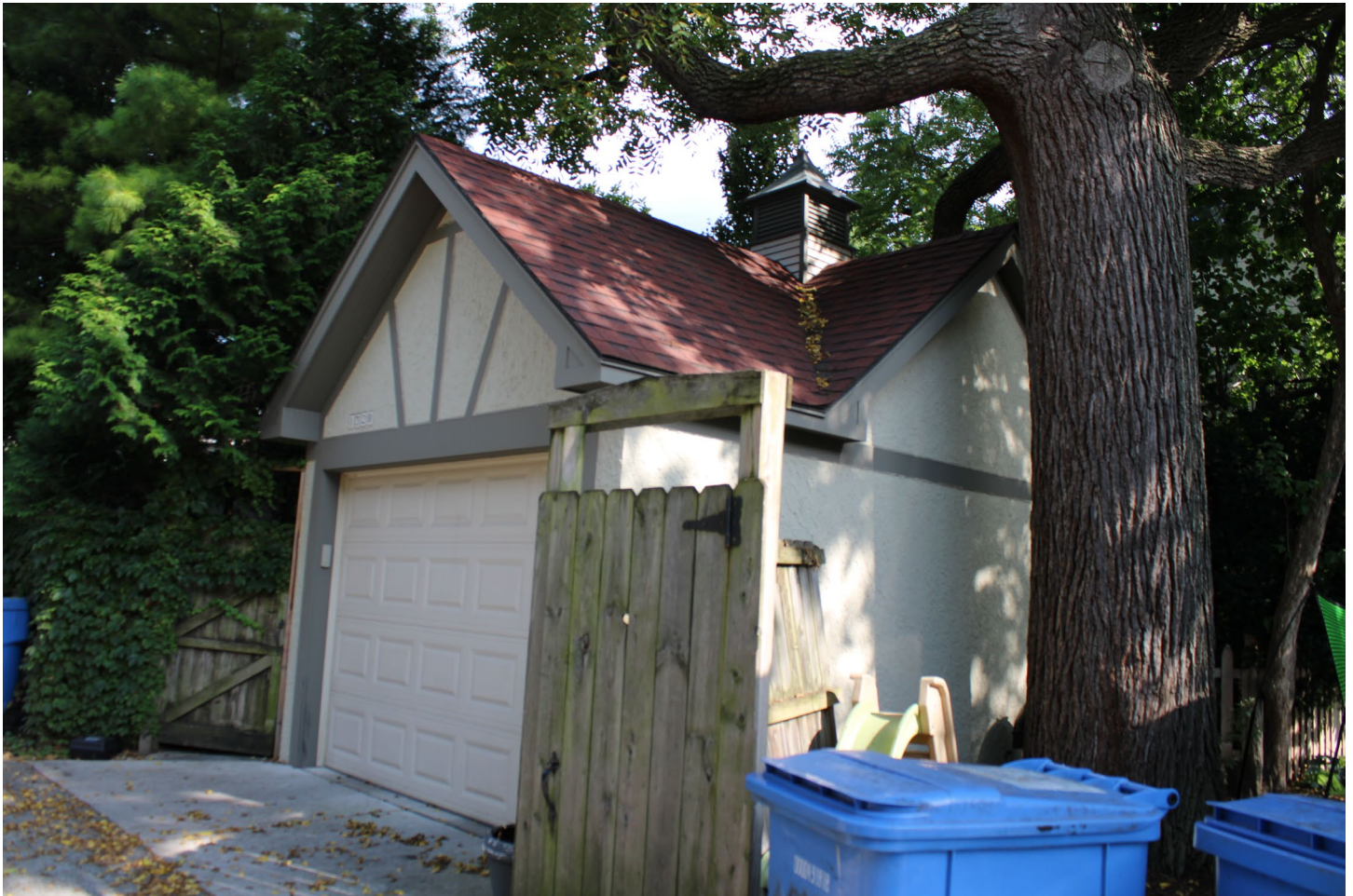
IMAGE 16: 1320 Glenlake: Example of a contributing garage with cross gable roof, stucco cladding with stickwork, and wood cupola.
