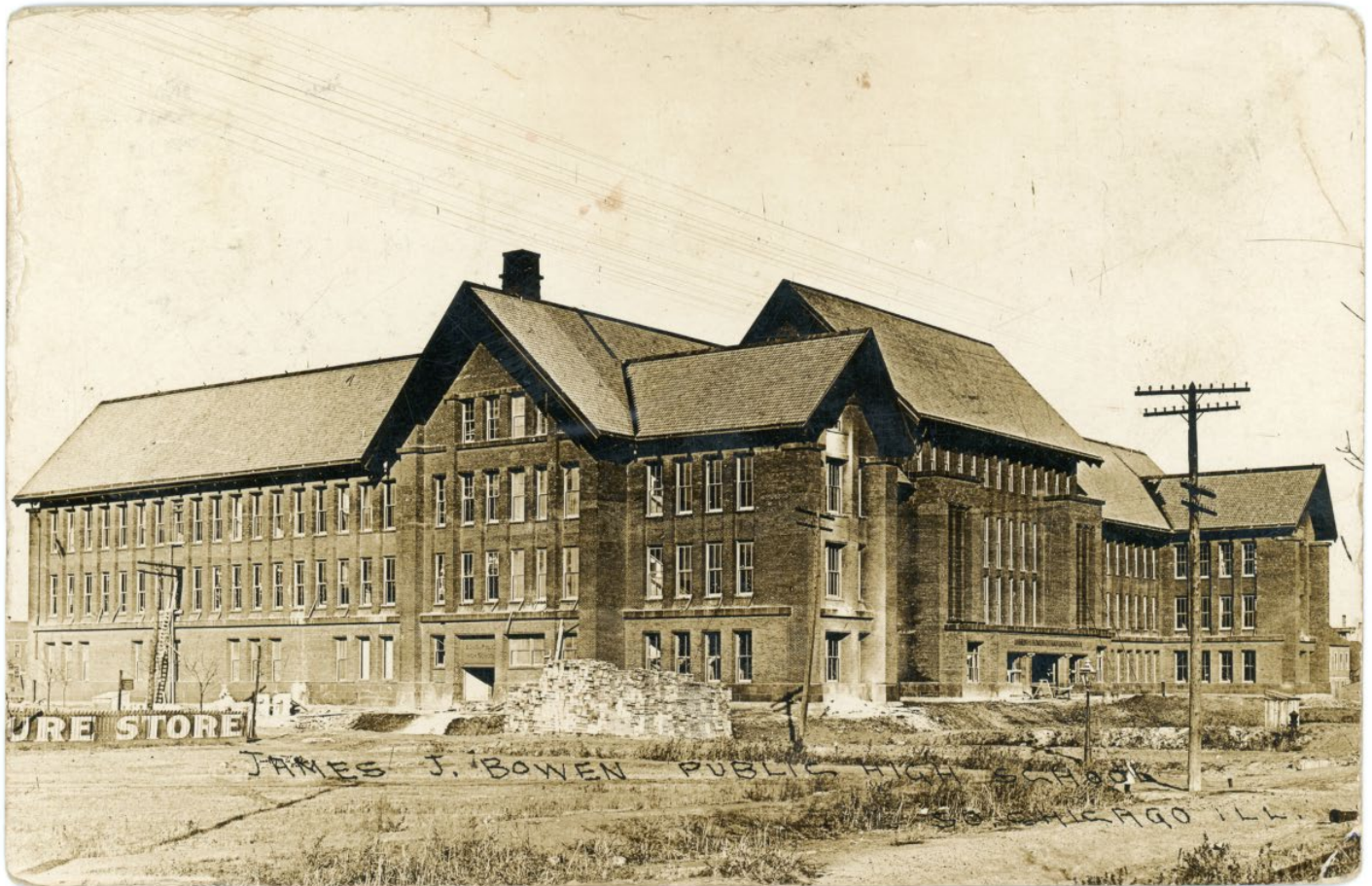
Figure 10: Bowen High School under Construction, 1910 (Southeast Chicago Archive and Storytelling Project)
