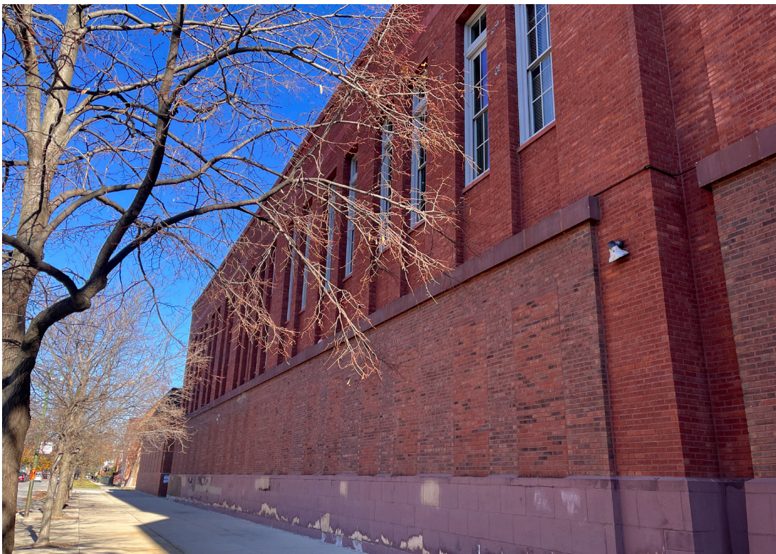
0008. West elevation of 1940 addition, looking northeast
