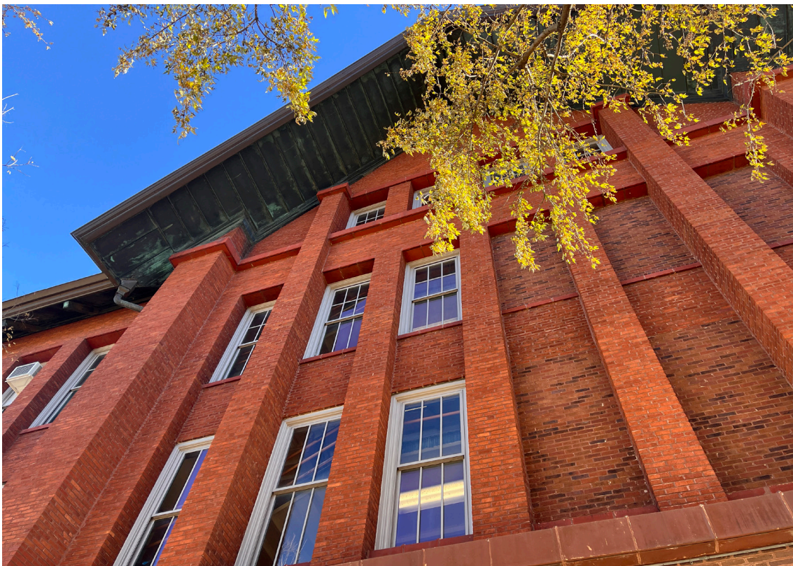
0006. West elevation, detail of upper floors and roofline at entrance
