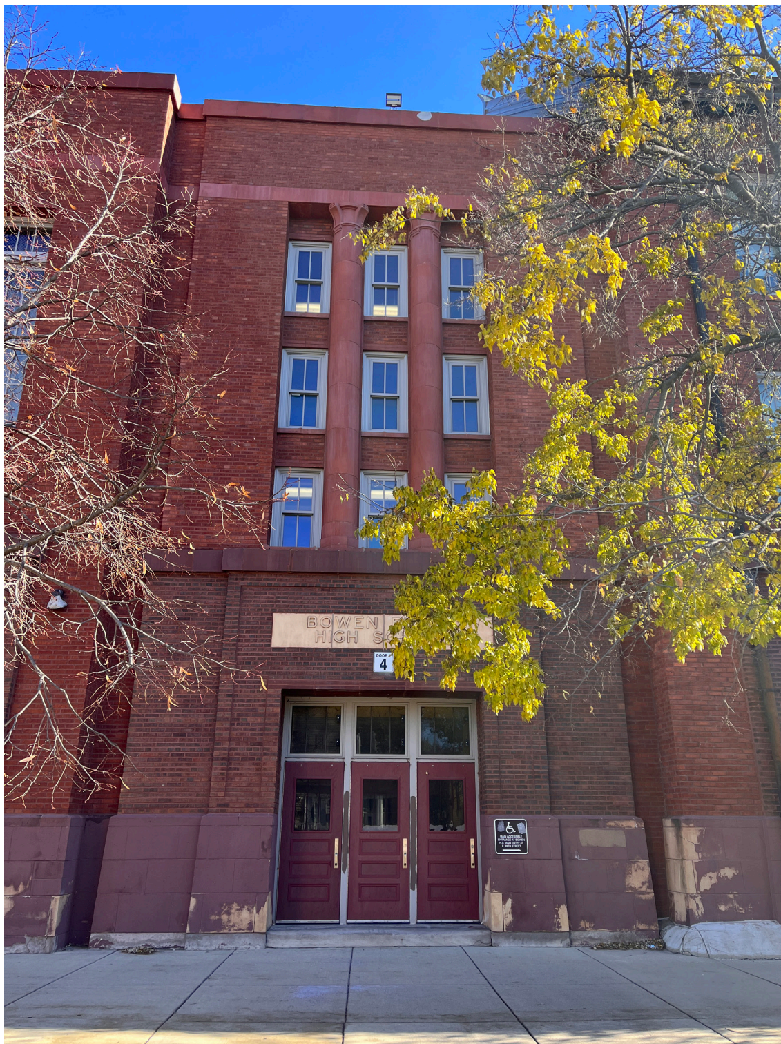
0009. West elevation of 1940 addition, looking east to entrance
