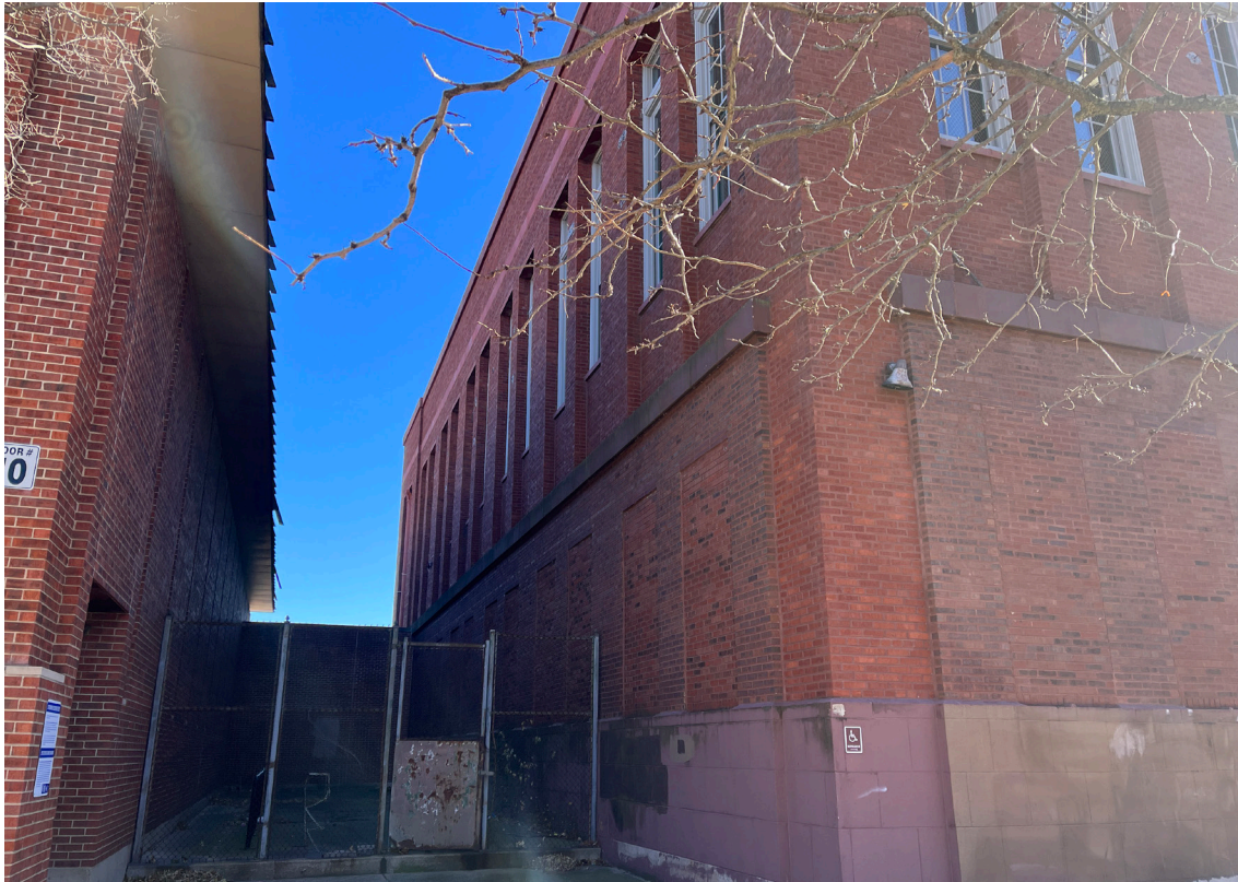
0010. Looking east between 1940 addition (right) and 1969 gymnasium addition (left)
