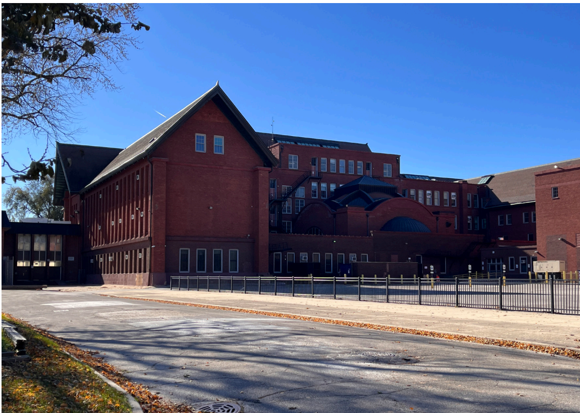
0013. North elevation of main building, looking southwest
