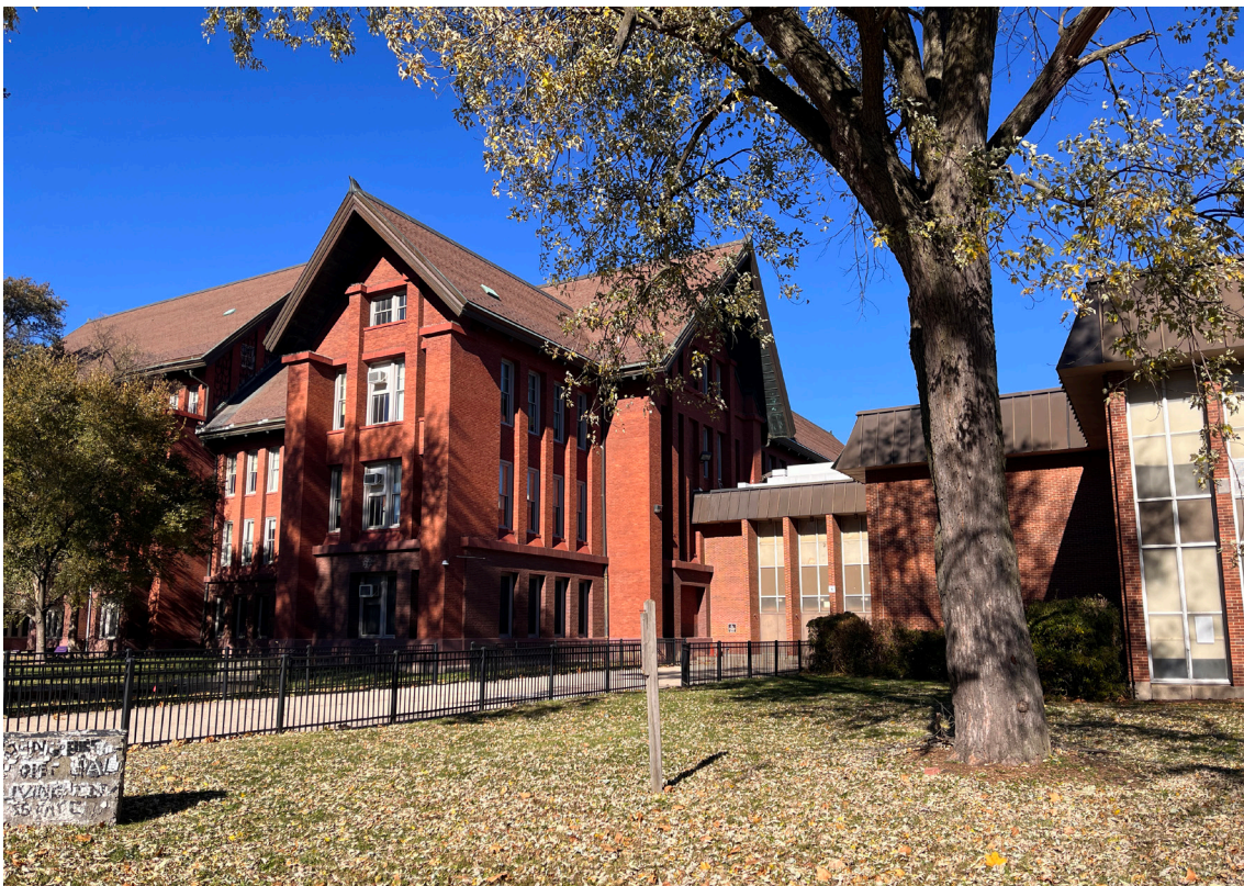
0004. South elevation, looking northwest to east end wing and connector to 1969 addition
