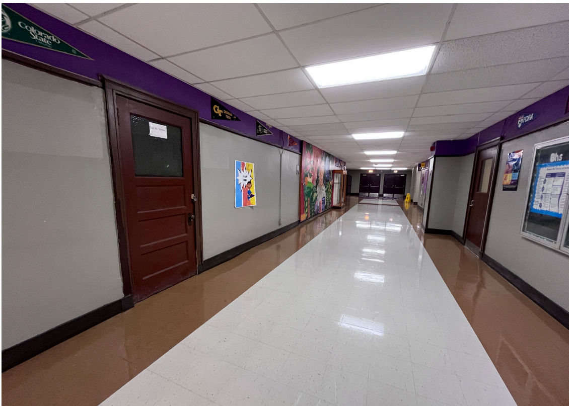
0017. First floor, typical corridor, looking east
