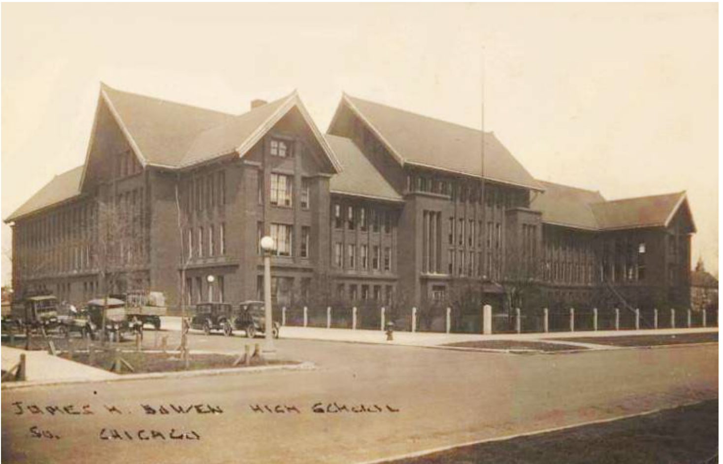
Figure 12: Bowen High School shortly after completion (1910)
