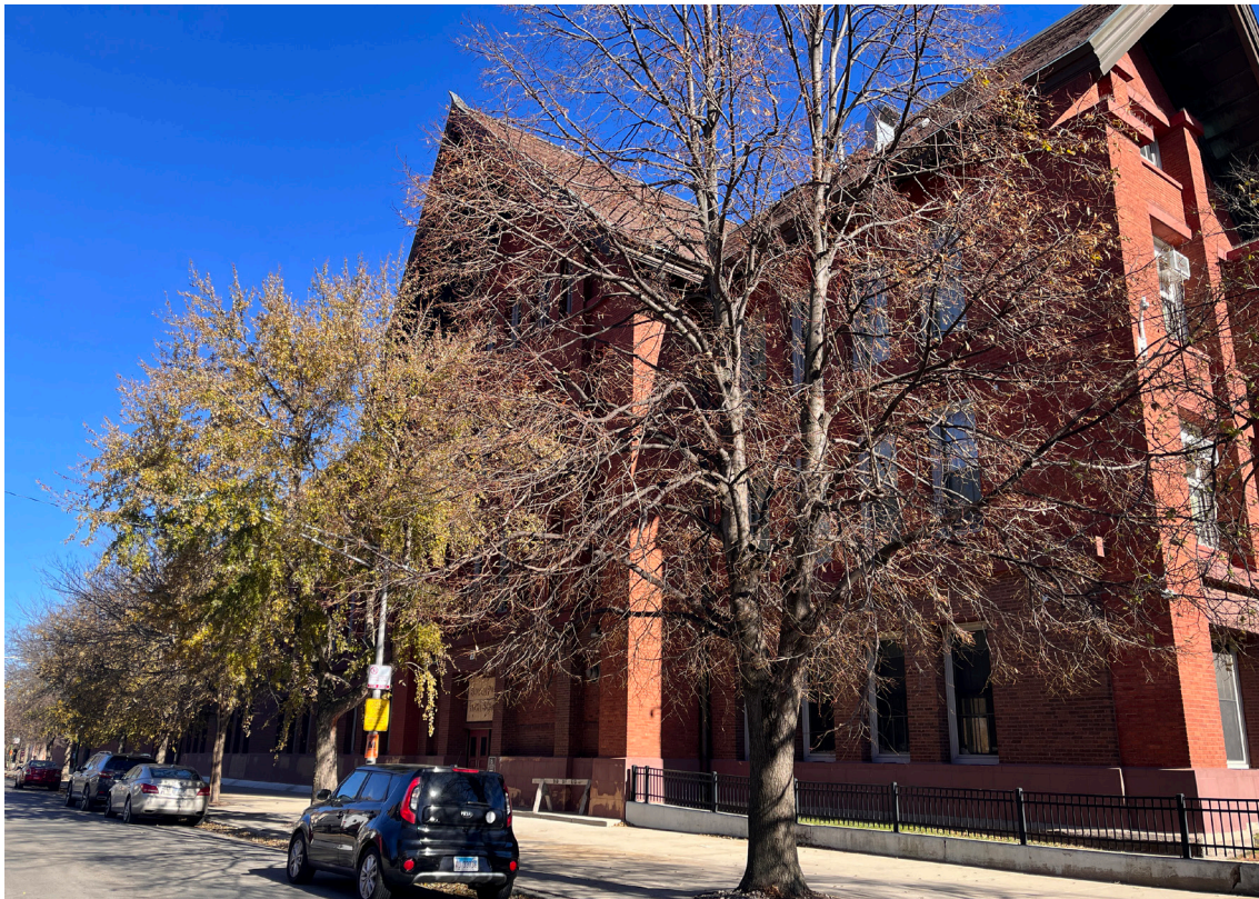
0005. West elevation, looking northeast
