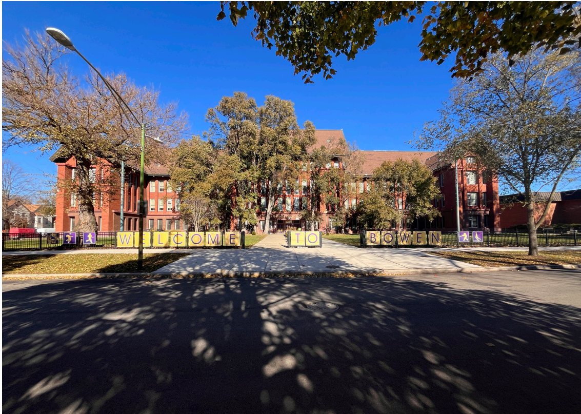
0001. South elevation, looking north
