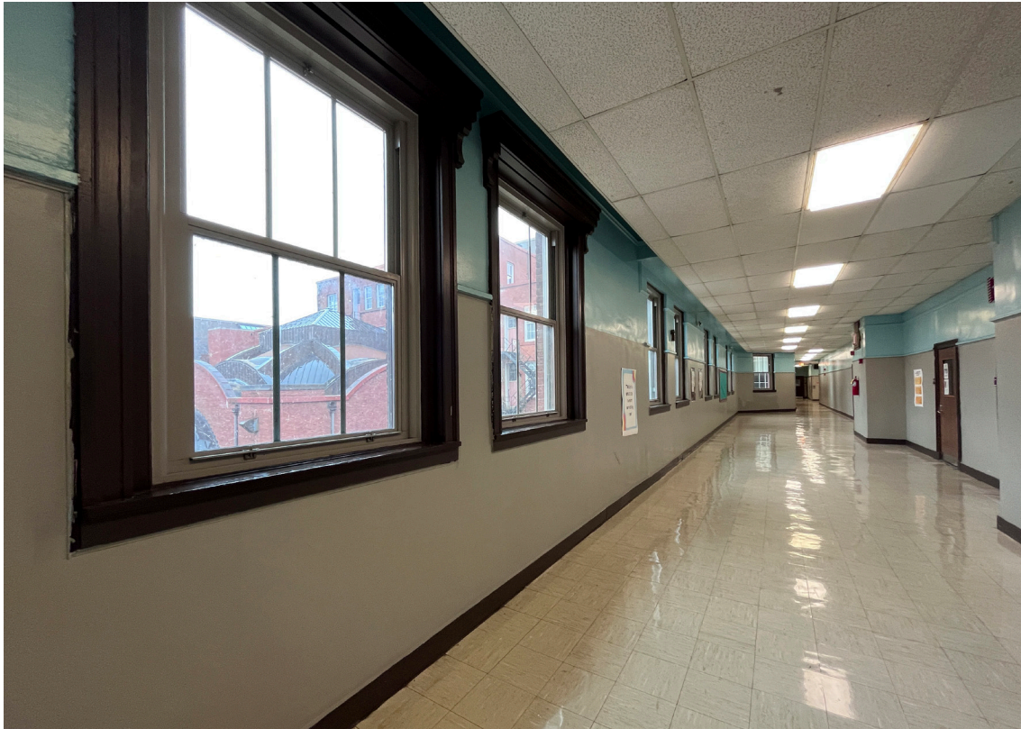
0029. Third floor corridor, looking south
