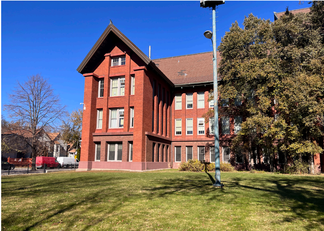
0003. South elevation, looking north to west end wing
