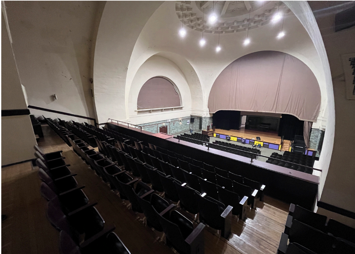
0020. First floor, auditorium, looking north from balcony
