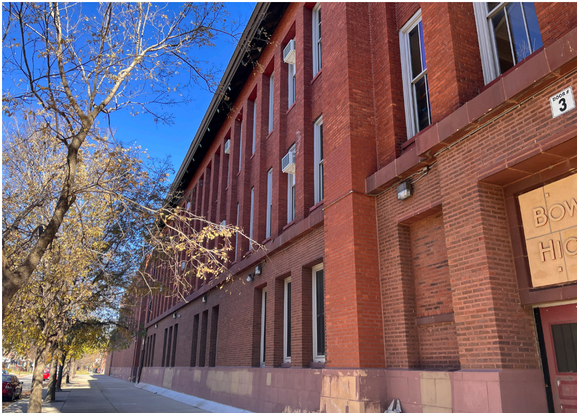
0007. West elevation, looking north
