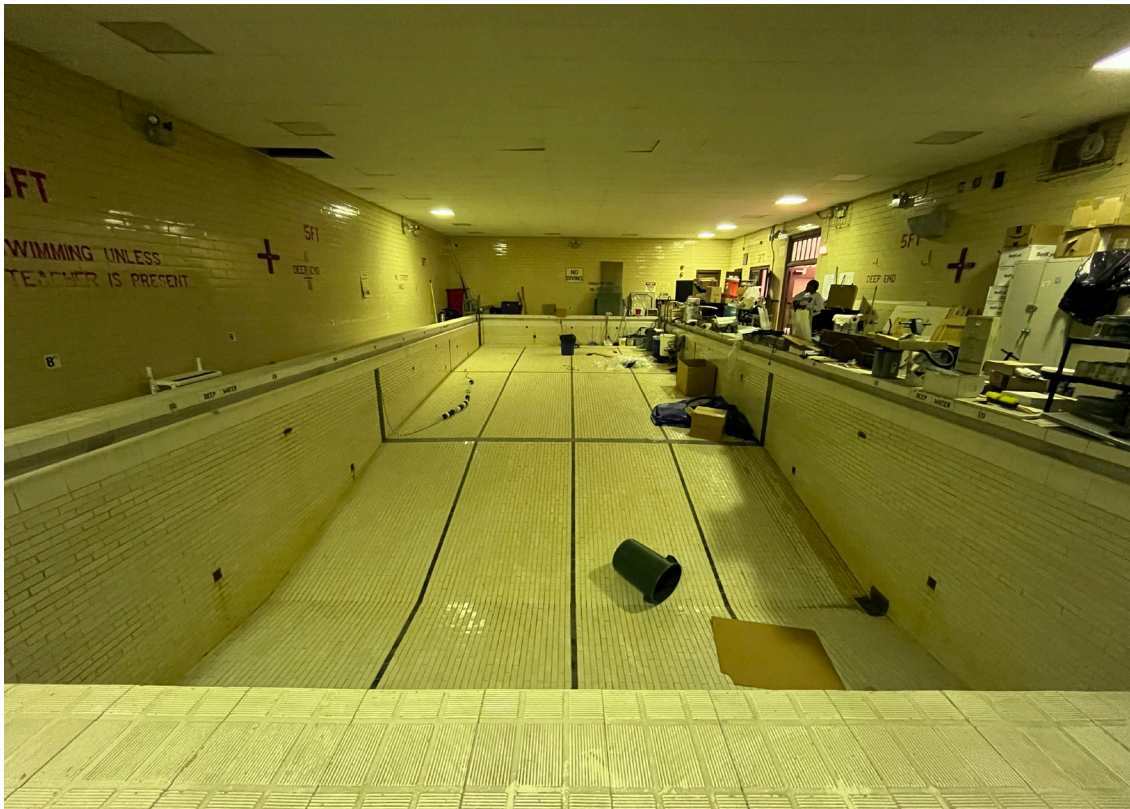
0022. First floor, swimming pool, looking east
