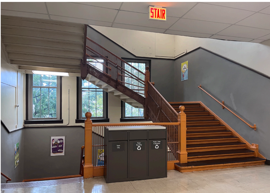
0027. Second floor, typical stair
