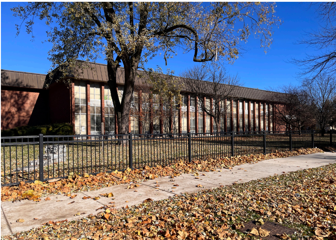
0015. South elevation of 1969 classroom addition, looking northeast
