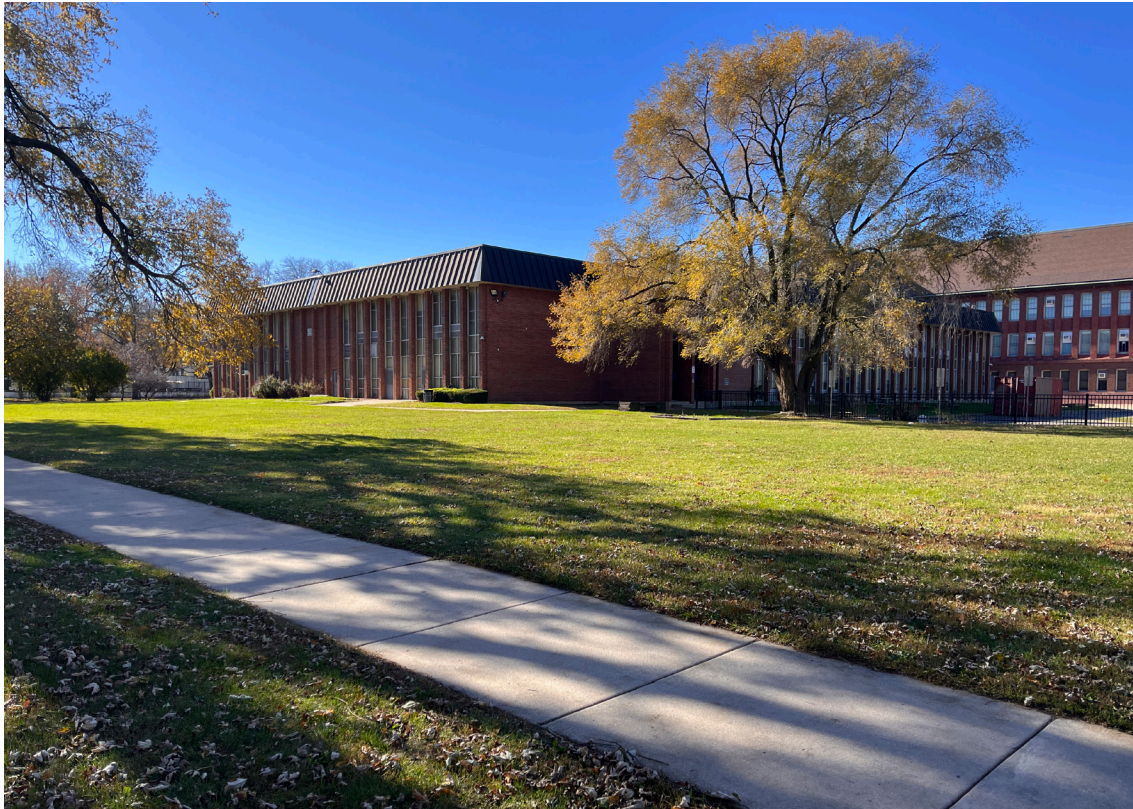
0014. North and east elevations of 1969 classroom addition, looking southwest
