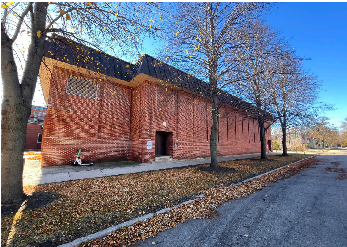
0011. North elevation of 1969 gymnasium addition, looking southwest
