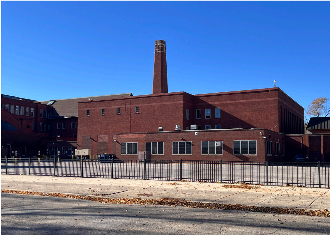
0012. East elevation of main building and 1940 addition, looking west
