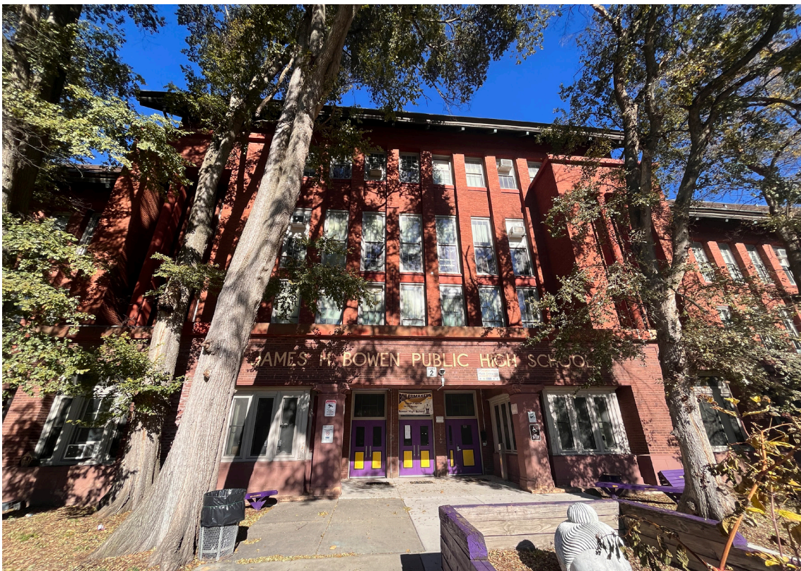
0002. South elevation, center entrance bay, looking north
