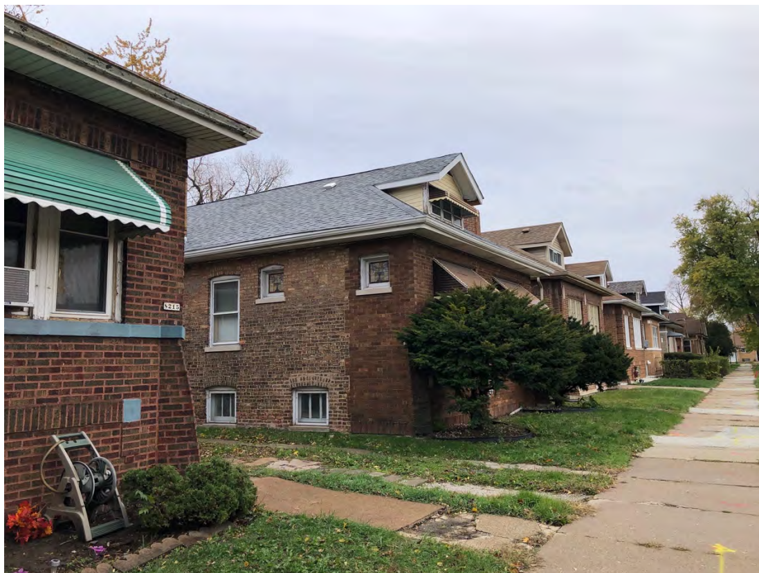
8200 Block S. Kimbark, west side, facing north
