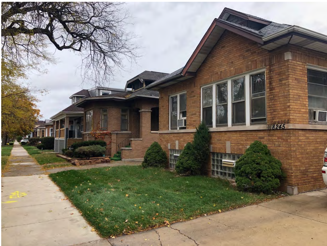
8200 Block S. Dante, east side, facing north
