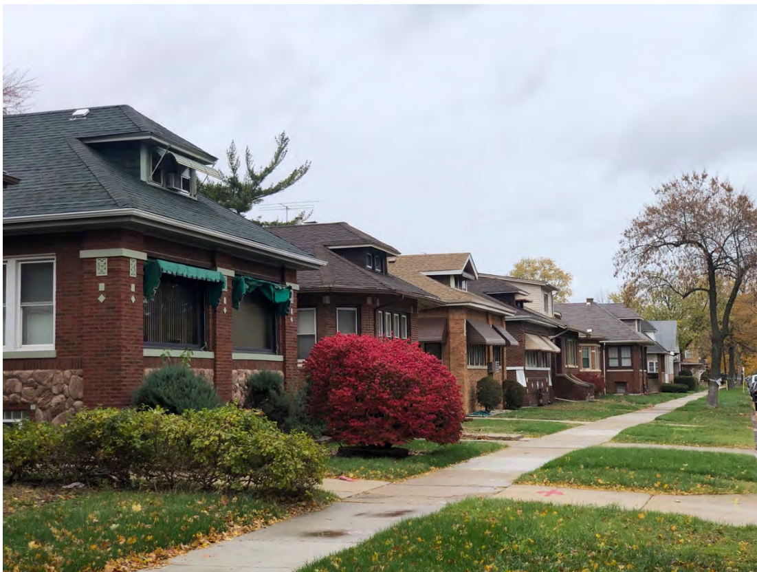
8200 Block S. Dante, west side, facing north
