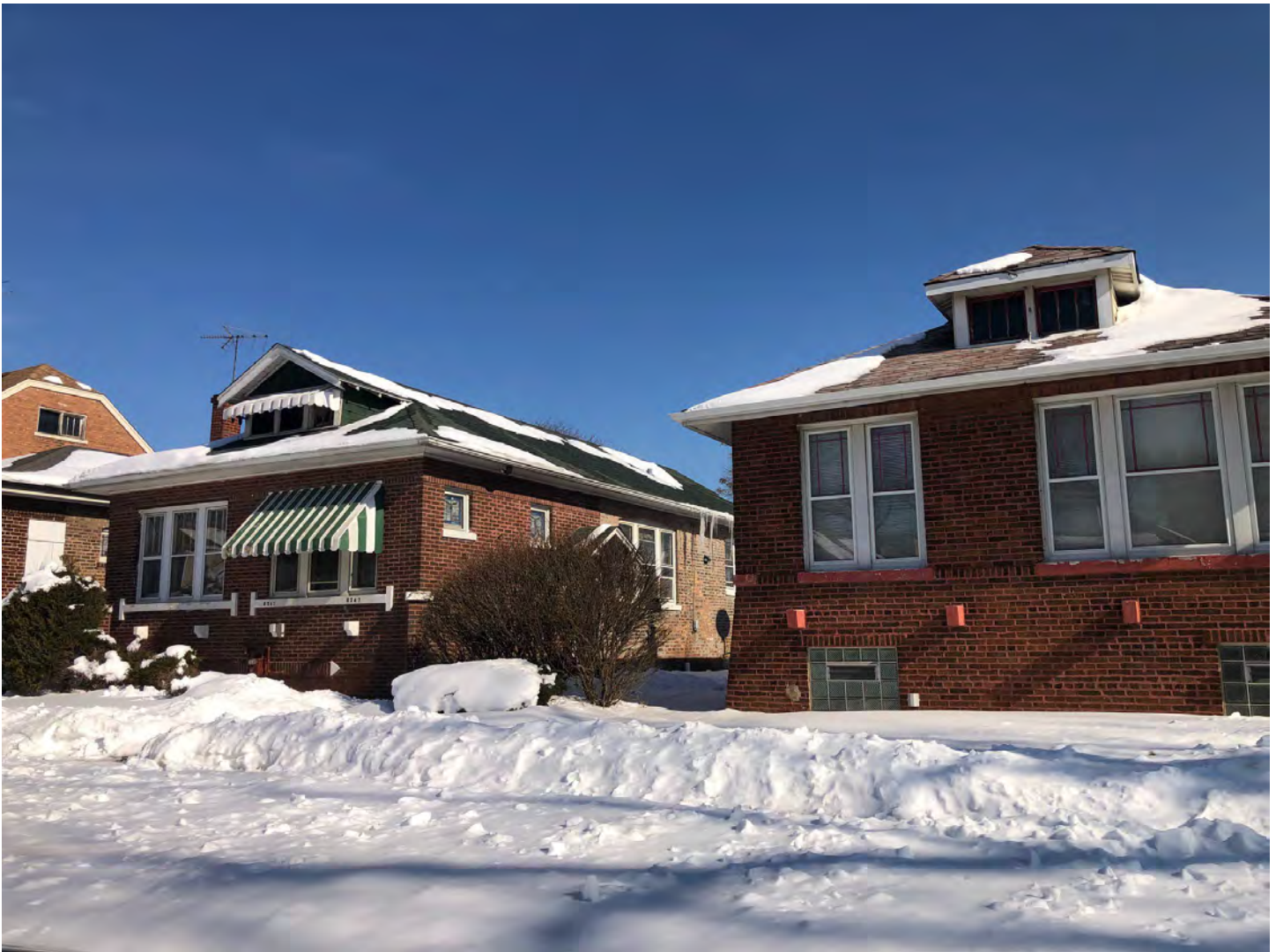
IMAGE 6: Flat bays with side entrances on the 8200 block of S Avalon Street.
