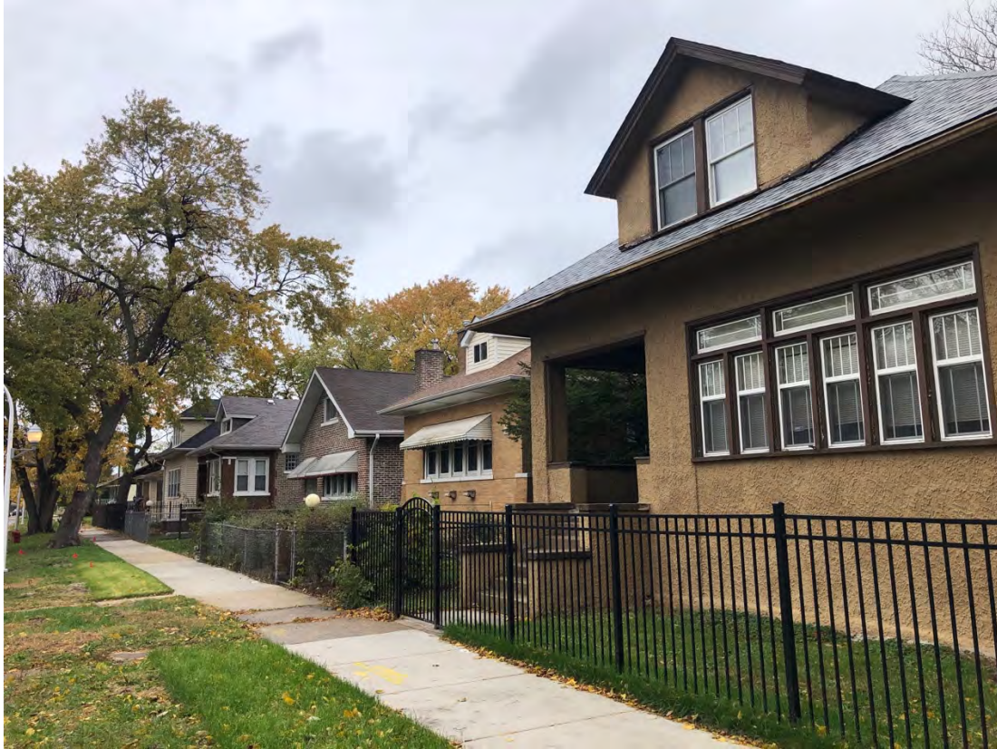
8100 Block S. Harper, east side, facing north
