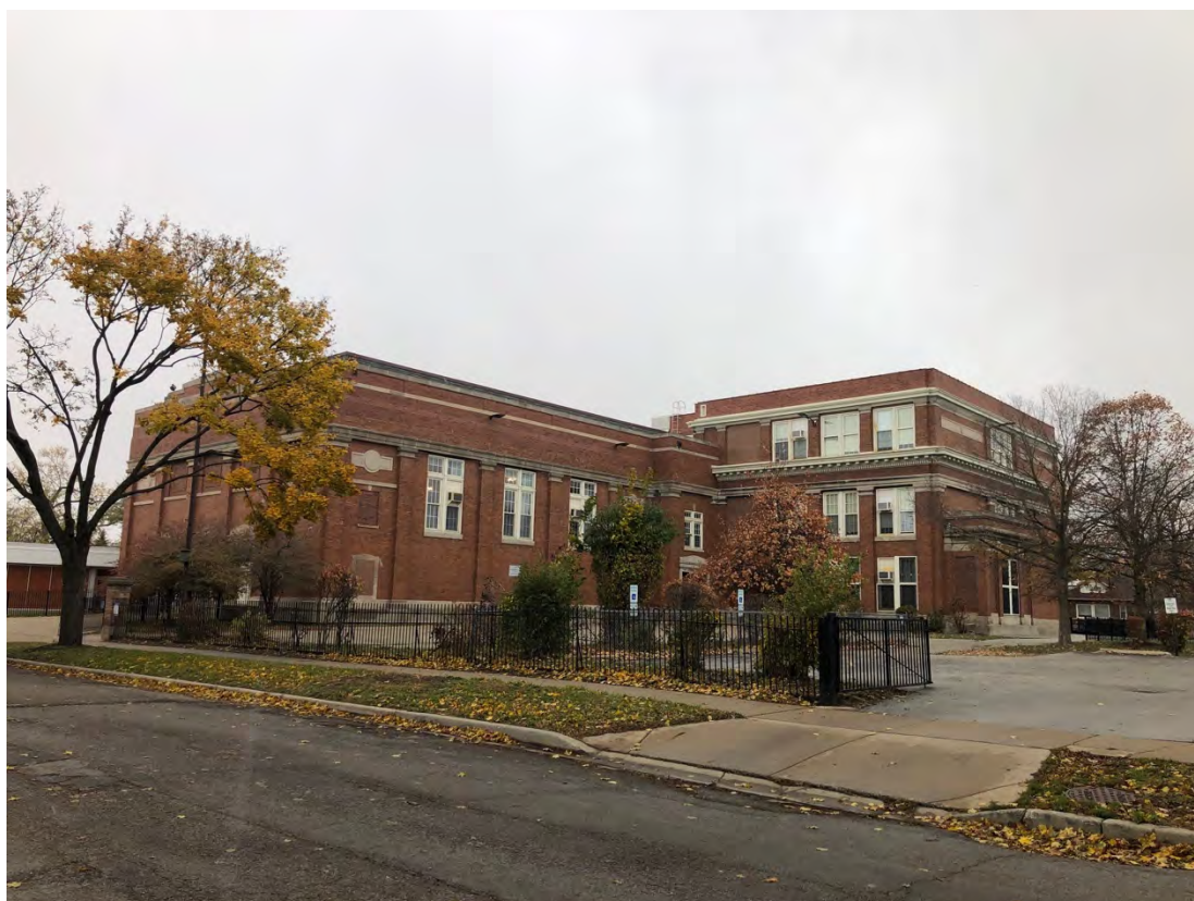
School at 8000 Block S. Dorchester, west side, facing south
