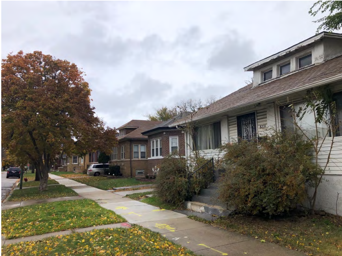
8200 Block S. Harper, east side, facing north
