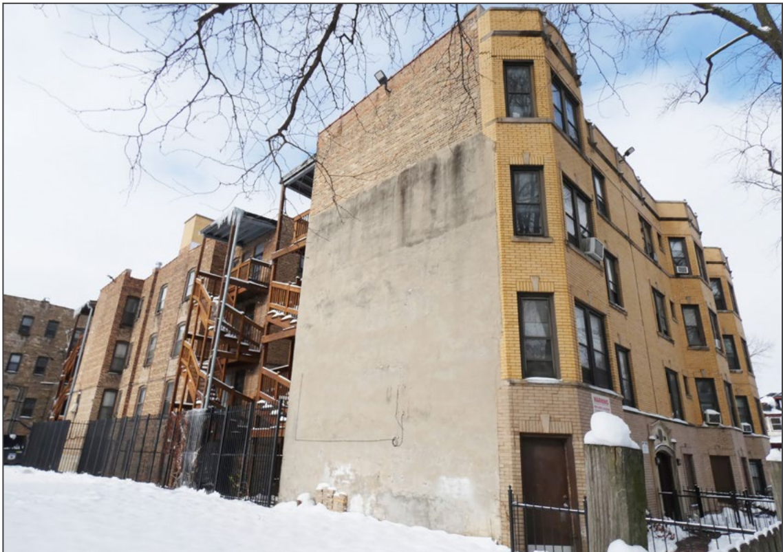
Photo 6. South facade (left) and Long Avenue facade (right), looking northwest.
