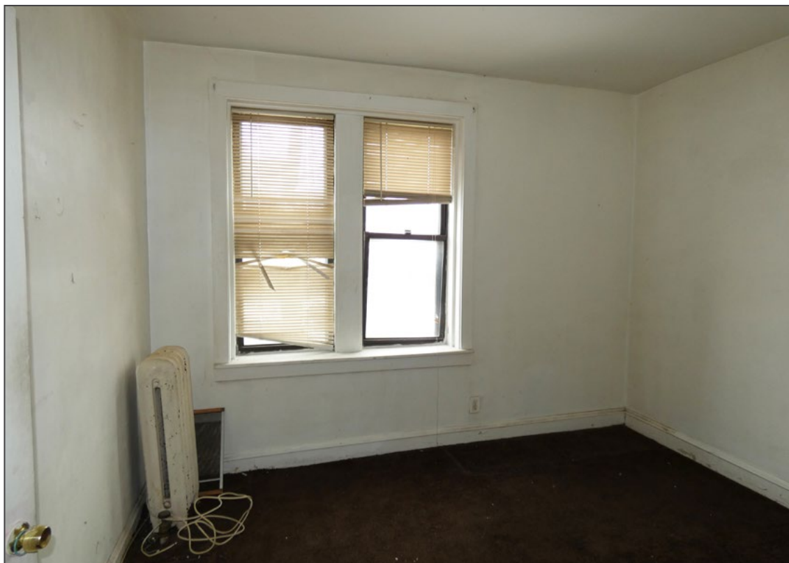
Photo 16. 56-58 N. Long Avenue, typical apartment bedroom.
