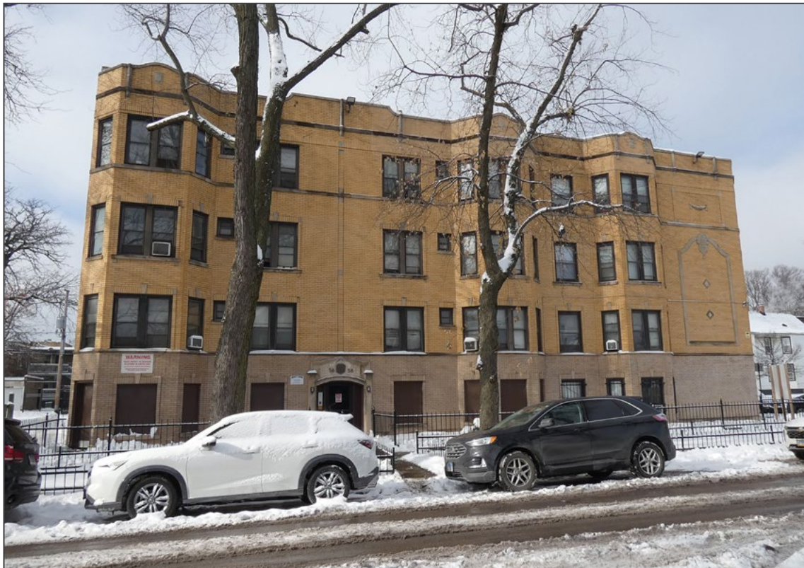
Photo 4. Long Avenue (west) facade, looking west.
