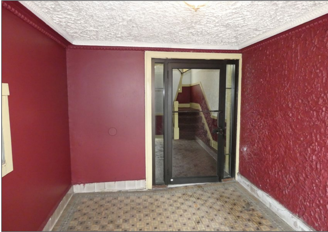
Photo 12. 56-58 N. Long Avenue, 1st floor entrance vestibule, looking west.
