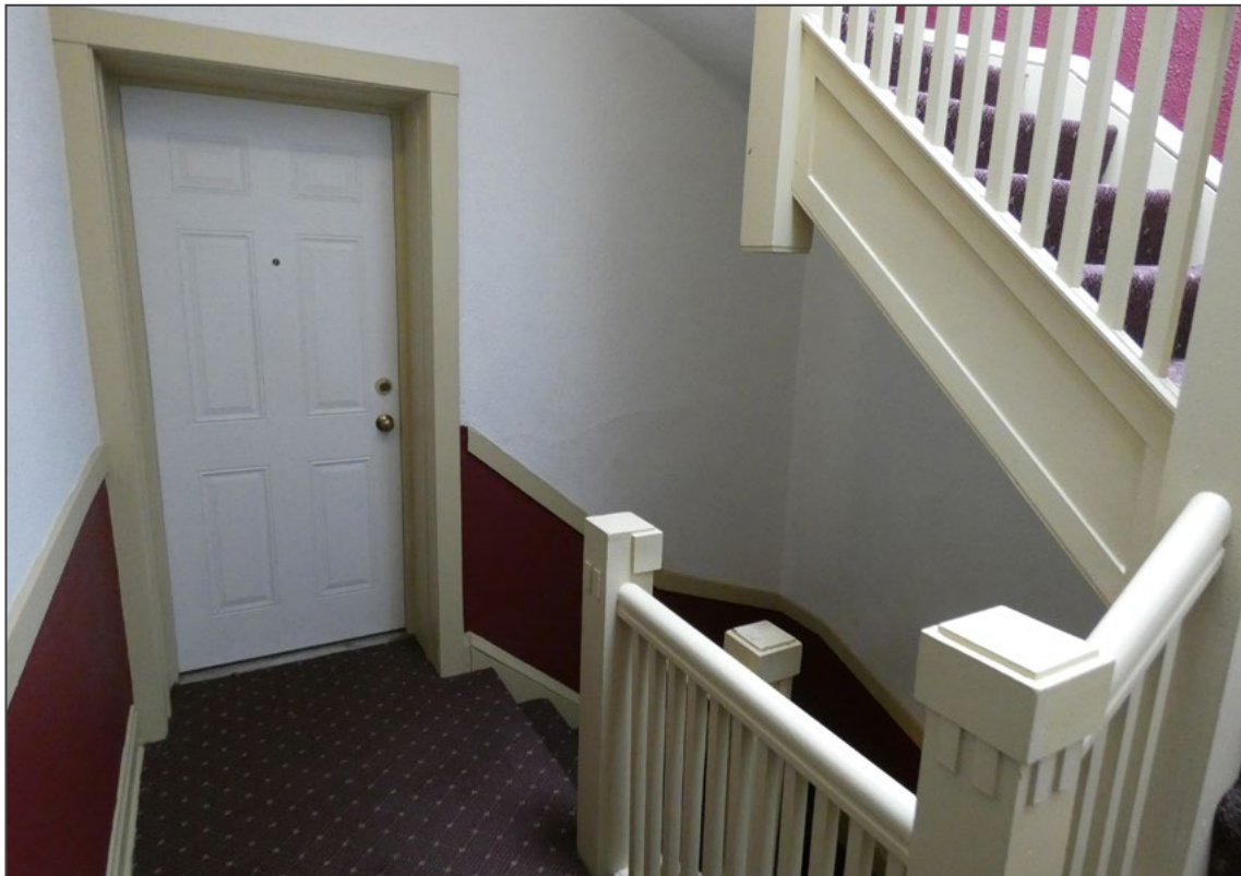
Photo 13. 5409-5411 W. Washington Boulevard, typical upper floor stairwell.
