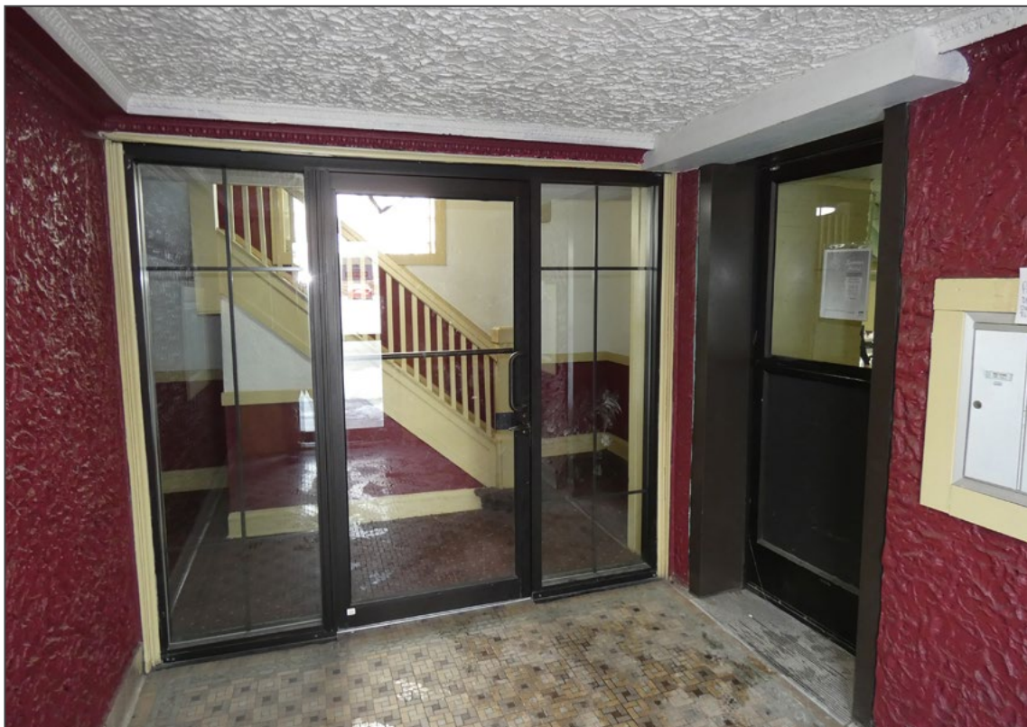
Photo 10. 5401-5403 W. Washington Boulevard, 1st floor entrance vestibule, looking south.
