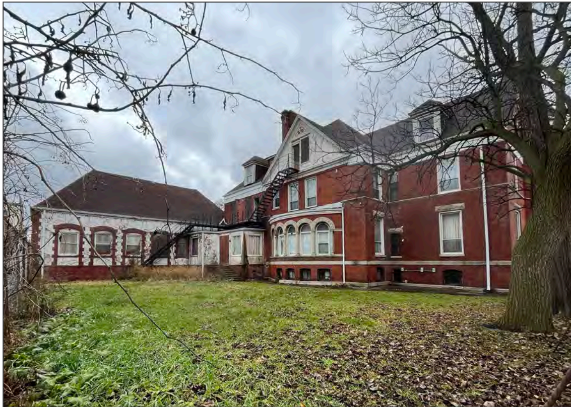
Photo 8. Dormitory (left) and Main House (right), looking northeast from Washington Boulevard.
