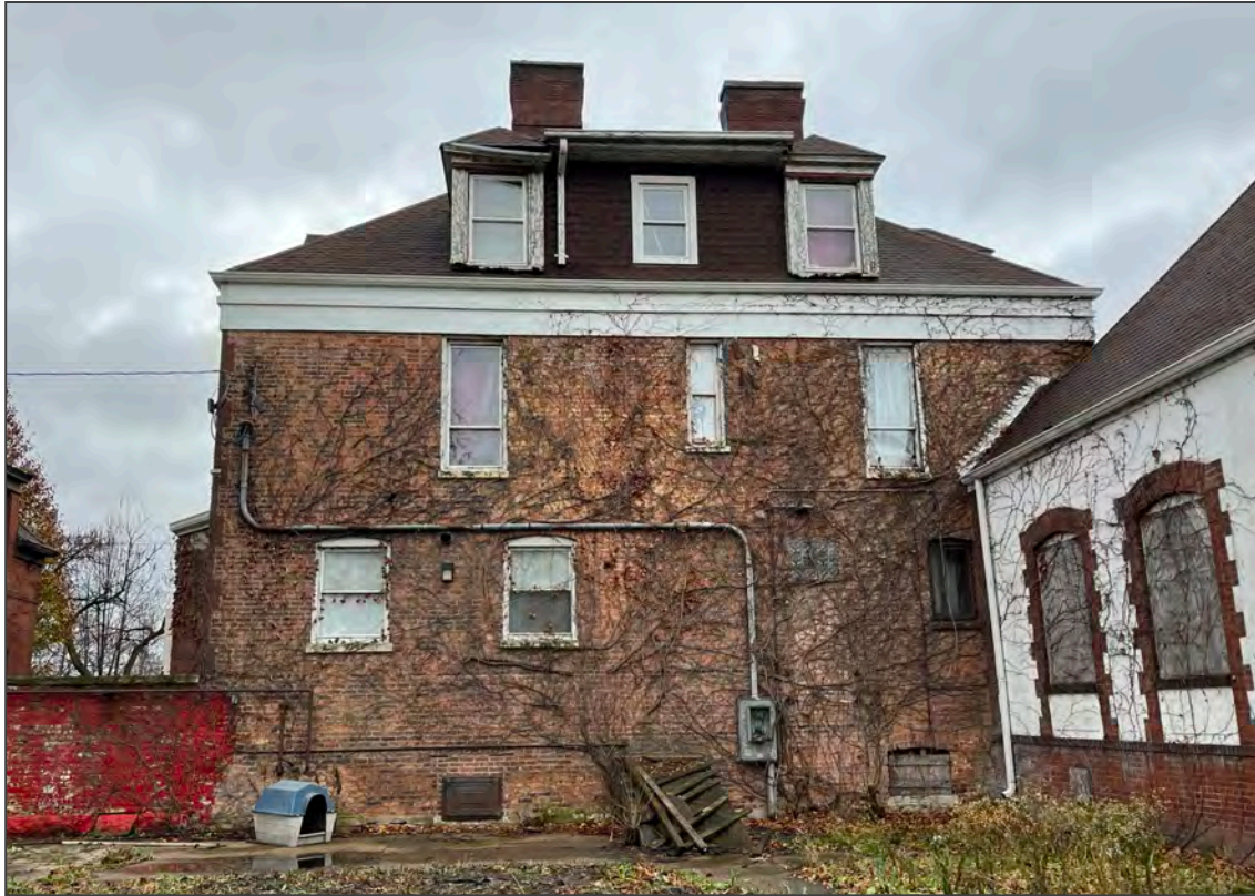
Photo 4. Main House rear (north) facade with Dormitory at right, looking south.
