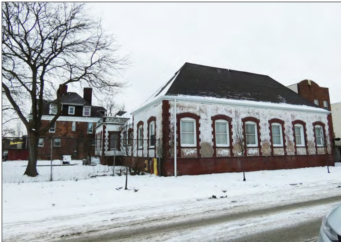
Photo 7. Dormitory north (right) and east (center) facades and Main House south facade beyond at left, looking south from Maypole Avenue.
