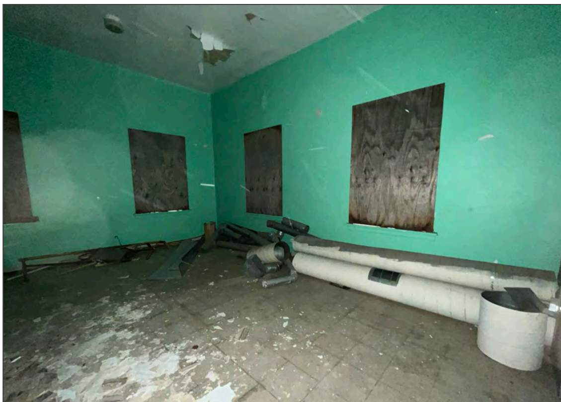
Photo 16. Dormitory room, looking northeast.
