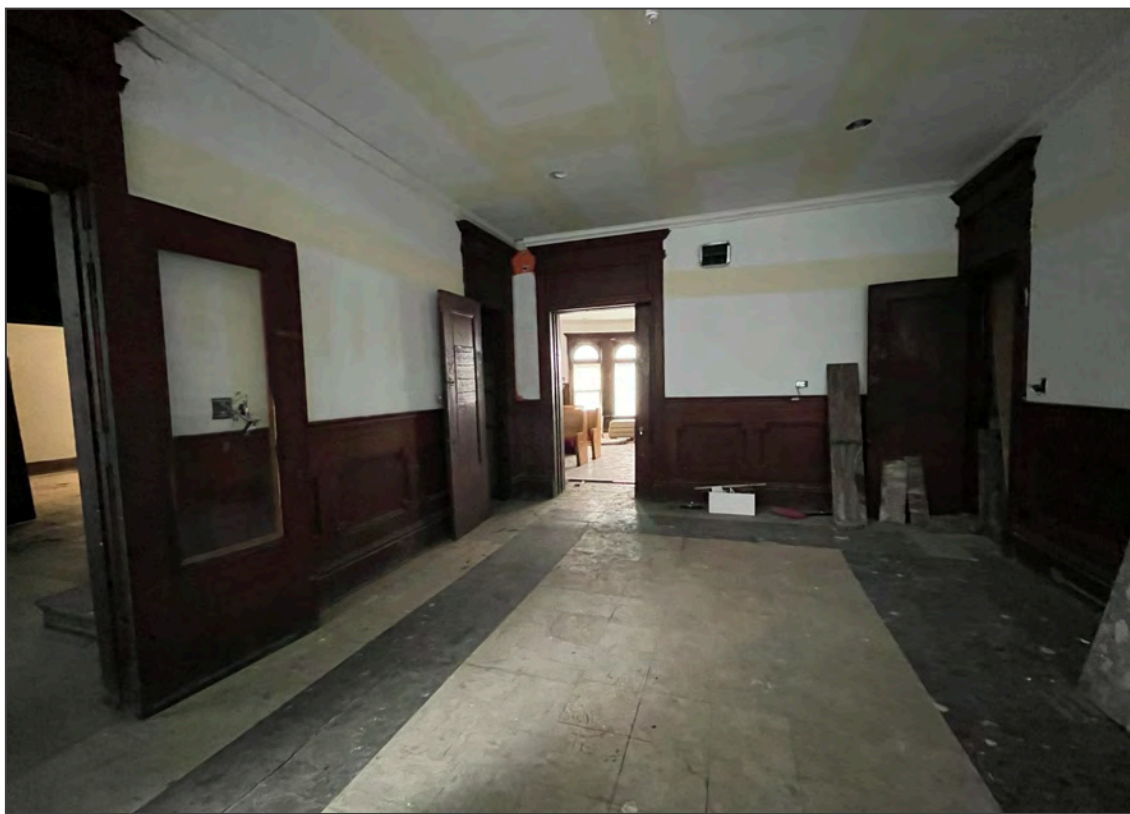
Photo 12. Main House, 1st floor dining room, looking west.
