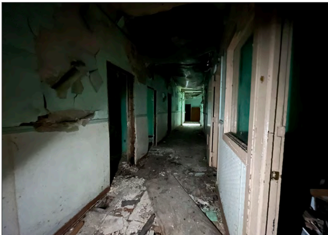
Photo 15. Dormitory corridor, looking north.
