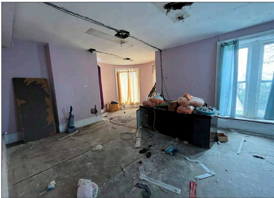
Photo 14. Main House, 2nd floor south bedroom, looking southeast.
