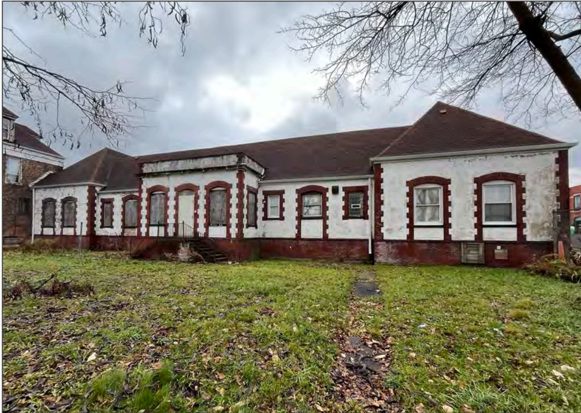
Photo 6. Dormitory east facade, looking west.
