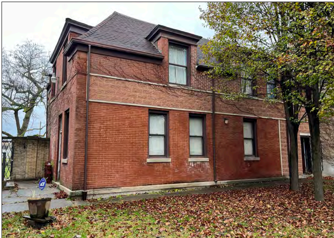
Photo 5. Coach House west (left) and south (right) facades, looking northeast.
