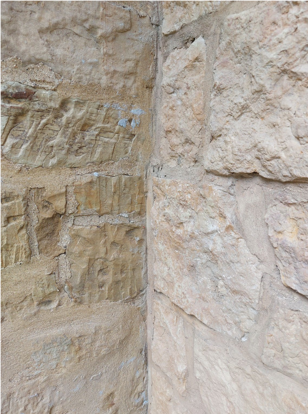
9. Zion Episcopal Church Connection between church and addition close-up Brimfield, Illinois
