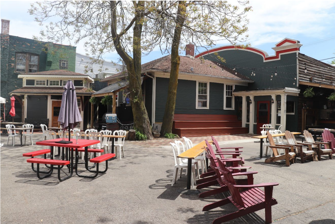
Photo 3: Exterior view of building looking southeast
