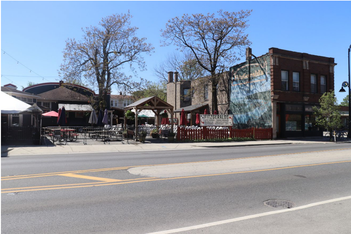
Photo 1: Exterior view of site looking southwest
