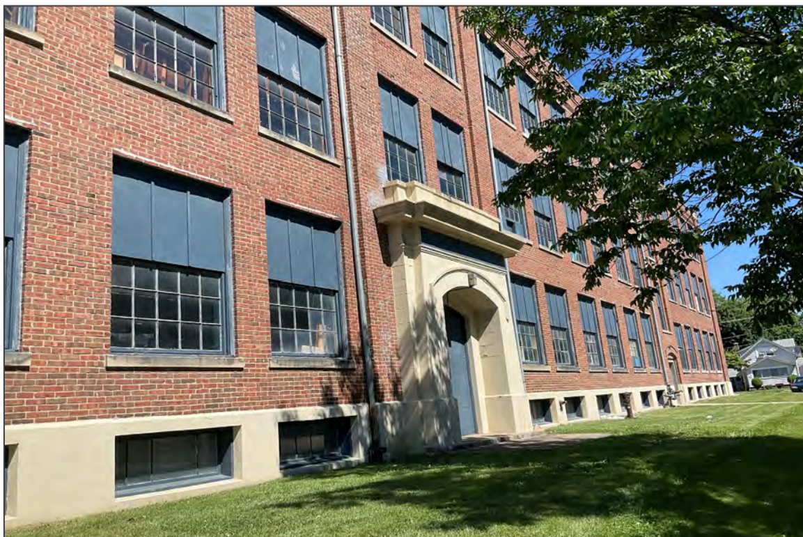
4. East elevation, 1912 block, facing northwest
