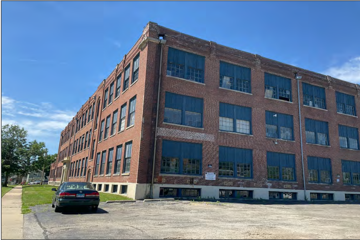
1. North and east elevation, 1917 north addition, facing southwest
