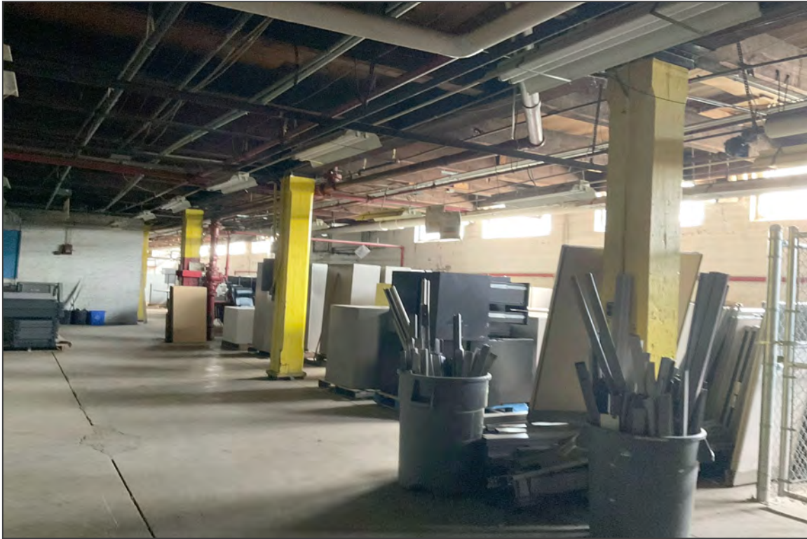
8. Basement, 1912 block, facing northeast
