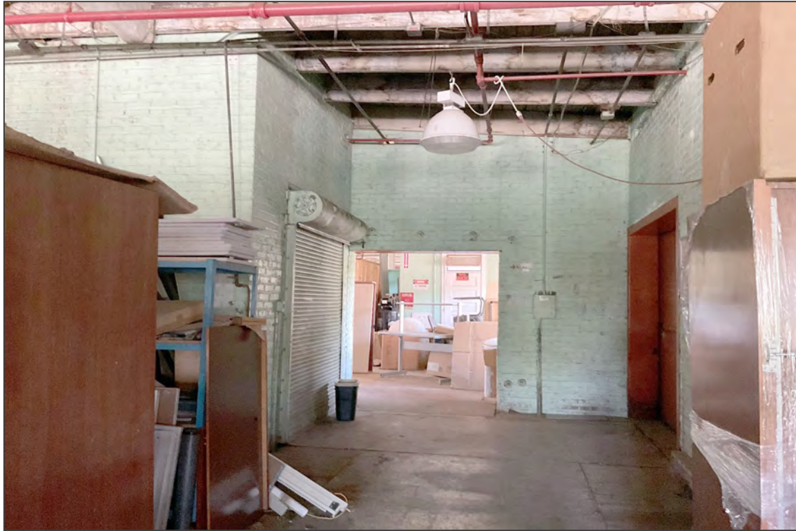
17. Third floor, 1912 block, facing north
