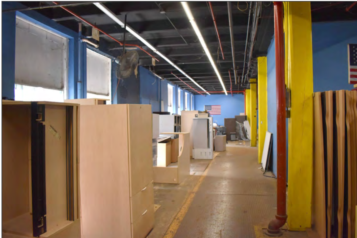
10. First floor, 1912 block – looking southeast.
