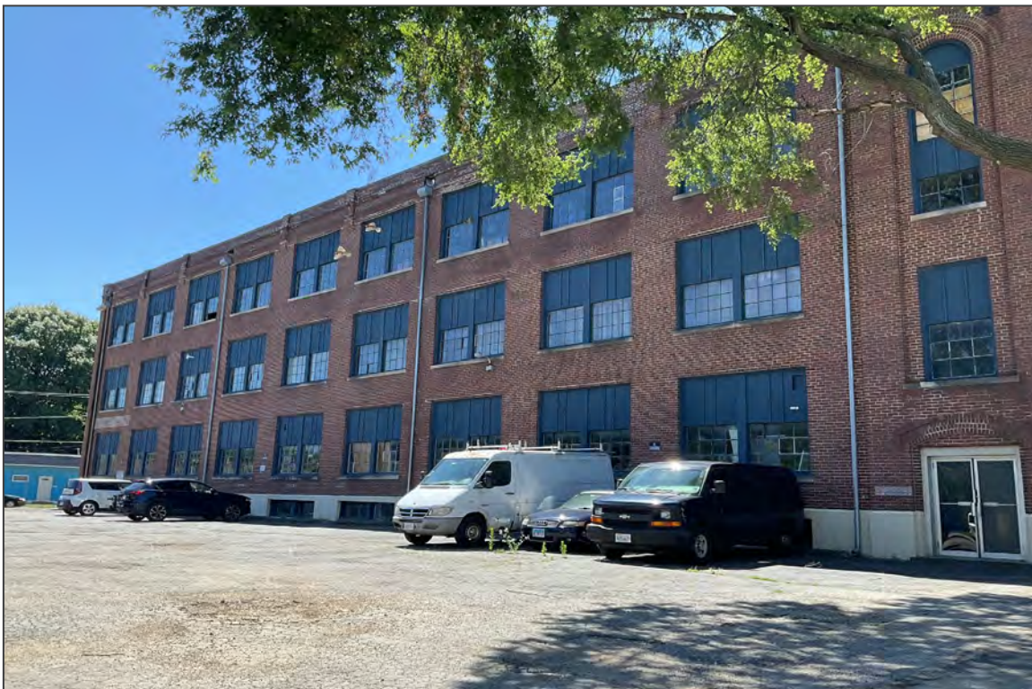
2. North elevation, 1917 north addition, facing southeast
