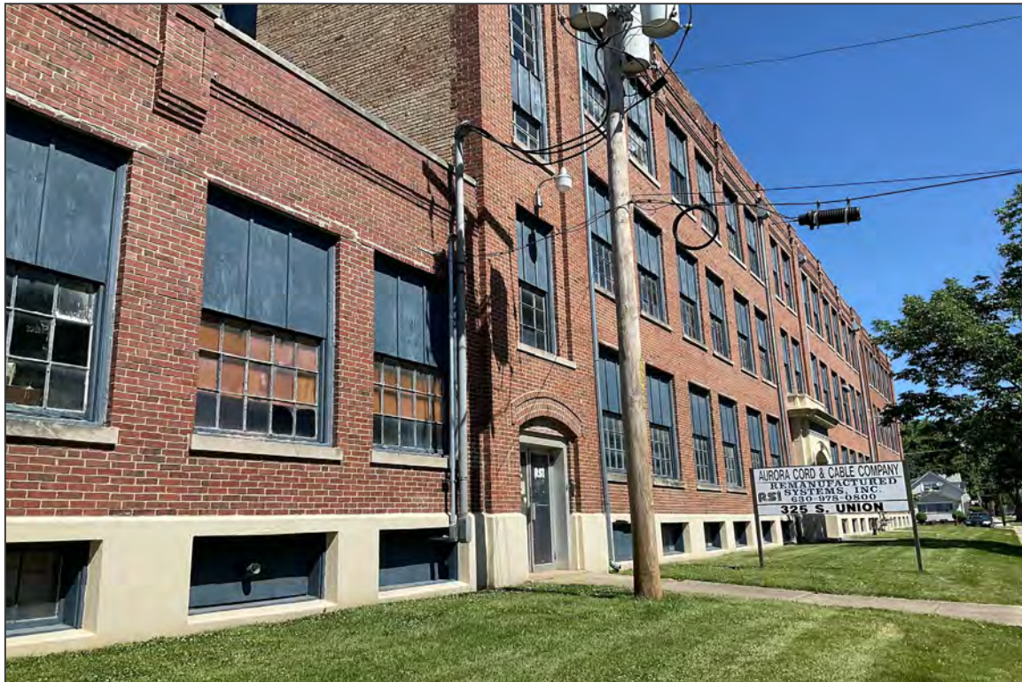
3. East elevation, 1917 south addition (left) and '1912 block (middle), facing northwest
