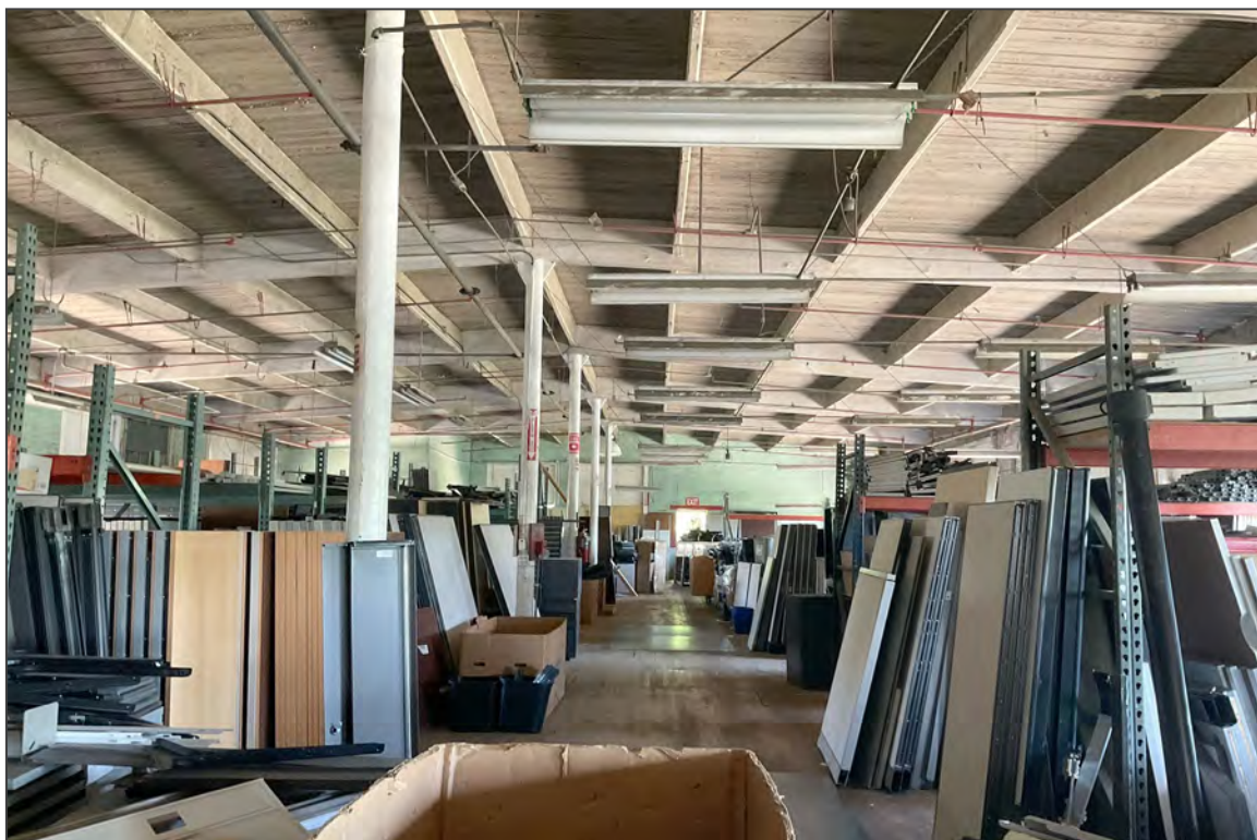
16. Third floor, north 1917 addition, facing west
