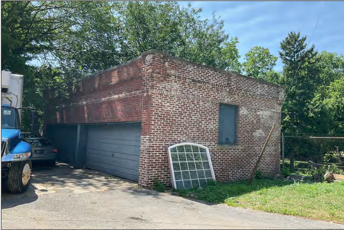
19. Garage, facing southwest
