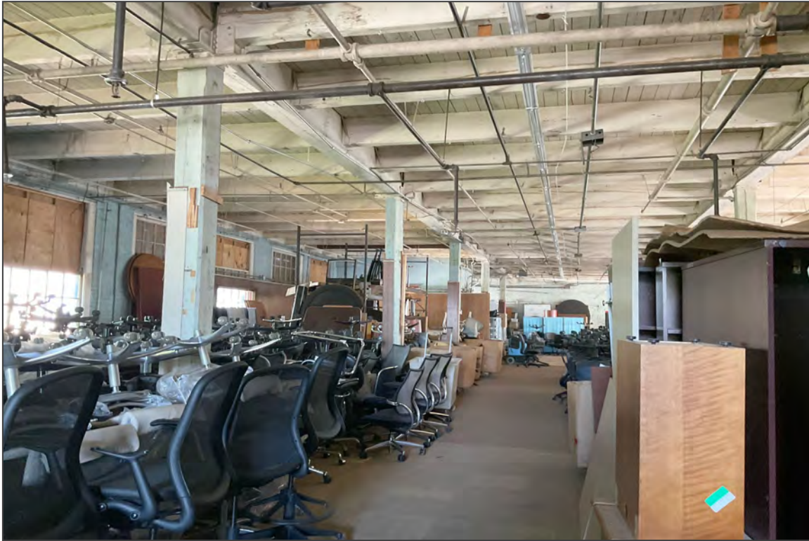
13. Second floor, 1912 block, facing northwest
